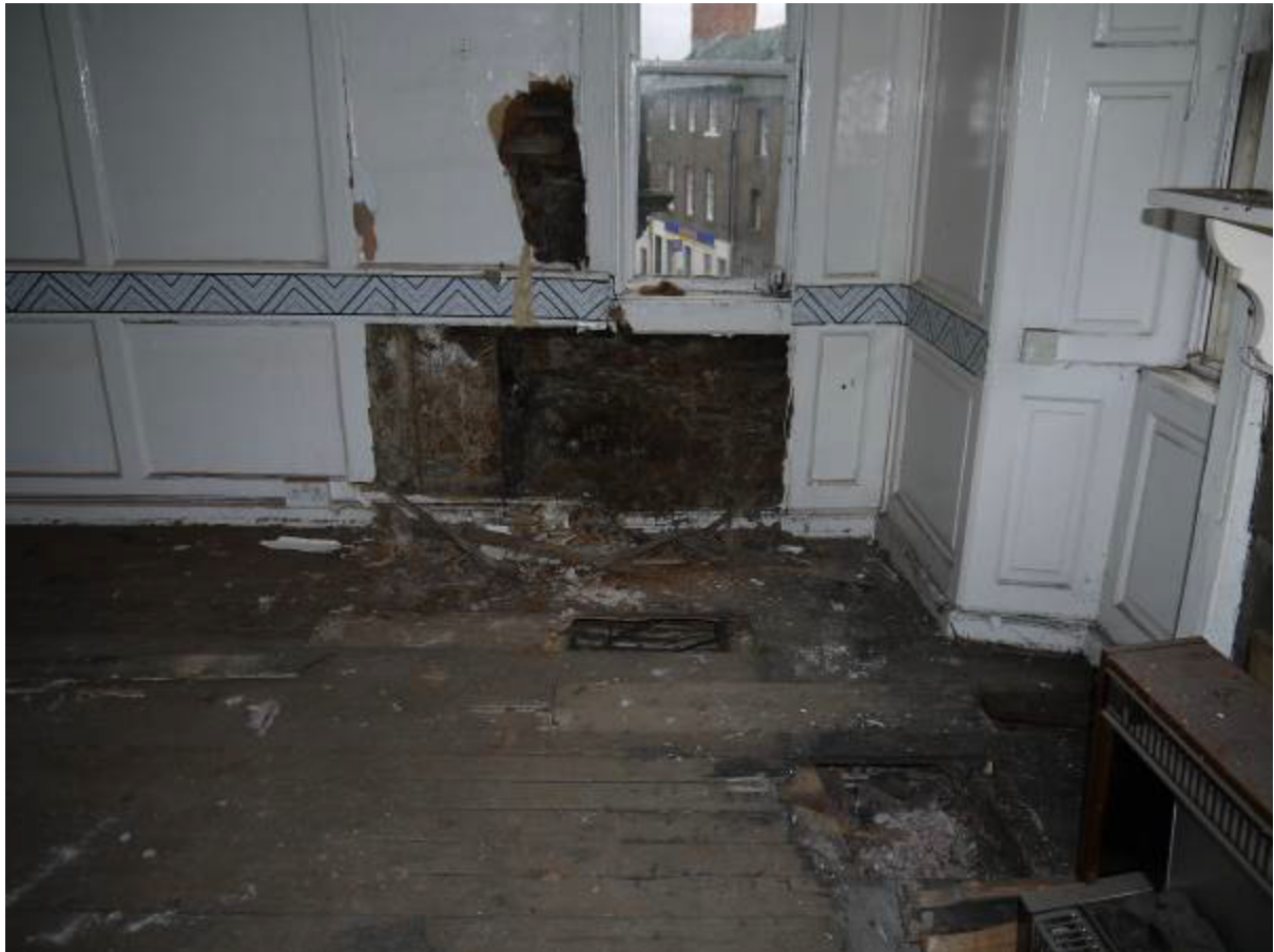
Illustration 29 Detail of junction of wall of neighbouring Episcopal church and frontage of no 47 High Street
