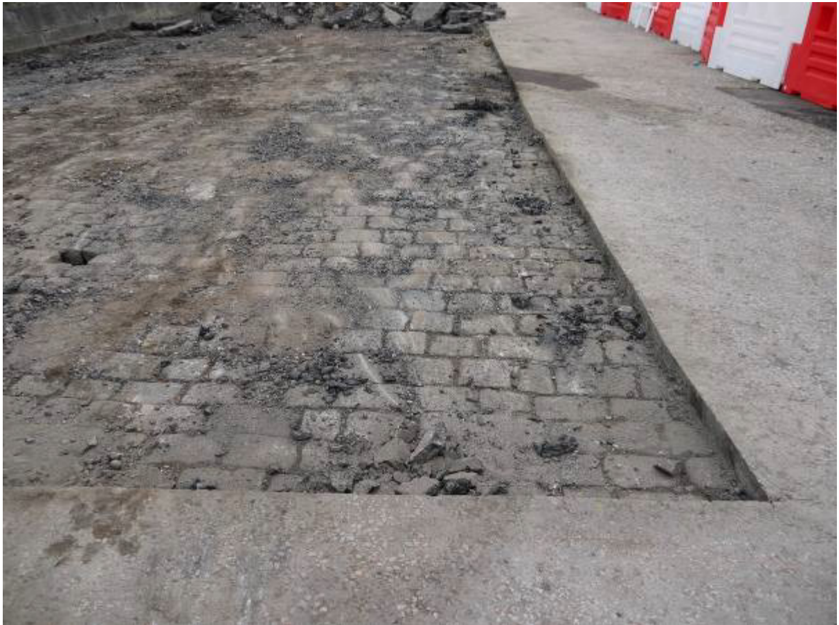
Illus 18 Setts revealed after removal of tarmac
