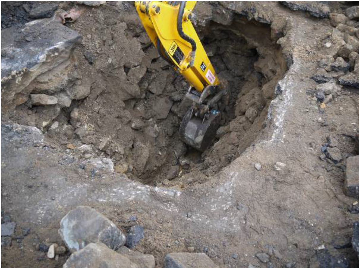
Illus 13 Excavation of engineers test pit (17 on Illus 5), digger bucket is resting on sandstone bedrock
