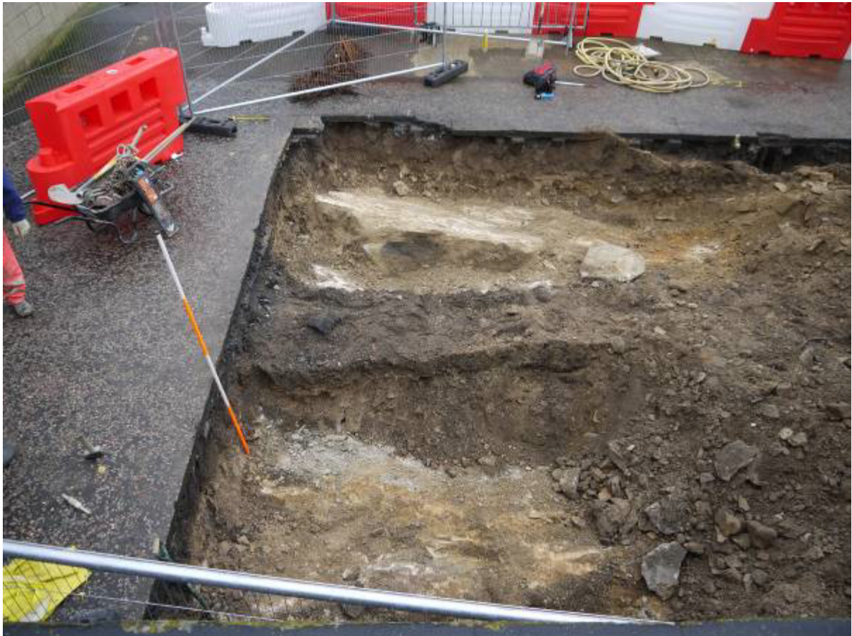
Illus 20 Sandstone bedrock visible at proposed location of pits 1 and 2 looking West from pier wall
