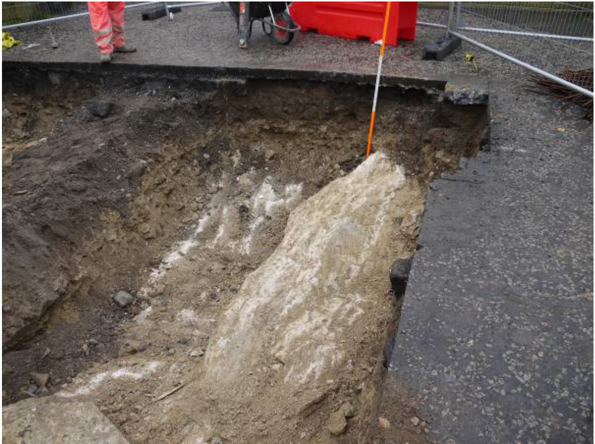
Illus 19 Sandstone bedrock revealed at proposed location of pit 2
