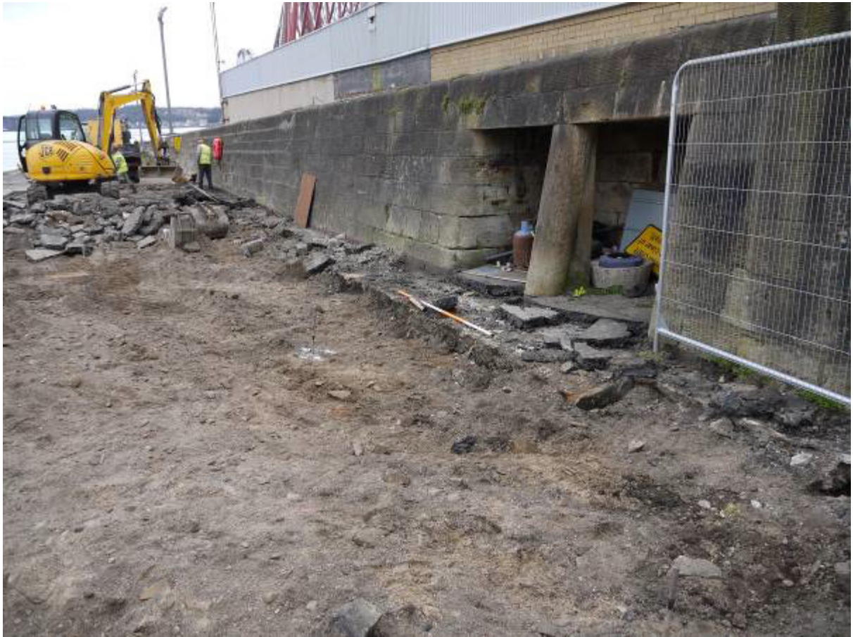
Illus 17 Wider sandstone foundation in front of alcove in pier wall
