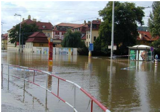
Fig. 2. The flood of Prague in August 2002. Buildings of the Institute in the centre, an entrance to the Prague Metro, fully flooded, in the right. Photo by J. Frolík.
