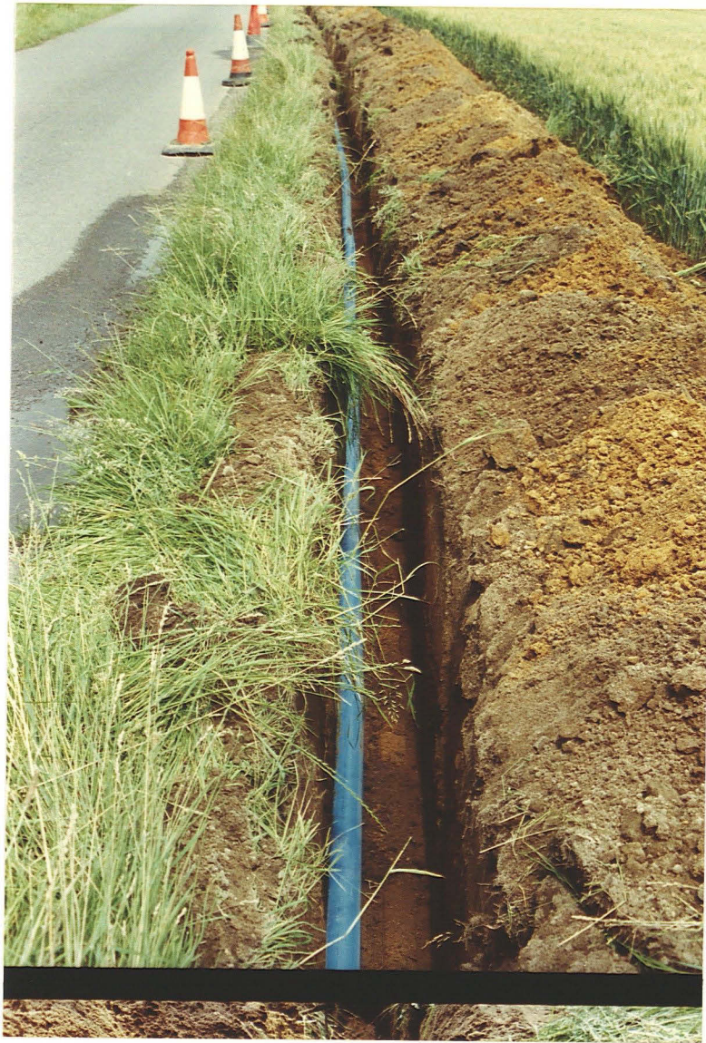
Pl. 18 Sand layer visible in trench base, Trench 43 (looking north).
