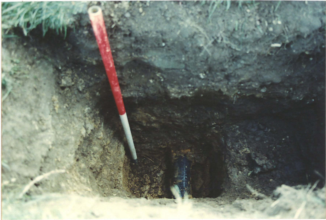
Pl. 5 Existing water main, Trench 3.
