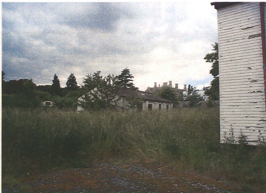
Plate 3 - The former hospital from the north- west corner of the site with Nocton Hall in the background
