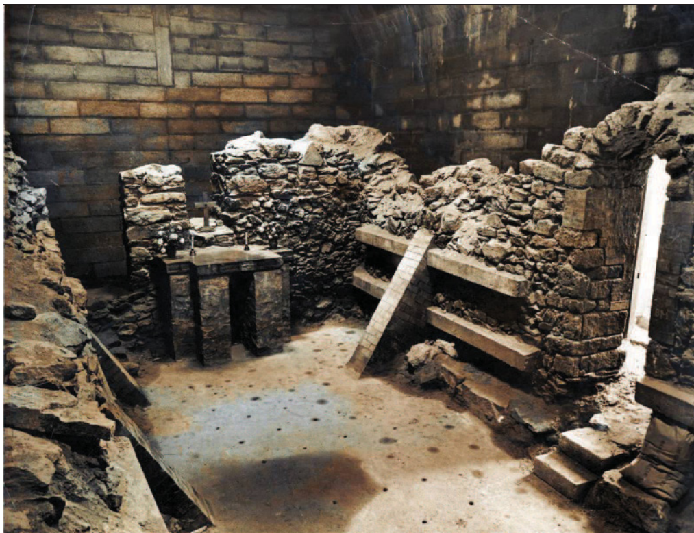
Fig 21 The interior of St Piran's Oratory. Not dated. Shows concrete floor, brick buttresses, rebuilt doorway and wall supports..
