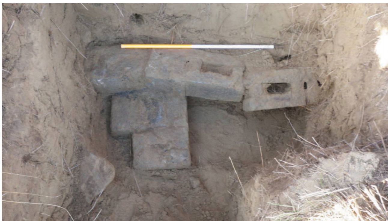
Fig 30 Photograph of Trench 1 showing revealed concrete blockwork of oratory 'shell'
