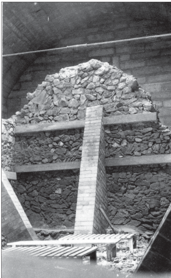
Fig 22 Inside face of west wall and exterior of north wall of St Piran's Oratory. Not dated. Illustrates the survival of the west gable wall and the impact of buttresses. Duckboards suggest that the floor was waterlogged at the time.
