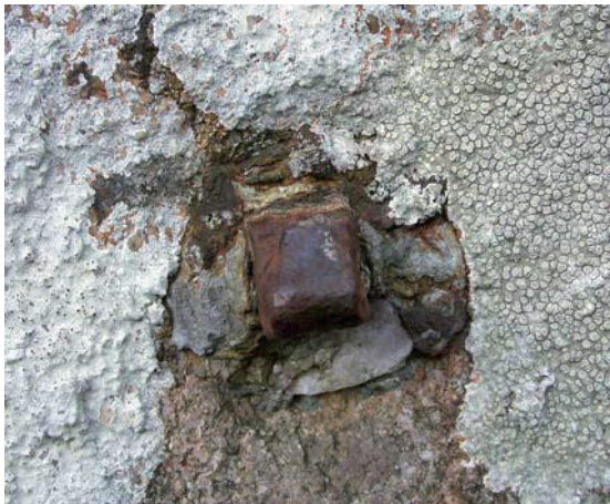
Fig 5 The condition of the stone: two views of both the upper and the lower gate-hangings
