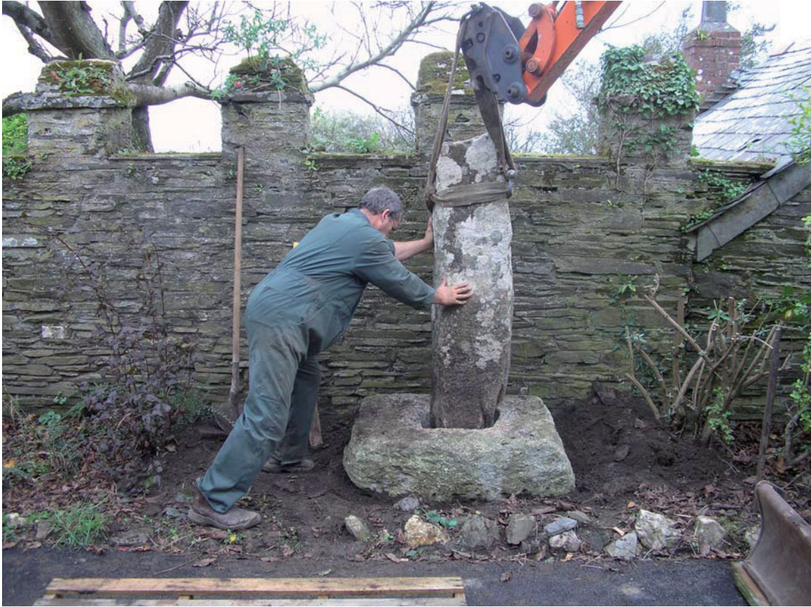
Fig 11 Restoring the stone on the verge at Trethevey
