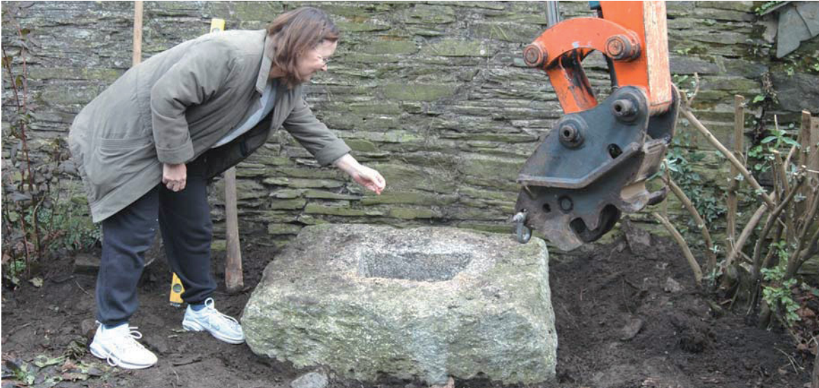
Fig 10 The new base: selecting, installing and putting dating evidence in the mortice
