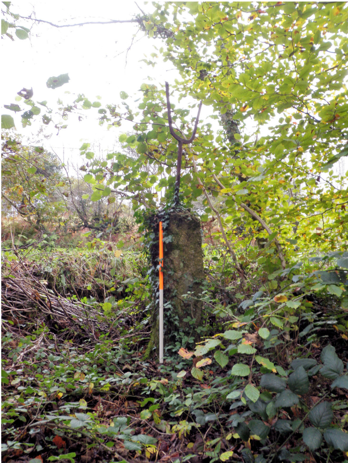
Fig 20 An old signpost – a granite pillar with wrought iron support for a wooden sign (located above the riverbank on the east side of Draynes Bridge)
