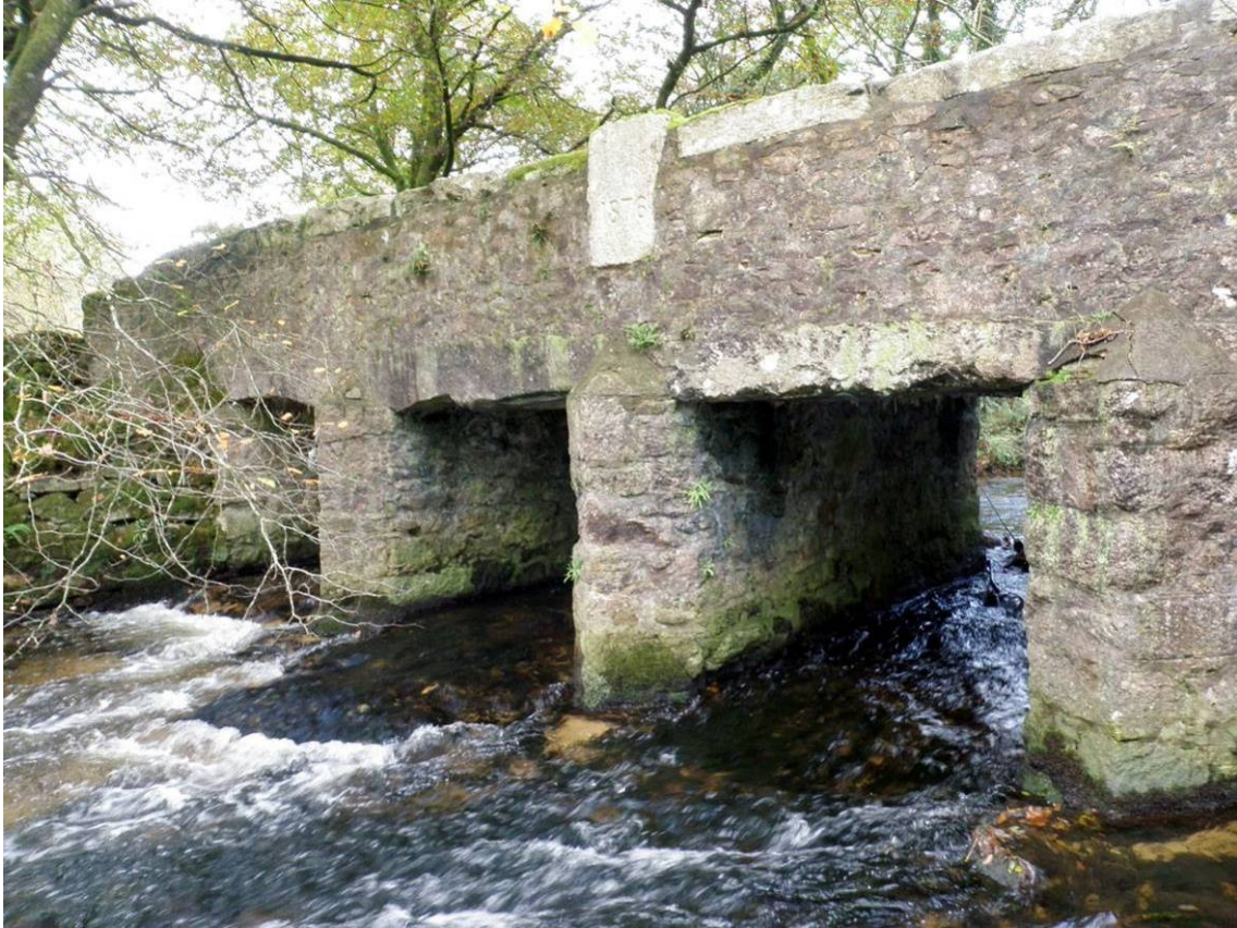
Fig 12 Draynes Bridge from the south (downstream side)
