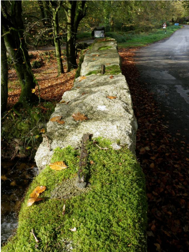
Fig 15 Rough granite coping stones fastened with iron cramps on south parapet
