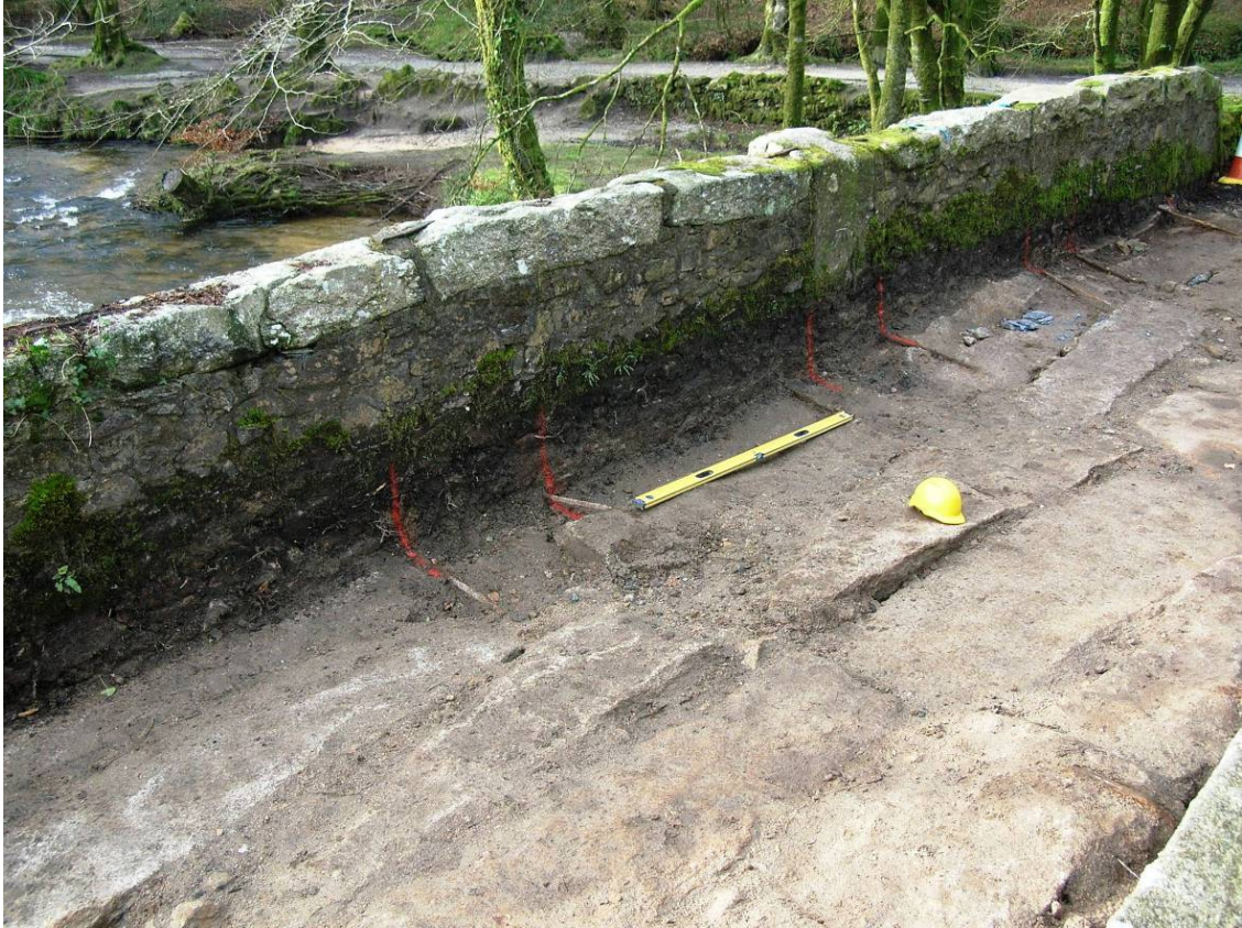
Fig 22 Draynes Bridge after removal of the road surface, January 2013 (looking SW)
