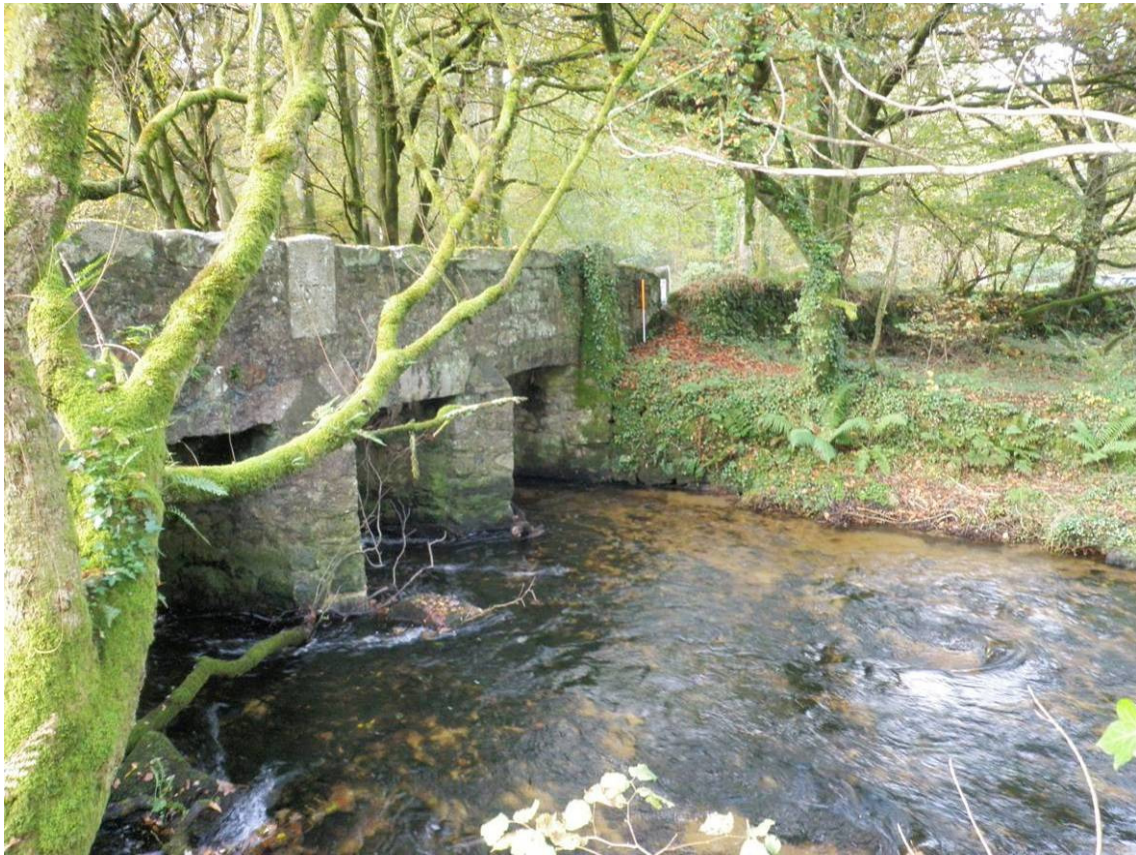
Fig 13 North (upstream) side of Draynes Bridge
