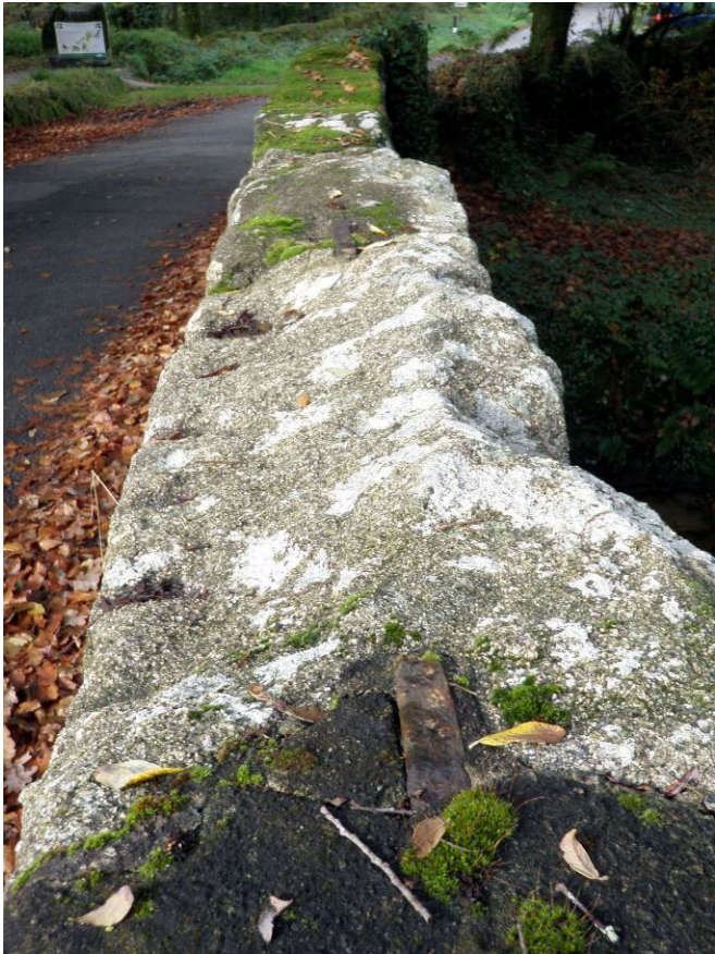
Fig 16 Rough-hewn granite coping stones on north parapet
