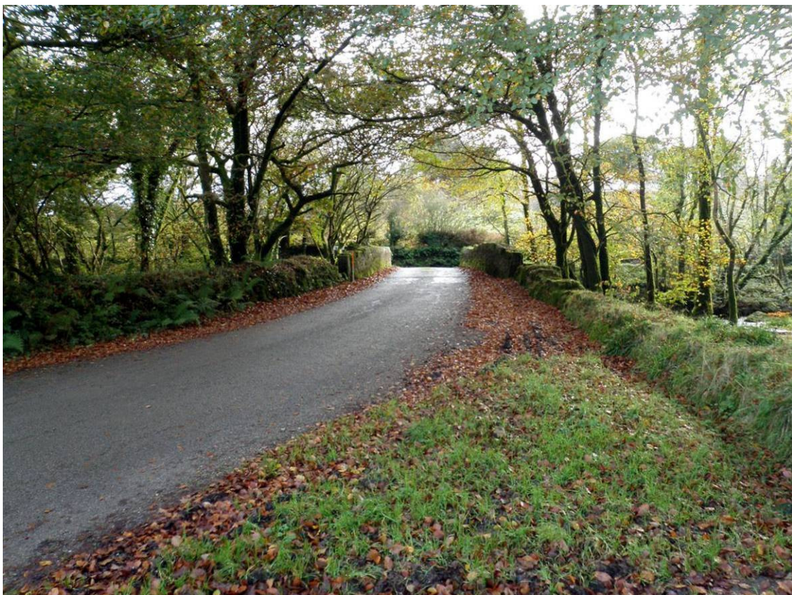
Fig 10 The approach to the bridge from the west
