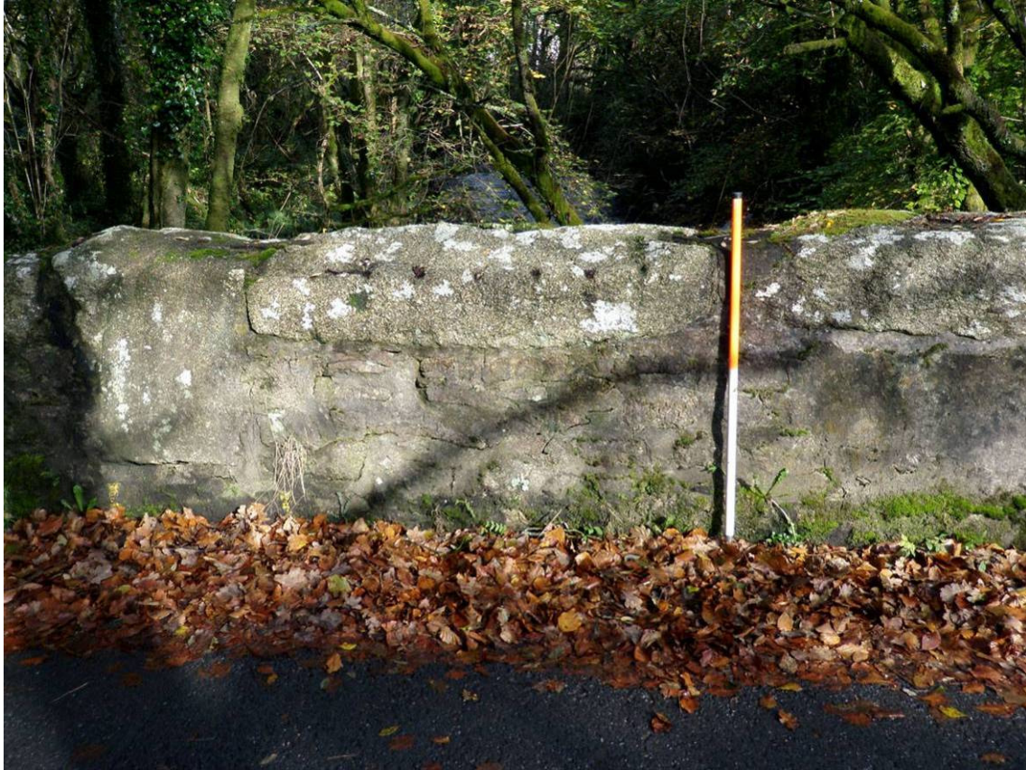
Fig 17 Rough-hewn granite coping stones on north parapet Drill marks (indicating 19 th century tare-and-feather splitting) are clearly evident
