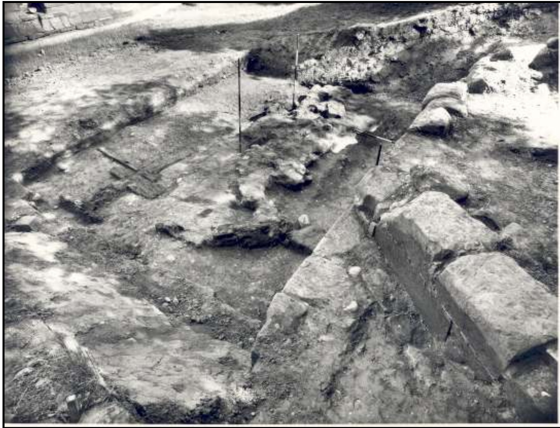
Fig. 3.12: The Northwest Bridge and West Abutment, looking southeast (Scan 126)
