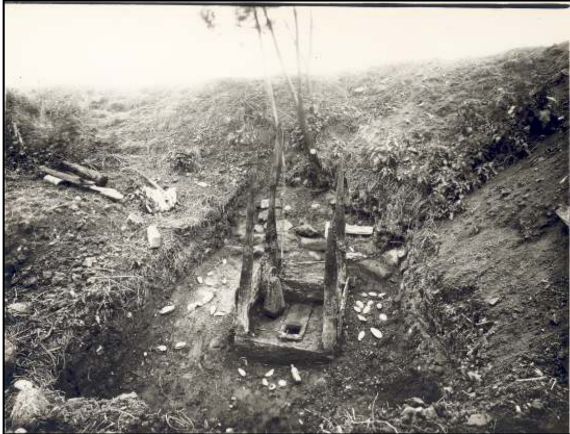
Fig. 3.03: The sluice, looking ? (Scan 957)
