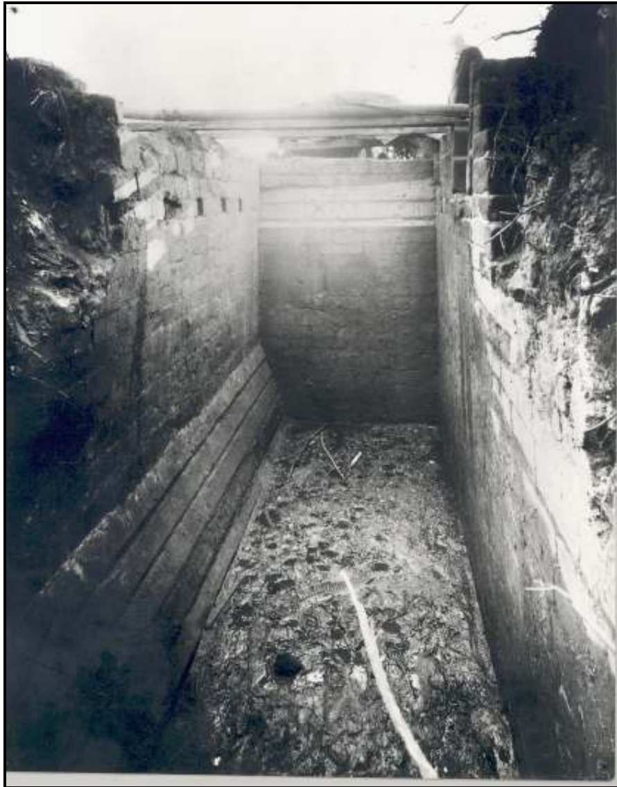
Fig. 2.18: The West Cellar, looking south (Scan 127)
