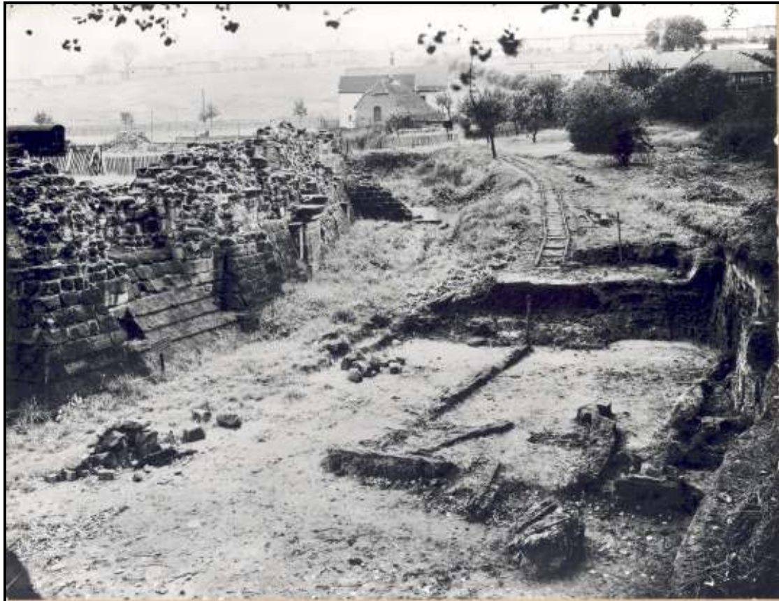
Fig. 3.02: The timber bridge at the Gatehouse Tower, looking south (Scan 953)
