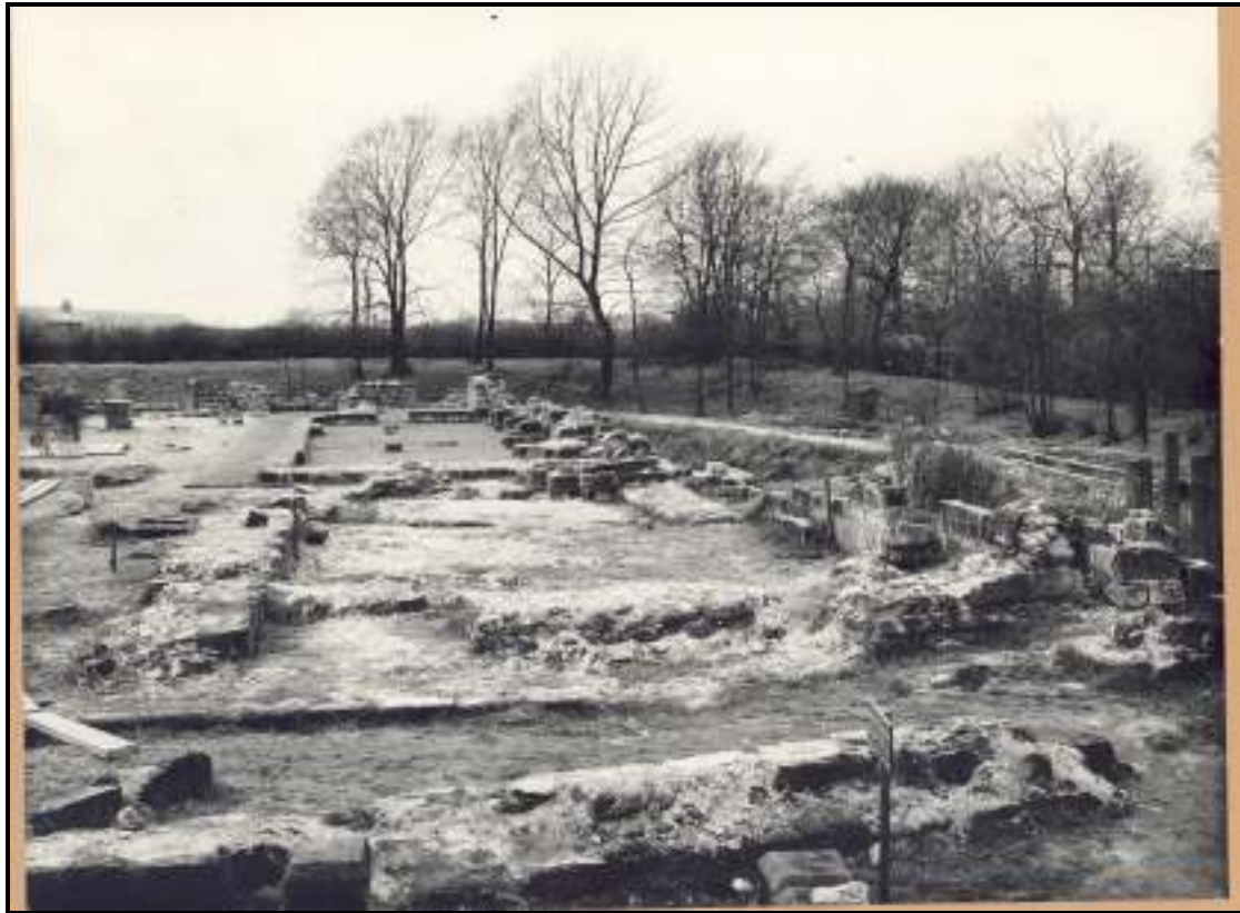
Fig. 2.15: The Chapel, looking west (Scan 944)
