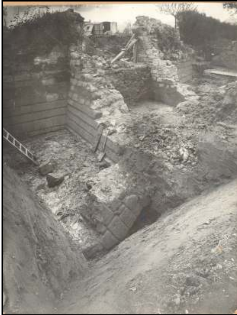
Fig. 2.8: The West Tower, looking southeast (Scan 912)
