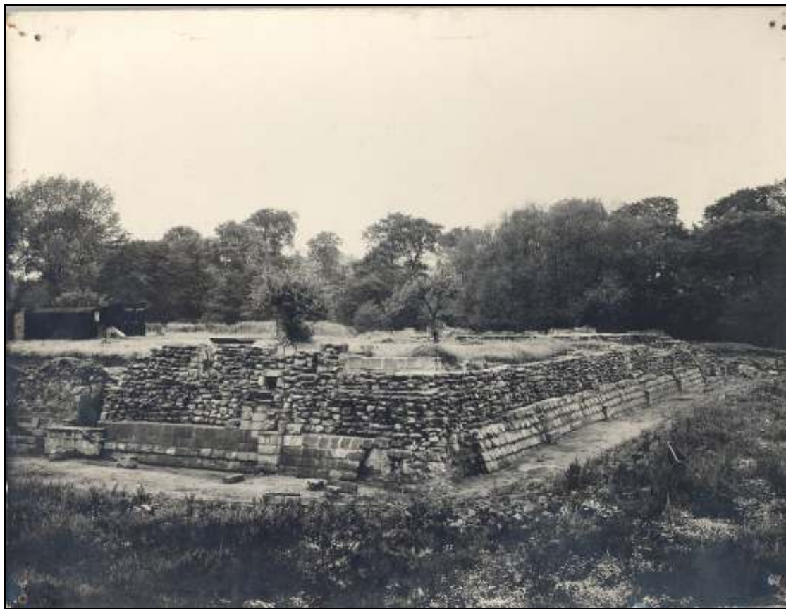
Fig. 2.10: The southeast corner, looking northwest (Scan 132)
