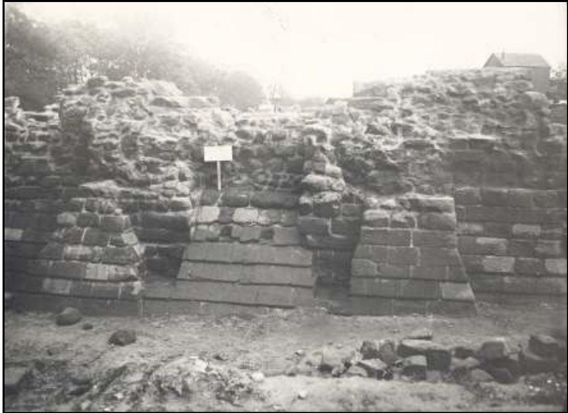
Fig. 2.6: The Gatehouse façade, looking east (Scan 931)
