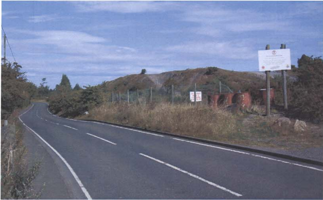
Plate 3. The pit heap, from the southern approach, looking NNE.
