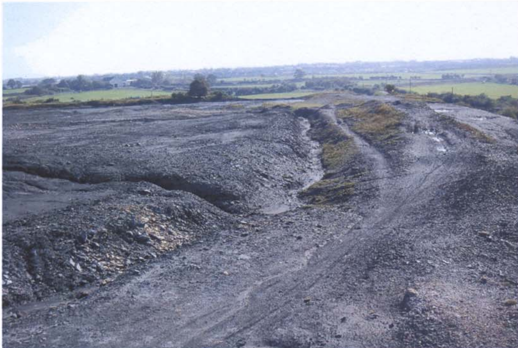
Plate 19. View along the top (south-west side) of the pit heap, looking south.
