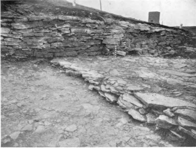
A. JUNCTION OF ORIGINAL END OF S. WALL WITH THE LATER ADDITION. NOTE ALSO THE PAVINGS OF Floor II ON THE LEFT, AND Floor I ON THE RIGHT ABOVE IT
