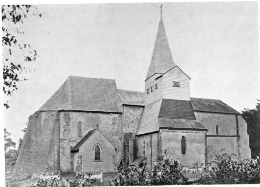
A. Photograph taken before the 1871 restoration, from the north
