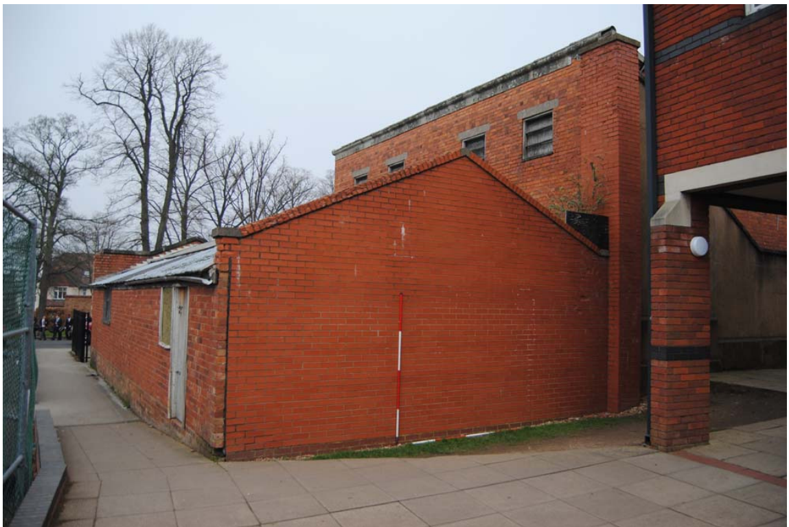
Plate 19: Store building (former firing range); south elevation in new brick, related to shortening of range in 1996. Note vent openings to upper west elevation of fives court wall (two per court).
