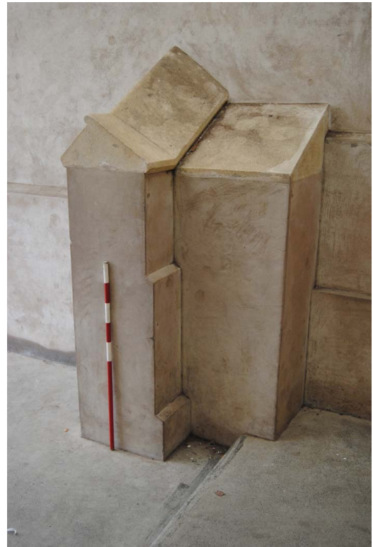
Plate 11: Court 2; buttress or 'pepper-box' to left hand wall, note trap or 'dead man's hole' at base.
