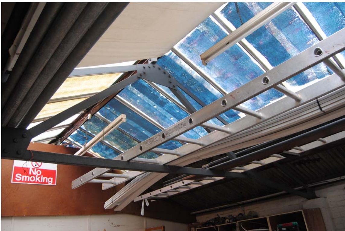
Plate 24: Store, interior; detail of steel roof truss.
