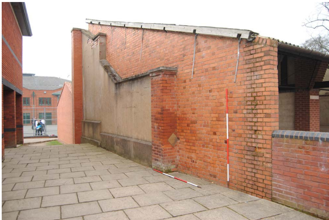
Plate 4: Oblique view of south elevation showing relic features of 'right hand' wall of former court. NB. plaque to brick pier (see Plates 5 and 6)
