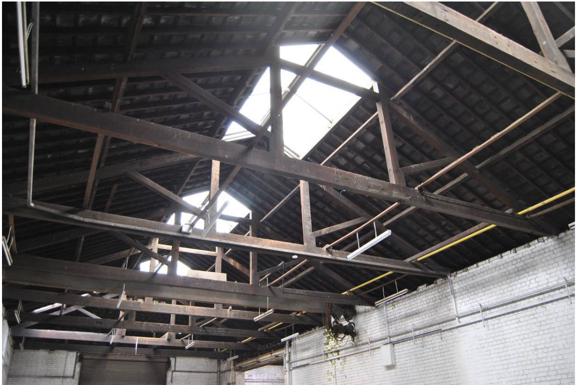
Plate 45: Queen-post roof structure over B2 looking west.
