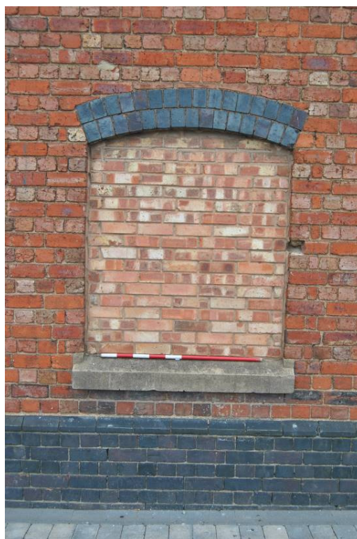
Plate 7: Blocked GF window and blue-brick plinth.
