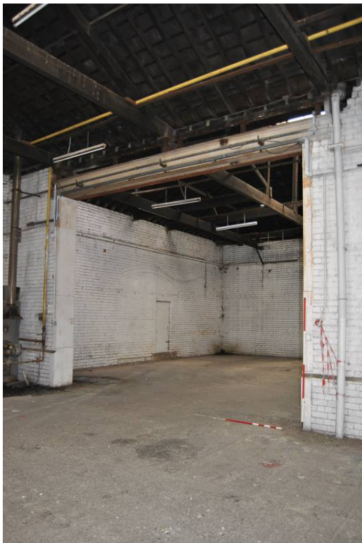
Plate 43: Wide inserted door between B1 and B2 .
