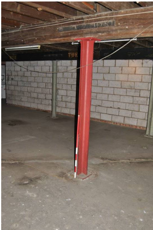
Plate 13: Detail of cross-section stanchion; NB: inserted blockwork walls beyond.
