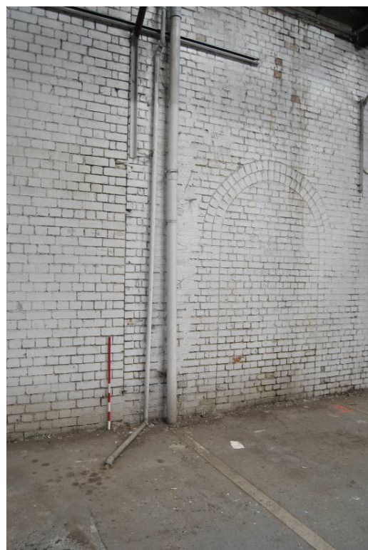
Plate 38: Full-height straight joint and blocked door in north wall of B1 (Bay 4/5).
