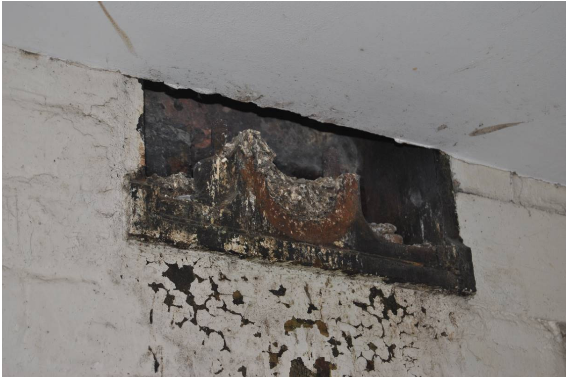
Plate 31: Remains of high-level wall-box for shafting at Bay 2 (E) of third floor level.
