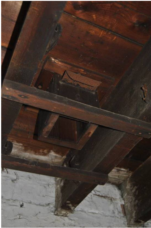
Plate 25: Surviving chute with steel closing plate.
