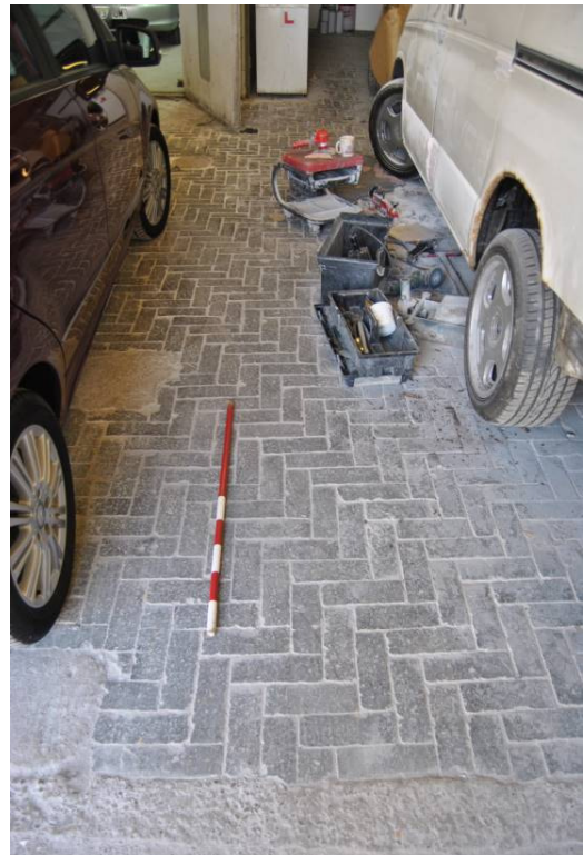
Plate 58: Detail of edge-laid, herring-bone blue-brick floor (Bays 1/2).
