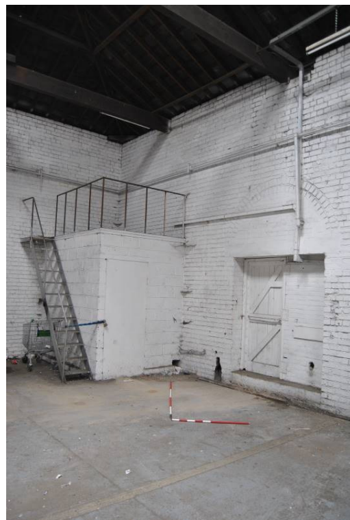
Plate 47: Primary door (partly blocked) and inserted store with raised platform (B2, SE angle).
