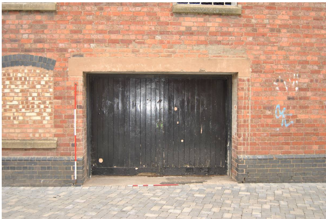
Plate 8: Inserted garage doors at south end of east elevation.
