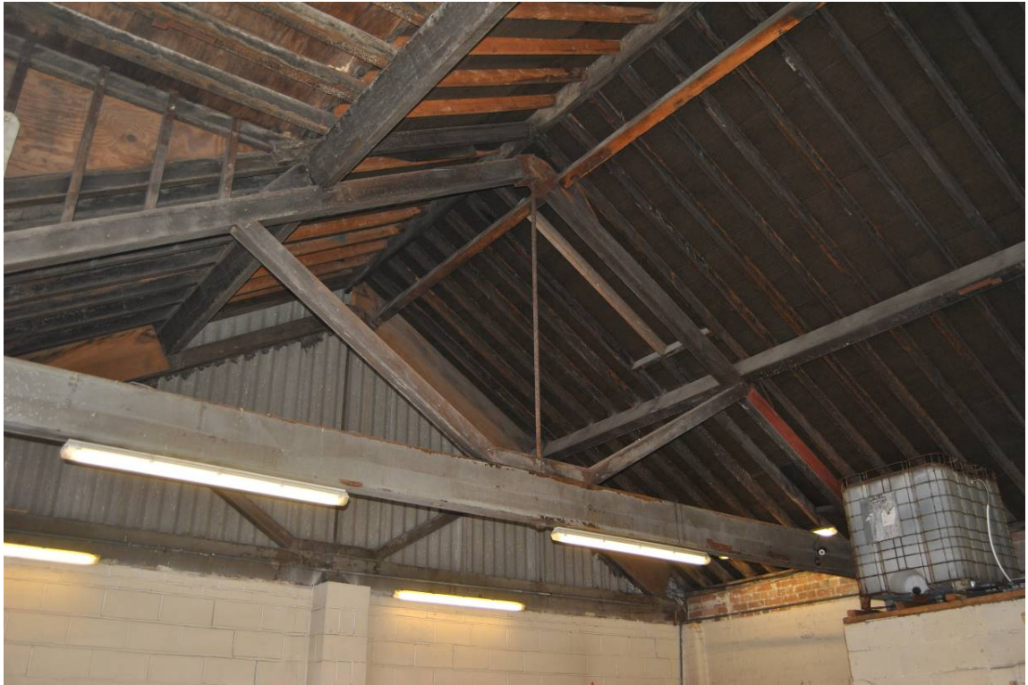
Plate 56: Roof truss T6, compare granary (Plate 37); NB: renewed rafter to upper north slope (left), originally glazed.
