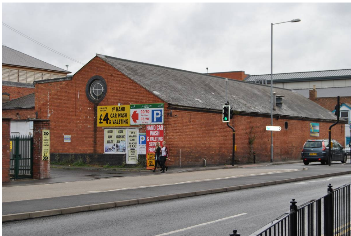
Plate 48: Filtering Shed C, looking north-east, NB: lack of blue-brick plinth to street elevation.
