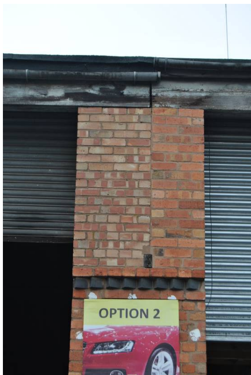
Plate 54: Straight-joint in brickwork of raised doorheads indicating two-phase development.
