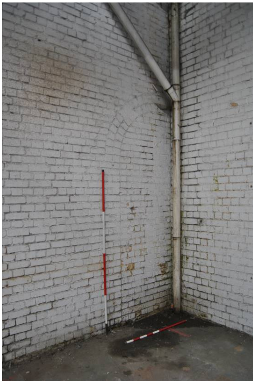
Plate 40: Blocked door at NE angle of B1 , abutted by east wall.
