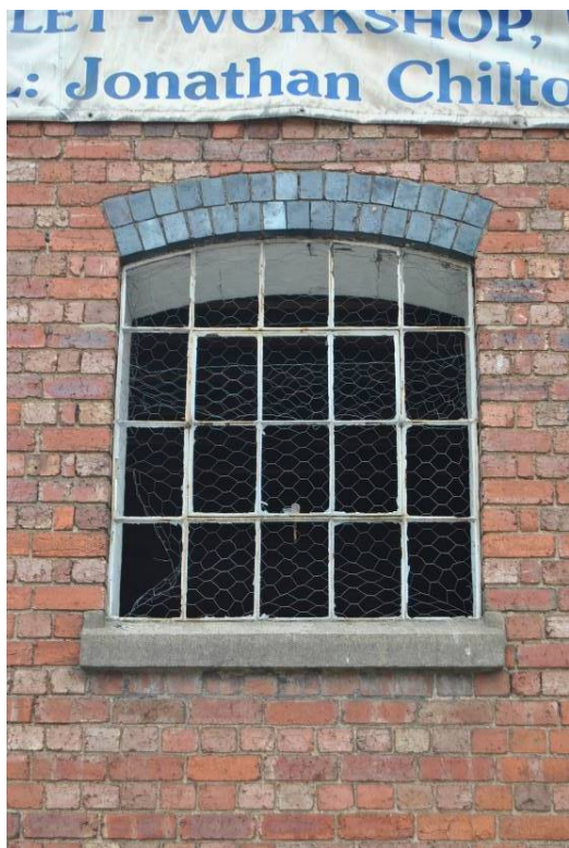
Plate 6: Typical primary window detail (NB: repaired cill).
