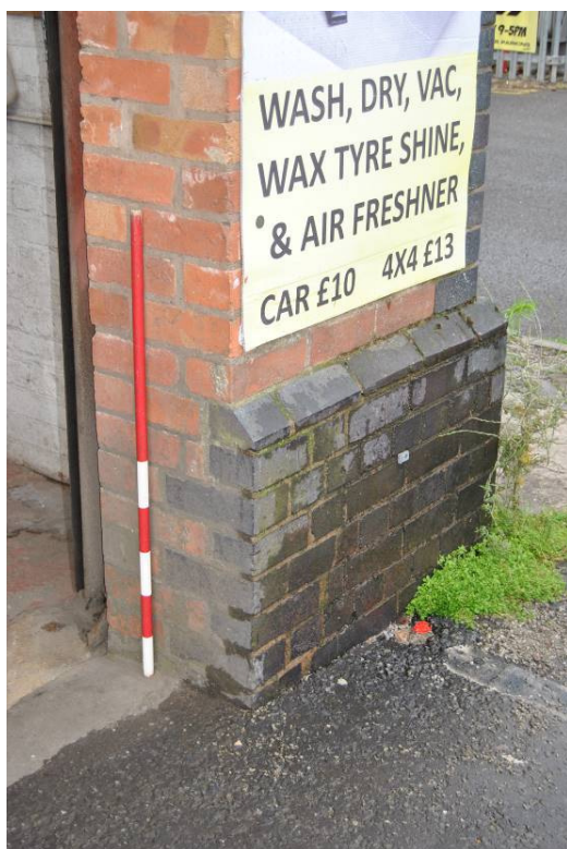
Plate 49: Detail of chamfered blue-brick plinth.
