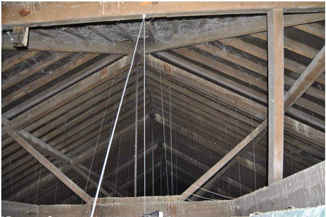
Plate 32: Granary, king-bolt roof structure looking south above suspended ceiling.
