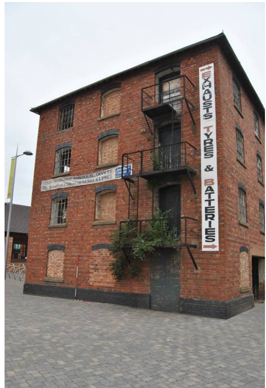
Plate 5: Granary; south elevation with secondary fire-escape stair. Central windows blocked for insertion of interior lift.
