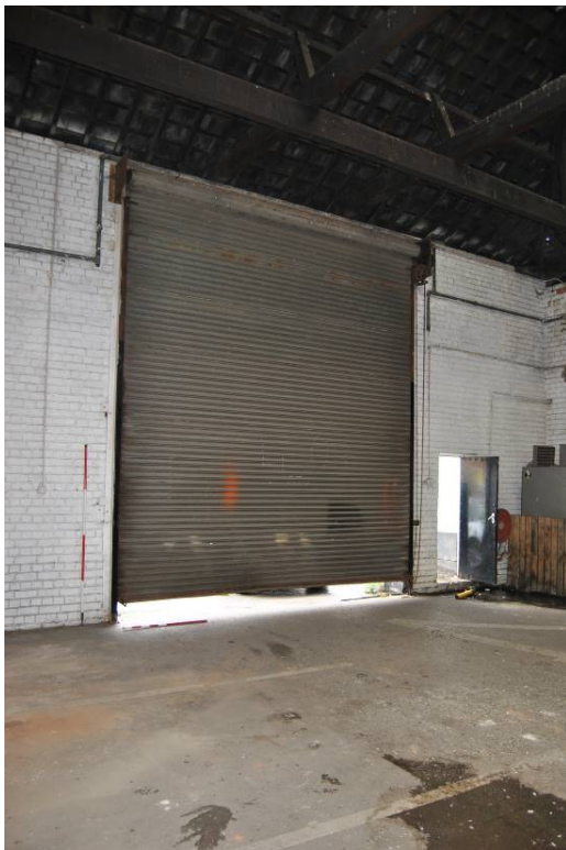
Plate 46: Inserted roller door to west end, B2.
