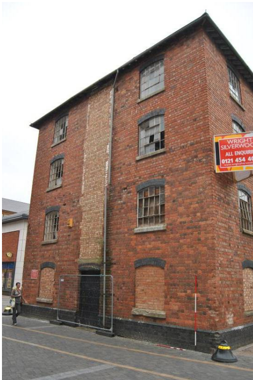
Plate 4: Granary; north elevation with superimposed blocked doorways to centre, formerly opening onto external lucam (see Figure 12b).
