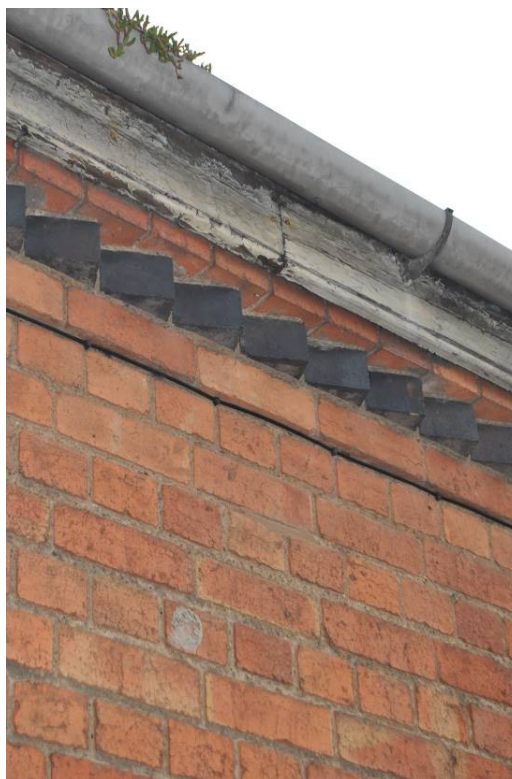
Plate 50: Detail of blue-brick dog-tooth eaves band.
