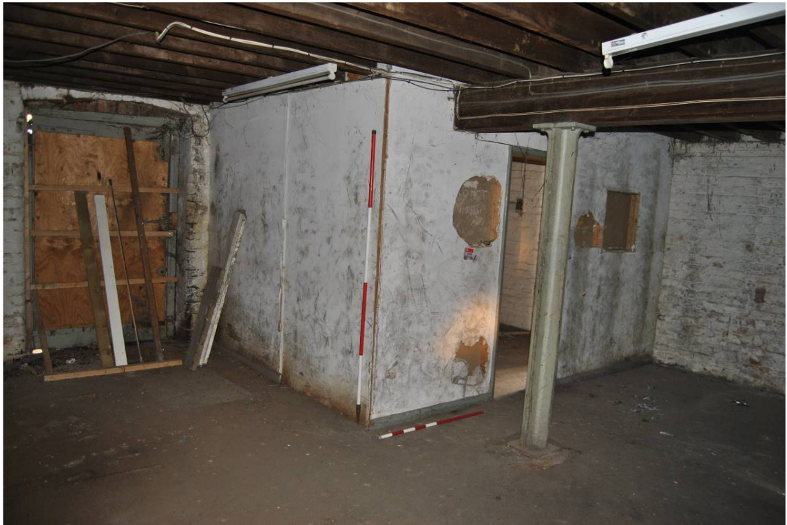
Plate 15: Studwork enclosing stair, with primary door to exterior (left) at base of lucam.
