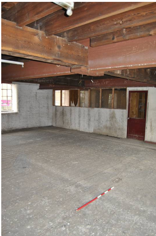
Plate 21: 1F stanchion removed for introduction of transverse steel beam.
