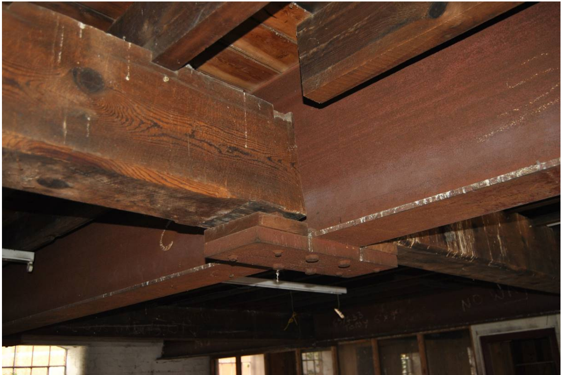
Plate 23: Detail of cutting through of primary longitudinal beam for insertion of transverse steels.
