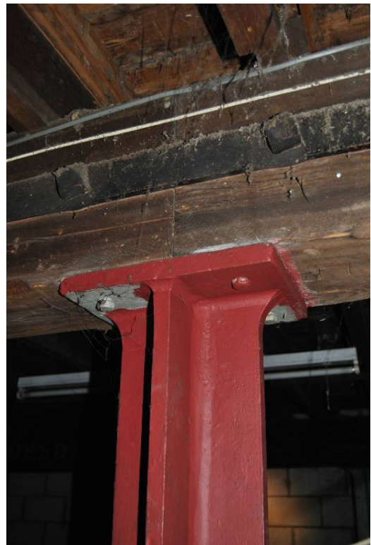
Plate 14: Head of stanchion with butt-jointed, timber longitudinal beam, strapped and bolted.
