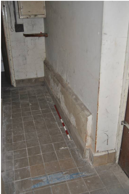
Plate 73: Chamfered plinth of B1 west wall, visible in corridor of infill block E .
