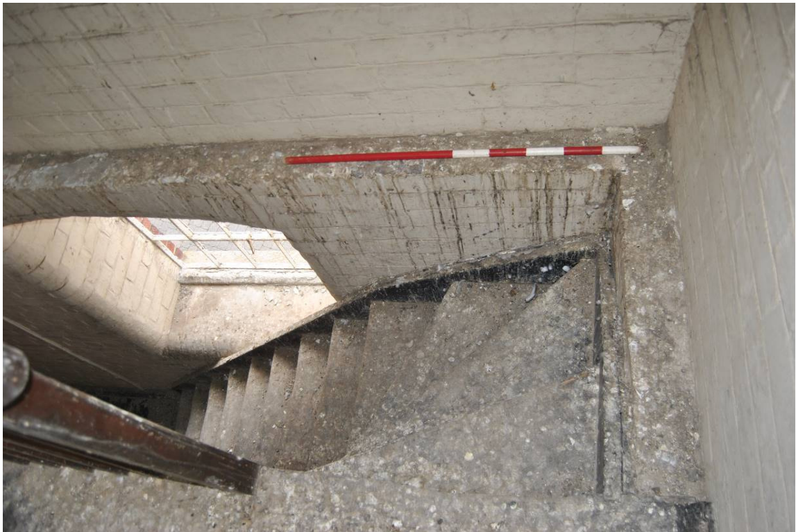
Plate 26: 5-inch offset in north and east walls as walls narrow from 24in.-19in. at 2F level.
