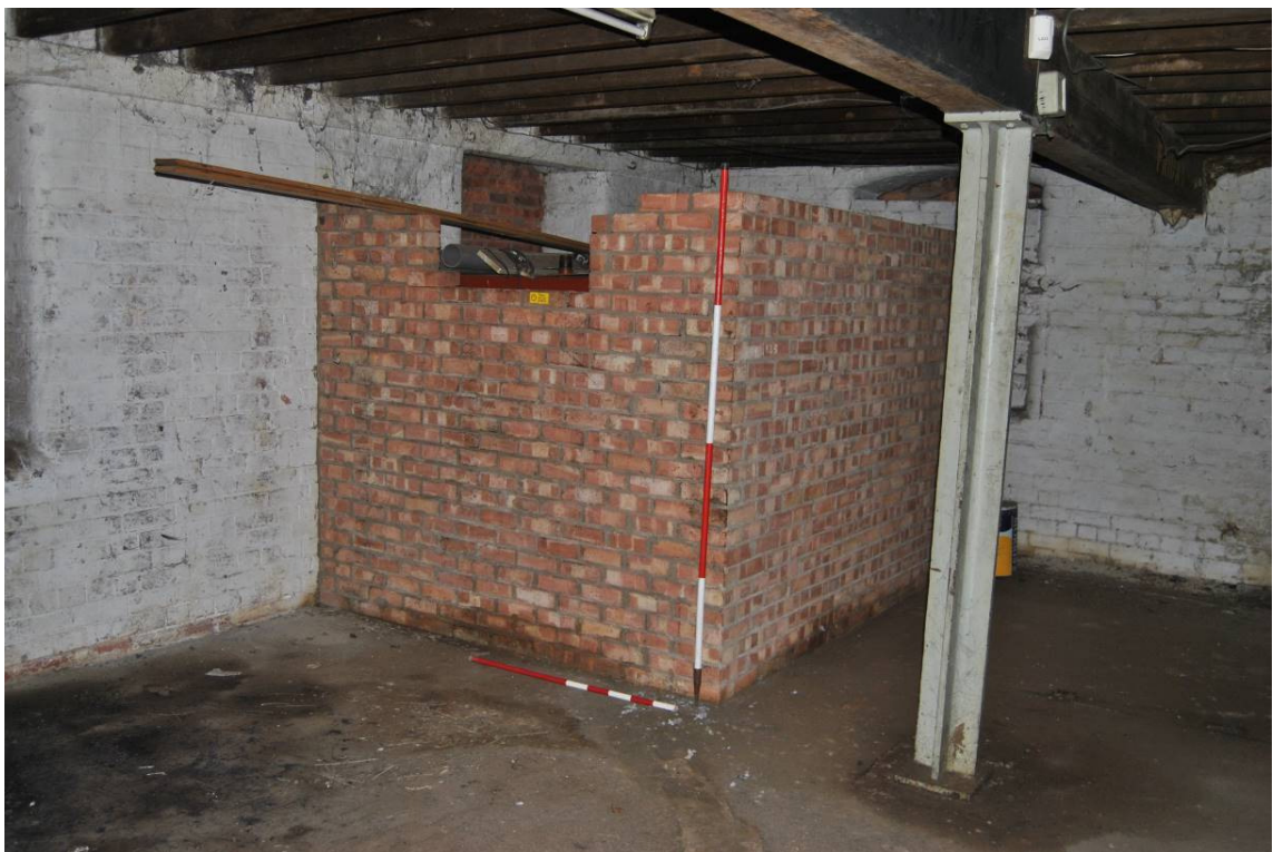
Plate 16: Inserted brickwork enclosing oil tank at north-west corner of ground floor.
