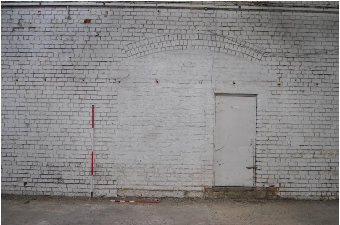
Plate 42: Partially blocked doorway in western gable of B1 , note stone hinge blocks and original chamfered jamb to right.
