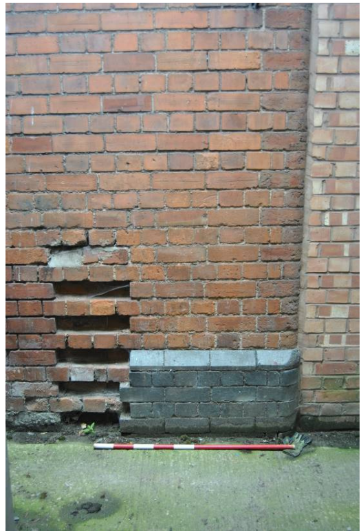
Plate 65: Plinth east of door terminates to respect former manure pit (keyed in brickwork) – see Figure 25b.
