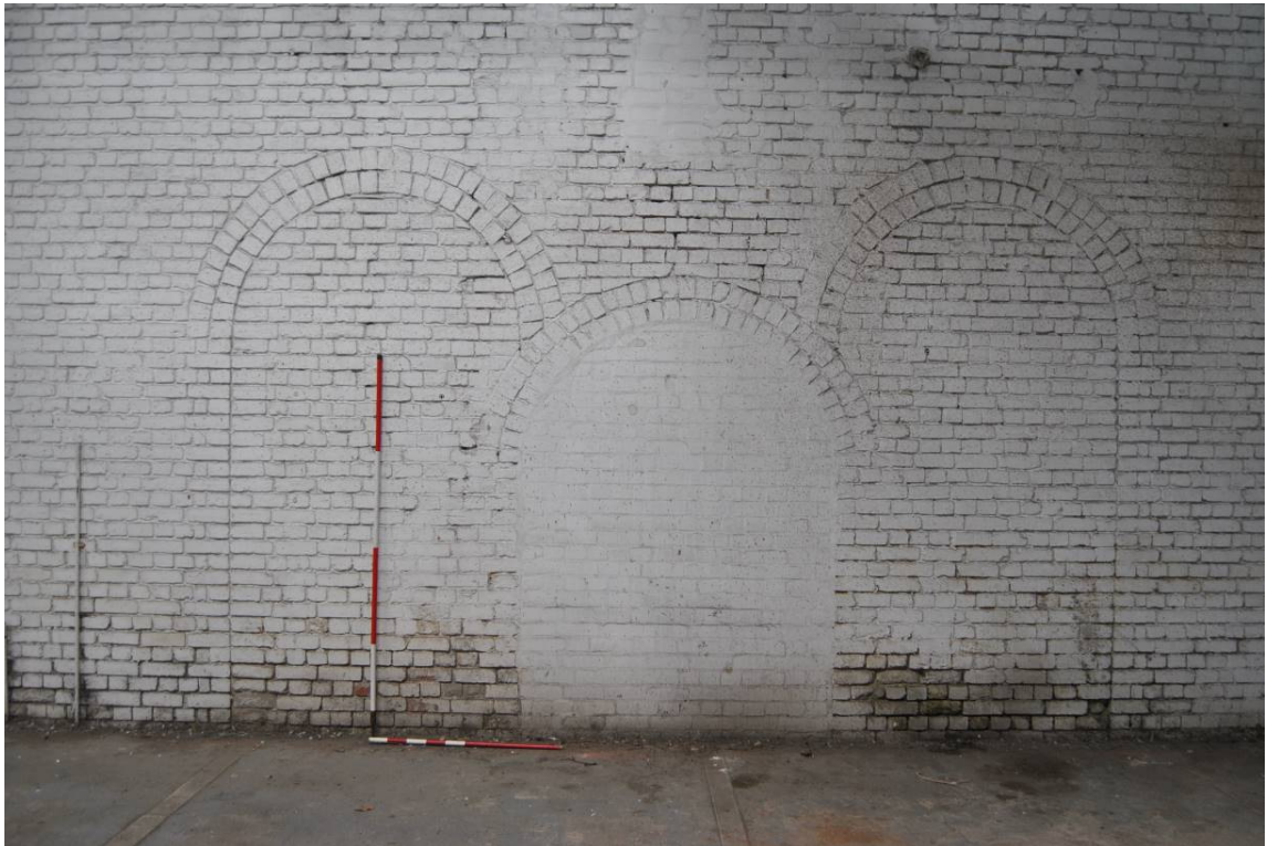
Plate 39: Sequence of blocked doorway openings in north wall of B1 (east end).
