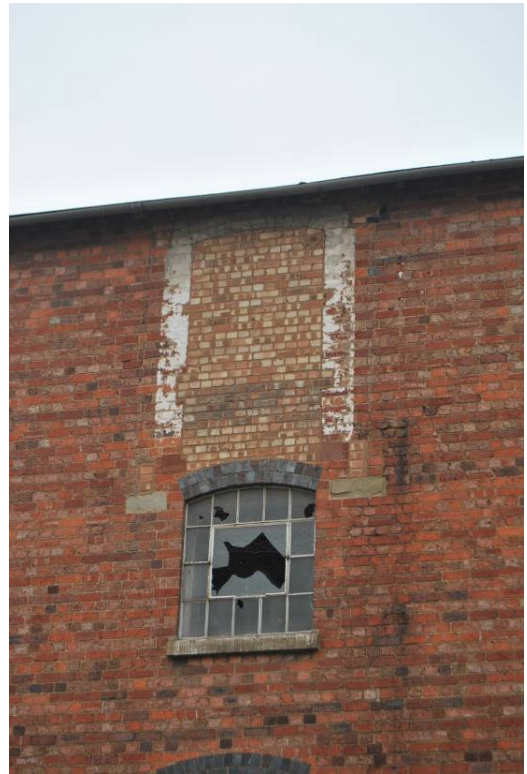
Plate 10: Blocked door at 3F level, east elevation formerly serving raised walkway to adjacent range.
