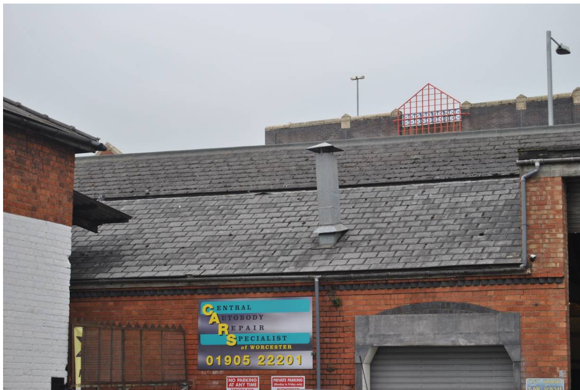
Plate 53: Two-part cladding of northern roof-slope; upper section originally glazed (see Figure 23).
