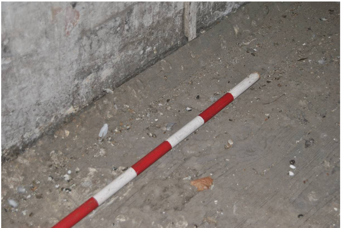
Plate 24: Plain 2-inch fillet skirting detail.
