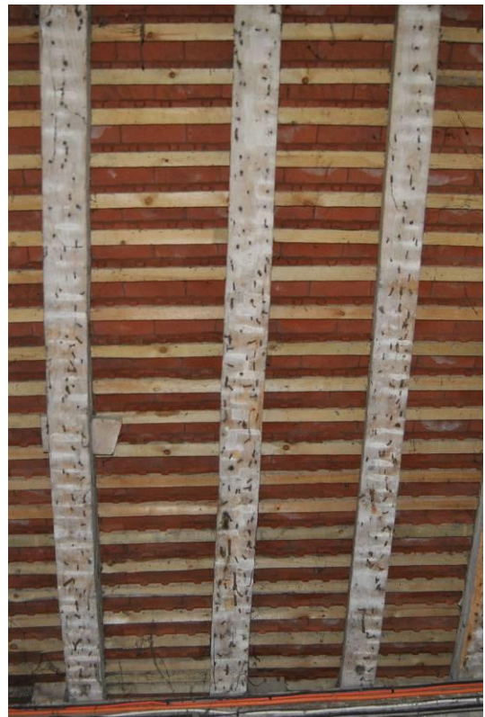
Plate 83: Tacks to common rafters for former L&P render, present over Bays 3-6 only.
