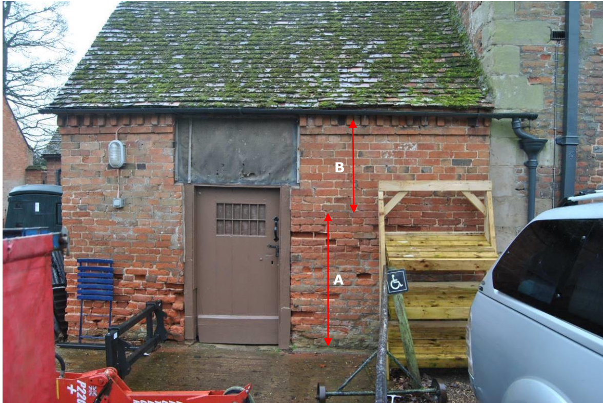
Plate 110: North elevation of slaughterhouse showing early brick boundary wall A, raised in 3in. brick B.
