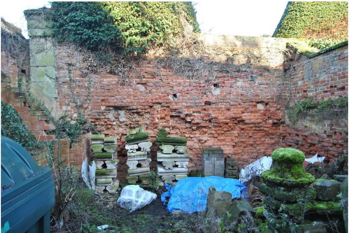
Plate 161: Yard M looking north-east NB. sloping line of sockets indicating former lean-to roof (marked).
