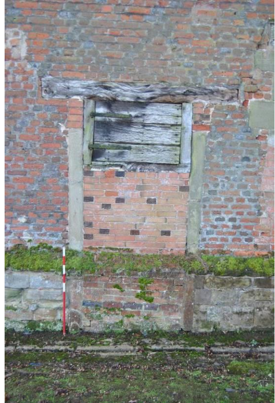
Plate 9: Former door [d2]; partially blocked leaving upper ventilation hatch.
