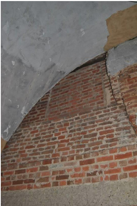
Plate 65: Inserted barrel ceiling cutting across blocked window [w27] in west gable.
