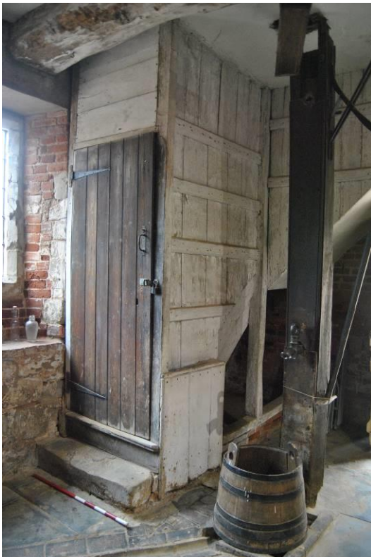
Plate 35: Stair [a] rising to 1F level at SW corner [G1], NB. tall pump (centre) feeds raised channel serving brewhouse B.
