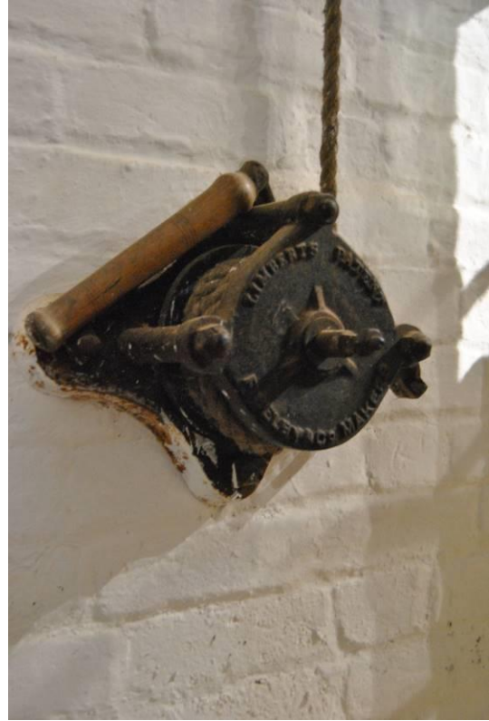
Plate 57: Winch to east wall; F Selby and Co. (of B'ham).
