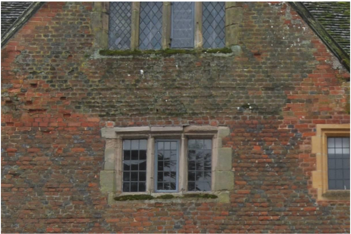
Plate 4: Detail of central gable showing discernible change in colouration of brick (immediately above [w8]) between 1F level and gable over (see also Plate 12).
