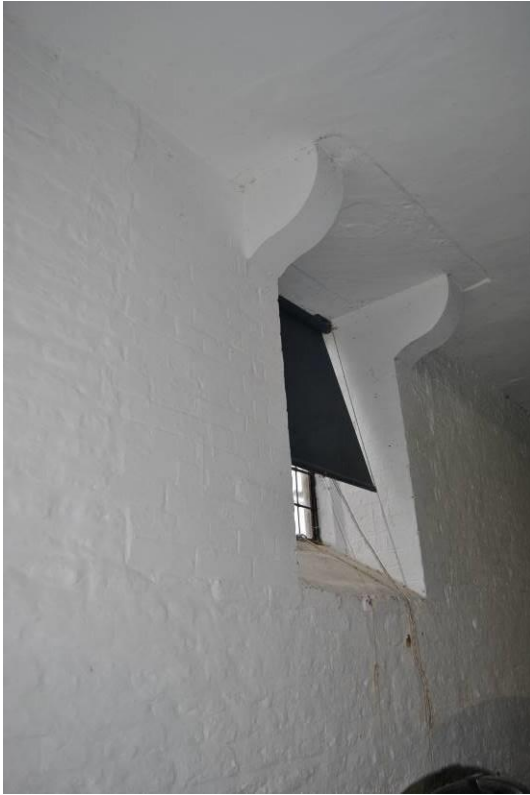
Plate 56: Partly blocked [w3] with corbels for 1F FP.
