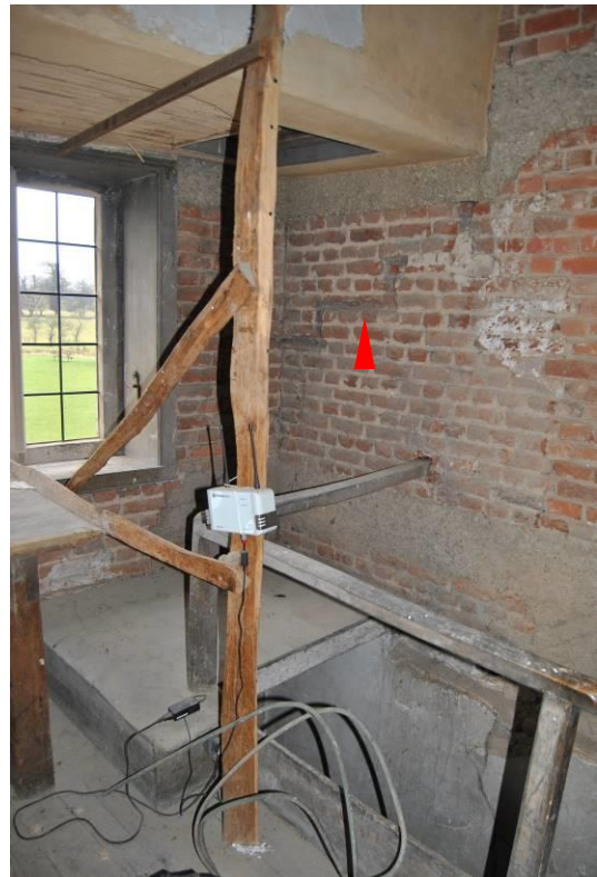
Plate 66: Stair [a] rising at south-west corner with scar of former continuation (1F – 2F; arrow).
