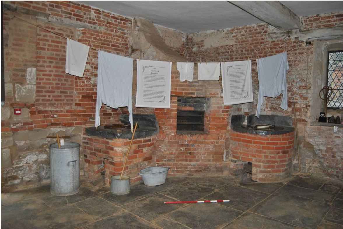
Plate 29: Laundry A (Room [G1]) looking north-west with bread oven to angle, flanked by coppers, NB. flue rising to west wall.
