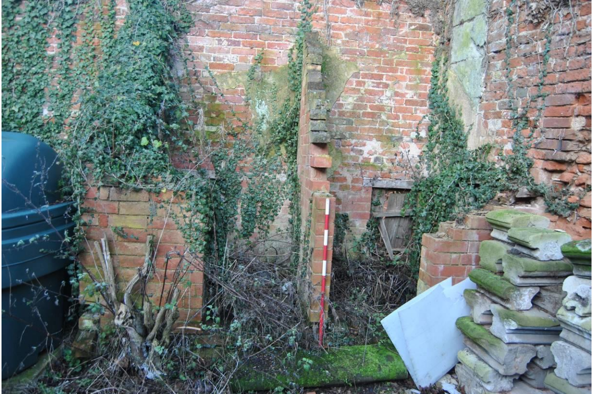
Plate 164: Secondary 'hutch' enclosures to north-west angle of yard M, served by openings in western woodyard wall.
