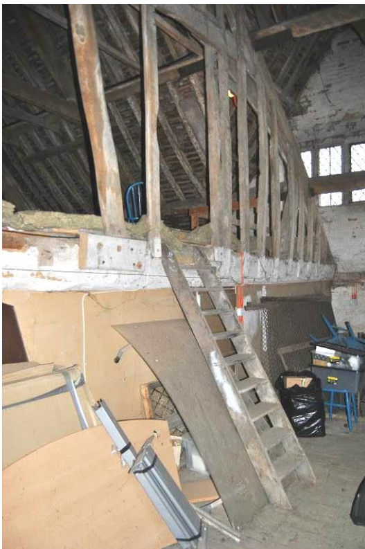
Plate 82: Stud infill to truss TIII.
