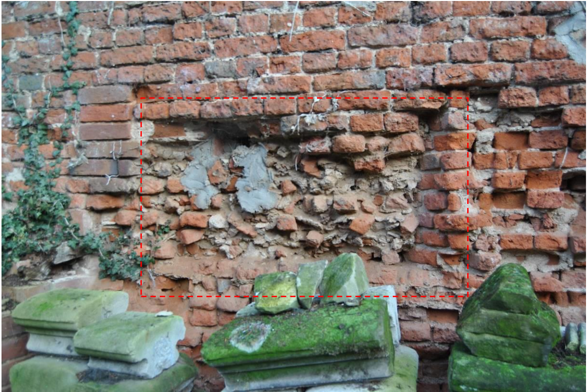
Plate 162: Apparent blocked opening to north wall with clear splayed jamb to right.
