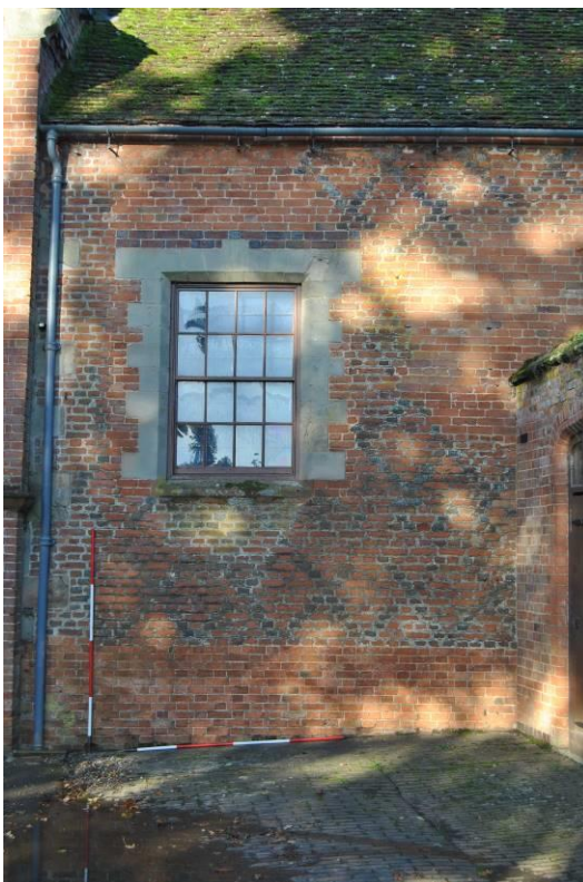
Plate 92: East range, east elevation (note underbuilt lower wall and quoins visible behind down-pipe to left).
