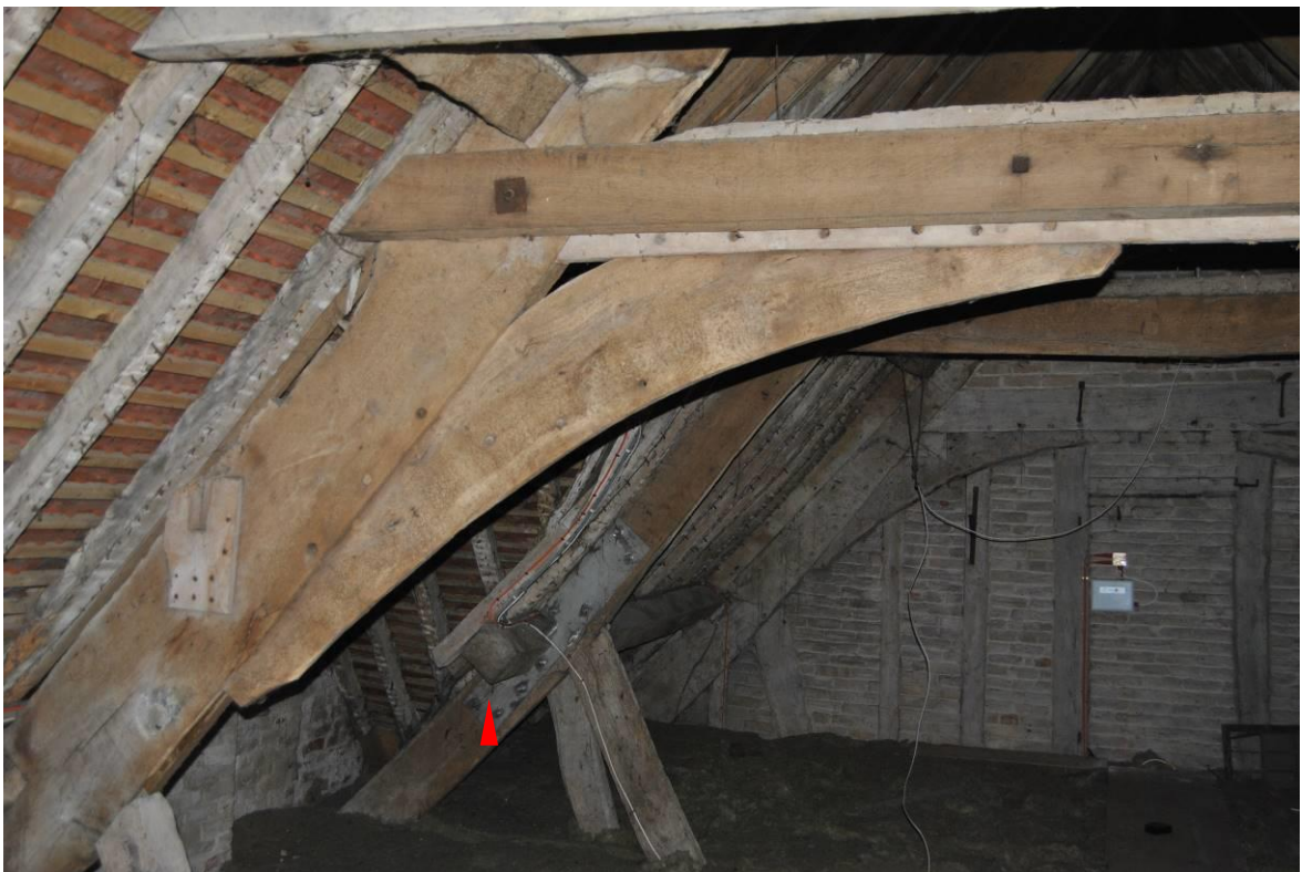
Plate 80: Detail of arch-brace to truss TV (S), note truncated lower purlin to truss TVI (arrow).
