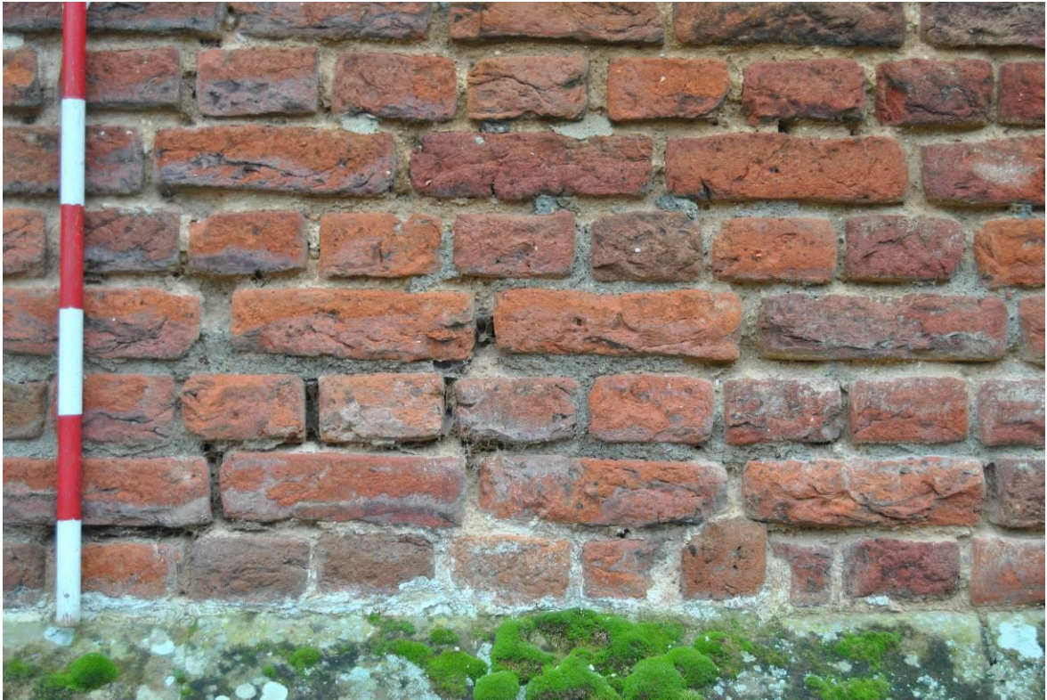
Plate 11: Detail of original English bond brickwork.
