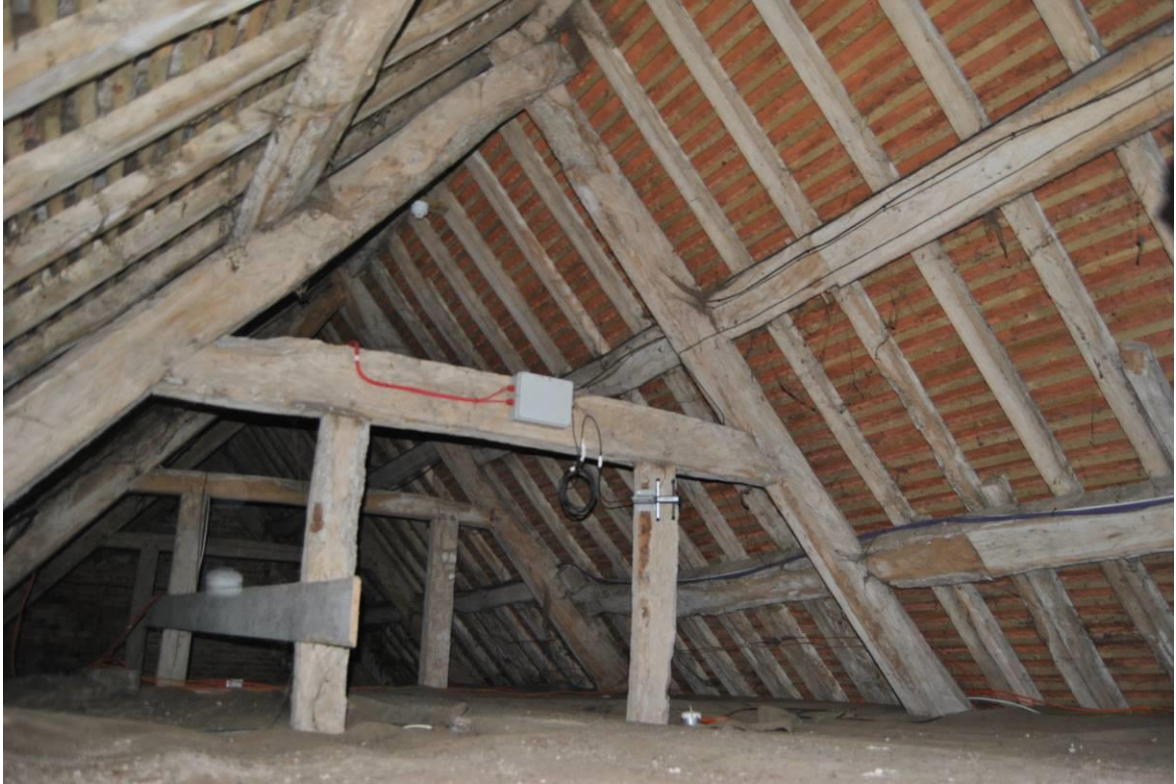
Plate 108: Regular, 4-bay queen-strut roof over [F11-13]; north end of east range, looking south.
