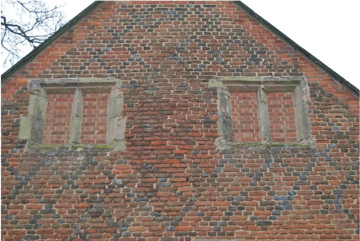
Plate 24: Primary, two-light stone-mullioned windows [w26/27] to second floor (attic) level. NB. raised/rebuilt parapet and disturbed diaperwork patterning between windows.
