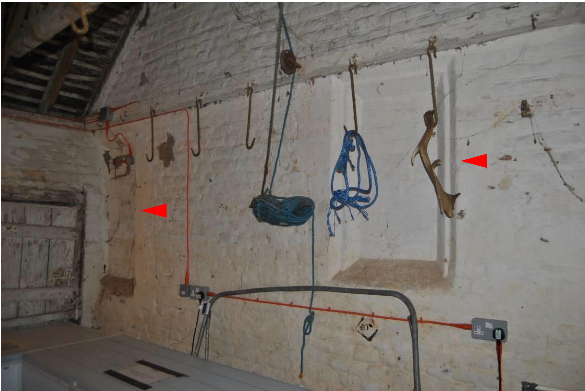
Plate 28: Two blocked single-light windows (arrows) visible within slaughterhouse G (compare 'Beighton' view of 1722).
