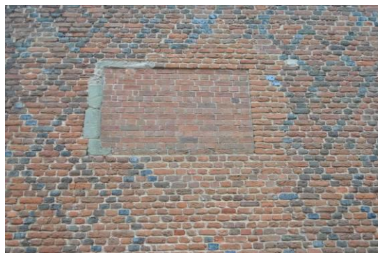
Plate 23: First floor window [w25], NB. patching around right hand jamb.
