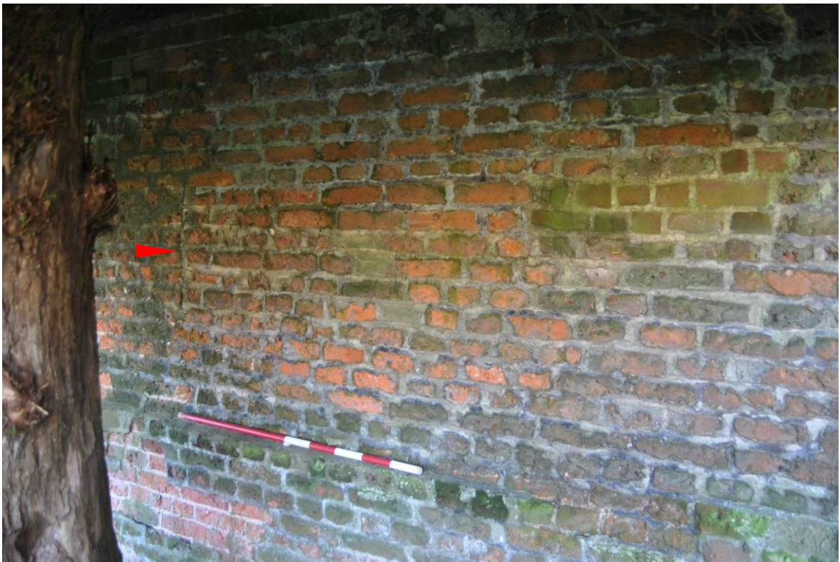
Plate 163: Vertical straight-joint (arrow) and blocking material related to opening as visible within Greencourt.
