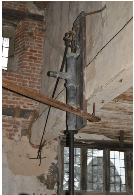
Plate 49: High-level pump from underback to second, boiling copper.
