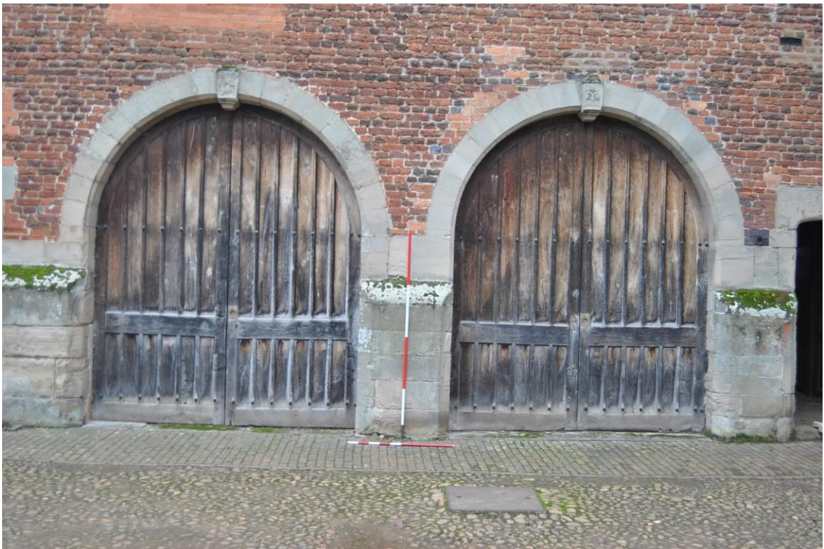
Plate 14: Carriage house doors [d4/5]. NB. disturbed primary brickwork around arched heads.
