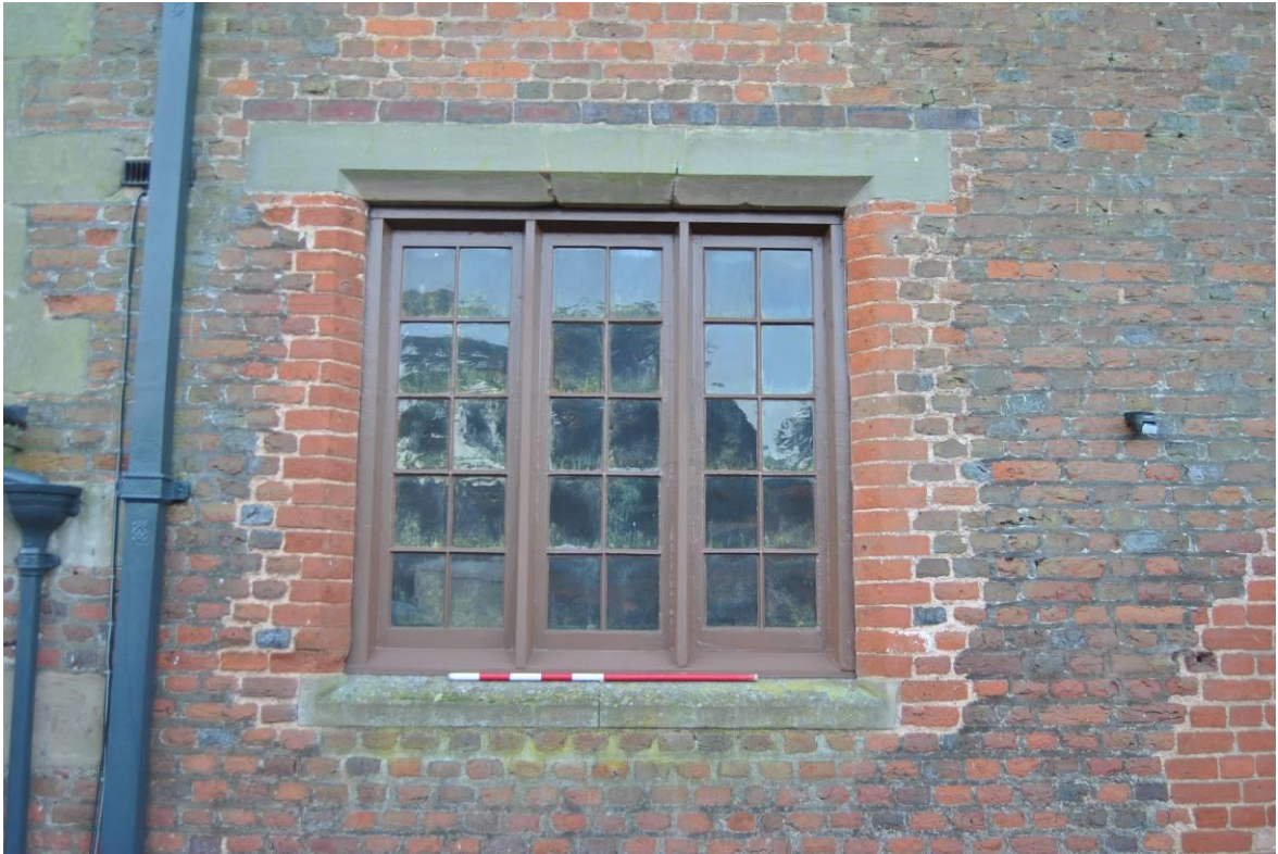
Plate 5: Window [w1] with renewed stone head and chamfered brick jambs.
