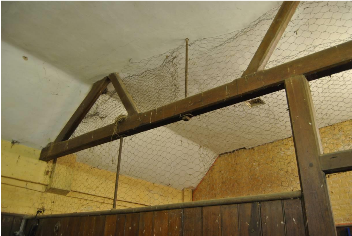
Plate 143: Detail of king-bolt roof truss.
