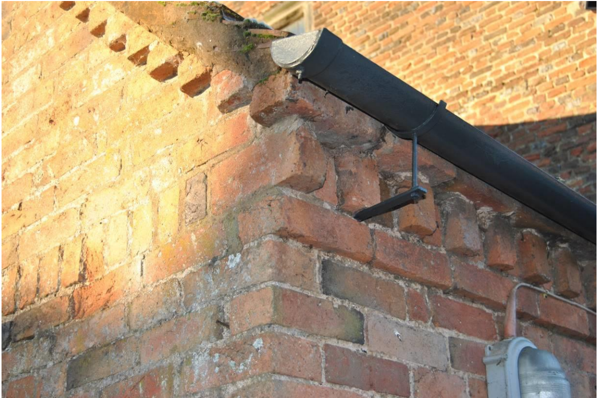
Plate 112: Building G; detail of ¼-brick oversail/dentil eaves band.
