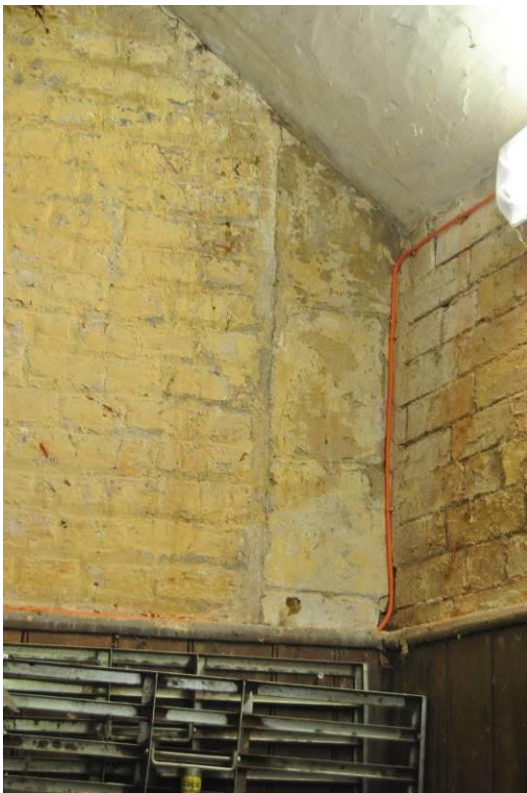
Plate 144: Quoins of SE angle of north service range, visible within loose-box.
