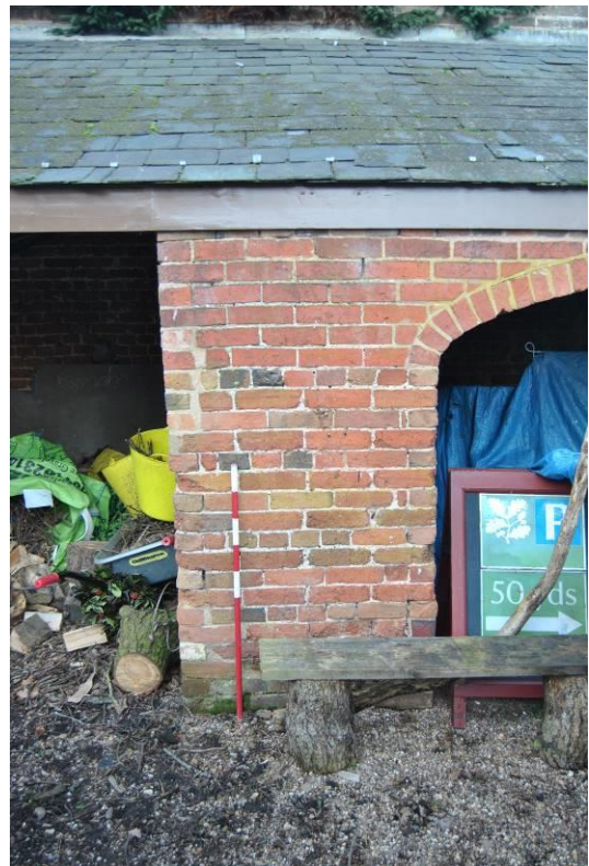
Plate 173: Partly rebuilt pier at O3/P1.
