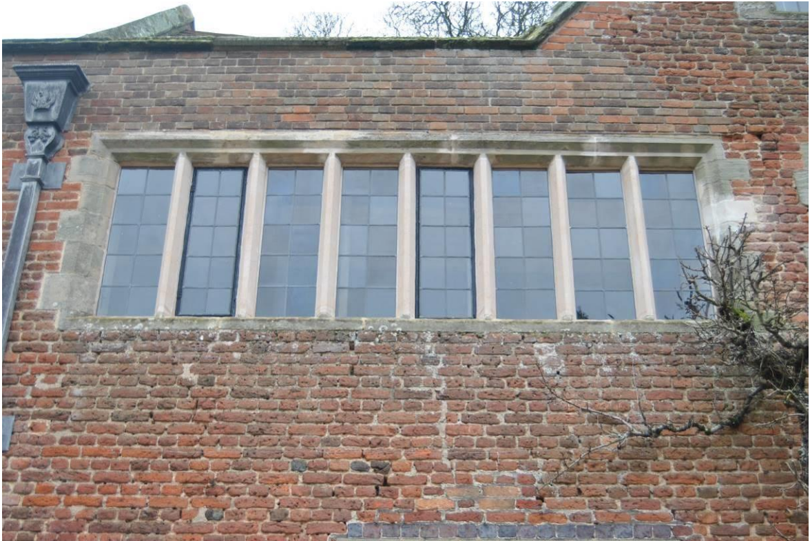
Plate 13: 19 th -century, 8-light window [w17], inserted to light dry laundry. NB. rebuilt parapet over.
