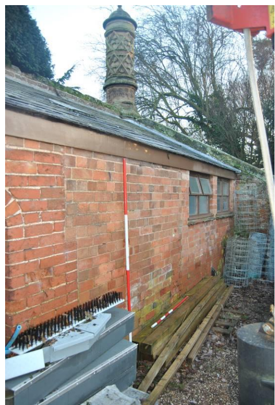
Plate 177: Converted outhouses Q looking north-east. NB. secondary Engl. Bond brickwork
