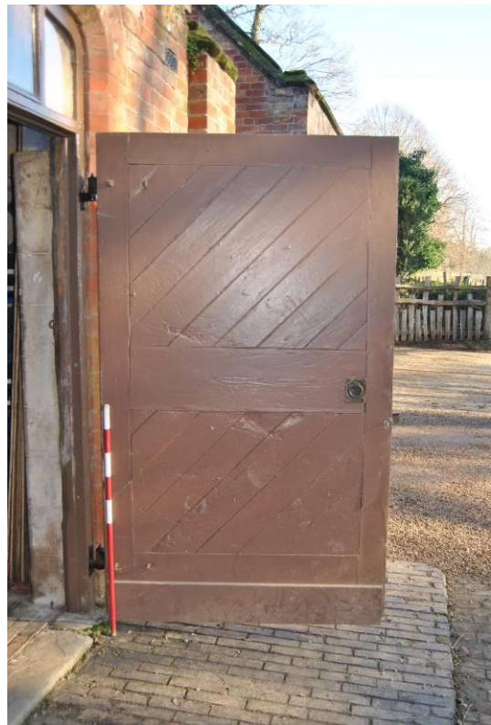
Plate 121: Detail of diagonal planked interior door lining.
