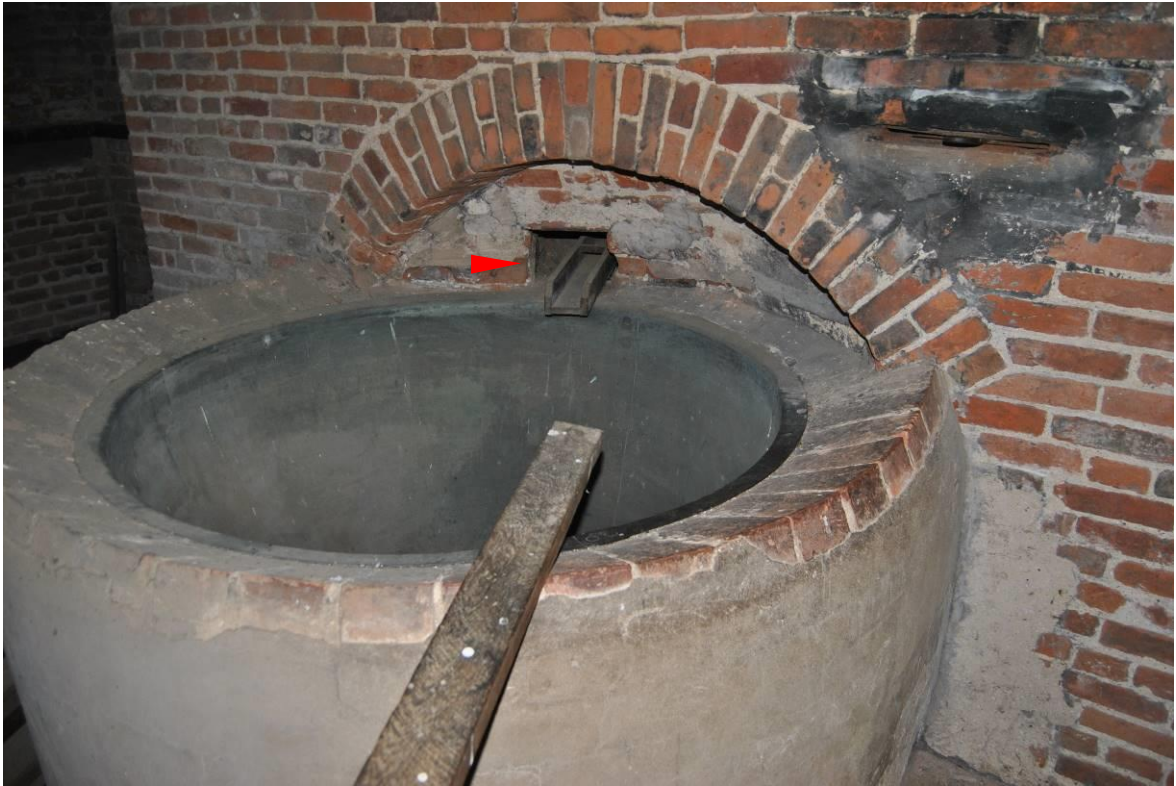
Plate 47: Southern copper fed by raised channel (arrow) passing through wall from adjacent laundry. NB. damper to right of brick arch.
