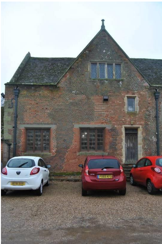
Plate 6: Eastern gable of north elevation. NB. multi-phase brick patching and raised / rebuilt parapet.
