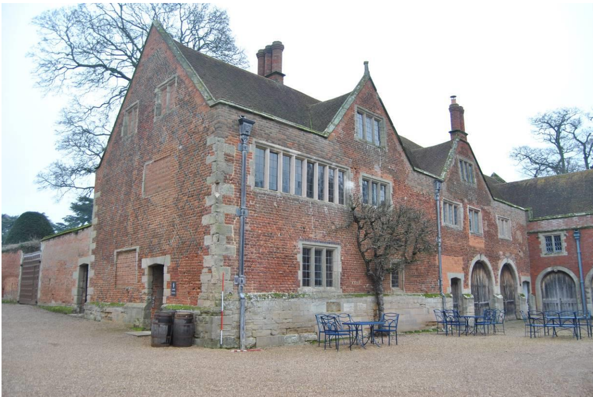
Plate 10: North service range; south elevation, oblique view looking north-east. NB. quoins to south-west angle do not extend onto parapet.
