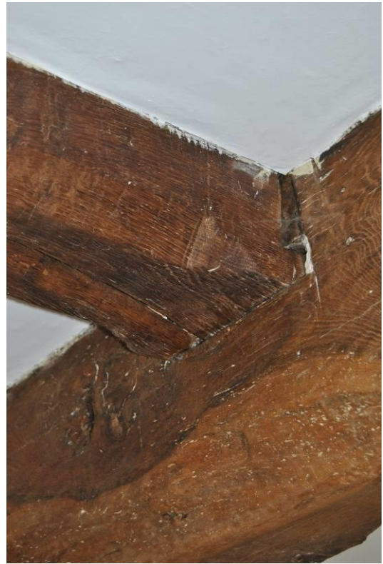
Plate 76: Bare-faced soffit-tenon (unhoused) of 1F ceiling beams Rm. [F7].
