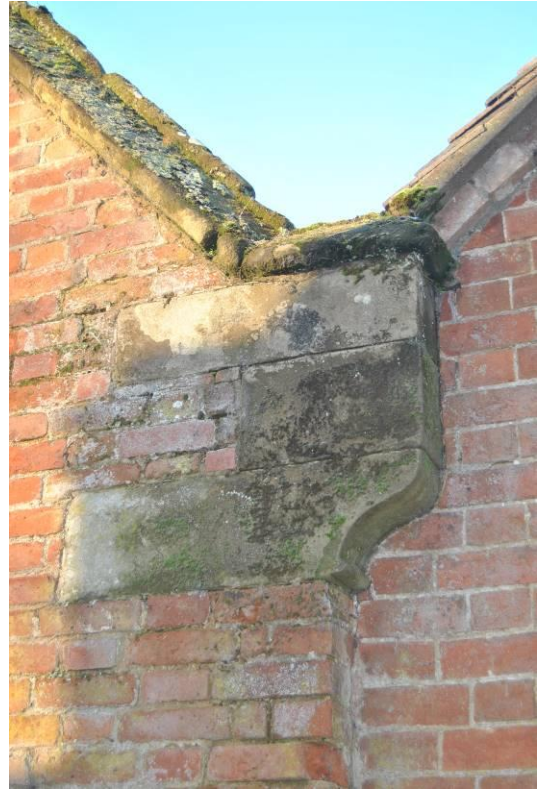
Plate 123: Bldg. H, stone kneeler to NE angle.
