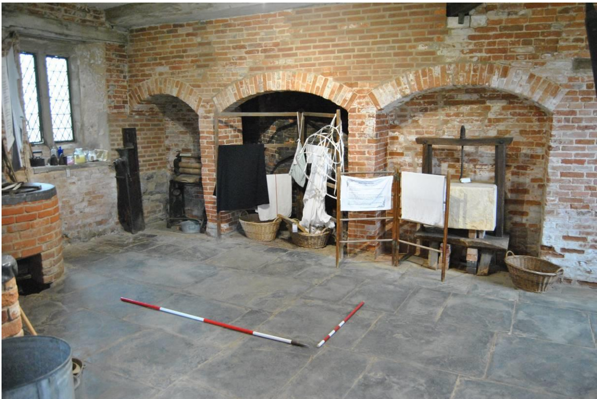
Plate 30: Laundry A ([G1]) looking north-east with triple arches; central recess houses fireboxes and ash-pits to the brewhouse coppers.
