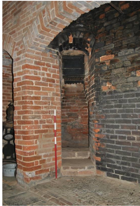
Plate 32: Detail of northern firebox / ash-pit.
