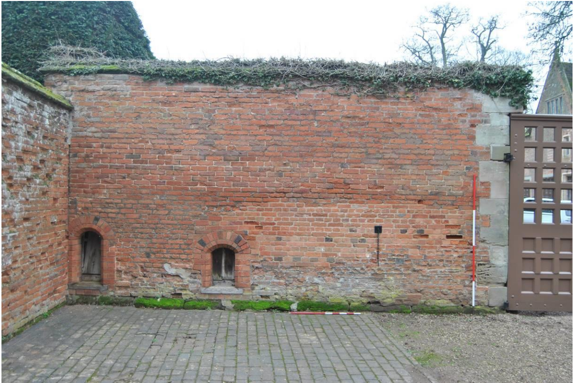
Plate 160: Western woodyard wall (north end), forming west side of enclosed yard M . NB. small, inserted access points to 'hutches' within yard M (see Plate 163).
