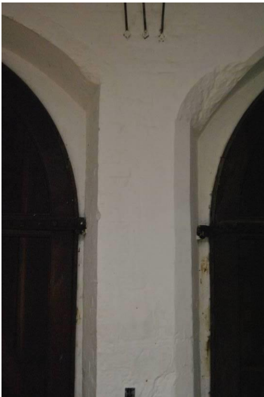
Plate 54: Variation in door arches. NB. cut-back springing of [d4] (right) to accommodate door.
