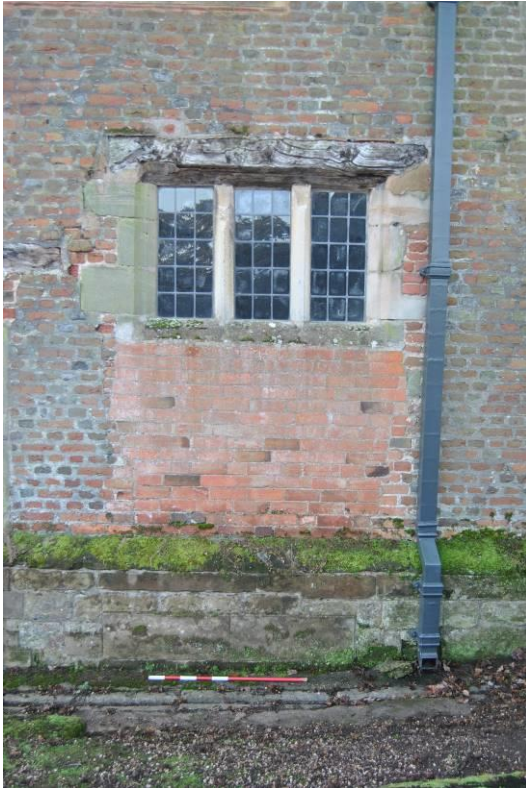
Plate 8: Window [w4] with ovolo-moulded mullions and timber lintel, NB. brick blocking below.
