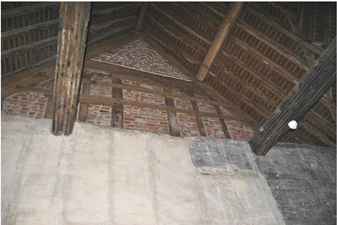
Plate 42: West face of infilled truss TVII above brewhouse, NB. central blocked door formerly serving attic floor.
