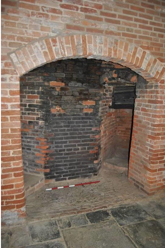
Plate 31: Brewhouse firebox access.
