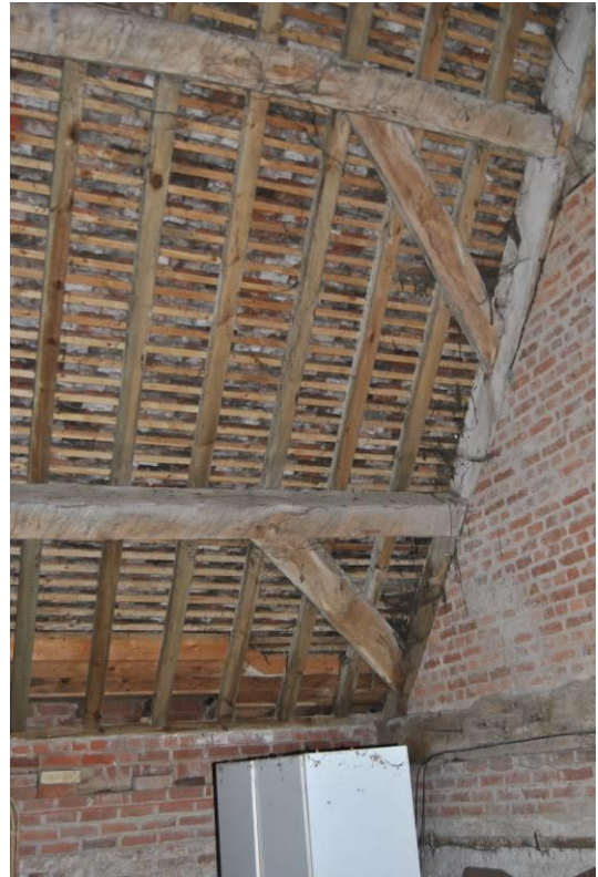
Plate 79: Wind-bracing to Bay 1 (N).
