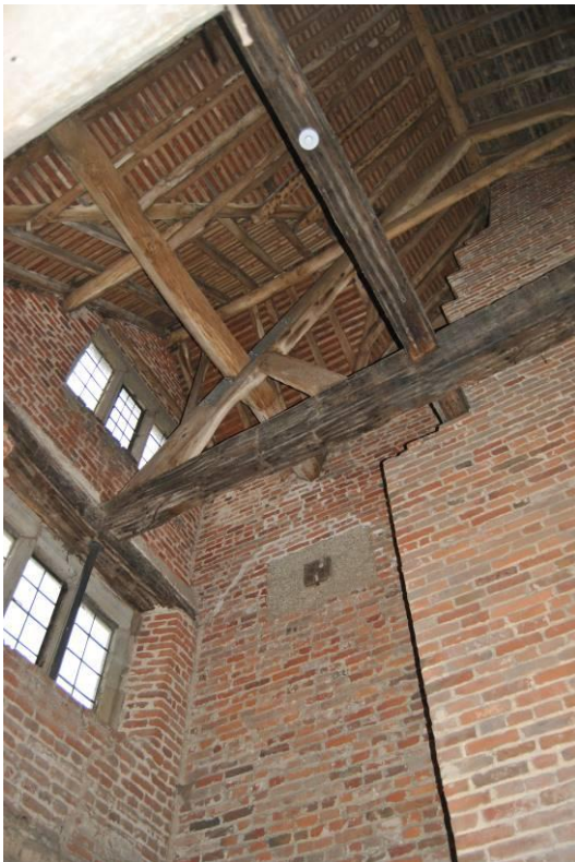
Plate 38: Open roof over western section of brewhouse Truss TVIII visible NB: uneven discolouration of timbers indicating former ceiling.
