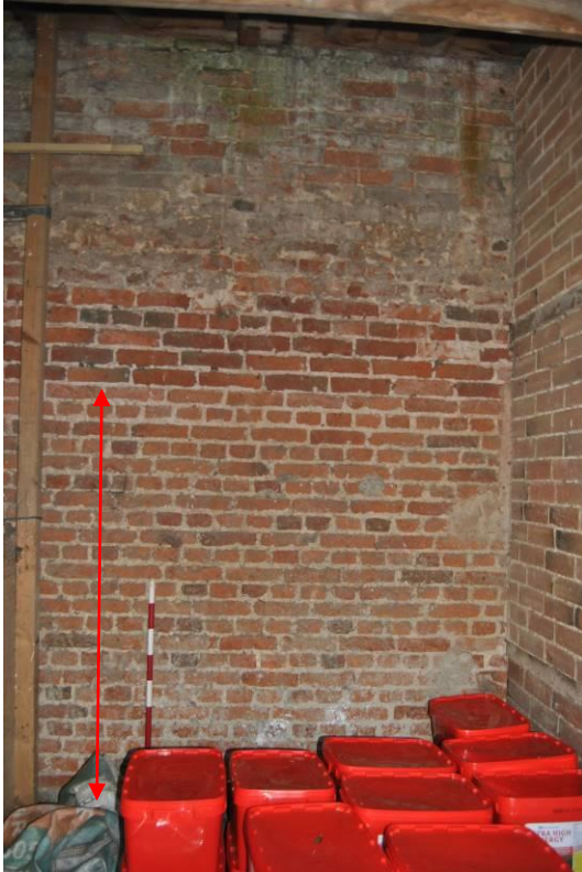
Plate 166: Detail of back wall (NB. lower, English bond brick of early Greencourt boundary wall).
