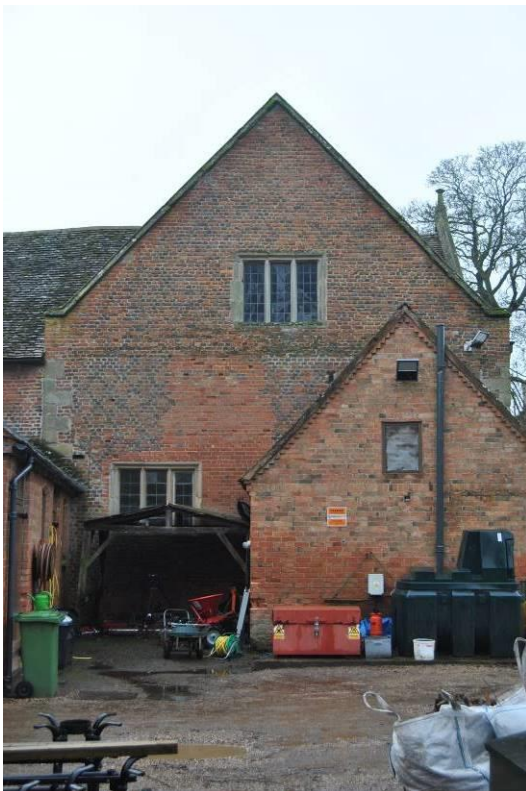
Plate 25: North Range, east gable end (with slaughterhouse G to right), NB. area of blocking ( BW ) upper right of ground floor window.
