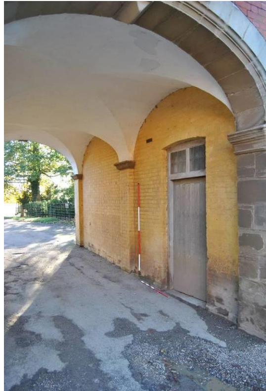
Plate 91: Carriage entrance with C19 th -brickwork walls and groin vault in two bays.
