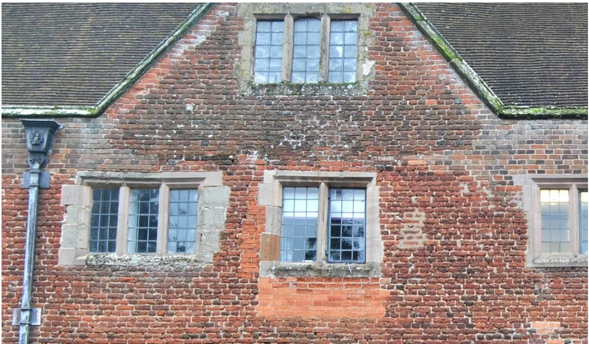
Plate 12: Detail of central gable showing discernible change in colouration of brick between 1F level (orange/red) and gable over (darker brown/red); see also Plate 4.
