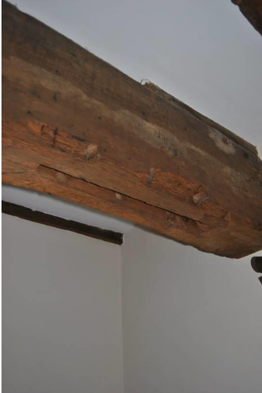
Plate 75: Peg-holes and soffit mortice for 'knee'-brace at north end tie (TVII) – visible in Rm. [F9].
