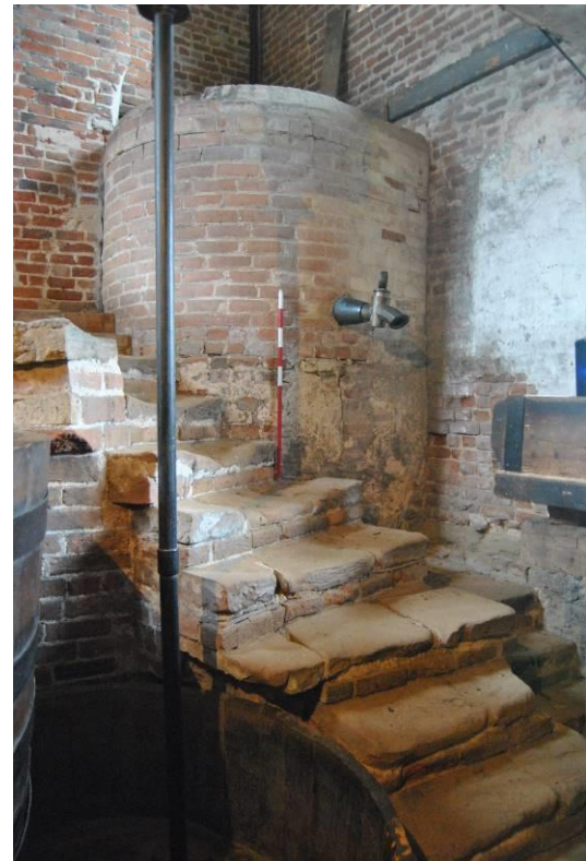
Plate 46: Access stair to working platform. NB. secondary upper brickwork of copper.
