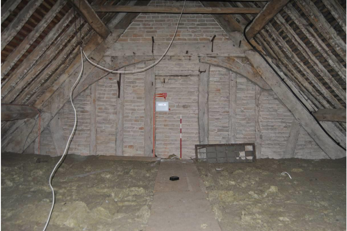
Plate 81: Closed truss at TVII, looking west, with central doorway (blocked). NB pattern of whitewash to timbers.
