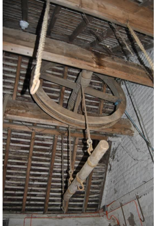
Plate 116: Re-set carcass-wheel.
