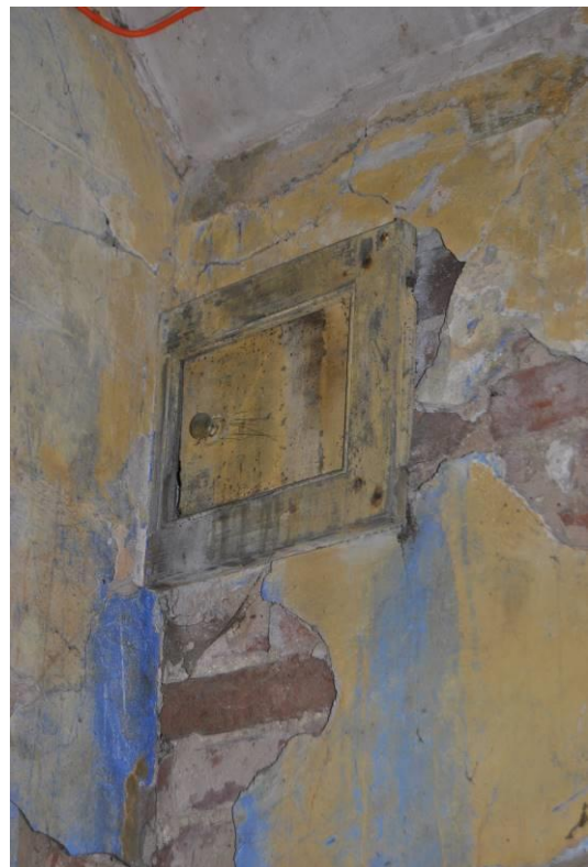
Plate 129: High-level vent with sliding timber shutter.
