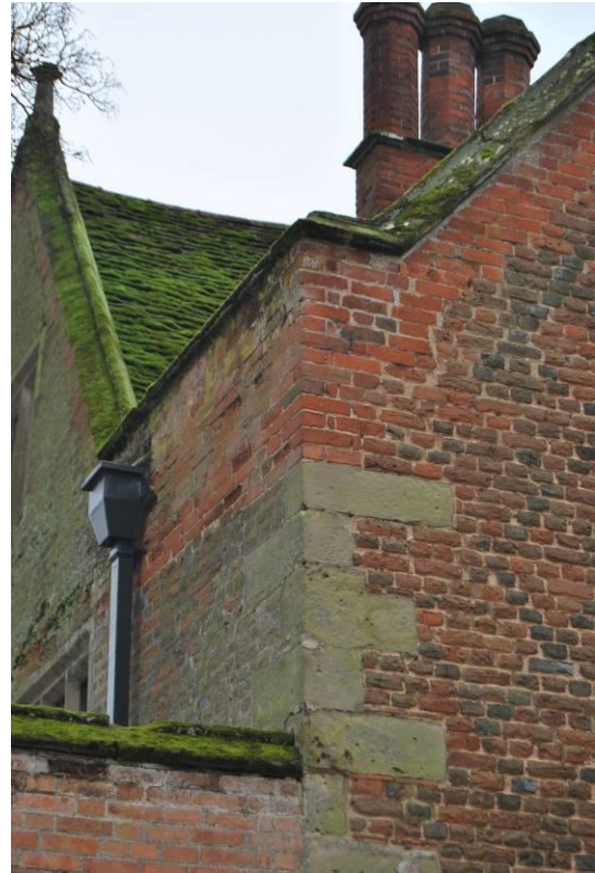
Plate 20: Secondary parapet wall above stone quoins.
