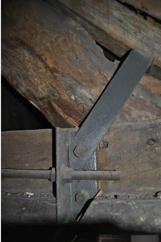
Plate 84: Tie rod at Truss TIX.
