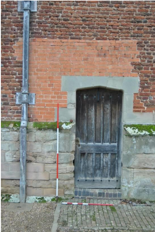
Plate 15: Tudor arched door [d3], inserted into former, larger doorway opening.
