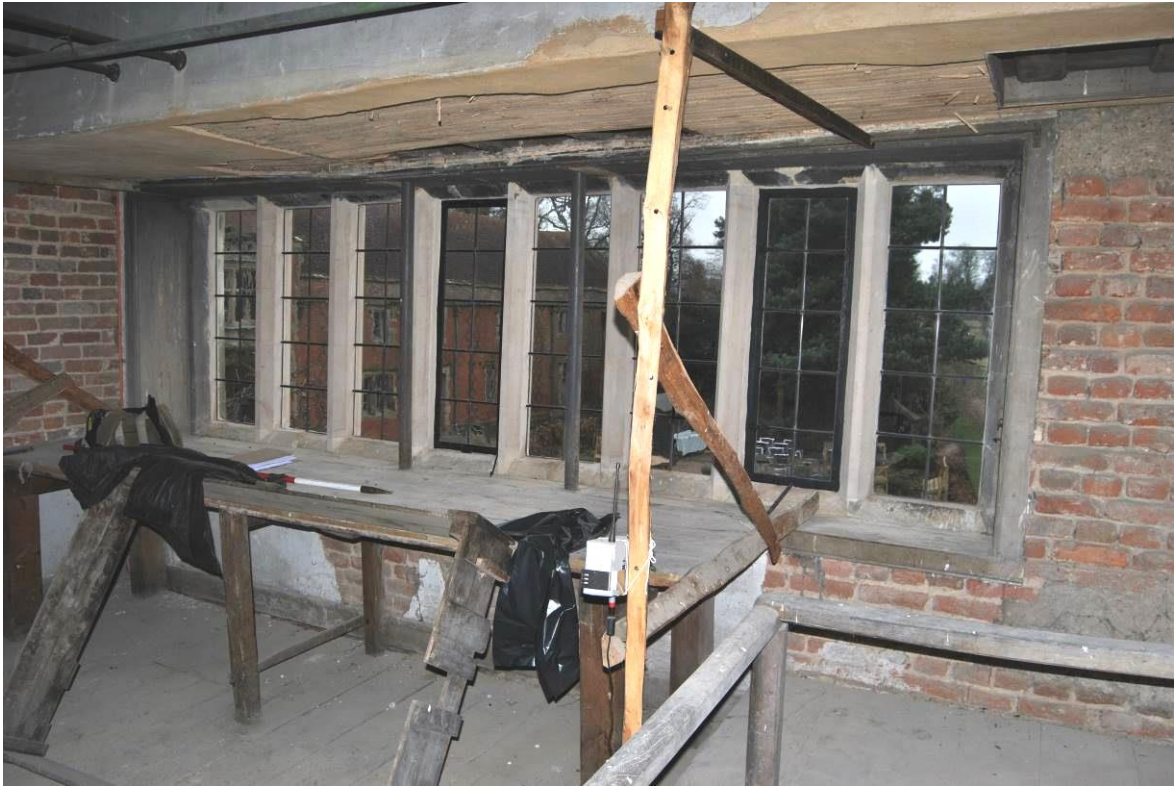
Plate 64: Inserted 8-light window [w17] to south elevation (mullions recently renewed), with ironing table.
