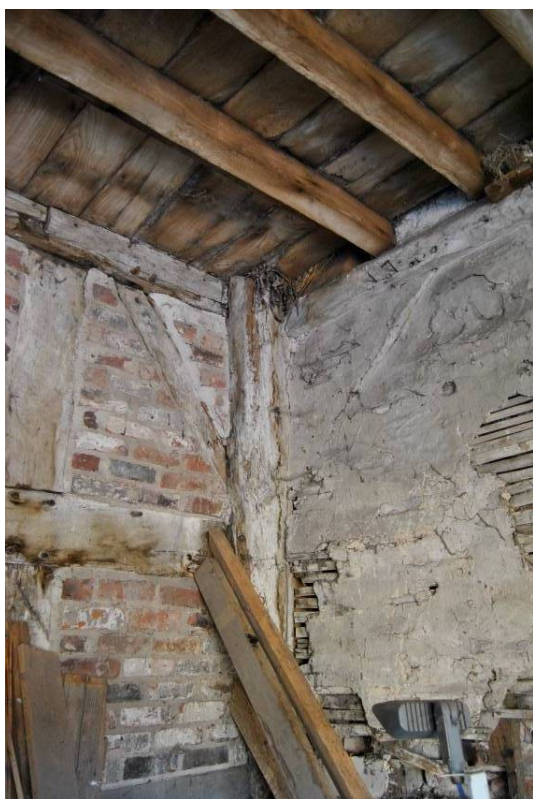
Plate 34: Primary south-east angle post with up-braces.
