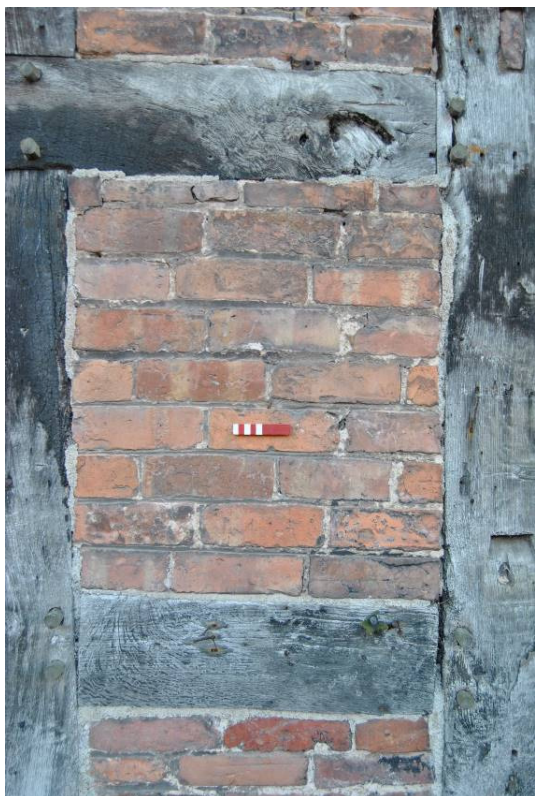
Plate 20: Brick nogging panel infill.
