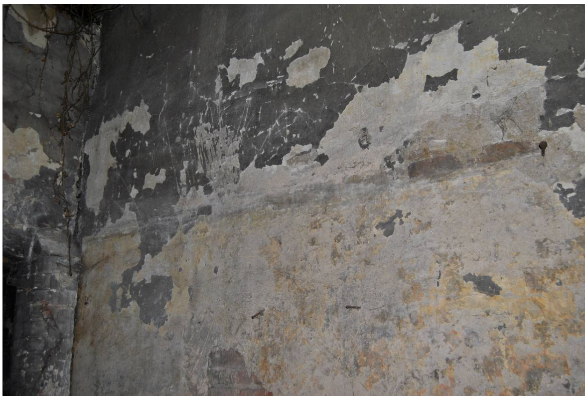
Plate 41: Line of former first floor evident in render of north wall.
