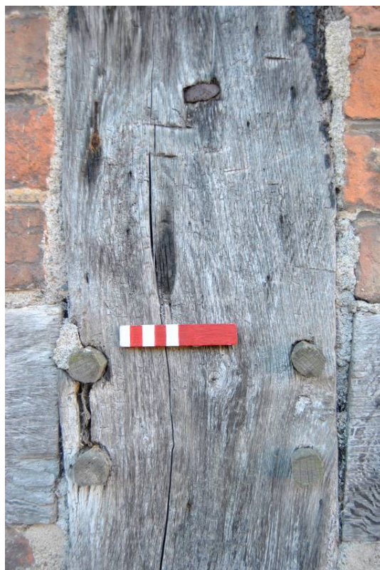
Plate 21: Taper mark on stud of north elevation.
