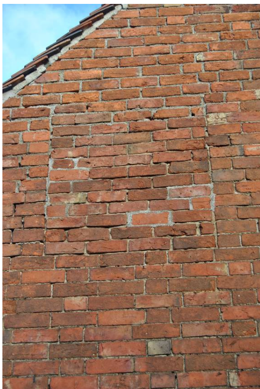
Plate 28: Blocked [w2] to upper south elevation.
