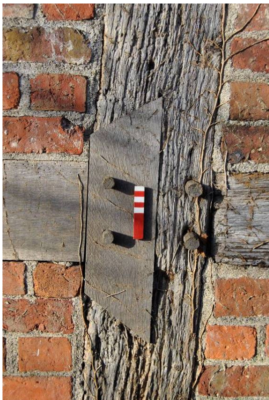
Plate 16: Face-plate repair at mid-rail joint.
