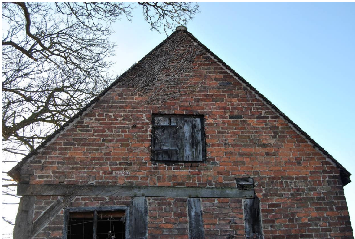
Plate 25: North elevation, brick gable (partly rebuilt).
