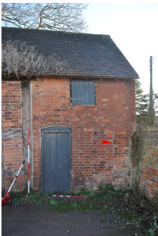
Plate 10: Door [d3] affording access to Phase III extension (NB. Straight joint marked with arrow)
