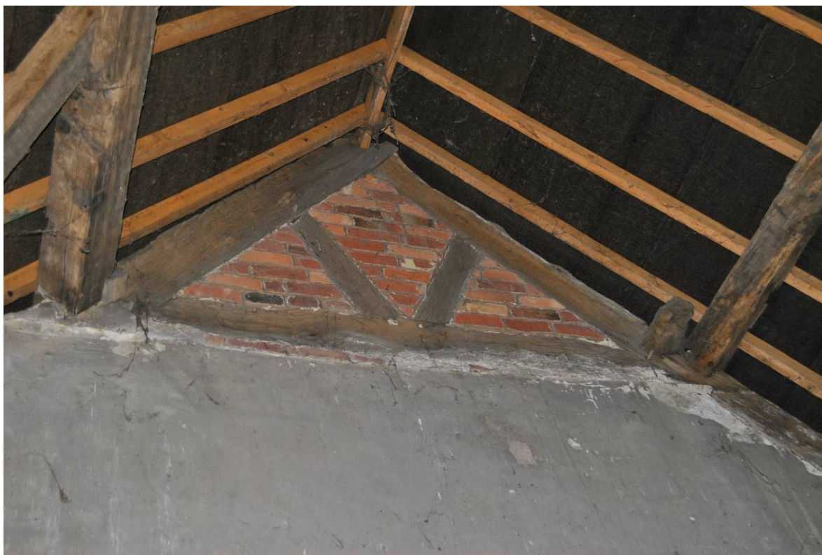
Plate 43: V-strutting above collar level of former Phase II gable end truss.
