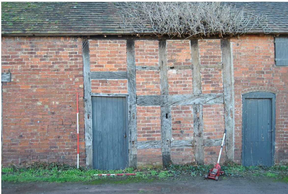
Plate 9: Surviving timber framing of Phase II extension with inserted [d2] accessing [G2].
