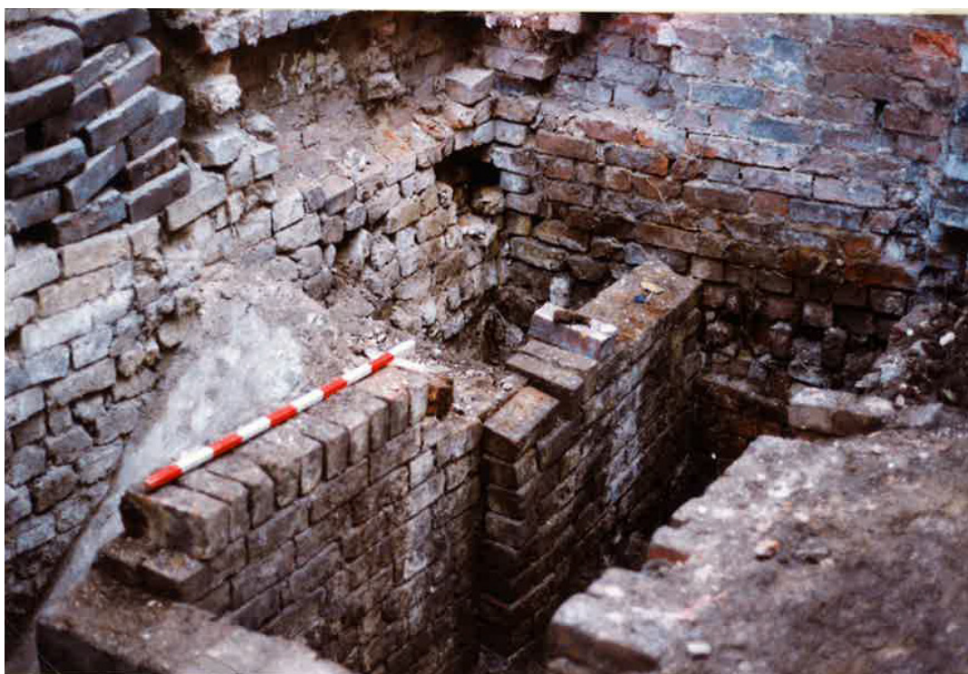
D.7: Detail of malt drying kiln beneath floor of [G3] exposed during conversion to garages, 1992.
