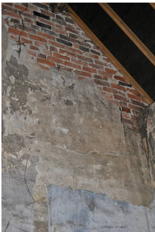
Plate 46: Window [w2] (blocked) to upper floor.
