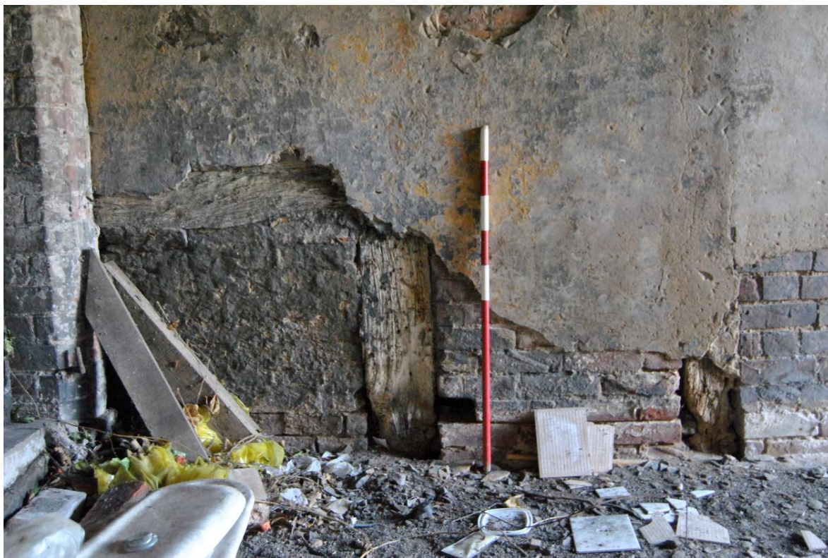
Plate 42: Phase II timber framing exposed at west end of north wall [G3].
