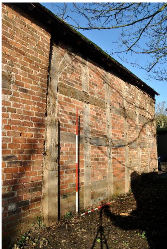
Plate 13: Primary timber framing of east elevation, north end.
