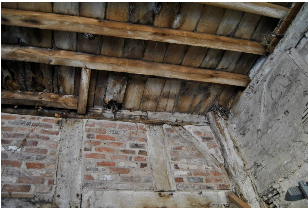
Plate 38: Trimmed former stair void at south-west corner of inserted floor structure.
