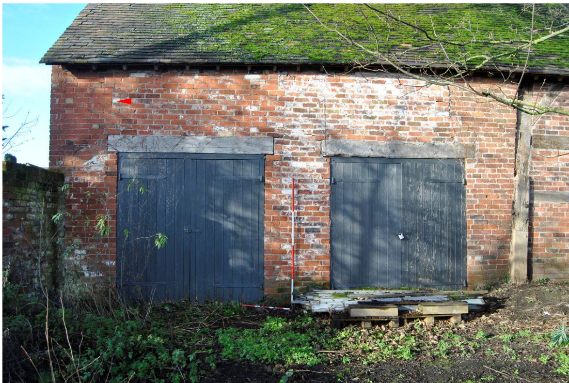
Plate 17: Inserted garage doors [d4/5] (1993) to south end of east elevation (NB. straight-joint marked with arrow).
