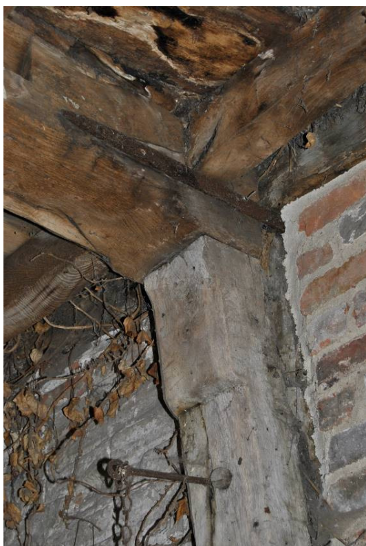
Plate 36: Main floor beam supported on applied bracket to east wall frame.
