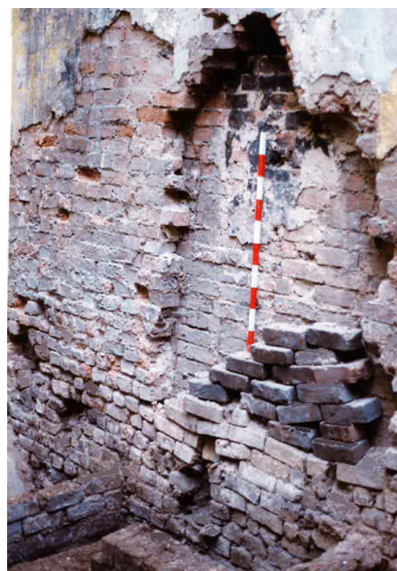
D.5: Former flue to south gable end, 1992.
