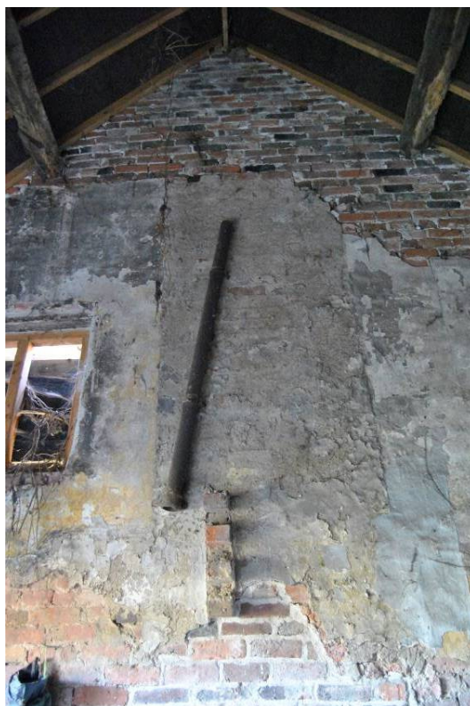
Plate 45: 'Ghost of former flue/stack against south wall; note vertical limit of plaster render.
