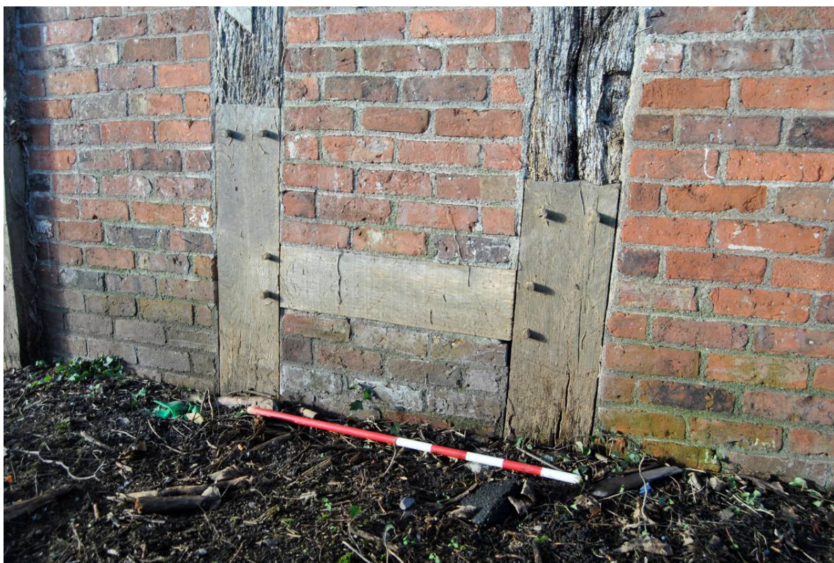
Plate 15: Secondary, face-plate repairs to base of vertical studs and replacement mid-rail.
