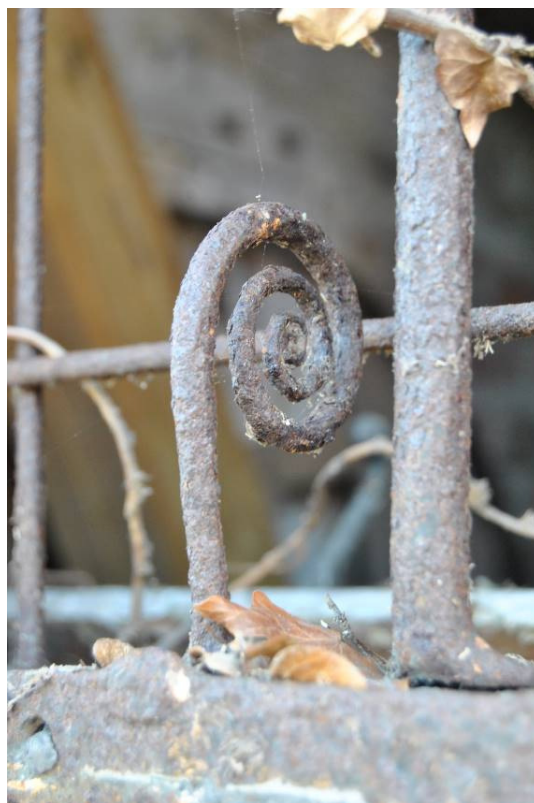
Plate 24: Spiral handle of window [w5].
