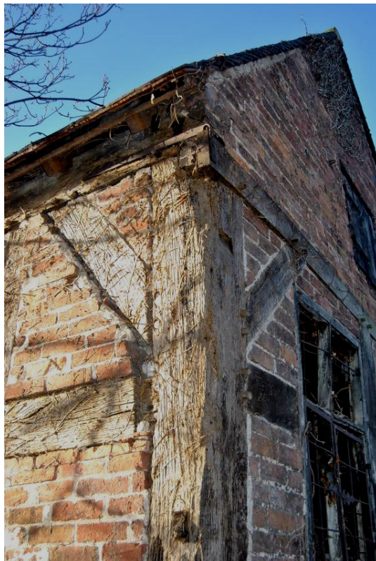
Plate 14: Up bracing to north-east angle.
