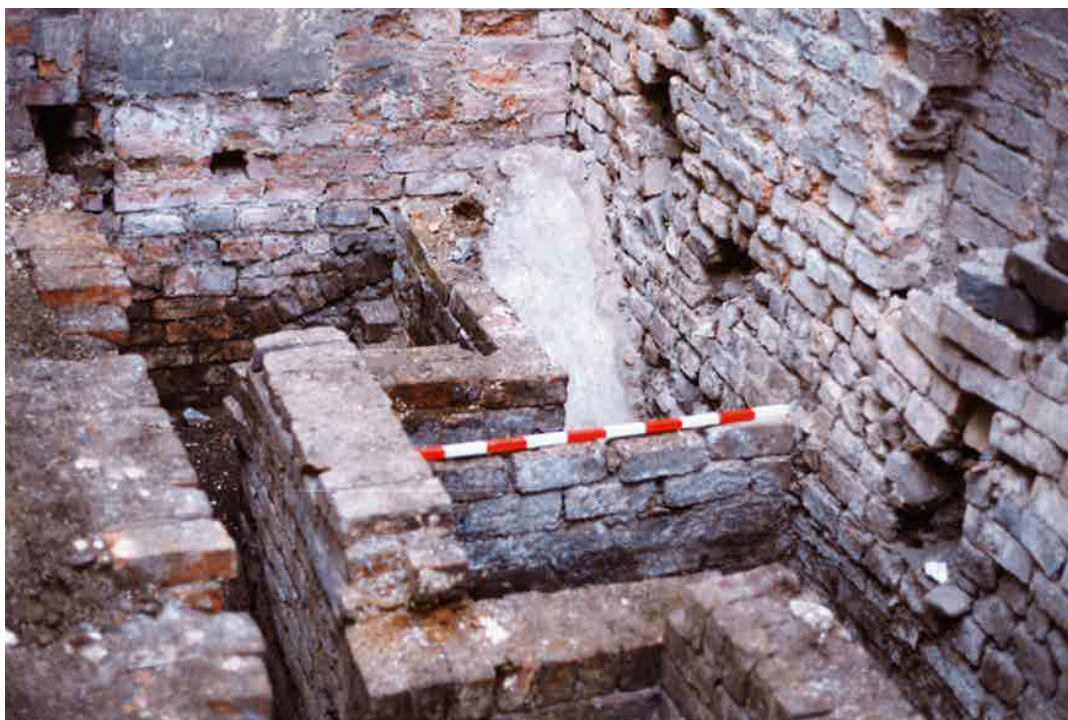
D.6: Detail of malt drying kiln beneath floor of [G3] exposed during conversion to garages, 1992.
