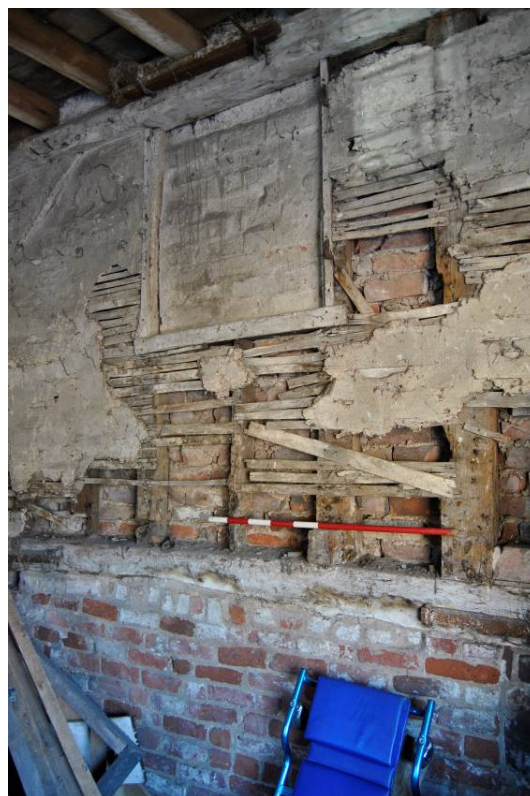
Plate 32: Studwork wall to south with lath and plaster
