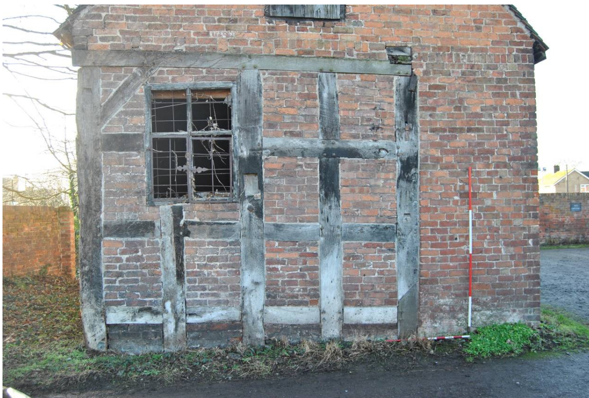
Plate 19: Exposed timber framing of Phase I elevation, rebuilt/underbuilt in brick to right (west), note soot blackening.
