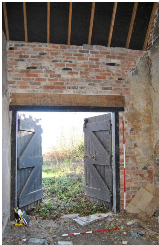
Plate 40: [G3], interior looking east with inserted door [d4].
