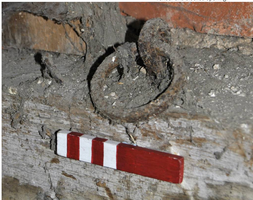
Plate 33: Tethering ring to timber cill, south wall of [G1].
