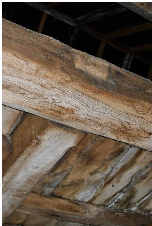
Plate 37: Empty mortice in west face of girder implying former continuation of floor structure.
