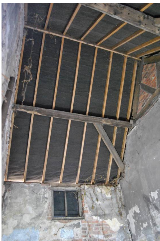
Plate 47: New roof structure.
