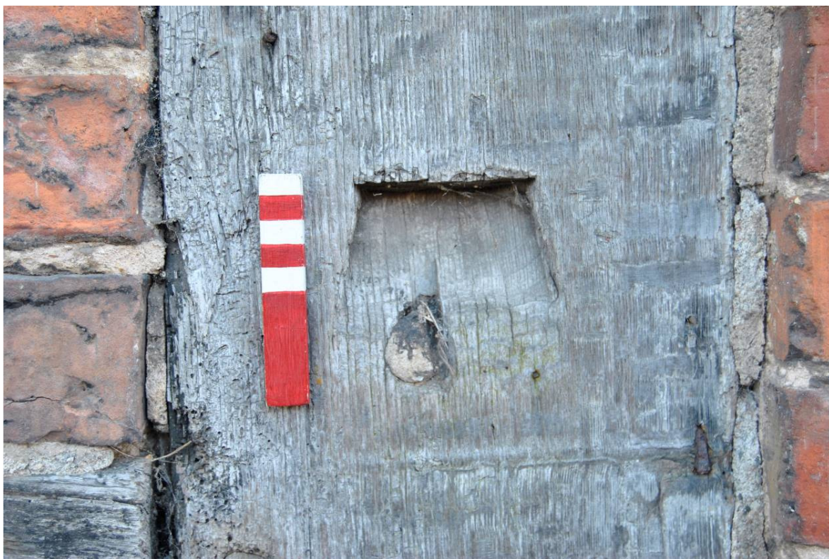
Plate 22: 'Scotch' within wall western wall-post of north elevation.
