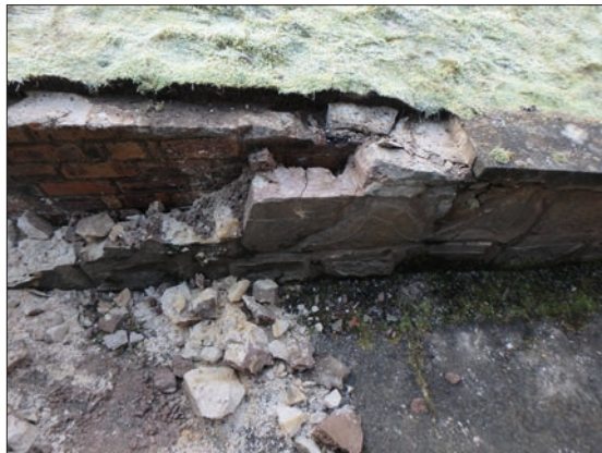
Plate 2: Retaining wall demolition.
