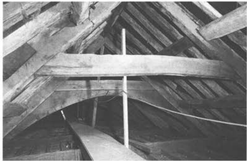
Figure 4.20 The north range roof looking west (photograph: English Heritage B870019/110).
