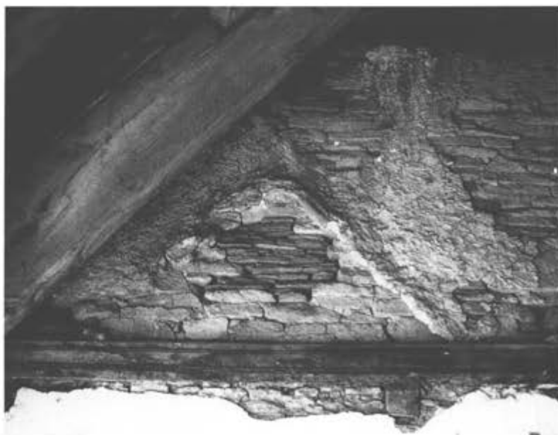
Figure 4.4 A pentice weathering preserved in the north range roof (photograph: Kirsty Rodwell).
