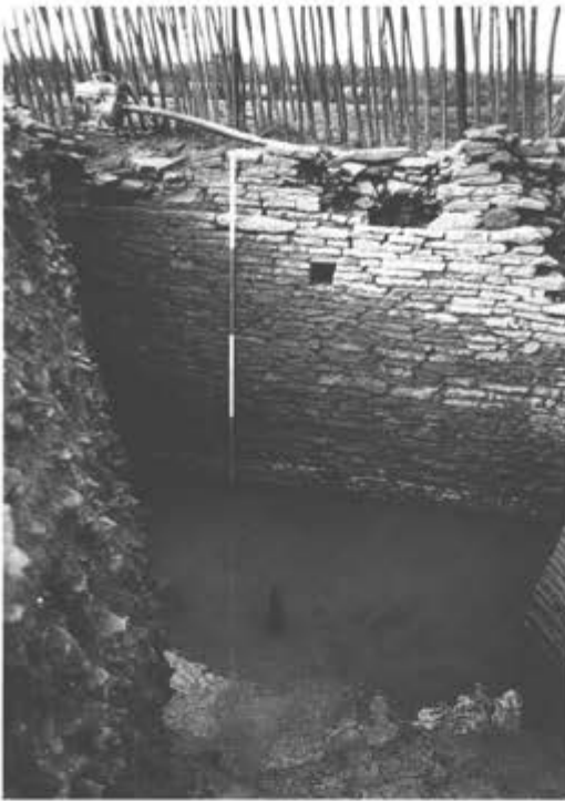
Figure 4.24 The west wall of the west range in the moat showing a scaffolding pole, from the east (photograph: Robert Bell).
