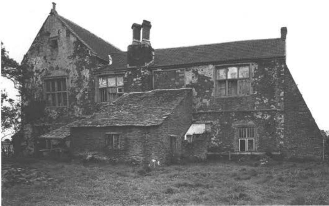
Figure 4.16 The north elevation of the house (E6) (photograph: © Crown copyright. NMR BB98/00597).
