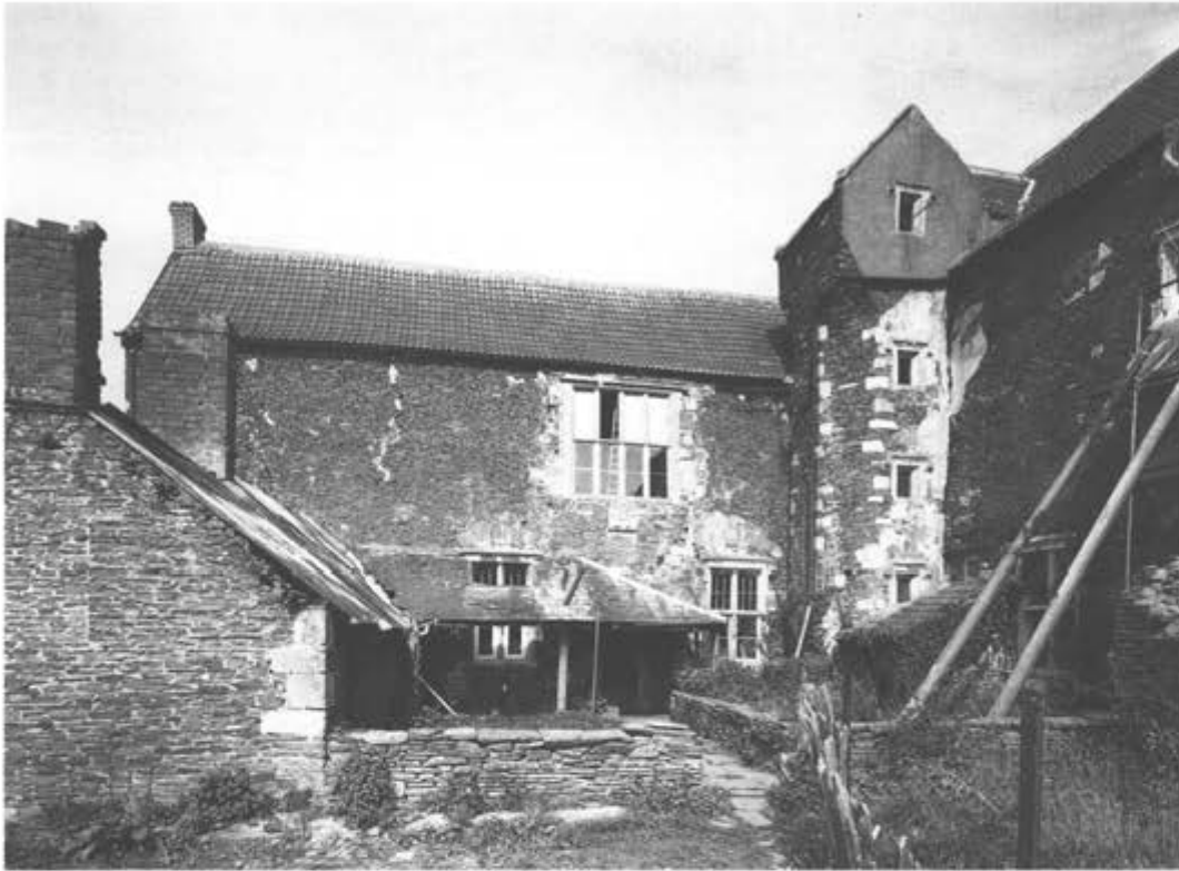
Figure 4.38 The courtyard elevation of the north range (E4)
