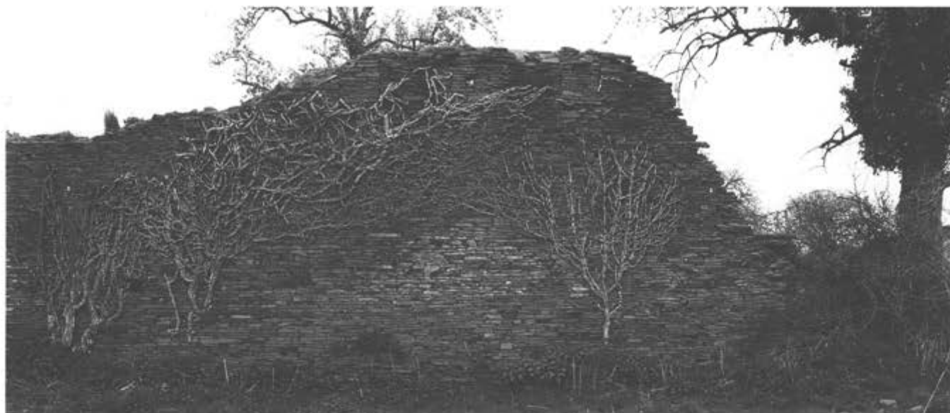
Figure 4.41 South court: the west wall with surviving crenellations. The demolished corner tower (Fig 4.43) is on the right of the picture (photograph: Photogrammetric Unit, Institute of Advanced Architectural Studies, University of York).
