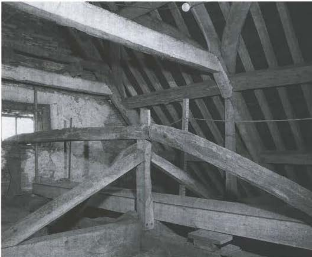
Figure 7.6 Brace in the east range roof (photograph: English Heritage B870019/41).
