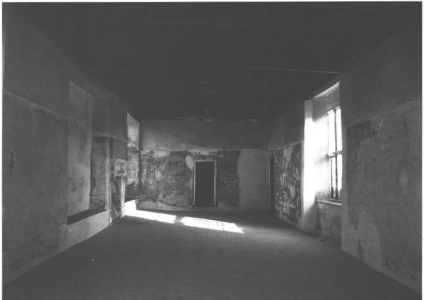
Figure 5.21 Room 1, long gallery, looking east (photograph: Kirsty Rodwell).
