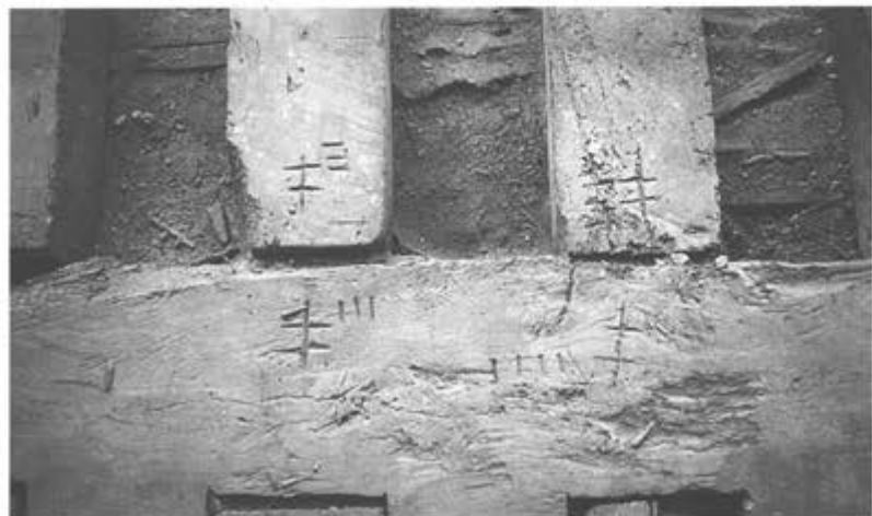
Figure 4.17 Carpenters' marks on floor joists in Room 1 (photograph: Kirsty Rodwell).
