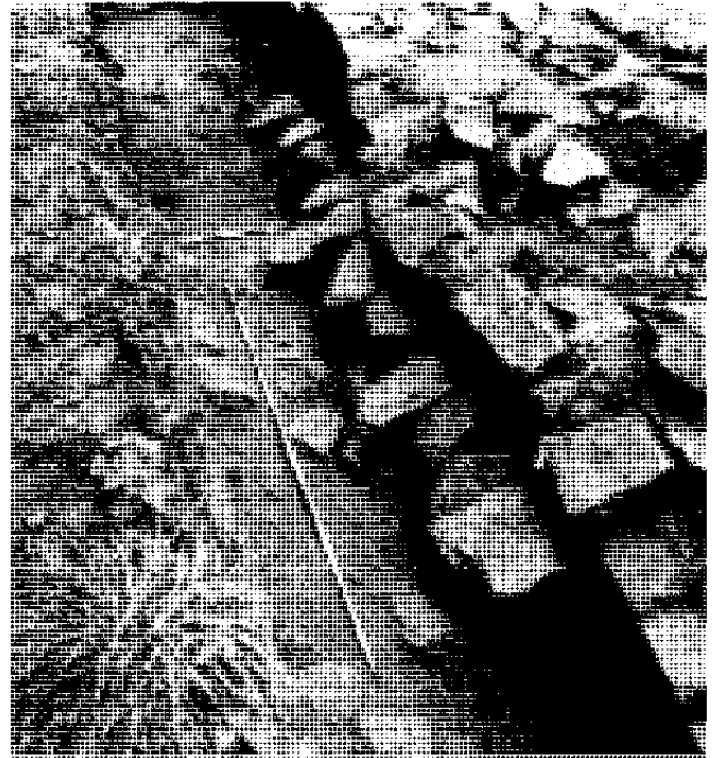
Fig 121 Section of slumping wall north of porta principalis sinistra , showing the surviving face of the late buttress (1634) inserted to support it
