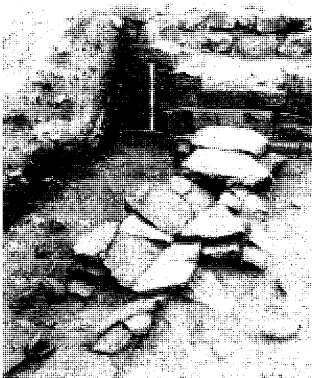
Fig 45 Drain 2546 leading to culvert in north wall of fort: the rampart section is visible to the left
