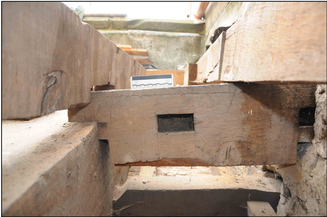
Appendix I.32: View of re-used struts along south wall of Section E (10cm scale) (Photo D166)
