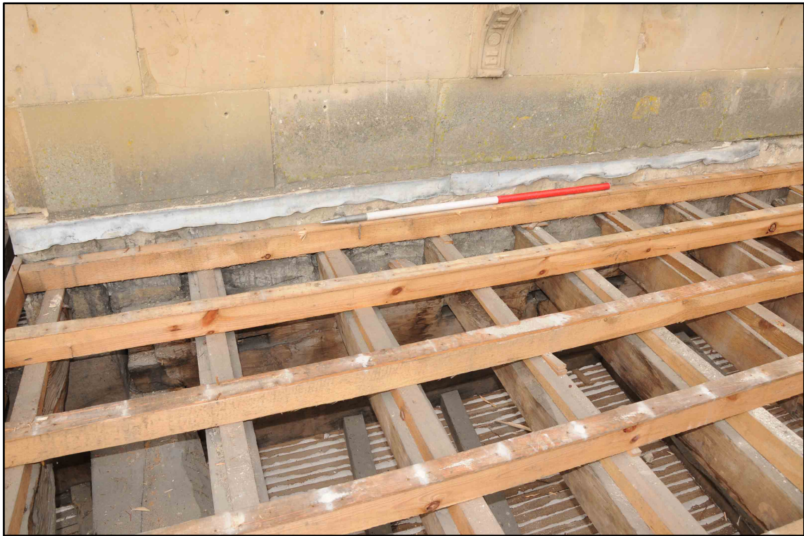
Appendix I.42: Inserted softwood timbers above oak beams in Section D (1m scale) (Photo D201)
