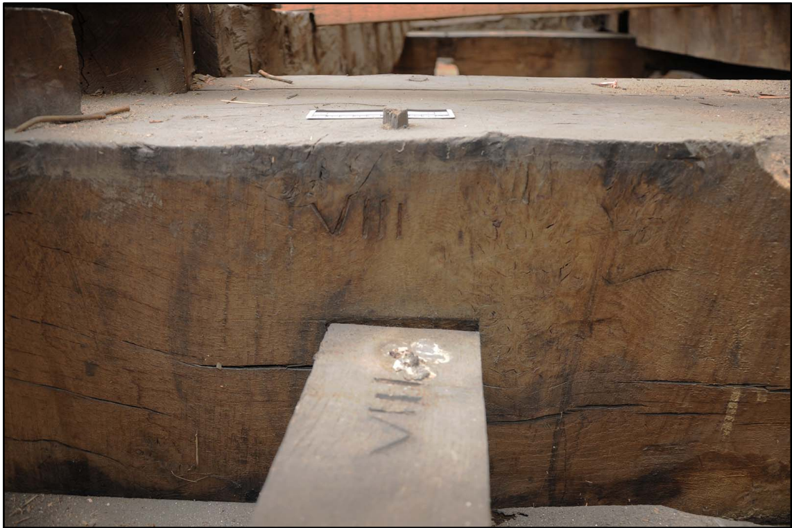
Appendix I.34: Detail of assembly marks 'VIII' for lower joist in Section E (10cm scale) (Photo D135)
