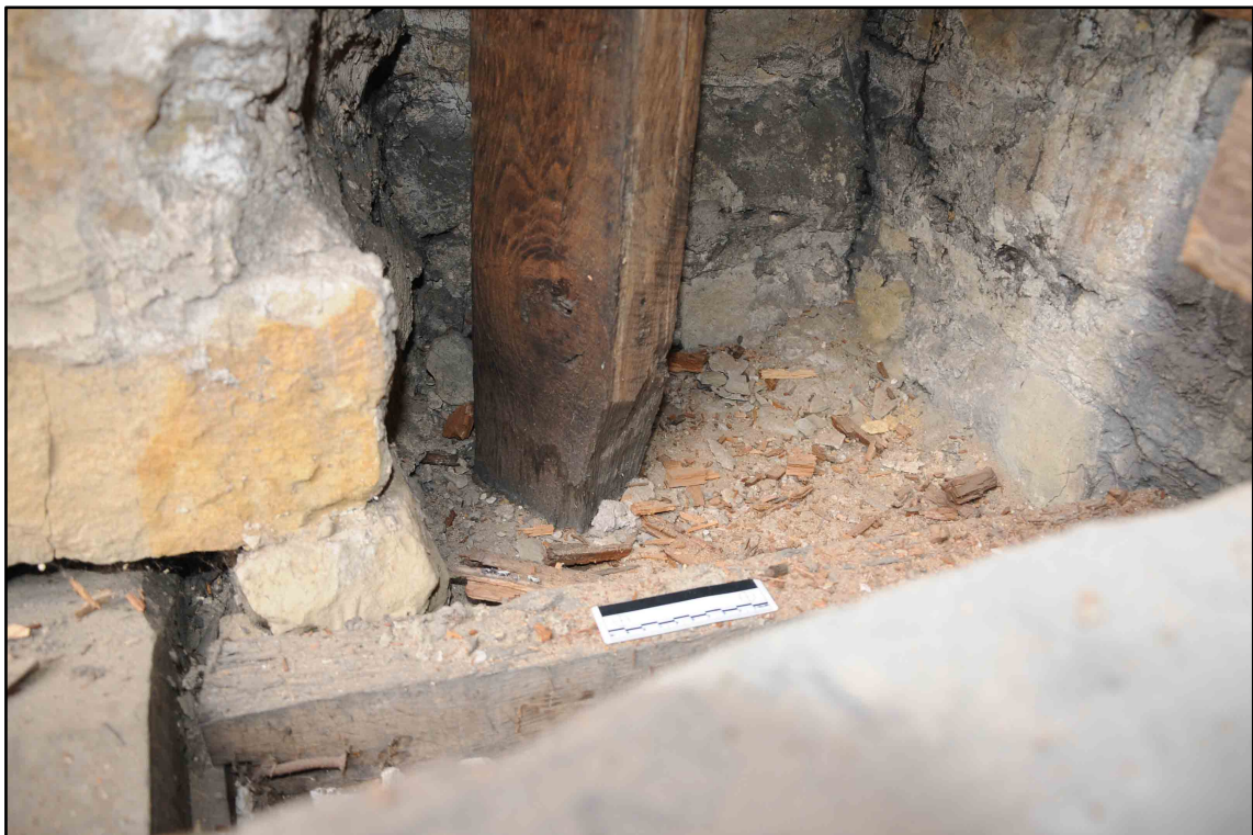
Appendix I.37: Oak post in square recess in south-west corner of Section E (10cm scale) (Photo D187)
