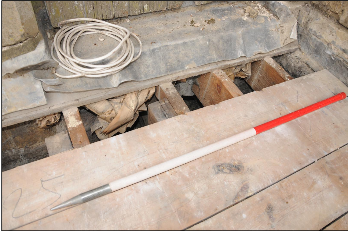
Appendix I.46: Detail of newspaper below pine boards in north-west corner (1m scale) (Photo D170)
