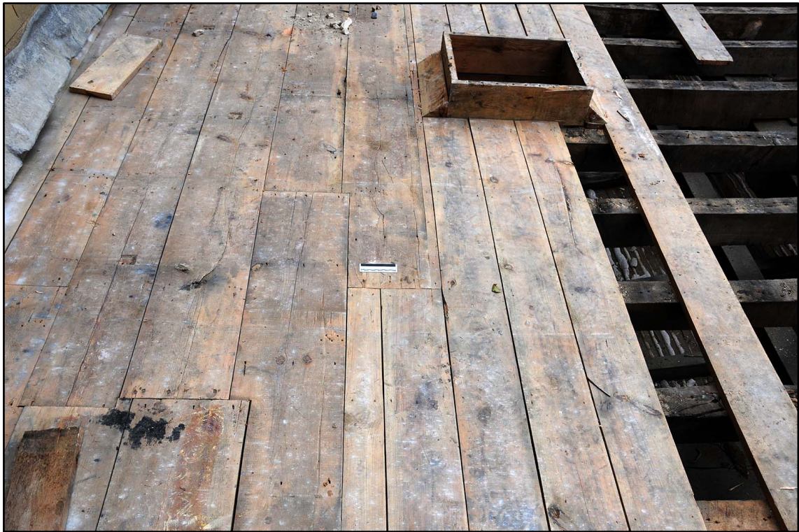
Appendix I.24: Pine boards in Section E; note two different widths (10cm scale) (Photo D124)
