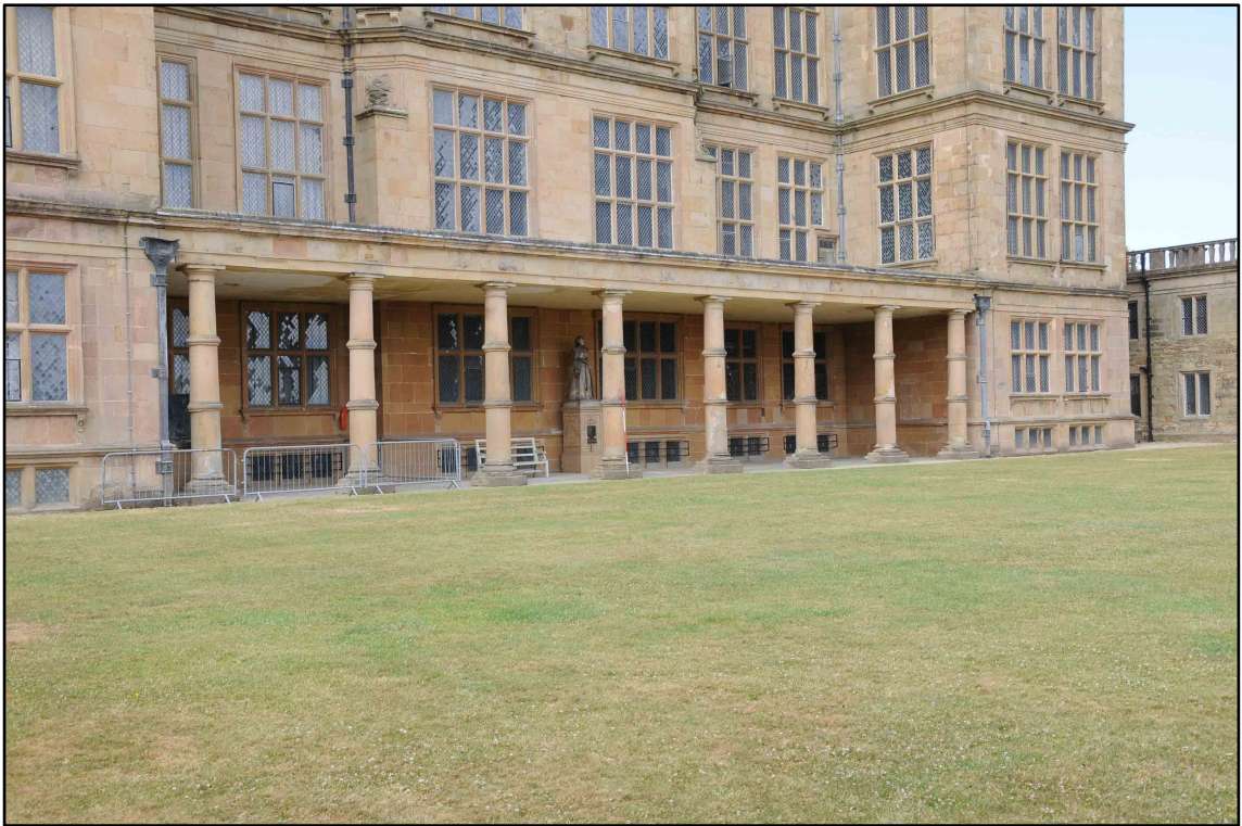
Appendix I.1: General view of the East Loggia, looking northwest (2m scale) (Photo D87)
