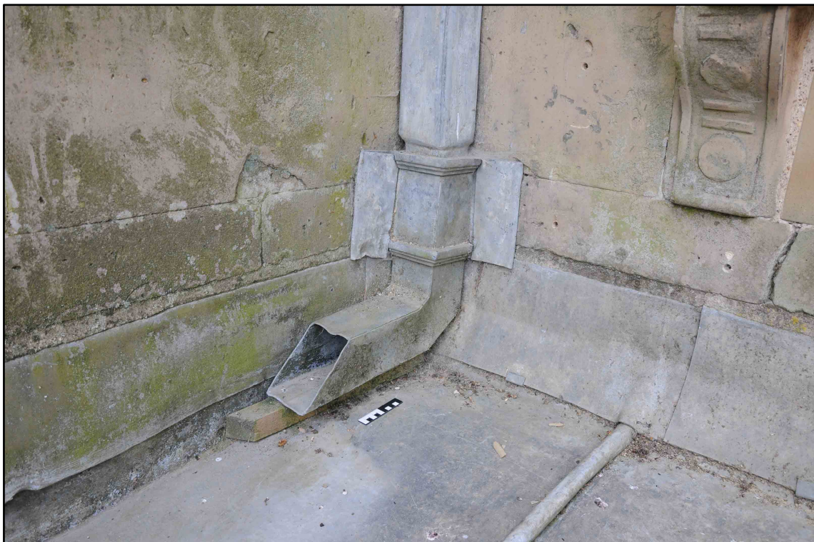
Appendix I.23: Detail of lead downpipe in southwest corner of Section E (10cm scale) (Photo D59)
