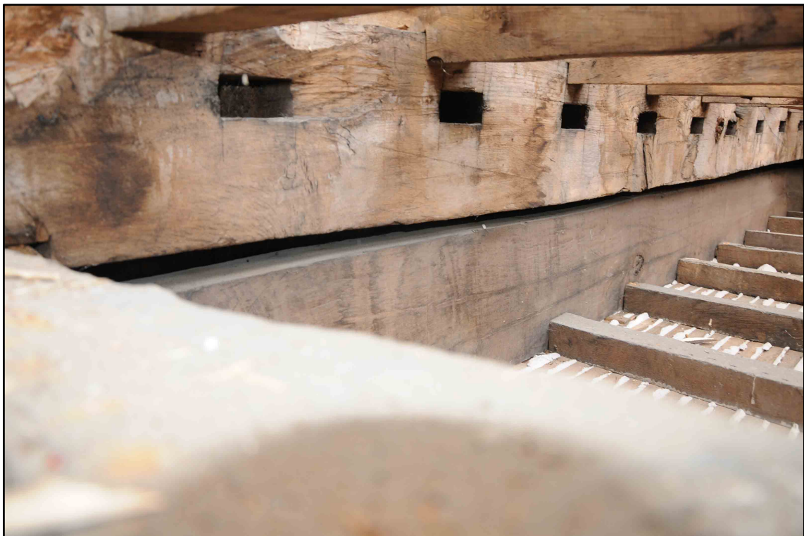
Appendix I.43: Reused timber floor beam along east wall of Hall in Section D (Photo D203)
