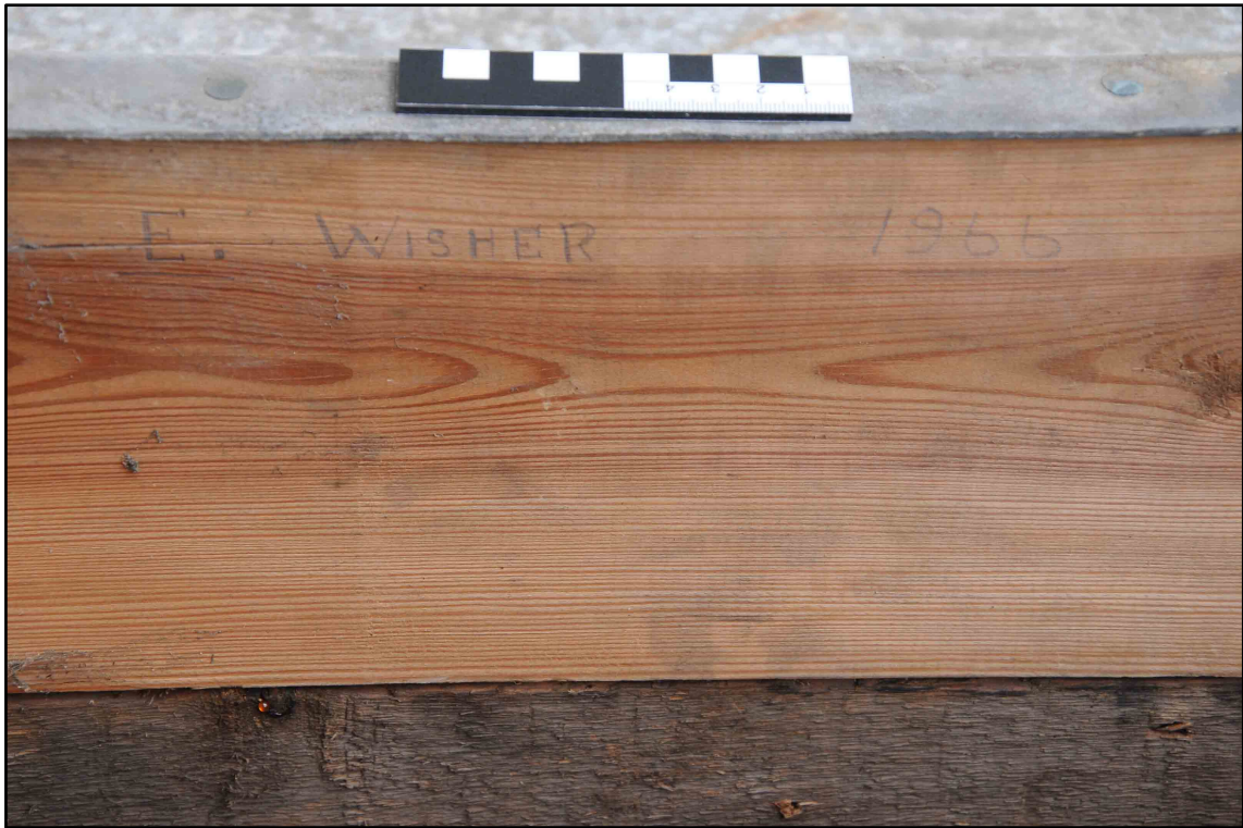
Appendix I.14: Graffiti in hatch in Section A 'E.Wisher 1966' (10cm scale) (Photo D25)
