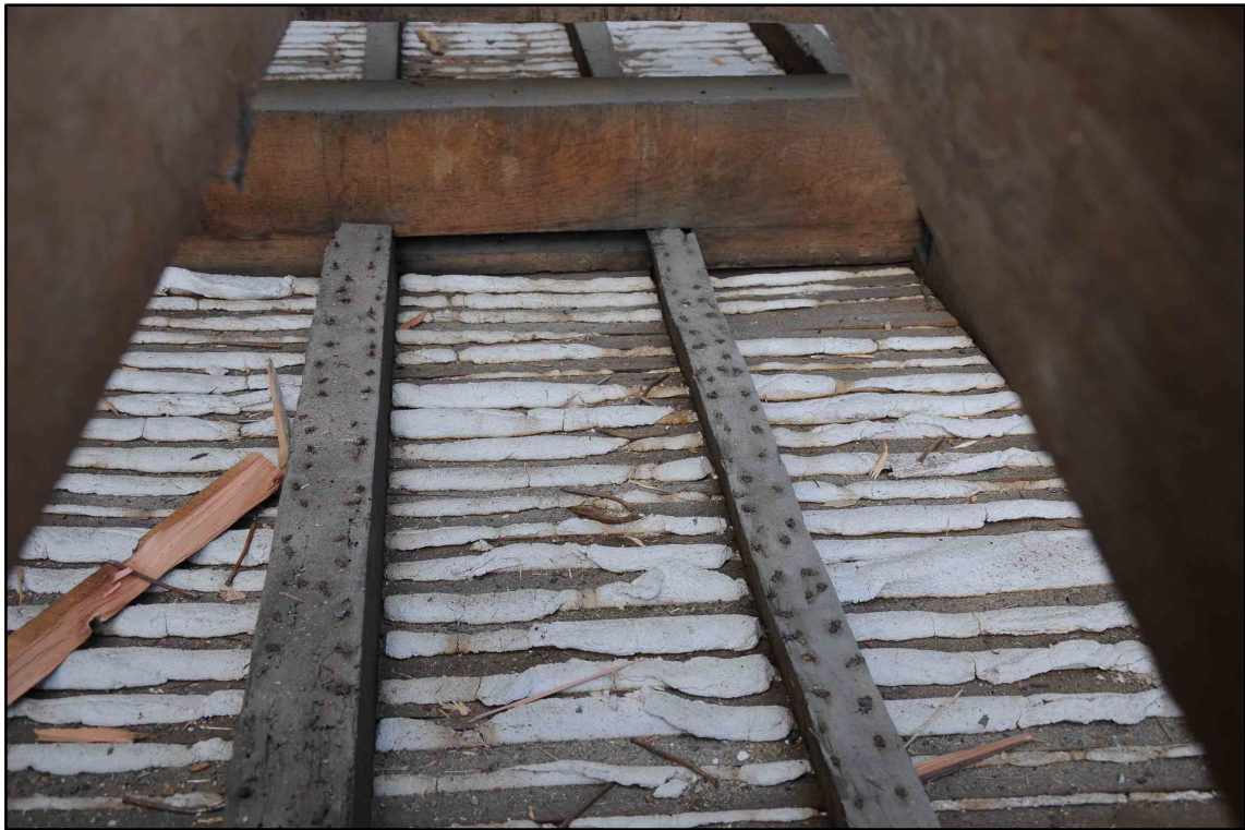
Appendix I.44: Detail of lath and plaster ceiling in Section E; note reused or rotated joists (Photo D207)
