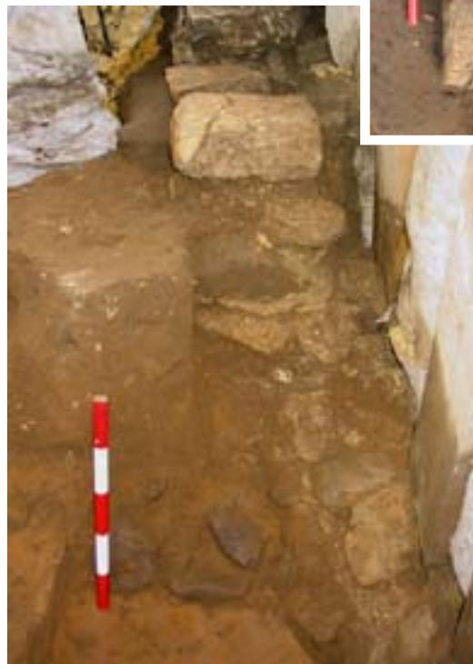
Fig. 23a (below): Southern aisle wall structure and foundation seen in section; Fig. 23b (inset) two oolitic limestone blocks, one interposed below an overhanging stone in the tower wall, viewed from above. Scale unit: 100 mm.
