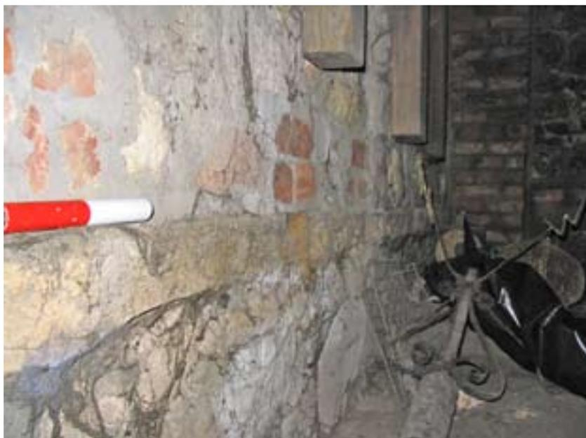
*Fig. 19: Possible wall plate, with the scale resting on its upper edge, in the internal north elevation of the tower. View looking east. Scale unit 100 mm.*
