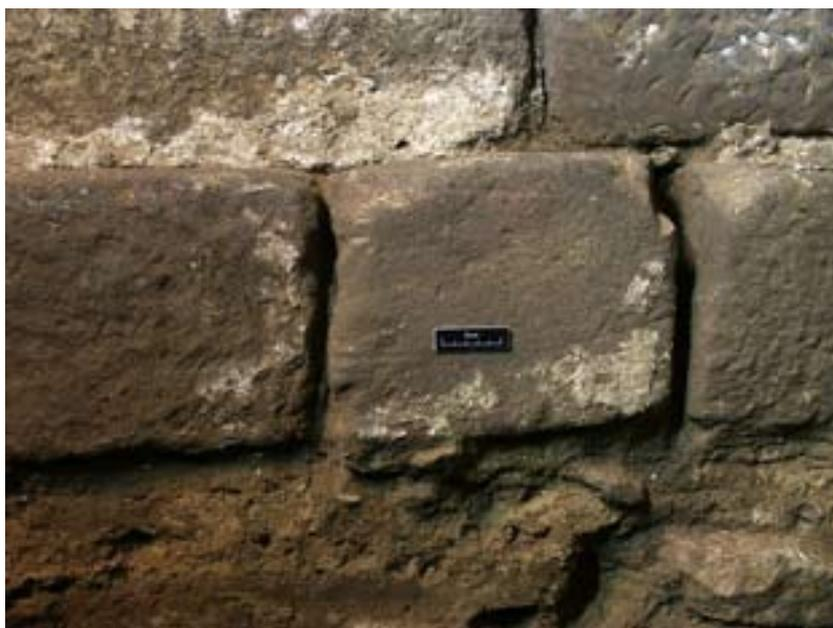
Fig. 10: Plaster/ render on internal face of re-used gritstone blocks in the foundation for the tower's west wall.
