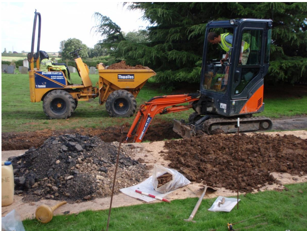
Plate 21 Southern soakaway showing spoil on boards for examination, looking east
