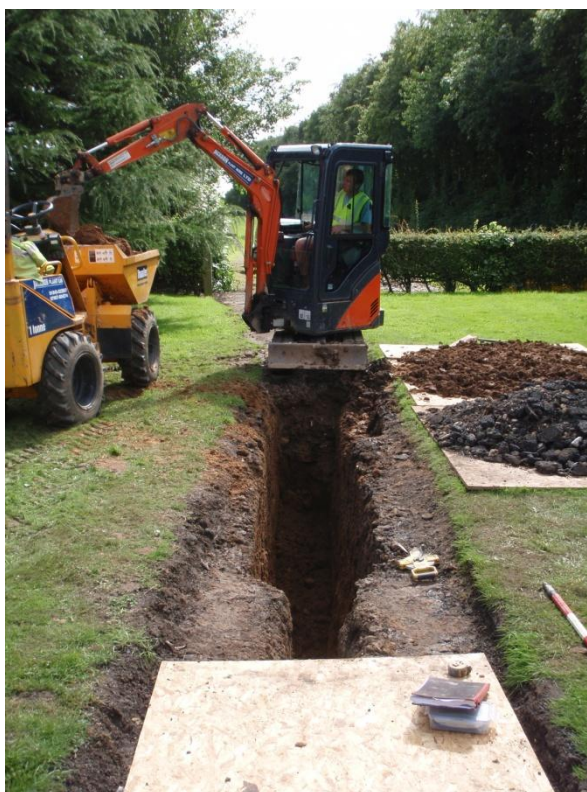
Plate 20 Southern soakaway, showing spoil on boards for examination, looking south
