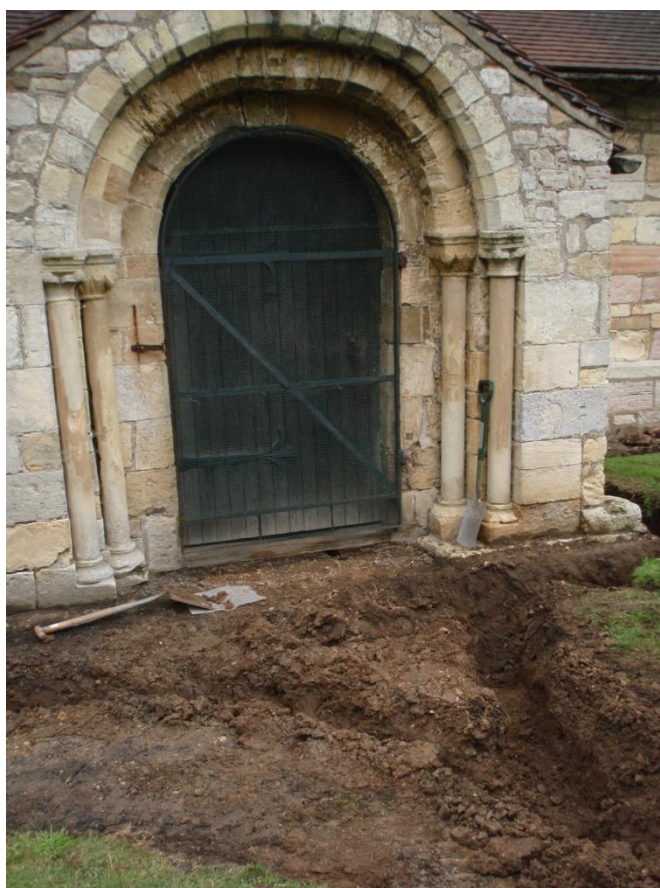
Plate 16 Confluence of drainage trench 2 in front of porch door, looking NNE
