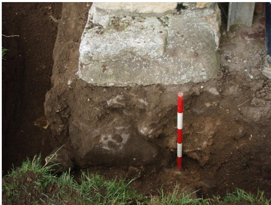
Plate 15 East facing section through porch foundations
