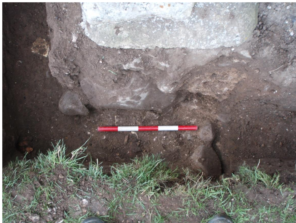
Plate 14 Porch foundations, disturbed by burials at c. 0.45m BGL, looking west
