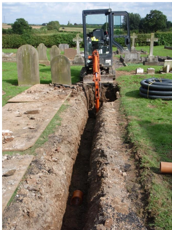
Plate 3 Trench 1 eastern end, looking east at the soakaway during excavation
