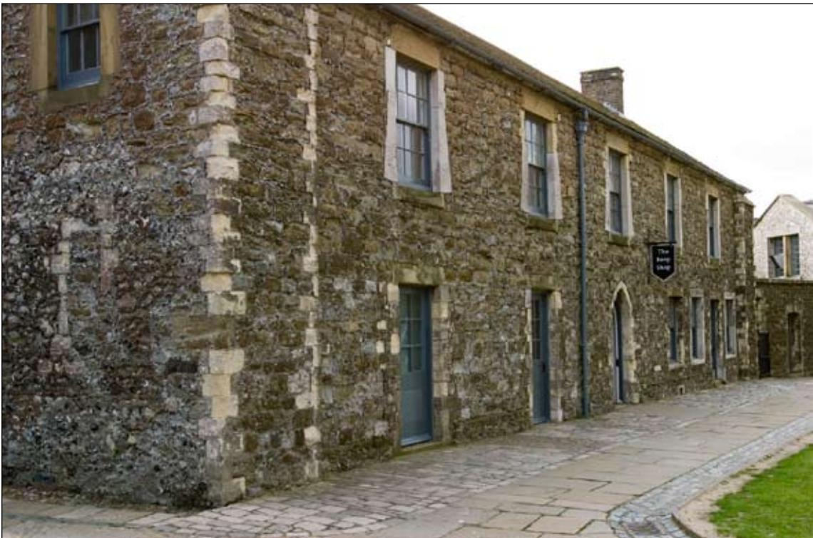
Figure 13. Arthur's Lesser Hall, now the shop. Rubble in the gable end and the lower walling of the façade contrasts with regular stonework at higher levels
