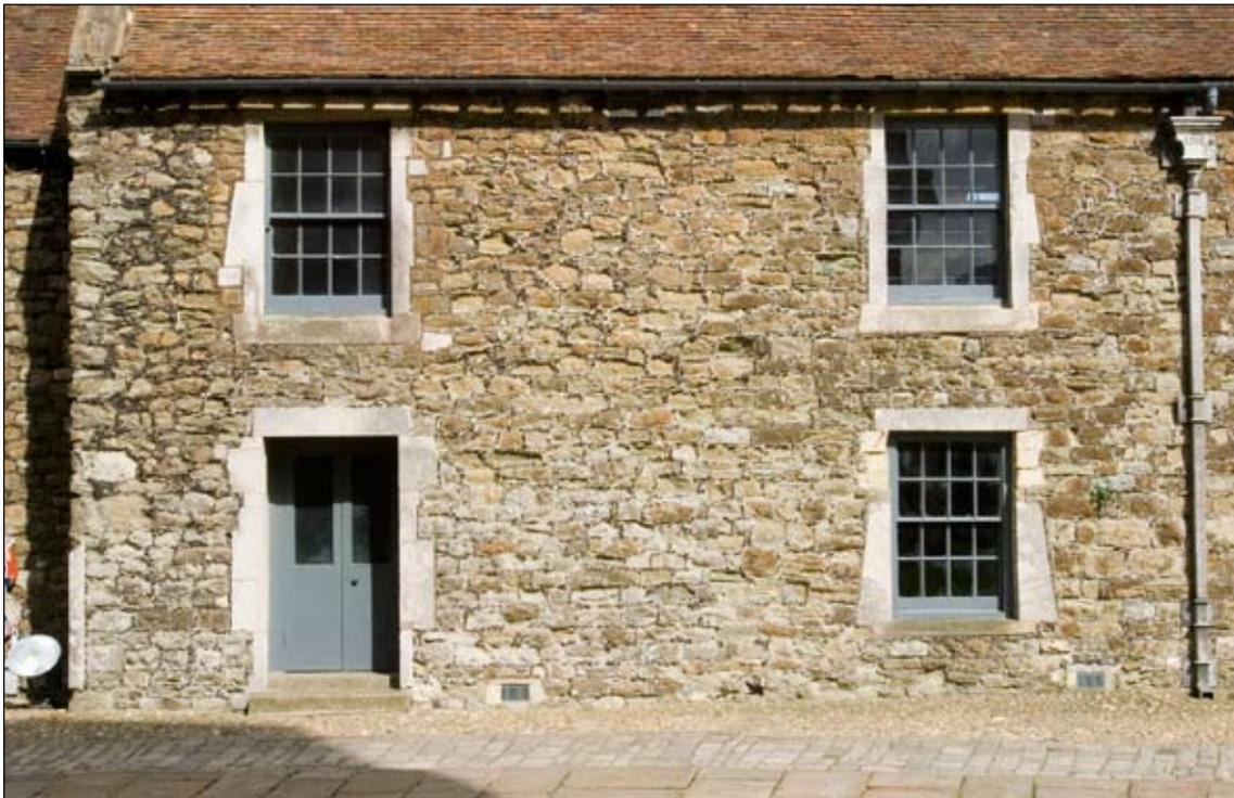
*Figure 10. Joint between medieval rubble and regular 18th-century walling, to the left of the right-hand sashes*
