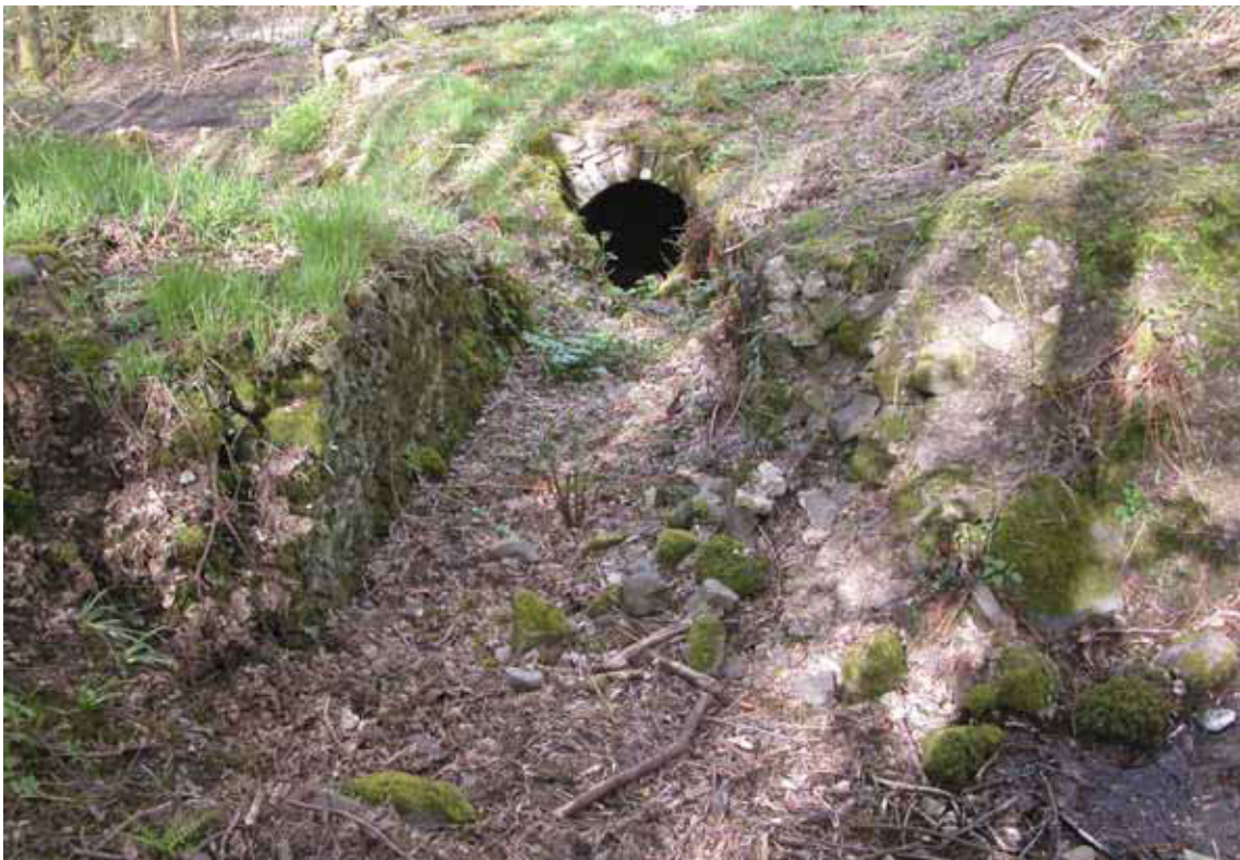
Figure 11: The sloping culvert looking west (downhill) (Photograph: Christopher Dunn 2006, © English Heritage)
