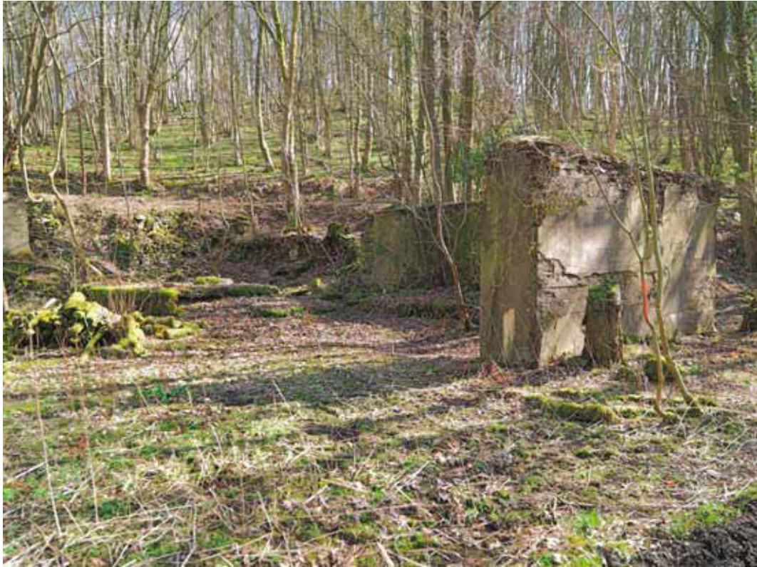
Figure 49: The southern end of the platform for the large corning house (building 12) shielded by blast walls BW2 and BW3 (Photograph: Bob Skingle 2006, DP028050 © English Heritage.NMR)
