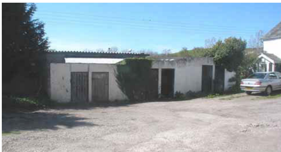
Figure 128: Ancillary block at Nos. 9-16 Gatebeck (Photograph: Simon Taylor 2006, © English Heritage)
