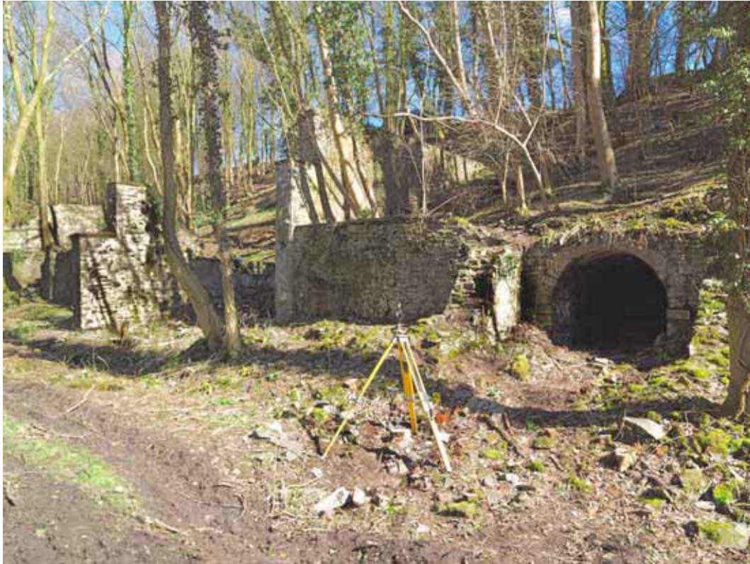
Figure 47: The southern charge house (building 2) from the west (Photograph: Bob Skingle 2006, DP028064 © English Heritage.NMR)
