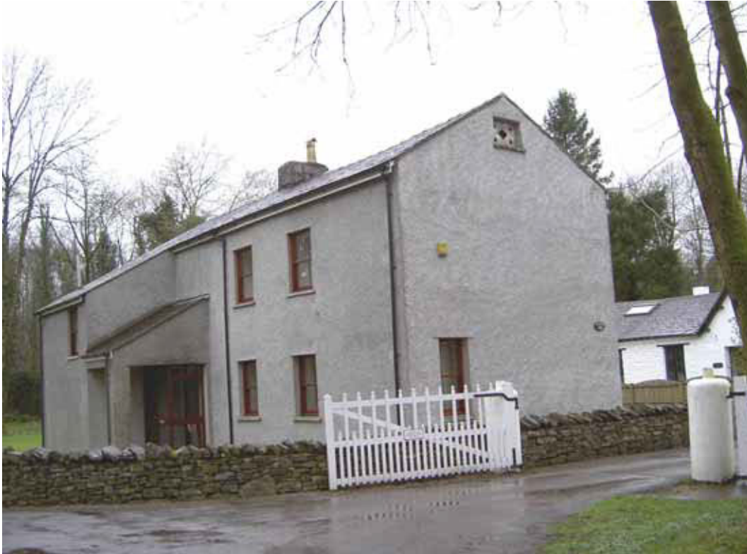
Figure 100: Millbrook House (formerly building 35: laboratory, store and tailor's shop or office), from the north-east (Photograph: Christopher Dunn 2005, © English Heritage)
