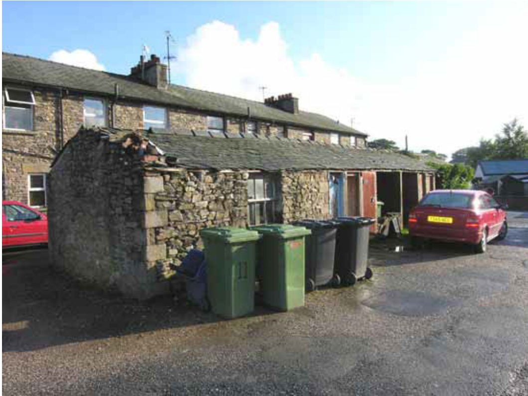
Figure 117: Peat and washhouses behind Nos. 7-12 Woodside, Endmoor (Photograph: Simon Taylor 2006, © English Heritage)
