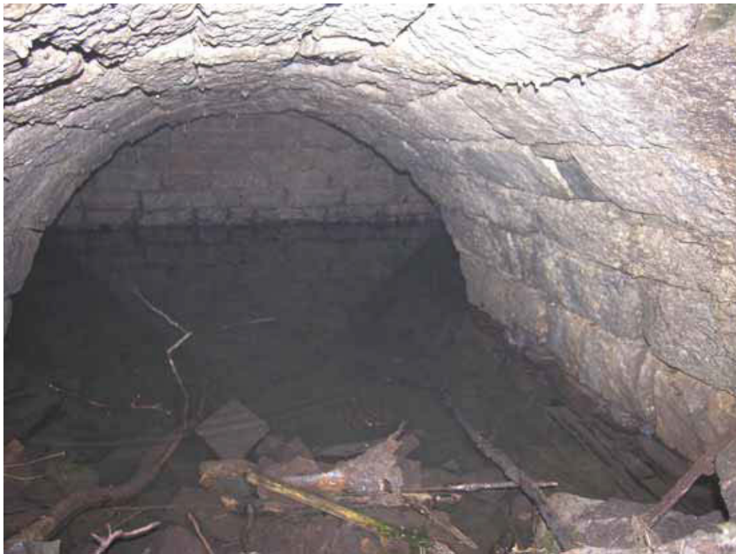
Figure 33: The tailrace from incorporating mill 3, showing its junction with the low-level culverted leat (Photograph: Marcus Jecock 2008, © English Heritage)
