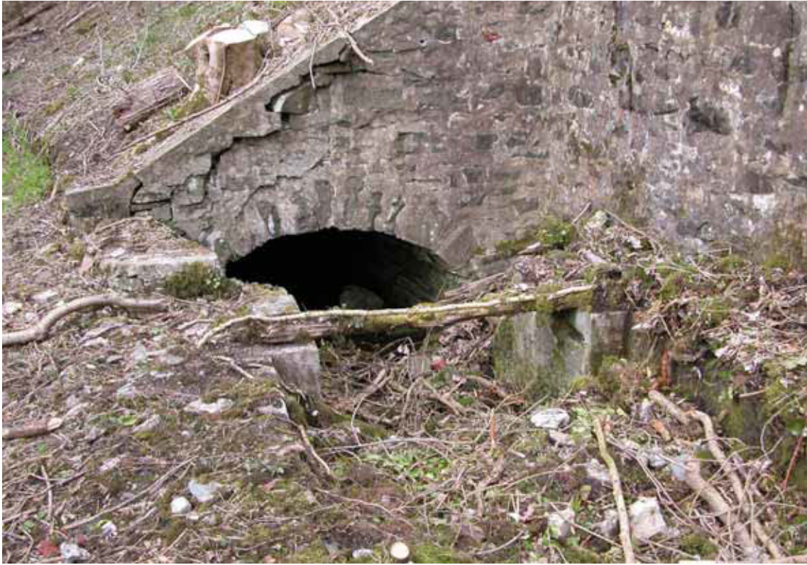
Figure 12: The short open-air section of the high-level culverted leat north of incorporating mill 7 (Photograph: Christopher Dunn 2006, © English Heritage)
