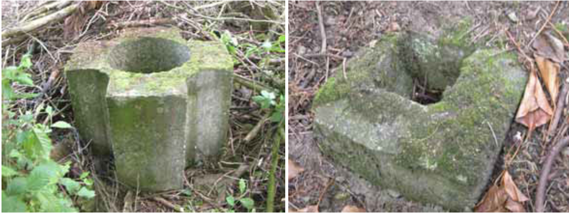
Figure 76 (above left): Concrete block at site of cartridge-pressing house 49 Figure 77 (above right): Concrete post-support behind cartridge-pressing house 50 (Photographs: Christopher Dunn 2006, © English Heritage)
