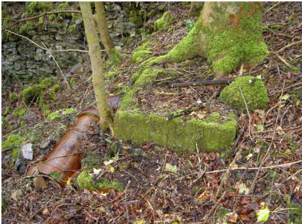
Figure 50: Concrete base with securing bolts, possibly part of the mark I engine-house flue (Photograph: Christopher Dunn 2006, © English Heritage)
