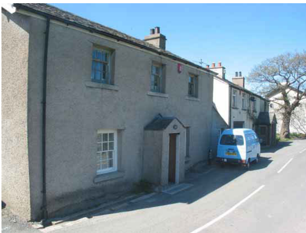
Figure 123: Front elevations of Nos. 5-6 Gatebeck (Photograph: Simon Taylor 2006, © English Heritage)
