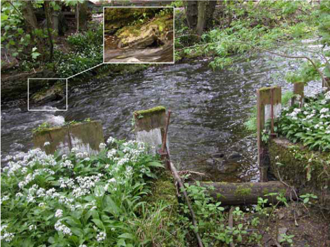
Figure 6: The pre-gunpowder weir (far side shown in detail at inset) and start of the headrace (Photograph: Christopher Dunn 2006, © English Heritage)
