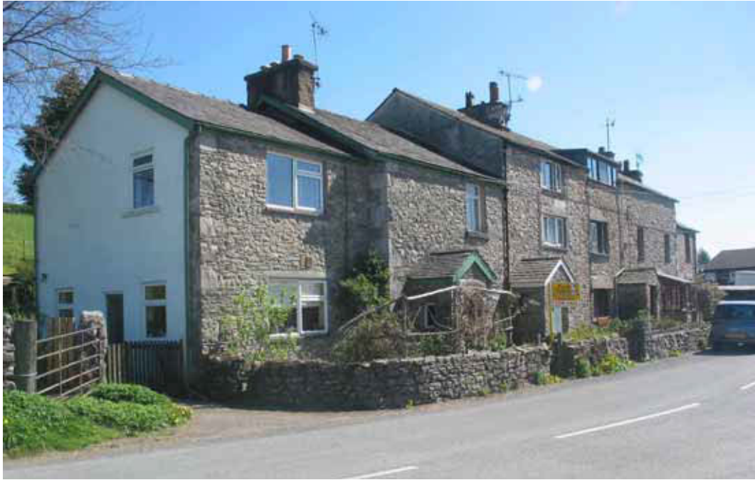
Figure 122: Front elevations of Nos. 1-4a Gatebeck (Photograph: Simon Taylor 2006, © English Heritage)
