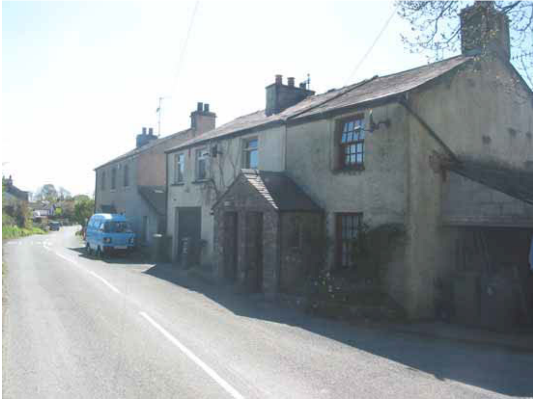
Figure 124: Front elevations of Nos. 7-8 Gatebeck (Photograph: Simon Taylor 2006, © English Heritage)
