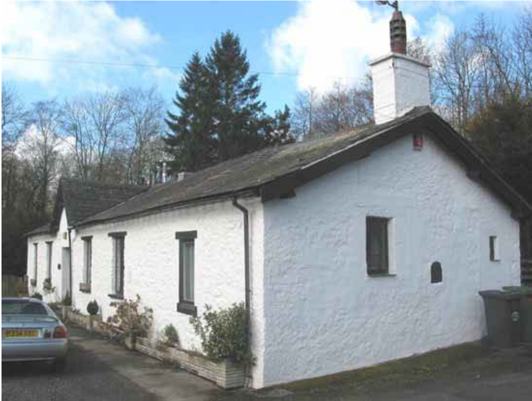
Figure 101: Millbrook Cottage (formerly building 36: office) from the north-east (Photograph: Simon Taylor 2006, © English Heritage)
