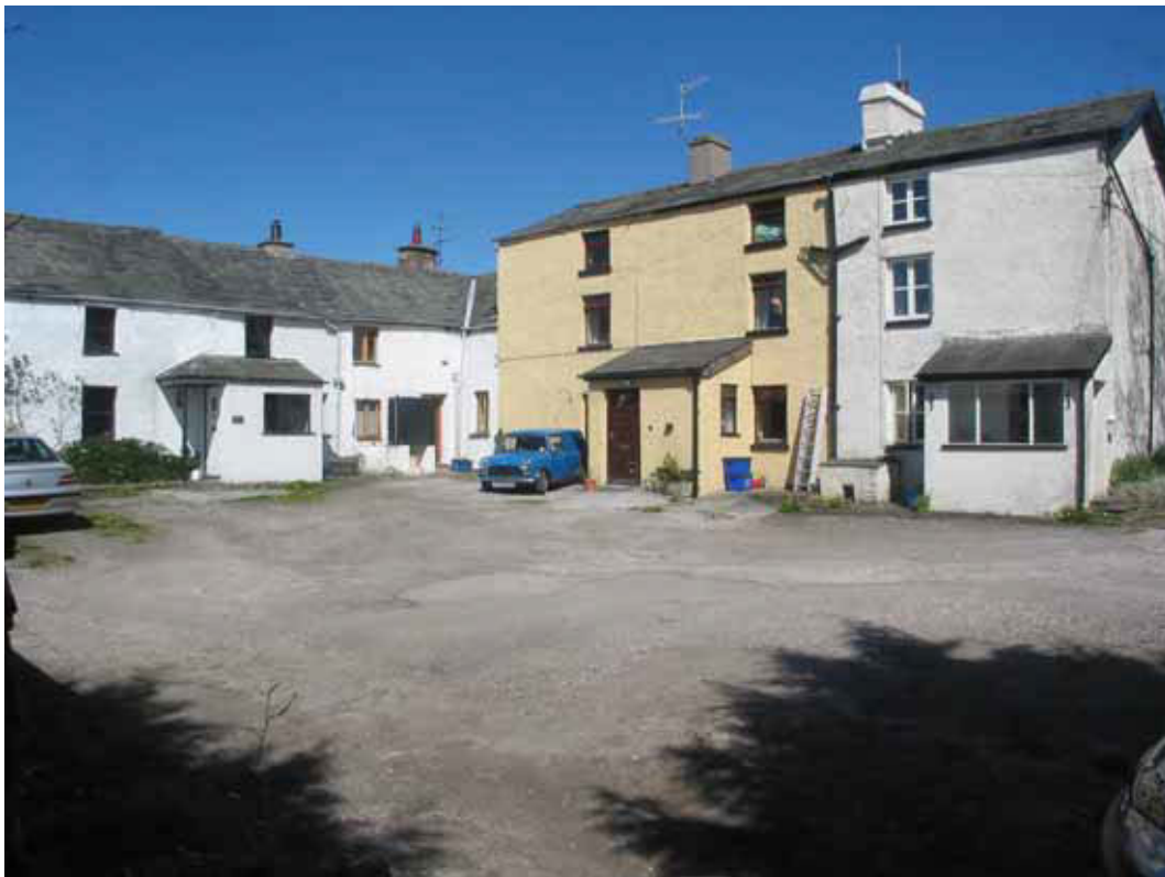
Figure 127: Rear elevations of Nos. 9-11 Gatebeck and south elevations of Nos. 12-14 (Photograph: Simon Taylor 2006, © English Heritage)
