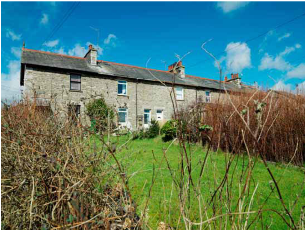
Figure 114: Front elevations of Nos. 1-6 Woodside, Endmoor (Photograph: Bob Skingle 2006, DP028034 © English Heritage.NMR)
