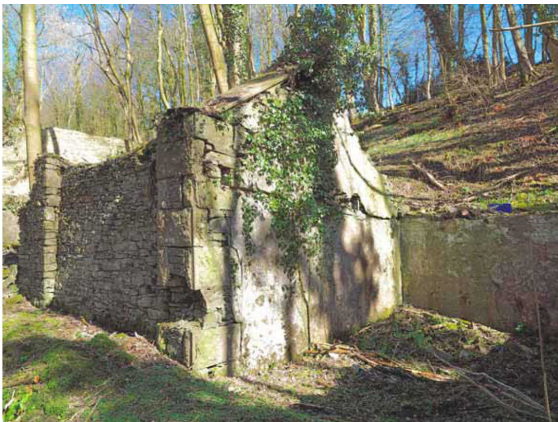
Figure 24: The north chamber of incorporating mill 3 and retaining wall to the north Photograph: Bob Skingle 2006, DP028069 © English Heritage.NMR)
