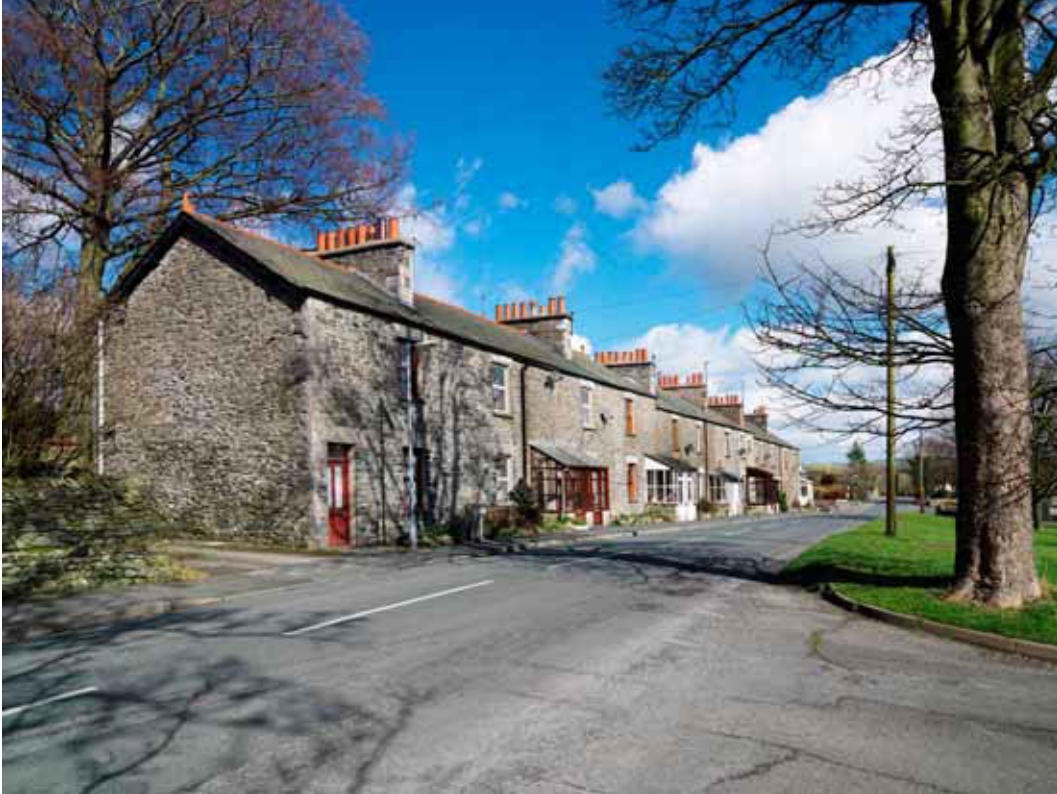
Figure 113: Front elevations of Woodside Terrace, Endmoor (Photograph: Bob Skingle 2006, DP028033 © English Heritage.NMR)
