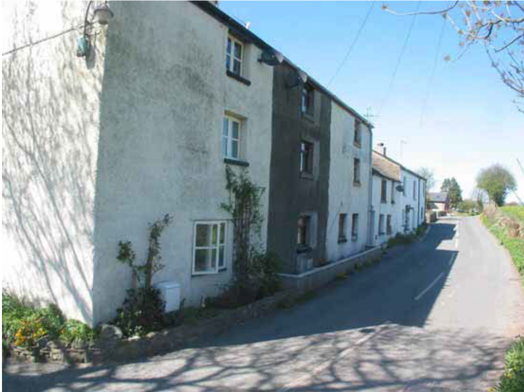
Figure 126: Front elevations of Nos. 9-11 Gatebeck (Photograph: Simon Taylor 2006, © English Heritage)
