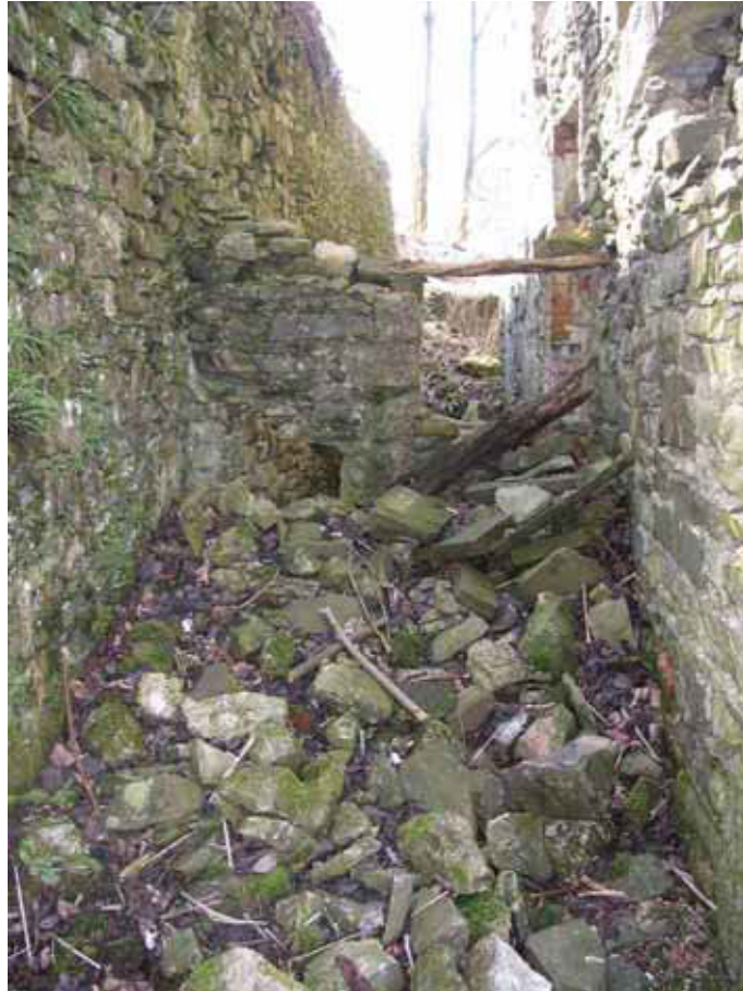
Figure 85: Roofed lean-to behind sawmill/mechanics' shop, used as a line-shaft alley (Photograph: Simon Taylor 2006, © English Heritage)
