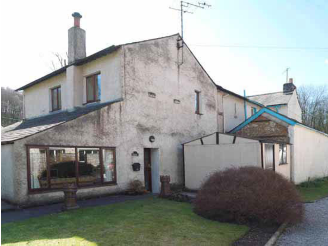
Figure 104: September Cottage (formerly building 33: stables), from the north (Photograph: Bob Skingle 2006, DP028045 © English Heritage.NMR)
