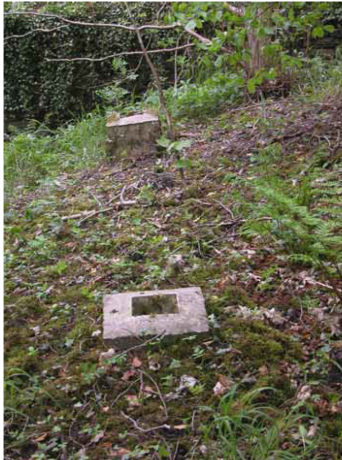
Figure 57: Post-supports for blast screen along tram embankment (Photograph: Christopher Dunn 2006, © English Heritage)
