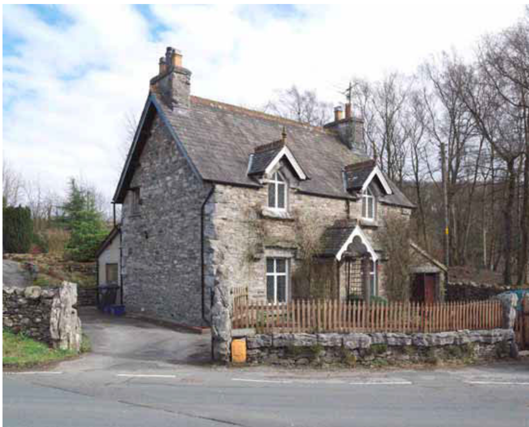
Figure 102: Holmleigh (formerly building 48: cottage), from the north-west (Photograph: Bob Skingle 2006, DP028092 © English Heritage.NMR)
