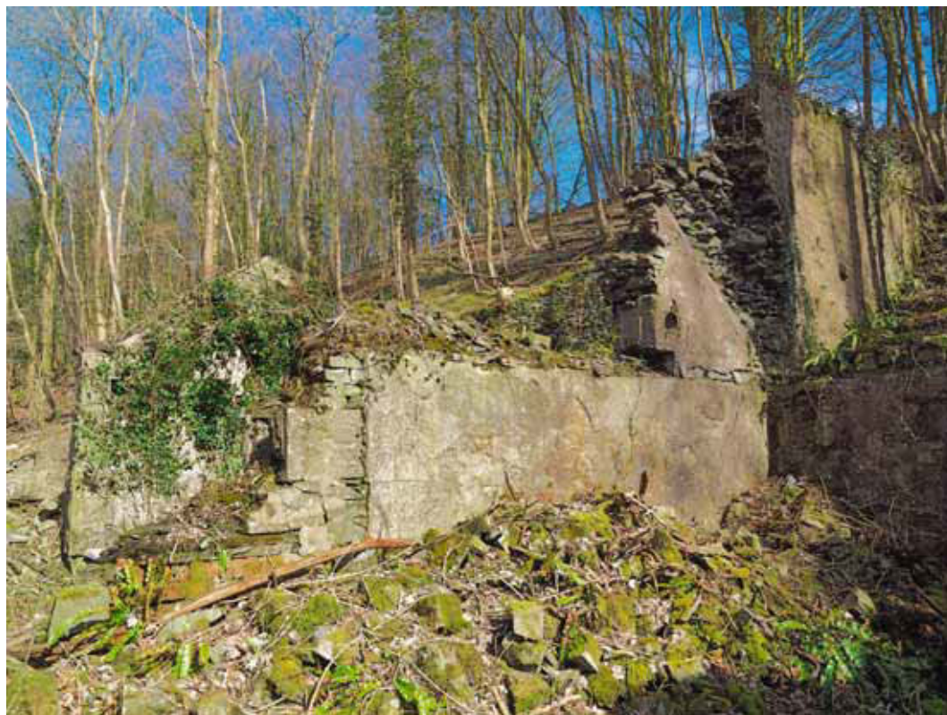
Figure 29: The drive-shaft aperture in the south chamber of incorporating mill 7 from the south (Photograph: Bob Skingle 2006, DP028078 © English Heritage.NMR)
