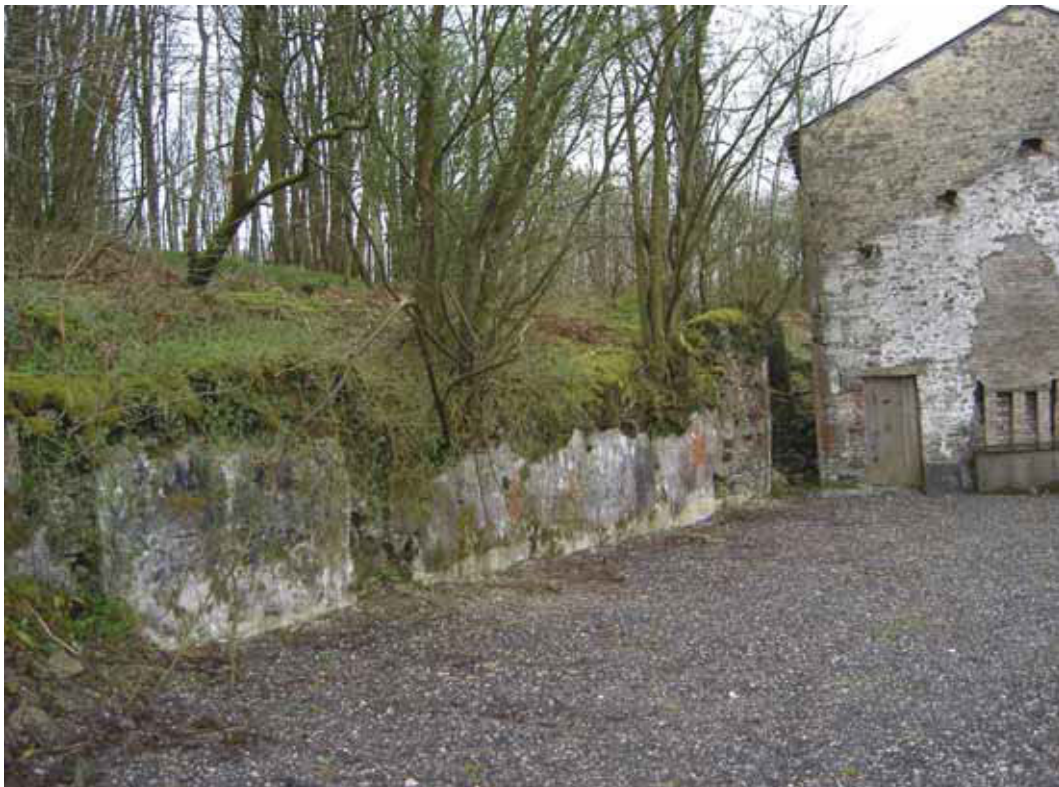
Figure 105: Rear wall of stables (building 22) and north gable of mechanics' shop showing the scar of the infill building (Photograph: Christopher Dunn 2005, © English Heritage)
