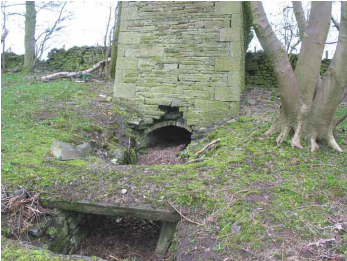
Figure 74: The flue from the glazing house and the base of chimney 9a. (Photograph: Simon Taylor 2006, © English Heritage)
