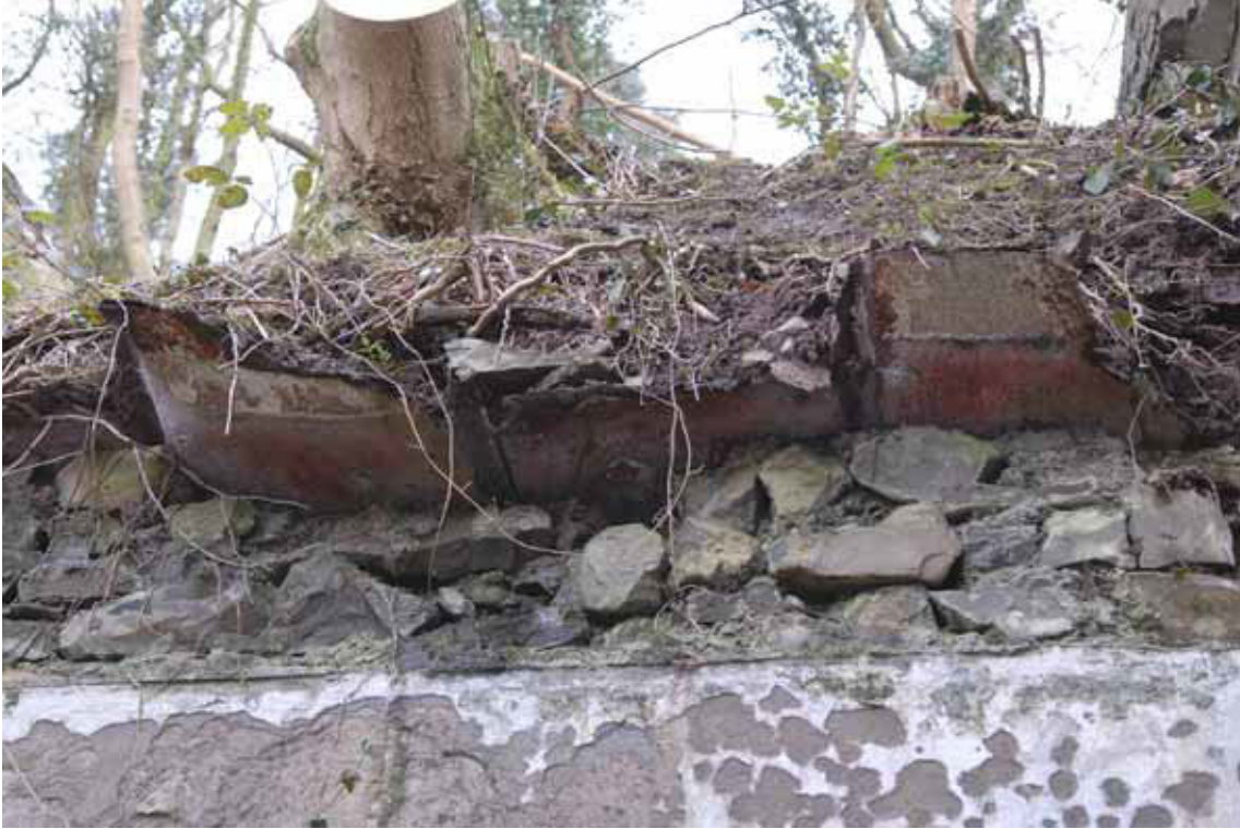
Figure 26: Detail of metal roof panels surviving in the rear wall of the south chamber of incorporating mill 3 (Photograph: Christopher Dunn 2006, © English Heritage)
