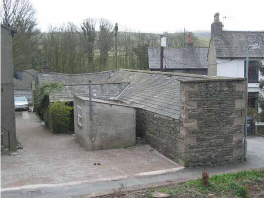
Figure 110: Rear elevations of peat houses and washhouse at Low Cottages, Endmoor (Photograph: Simon Taylor 2006, © English Heritage)
