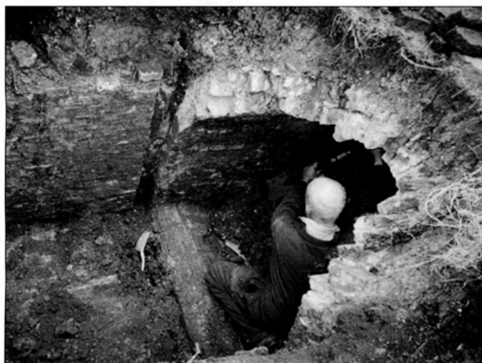
Figure 8. Culvert at The Old Plough, viewed from the west (water flow from right to left). Note the horizontal and vertical rebates in the brickwork. Gerald Rigby at work. March 2006. Photograph by Judith Chisholm.
