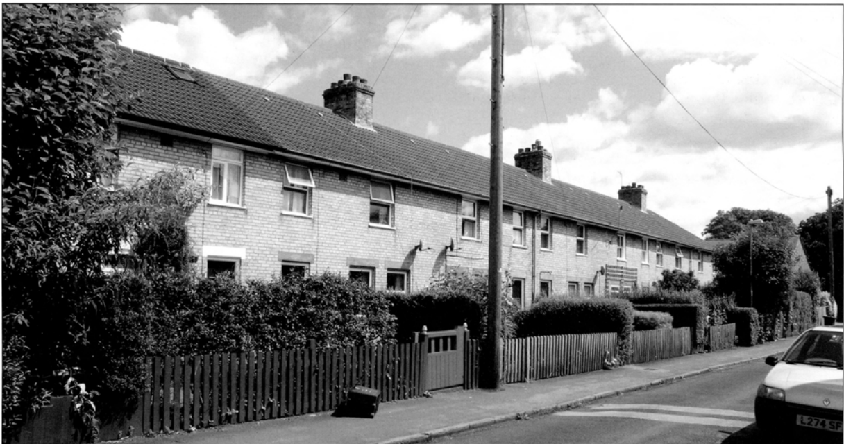
Figure 4. Council housing in Selwyn Road, erected in 1924/1925
