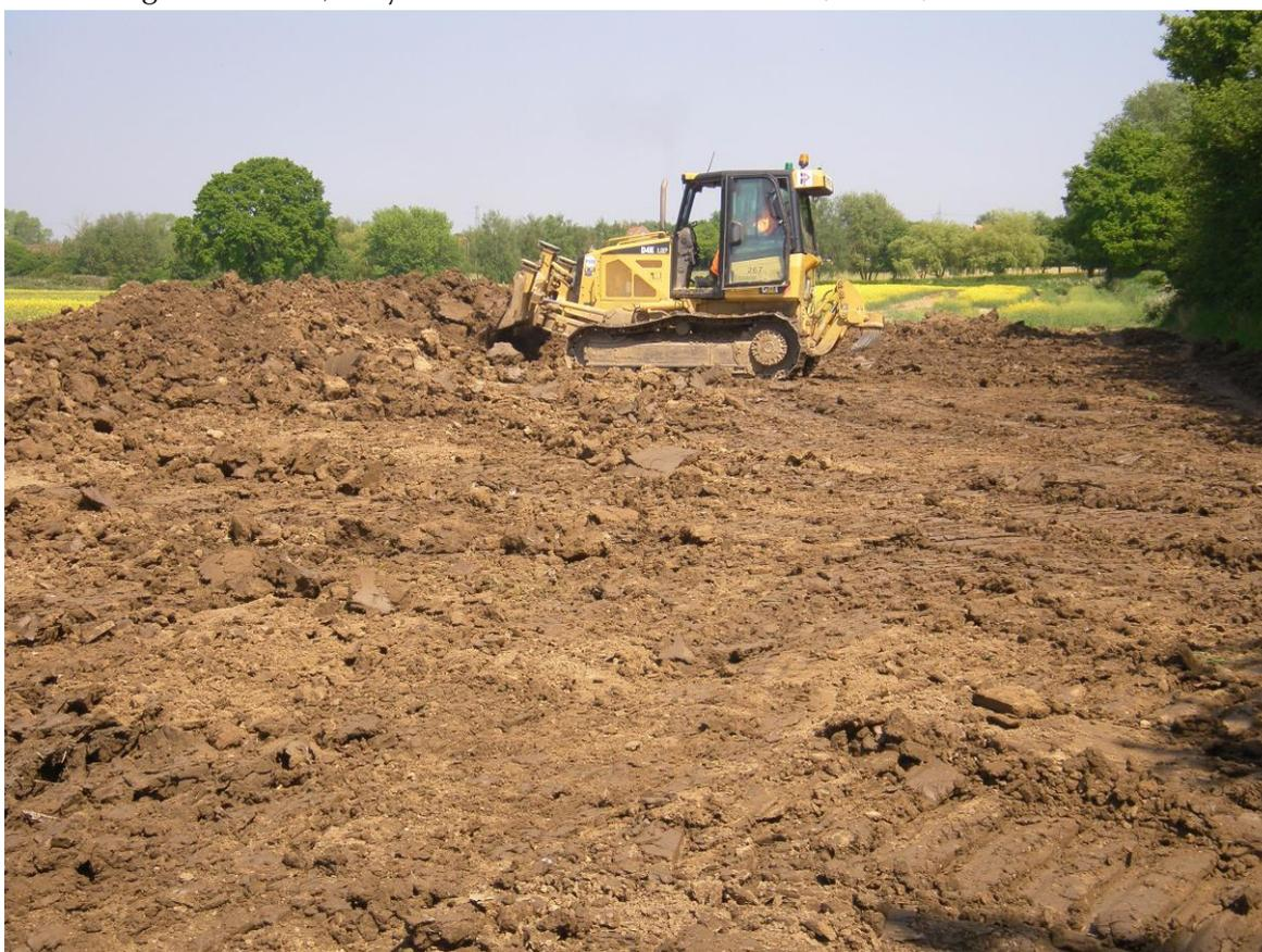
*Plate 1. Bulldozer stripping topsoil*
