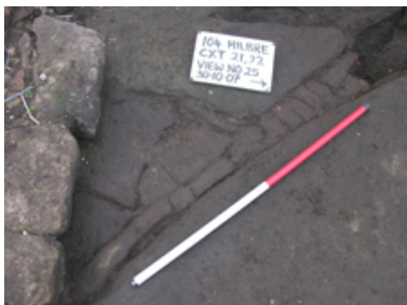
Plate 9. ?Natural fissure 22 showing brickwork repair within interior floor surface of structure. From the east.
