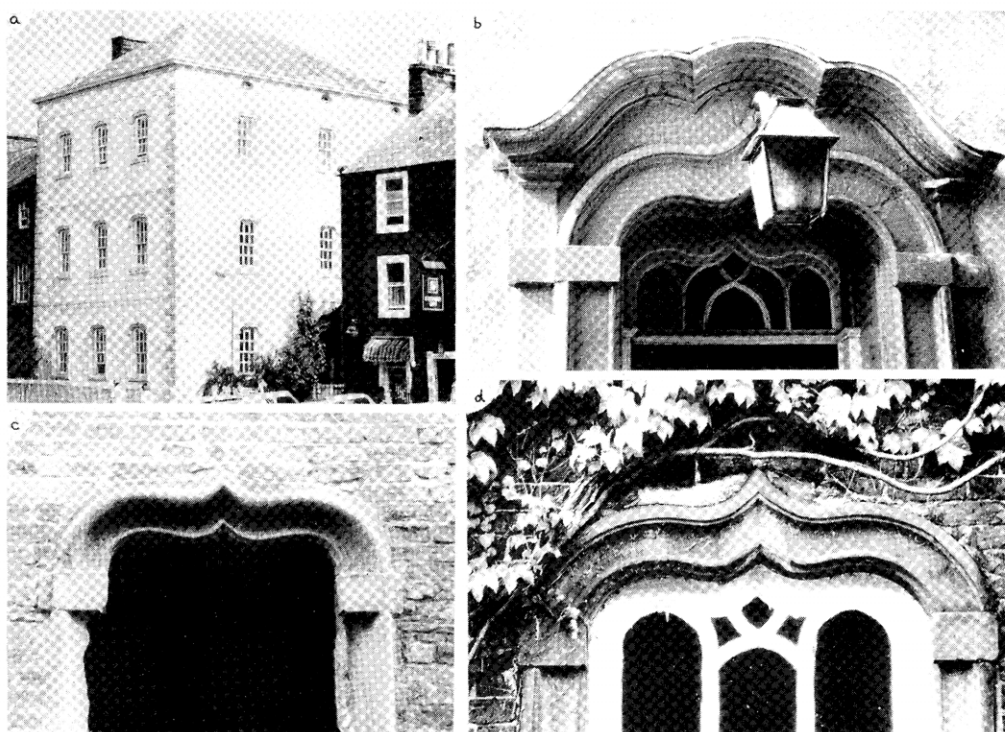
FIG. 7. – The White House, Appleby. (a) General view from the SW, showing an ogee-headed window occupying the position of the former central doorway. (b) Decorative details of the present main entrance showing the same moulding as all the windows of c.1765 (e.g. (d)). (c) Ogee-headed window in the outbuilding with a different moulding typical of a later building phase. (d) Back kitchen window with brickwork built round the obtuse angled lintel. The moulding is the same as the windows in (a).
