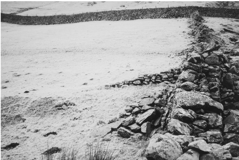
PLATE 2. The dry-stone cap superimposed on the rising terrace at the first cross-wall, looking east.
