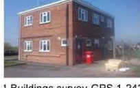
Level 1 Buildings survey-GPS 1-242
