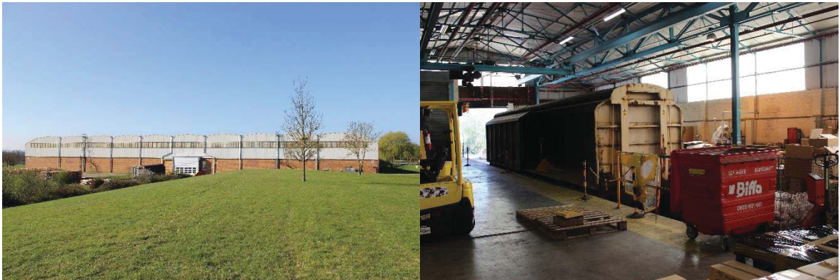
Figure 19: View of storage hangar (Building D7) Figure 20: Interior of storage hangar
