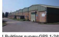
Level 1 Buildings survey-GPS 1-249
