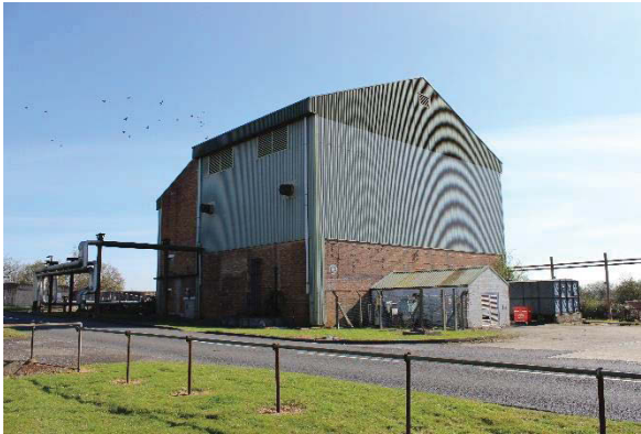
Figure 33 : View of boiler house from north
