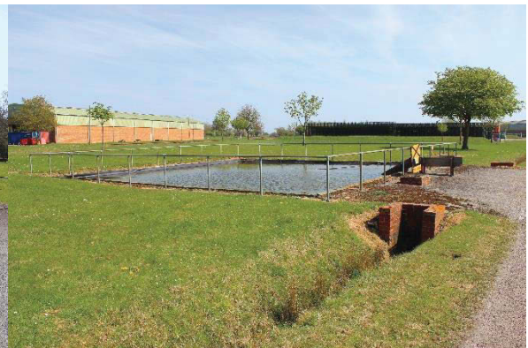
Figure 32: Pond adjacent to Building D4
