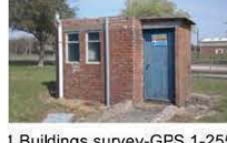
Level 1 Buildings survey-GPS 1-255
