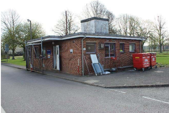
Figure 37: Guard post at E Site entrance
