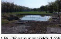
Level 1 Buildings survey-GPS 1-246
