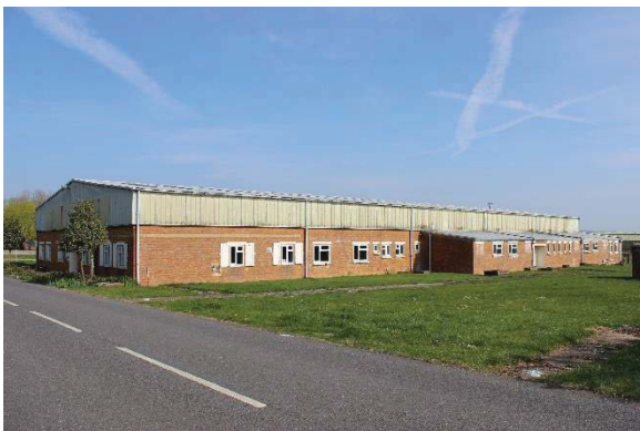
Figure 35 : View of Building D3 from north west
