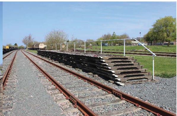
Figure 24: Platform made of sleepers (D Site)
