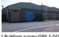
Level 1 Buildings survey-GPS 1-247
