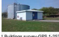
Level 1 Buildings survey-GPS 1-253
