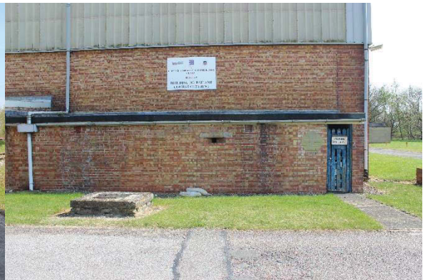
Figure 28: Air raid shelter incorporated into Building D7
