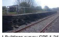
Level 1 Buildings survey-GPS 1-243
