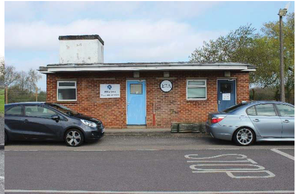
Figure 38: Guard post at E Site entrance
