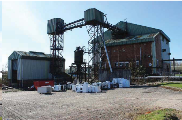
Figure 34: View of boiler house from south east
