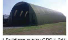
Level 1 Buildings survey-GPS 1-244
