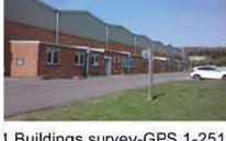
Level 1 Buildings survey-GPS 1-251
