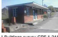
Level 1 Buildings survey-GPS 1-241
