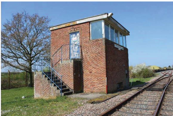
Figure 23: D Site Signal Box
