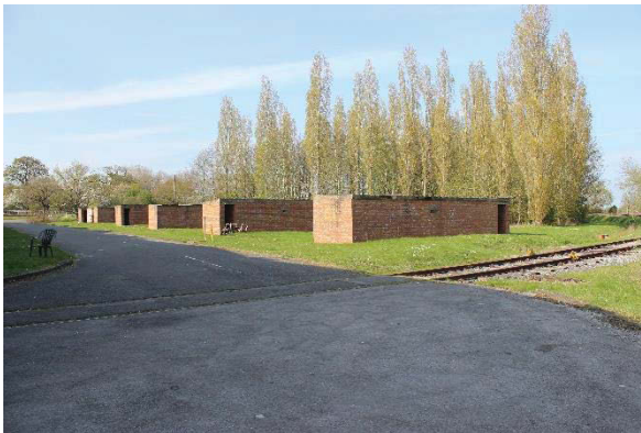
Figure 27 : Air raid shelters adjacent to Building D2
