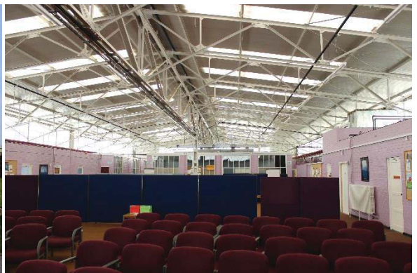
Figure 36: Interior view of Building D3
