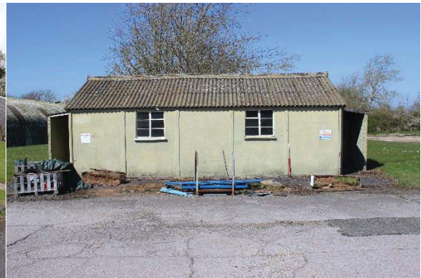
Figure 30: Hut adjacent to Building E31
