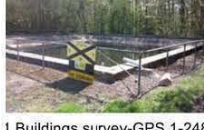
Level 1 Buildings survey-GPS 1-248
