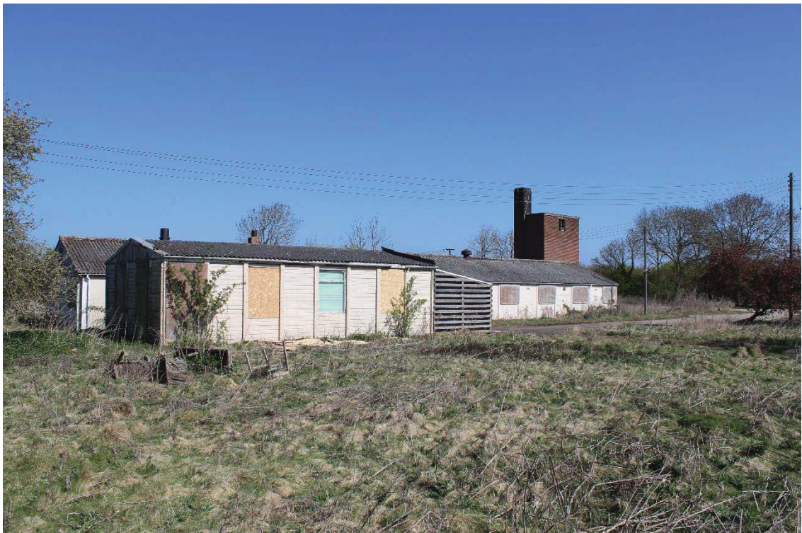
Figure 14: View of Rodney House from south-west
