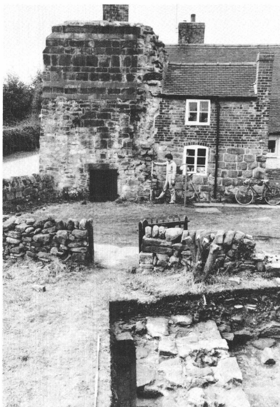
Plate 4 Dale Abbey. Areas I and V: view facing east, showing the south wall of the South Range [ABK] and, in the background, the chimney [AFA] and the east wall of Abbey/Manor House. Note core and damaged stonework at the junction with the south wall of the South Range.
