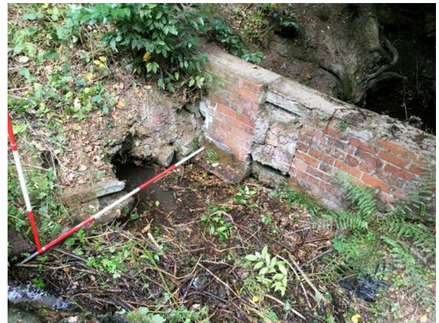
Fig. 43 IP10 Brick sluice looking north.
