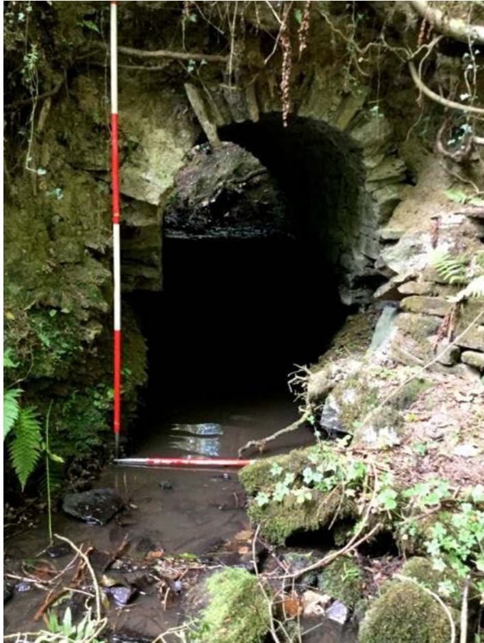
Fig. 46 IP10 Culvert looking west.
