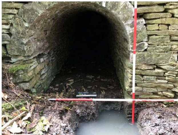
Fig. 16 IP3 view of tunnel entrance and trench looking west.
