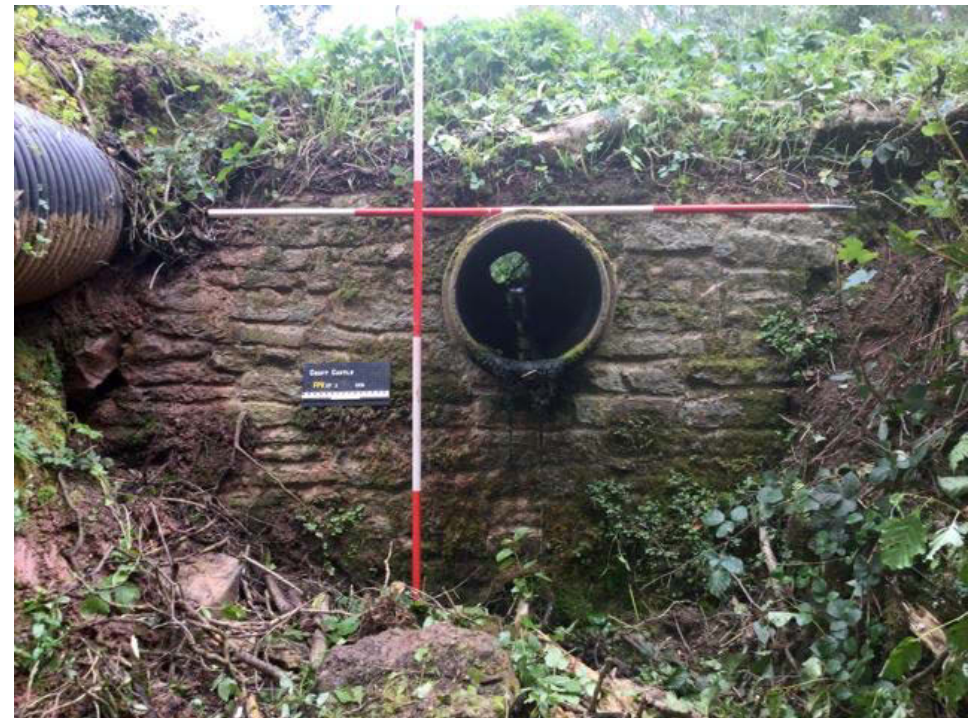
Fig. 7 IP1 Retaining wall and pipe view looking west.
