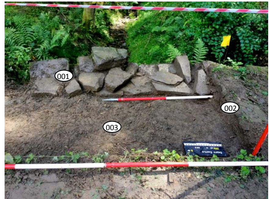
Fig. 23 IP5 Rear of retaining wall and clay make up looking east.
