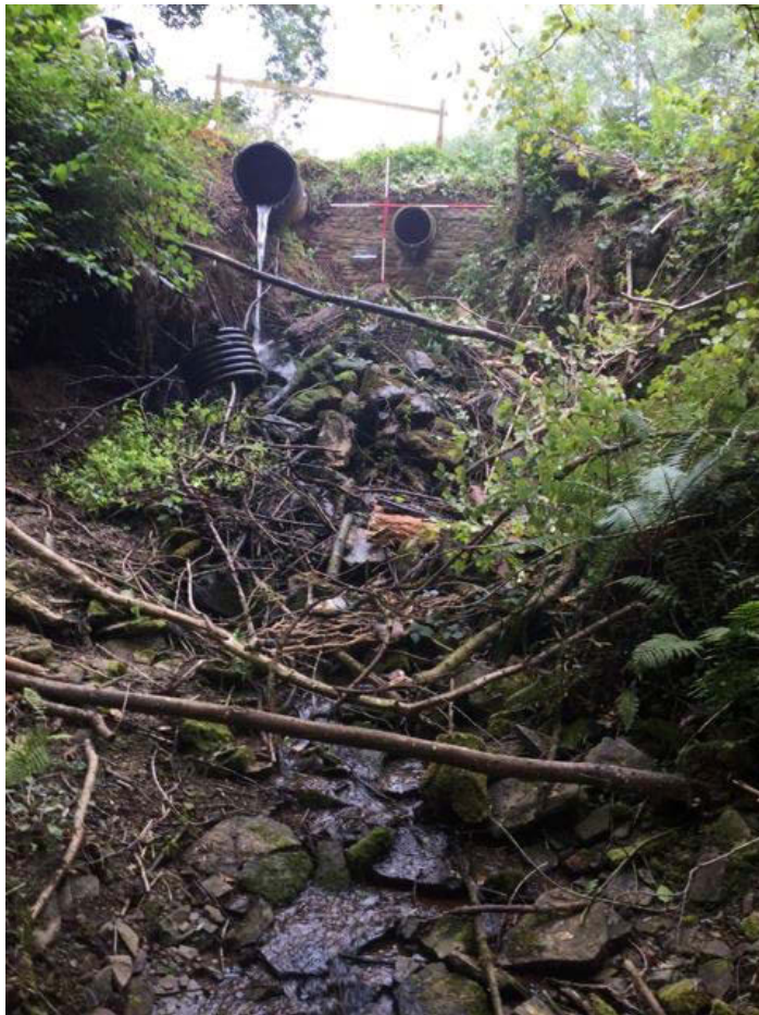
Fig. 6 Southern scour channel, looking west towards IP 1 and overflow pipes.
