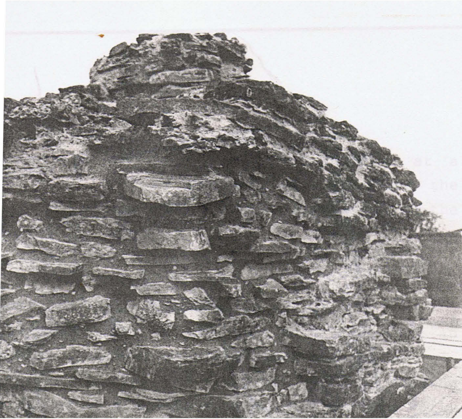
The upper part of the masonry fragment from the south-west showing the new core-work
