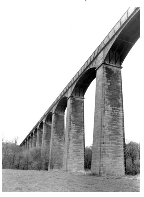
Figure 2.5 Pontcysyllte Aqueduct, completed by Telford in 1805, 1,007ft (307m) long and 127ft (38m) high, built to carry the Ellesmere Canal in an iron trough (Ken Hoverd)
