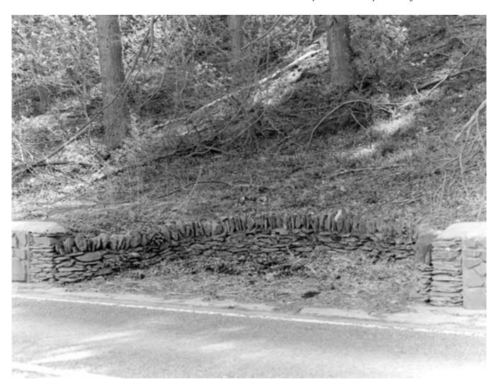
Figure 8.6 Modern revetment wall retaining an original depot (Ken Hoverd)
