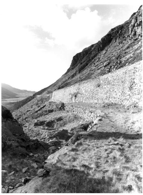
Figure 2.2 Nant Ffrancon, showing the turnpike road of 1802-08 below Telford's Holyhead Road (Ken Hoverd)
