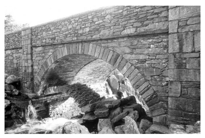
Figure 5.13 Pen-y-benglog Bridge from the north-east, showing the span from the earlier turnpike bridge, beneath the 20th-century widening of Telford's bridge (Ken Hoverd)
