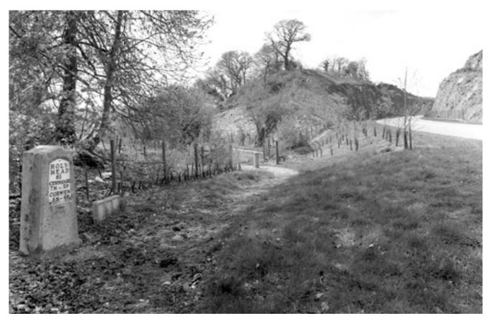
Figure 8.4 The eastern approach to the Glyn Bends cutting (Ty Nant) where it diverges from the original line, showing the relocated milestone [088] (Ken Hoverd)
