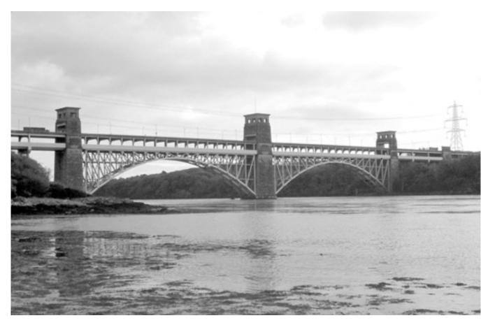
Figure 8.2 The Britannia Bridge following its conversion to road and rail carriage (Rick Turner)
