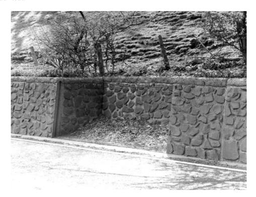
Figure 5.18 Modern pre-cast, stone-faced, concrete walling and depot towards Maerdy (Ken Hoverd)
