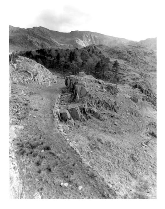
Figure 4.19 Line of the 1802–1808 turnpike through Nant Ffrancon showing the meandering course of the road through and around prominent crags (Ken Hoverd)
