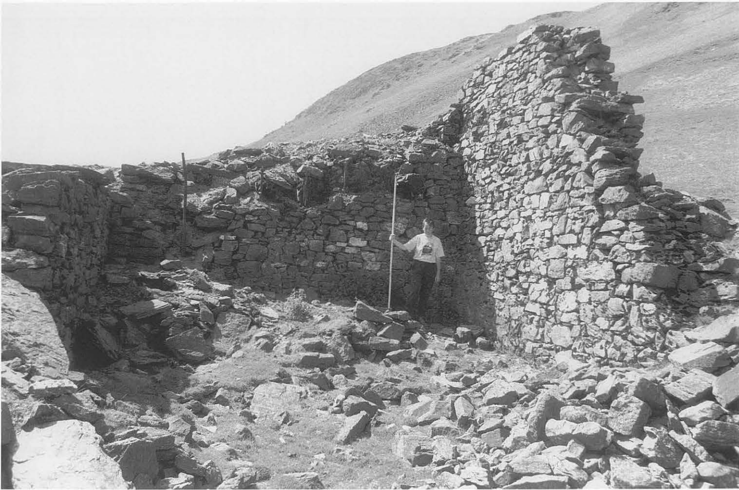
Figure 45 Nant y Car South mine: remains of the substantial crusher house (18523) viewed from the east. There are four remaining beam ends in situ in the far wall, indicating that two sets of crusher rolls were in operation. The crusher was powered by a water-wheel which was also pumping and winding the engine shaft, the wheelpit of which (18522) adjoins the south wall of the crusher. (CPAT 330-04)
