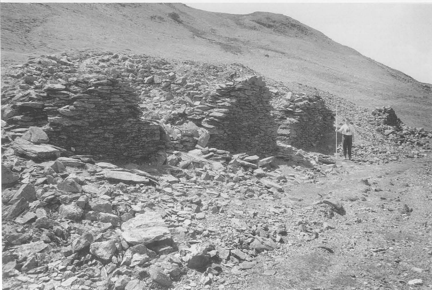
Figure 40 Dalrhiw mine: bank of three ore-bins (18490) built into the tip of development rock north of the engine shaft, viewed from the north-east. (CPAT 285-16)
