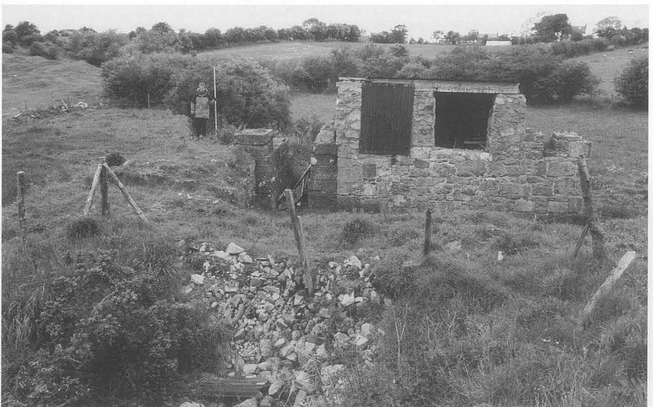
Figure 109 Remains of the later 19th-century engine house at Central Minera (18735, see Fig 107), viewed from the south-east. The figure is standing on the engine bed for the original horizontal engine, to the left of the wheelpit. The original boiler house would have lain to the left, with a chimney beyond. The building to the right of the wheelpit has been adapted as an animal shelter. The engine would have raised and lowered cages carrying ore from the shaft (18736) in the foreground. (CPAT 349-02)
