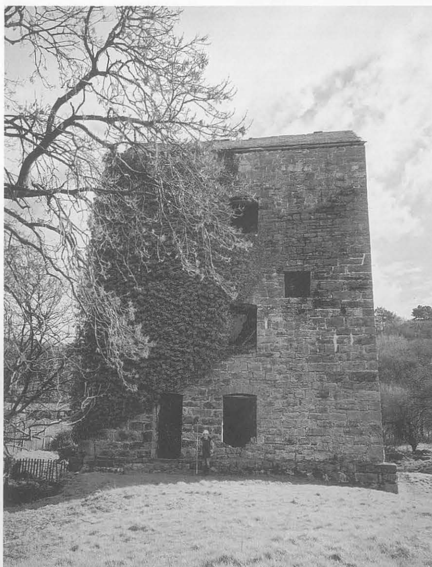
Figure 133 Talargoch, Clive Shaft: the engine house (23382) from the west with the Clive Shaft and drainage culvert to the left. (CPAT 1161-07)
