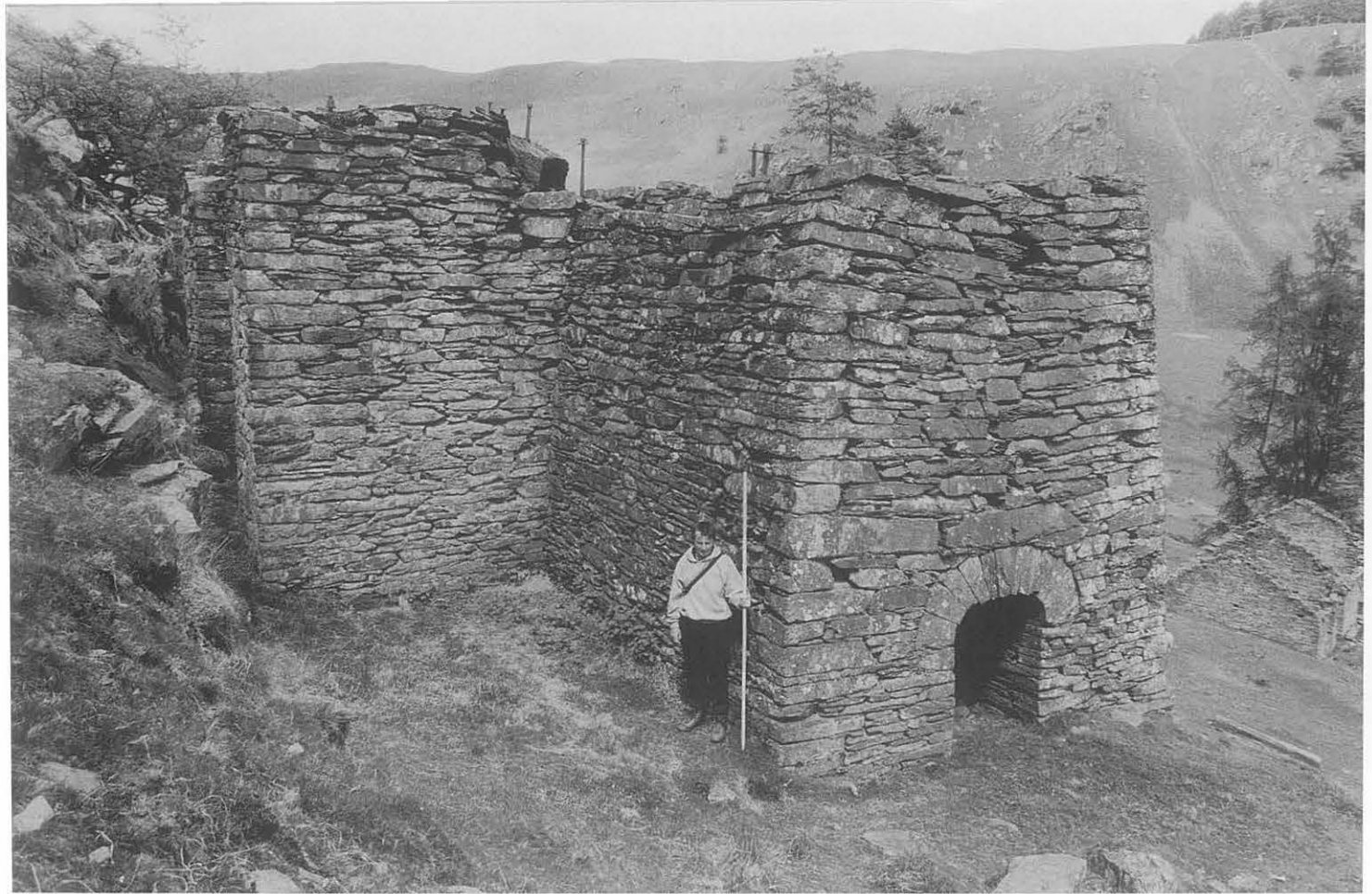
Figure 22 Cwm Elan mine: wheelpit (18469) for pumping and winding the engine shaft. It once held a waterwheel 36 feet in diameter and 4 feet wide (Hall 1993, 80–1). Supporting walls for the winding drum adjoin the west (left) side of the wheelpit. Iron pumping rods and supports lie scattered around the immediate area. (CPAT 283–35)
