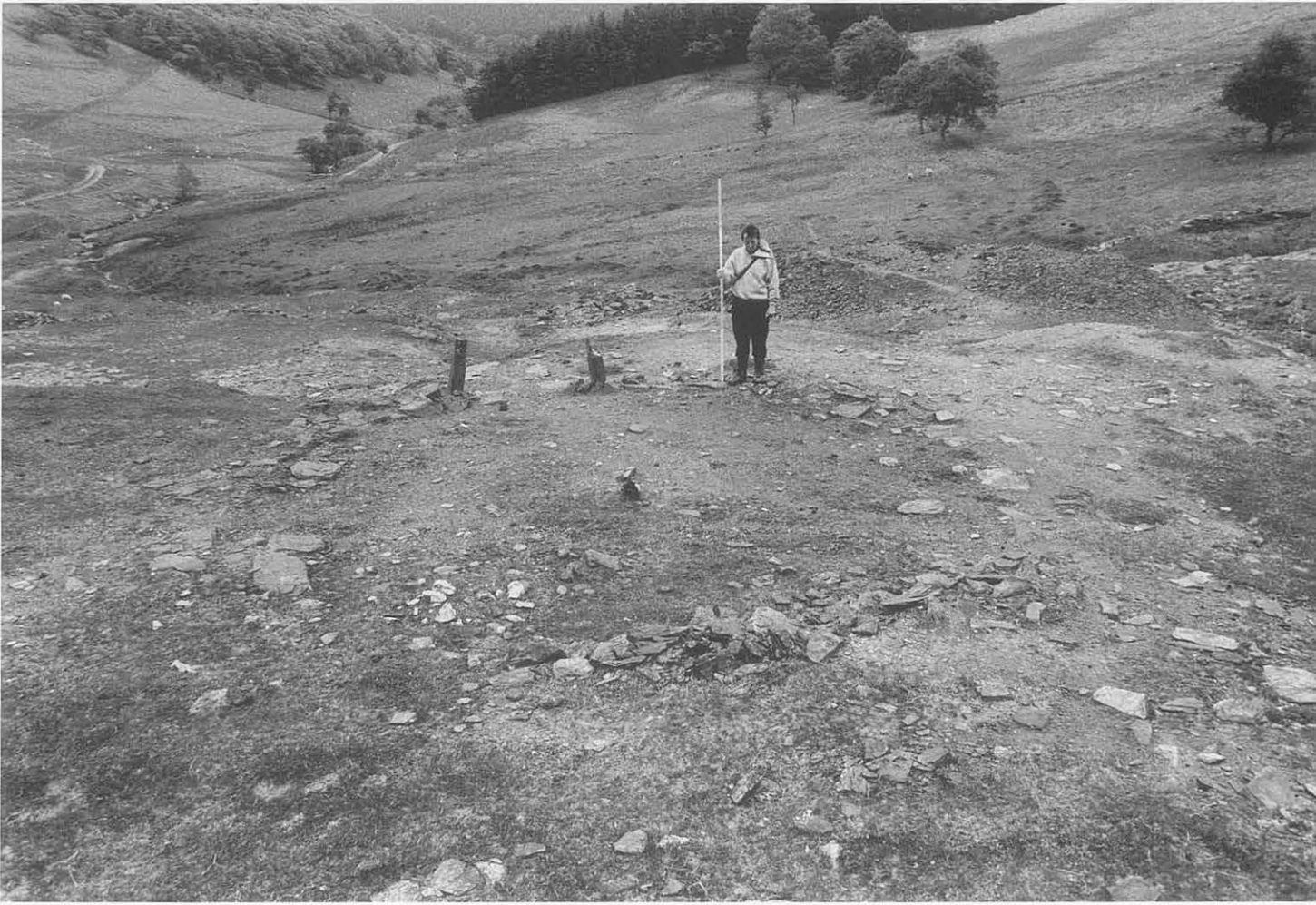
Figure 24 Cwm Elan mine: remains of circular buddle (18480) showing traces of the timber centre post and two supports for a launder. The buddle was powered by a small wheelpit to the west (18479), measuring 6 metres by 1 metre, driven by water emitting from the crusher wheelpit. A slight channel to the south of the wheelpit suggests that when the buddle was not in operation the water would have been diverted directly into the stream. (CPAT 283-04)
