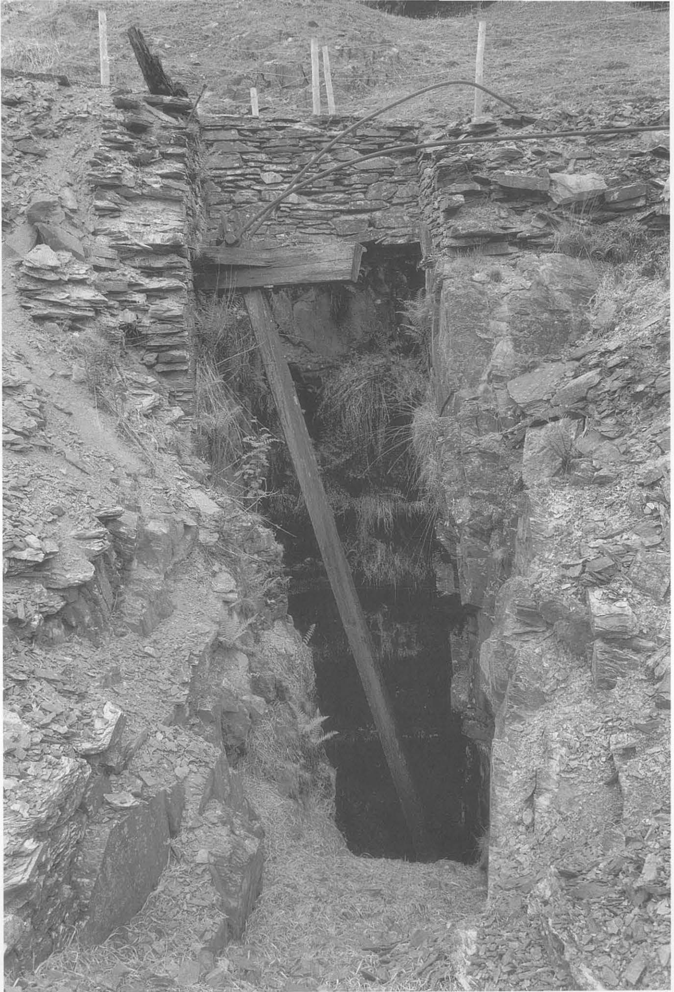
Figure 21 Cwm Elan mine: engine shaft (18467) viewed from the east, showing timber pumping rod surviving in situ . (CPAT 283-23)
