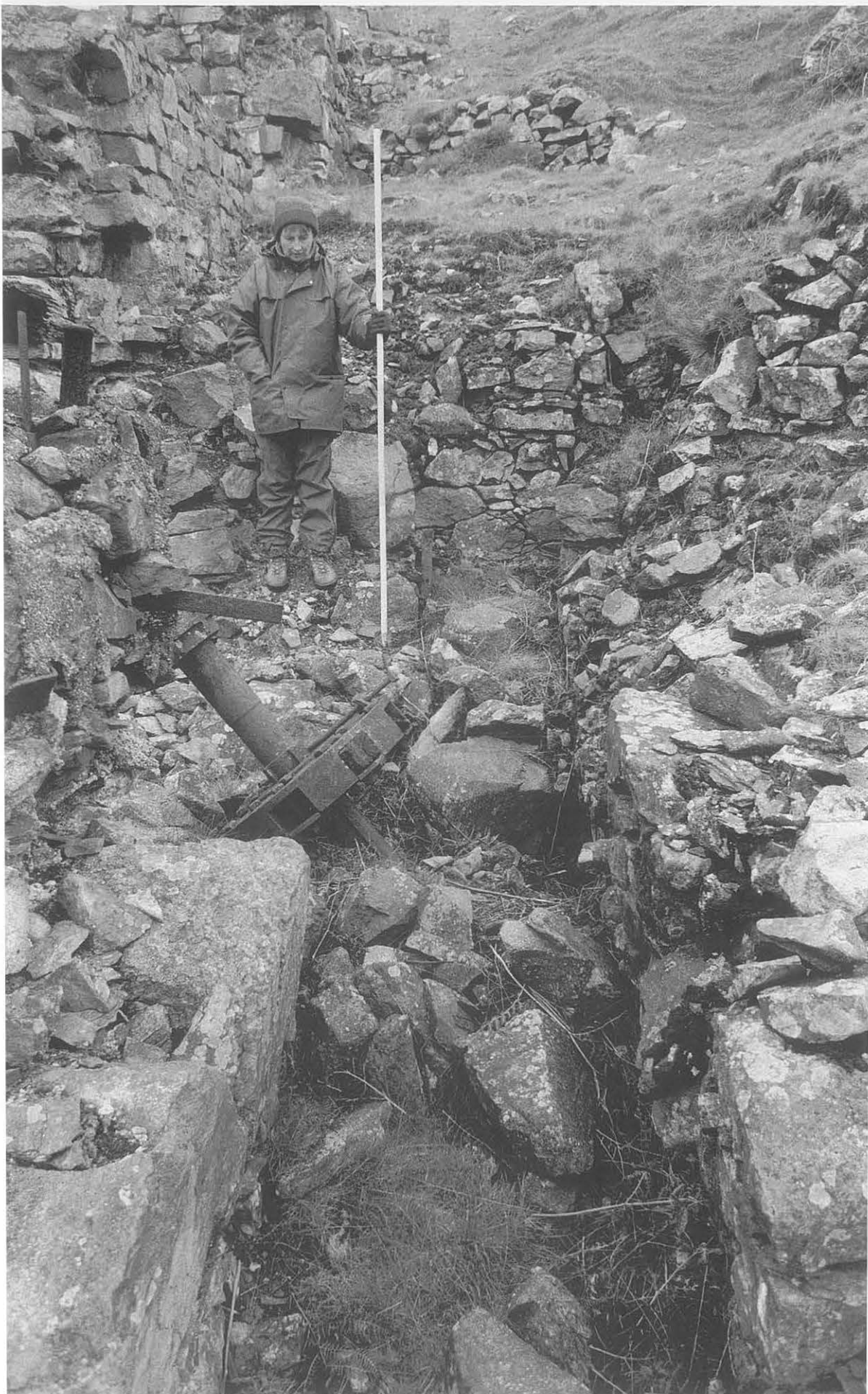
Figure 33 Cwm Orog mine: crusher house wheelpit (18442) with remains of cast- iron waterwheel lying amongst the collapsed masonry. (CPAT 275-03A)
