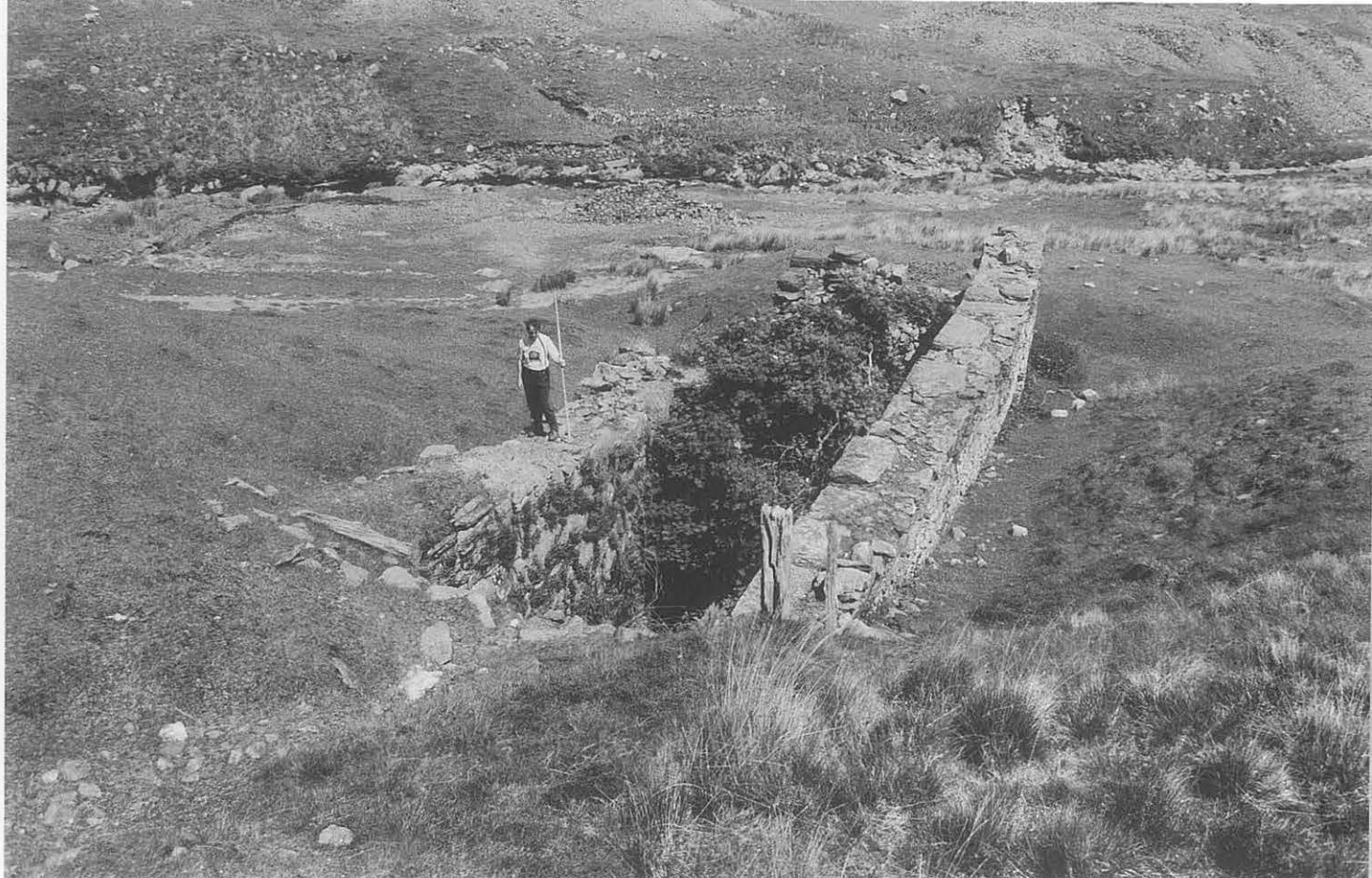
Figure 39 Dalrhiw mine: pumping wheelpit (18502) from the south, looking towards the Rhiwnant stream. The waterwheel drove pumping rods via a system of flat-rods, for which part of the track-bed (18506) is visible in the foreground. (CPAT 285–10).
