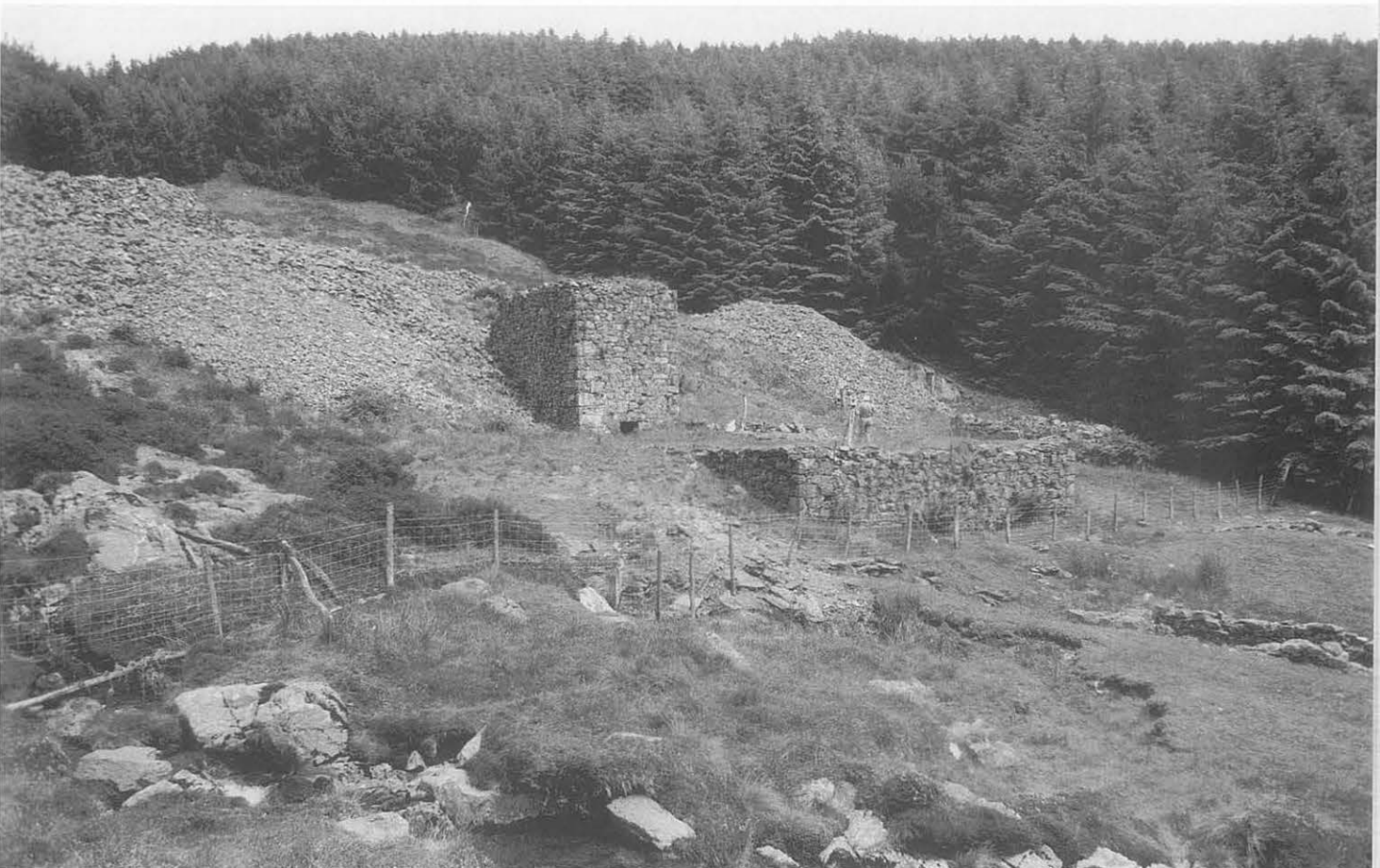
Figure 52 Nant yr Eira mine: crusher wheelpit (18536) and stone-revetted platform (18538) viewed from the south-west. Part of a second wheelpit (18540) visible to the right probably powered jiggers on the jig platform (18542) to the east. (CPAT 330-23)
