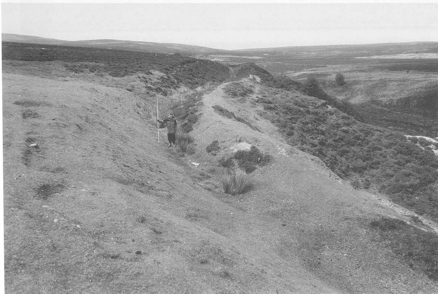
Figure 125 Pool Park mine: substantial leat (18181, Fig 122) running along the edge of the Aber Sychnant Valley, looking towards Llandegla moor and Eglwyseg. The leat by-passed the west side of Pool Park, and supplied water to the large mines at Minera. (CPAT 351–16)
