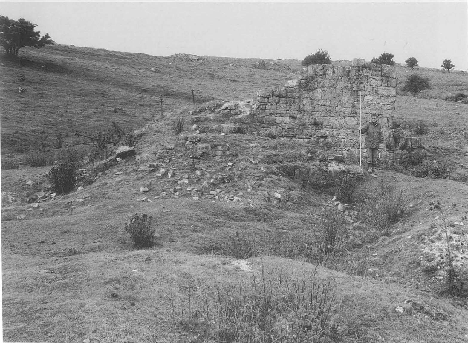
Figure 93 Belgrave mine: remains of the wall of the pumping engine house (12060) towards the south-east side of the mine. A steam engine once housed in the building drove a beam-pumping engine at the main shaft via a system of flat-rods, pumping water from underground to fill reservoirs for feeding the boiler of a winding engine house and possibly for water-power for driving machinery on the dressing floor. The underground workings appear to have been drained by gravity-fed adits which ran into River Alun towards the west. (CPAT 381–22)
