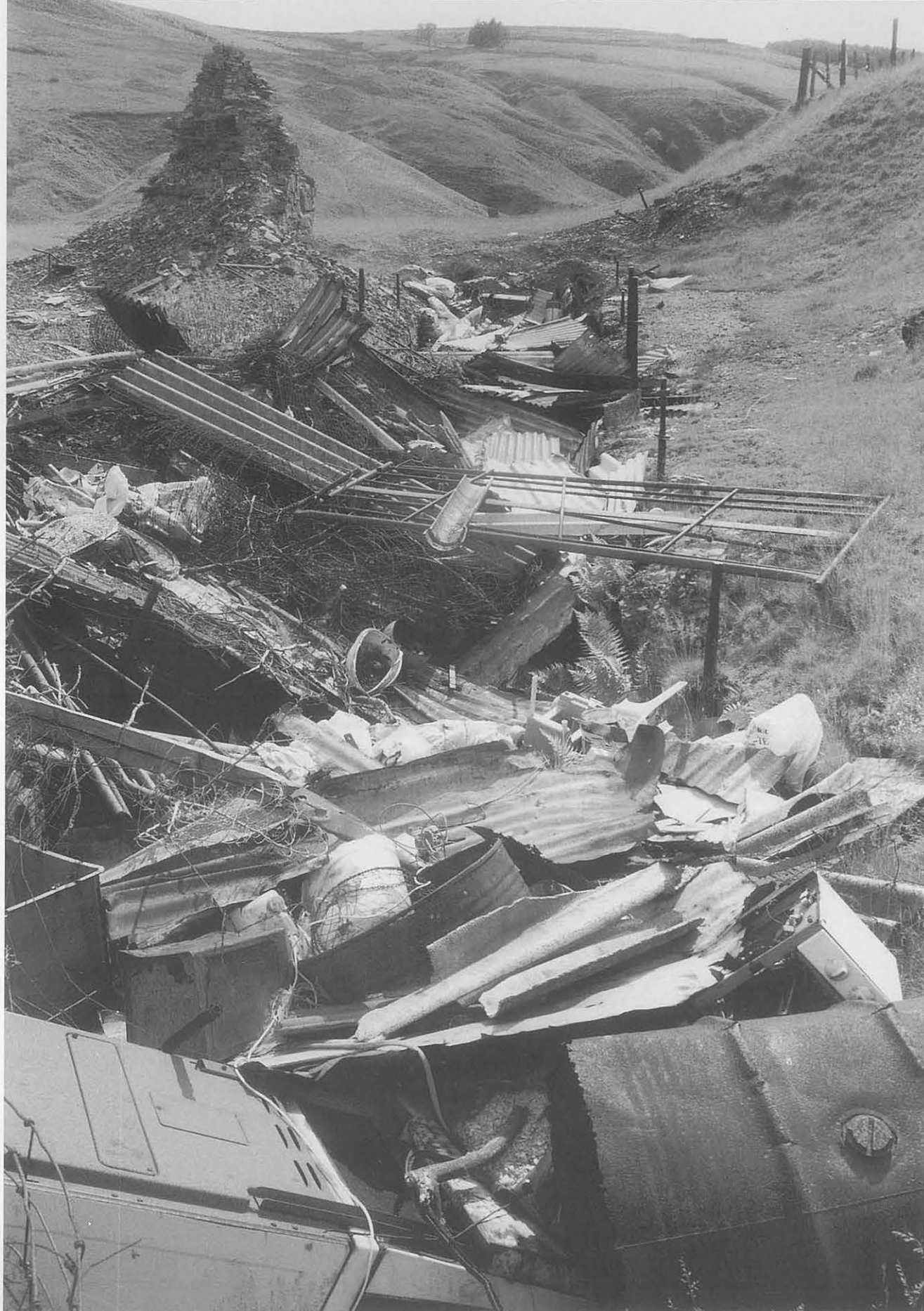
Figure 134 Pen Dylife mine, Llanbrynmair, Powys: the foundations of the wheelpit for the 63-foot diameter Red or Martha Wheel constructed in the 1850s which used to pump and draw from the Llechwedd Ddu shaft. The wheelpit once held the largest diameter waterwheel employed on a metal mining site in Wales, but is almost unrecognizable beneath heaps of discarded rubbish. Regrettably, many mining sites in upland Wales are seen as a convenient dumping ground for old machinery and often attract fly-tipping. (CPAT 153-26)
