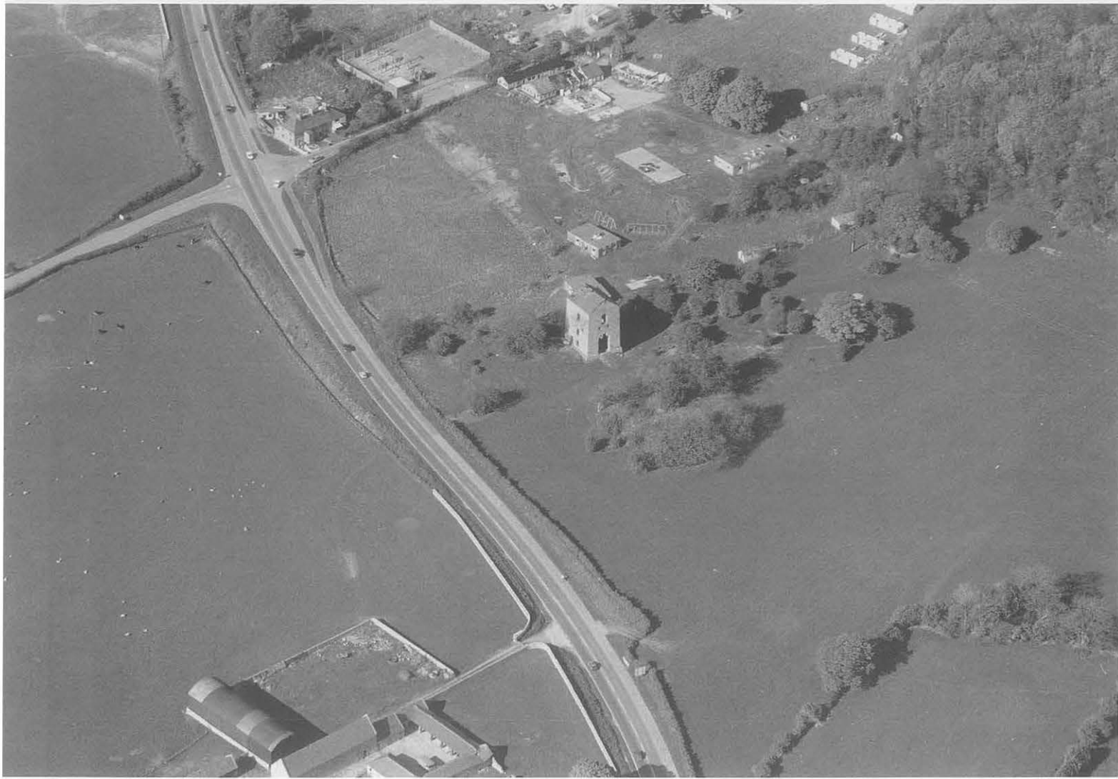
Figure 129 Aerial view of Talargoch, Clive Shaft, seen from the south-west showing the substantial stone-built engine house with the Drawing Shaft in front. The curving course of an early leat can be traced to the west of the road. (CPAT 88-9-16)
