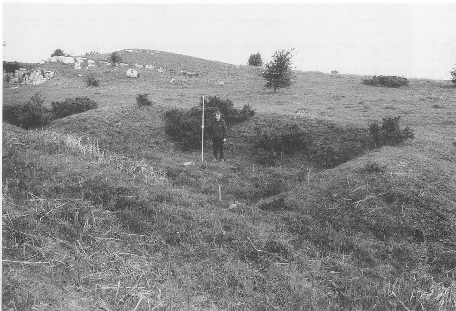
Figure 103 Eisteddfod mines: reservoir (18817, shown on plan in Fig 105) on the northern edge of the Hush, towards its western end. It was probably used to store water for the boilers on the engine house (18811) about 20 metres to the west. It was fed by a leat (running diagonally across the foreground) dug along the north side of the Hush to draw water from the Aber Sychnant stream. (CPAT 348-13)
