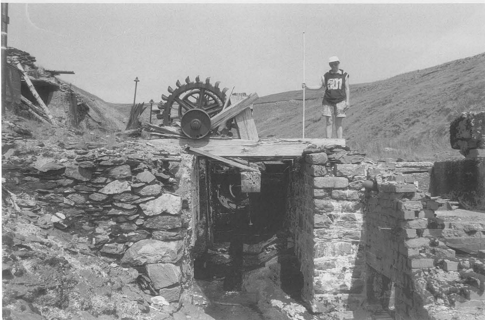
Figure 66 Nantiago mine: the surviving Pelton-wheel. (18635) (CPAT 329-03)
