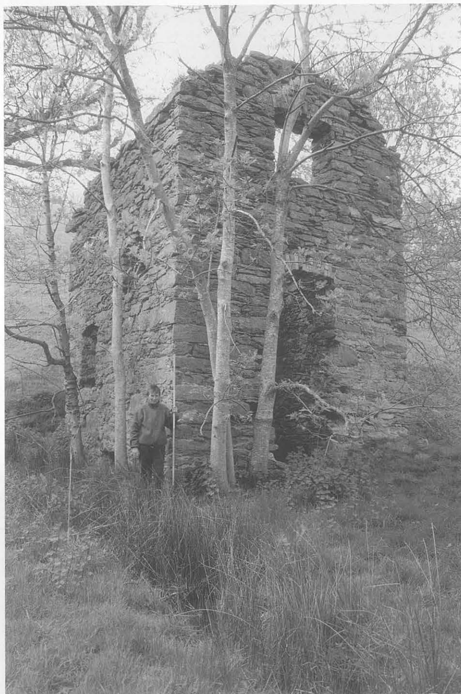
Figure 79 Penyclun mine: engine house (18338) viewed from the south- east. This small Cornish rotative engine house measures only 5.5 by 4 metres across, still stands to its full height of about 8 metres. The roof has long since fallen in and the structure is now unfortunately in a relatively poor state. (CPAT 276-27)
