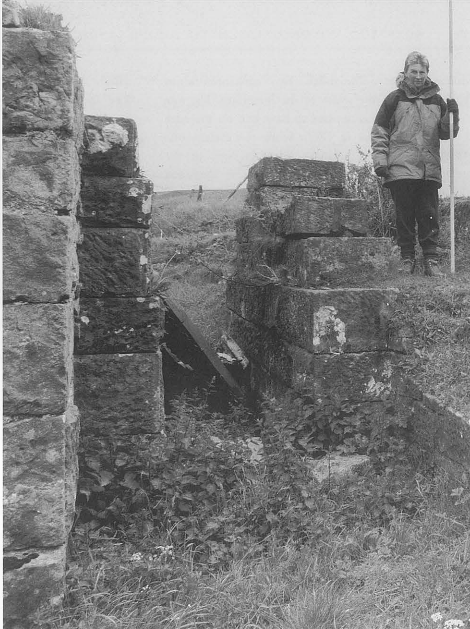
Figure 110 Wheelpit of of the later 19th-century engine house at Central Minera (18735, see Fig 107), viewed from the north-west. The stonework once supported the wheel which drove the winding-drum, raising and lowering cables in the shaft beyond. (CPAT 349-05)
