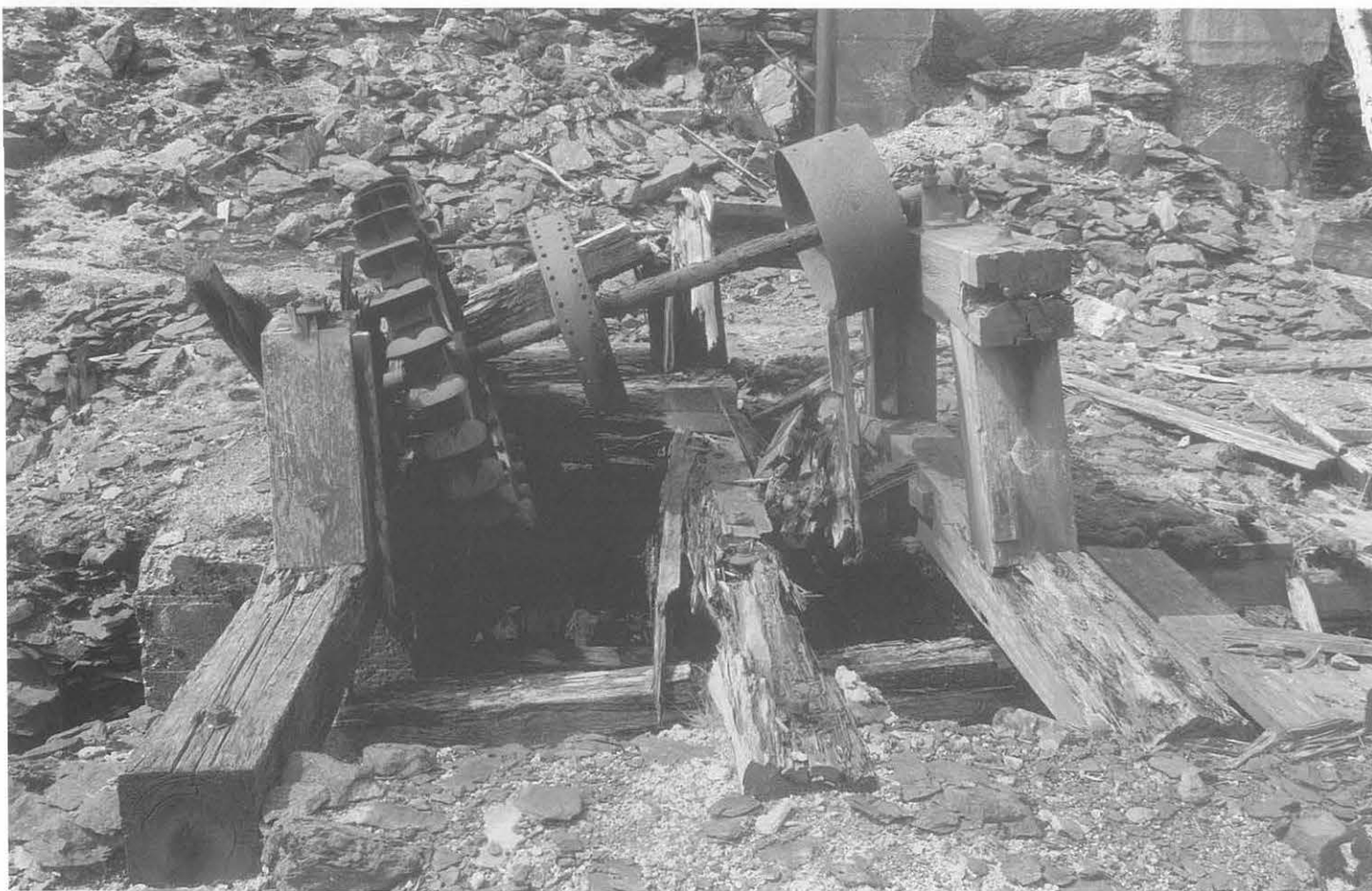
Figure 10 Iron Pelton-wheel and its timber supporting frame within the late dressing mill of about 1900 at Nantiago mine, Llangurig, Powys. Nantiago characterises the mining sites of the Industrial era in mid Wales, where large-scale processing mills were installed.
