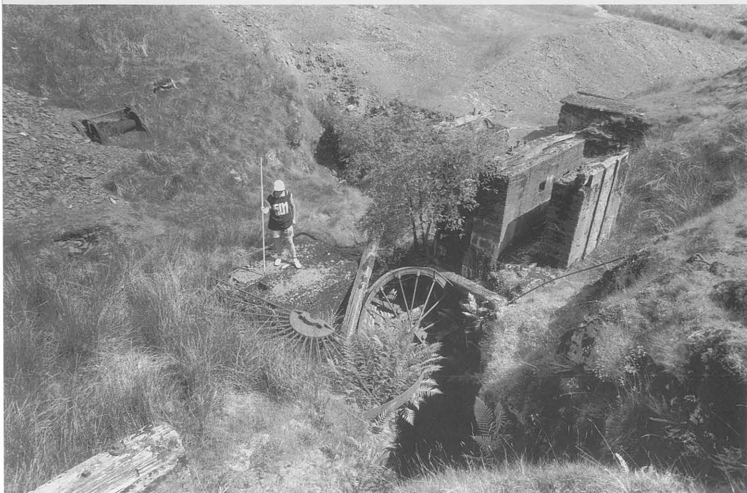
Figure 62 Nantiago mine: engine shaft (18578) from the north-west, with the remains of the iron winding wheel and wooden pumping rod at the top of the open shaft. The concrete structure visible to the right is the base for the pumping mechanism. (CPAT 329-29)
