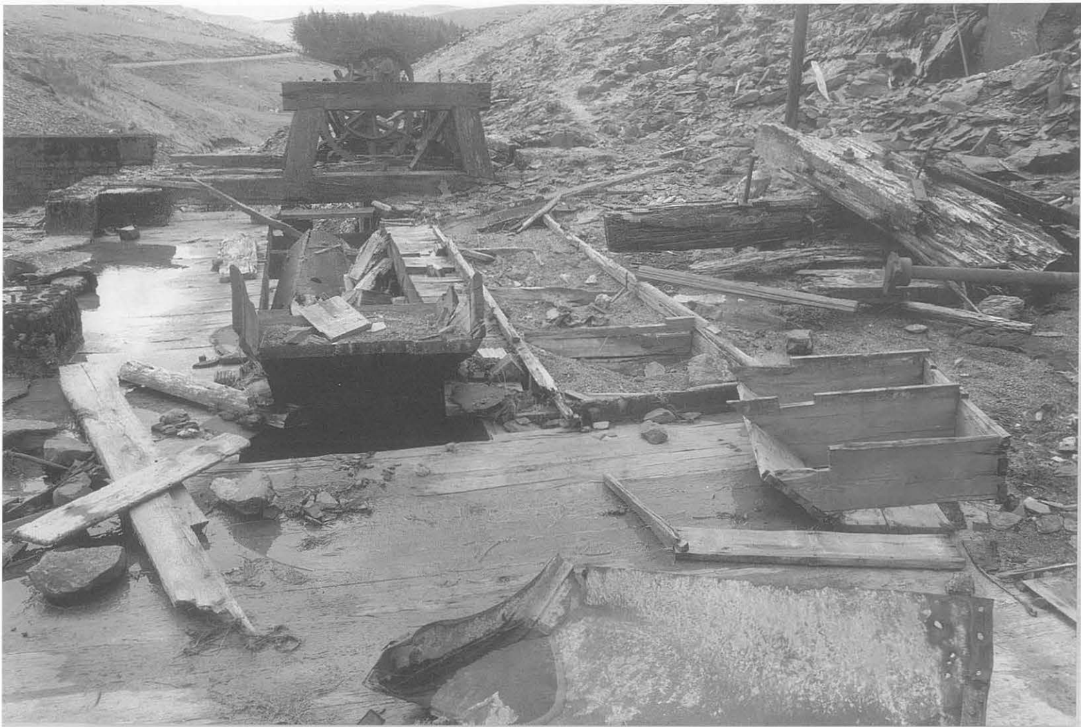
Figure 65 Nantiago mine: the later dressing floor, supported on timber planking above the Nant lago stream. (CPAT 144-35)
