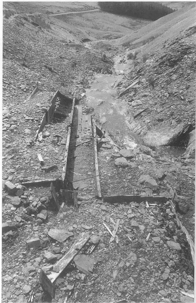
Figure 11 Remains of timber launders at Nantiago mine, Llangurig, Powys. The launders were used to carry slimes from the dressing floors to the settling pits (CPAT 144–31)
