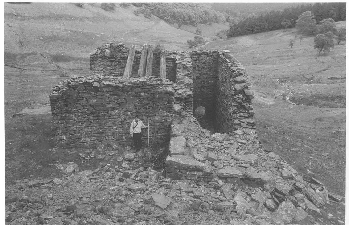
Figure 23 Cwm Elan mine: crusher house (18478), viewed from west. The walls survive to more or less their full height. Inside the building the large support beams which would have held two sets of crushing rolls are now partly collapsed, along with the axle for the waterwheel. The wheelpit (18477), 14 metres long and 4 metres deep on the south (right) side of the crusher, survives to its full height. The waterwheel appears to have been driven by water reused from the pumping wheelpit (18469) via a system of launders, possibly supplemented by additional water drawn from the stream to the south where two leats can be traced. (CPAT 283–14)
