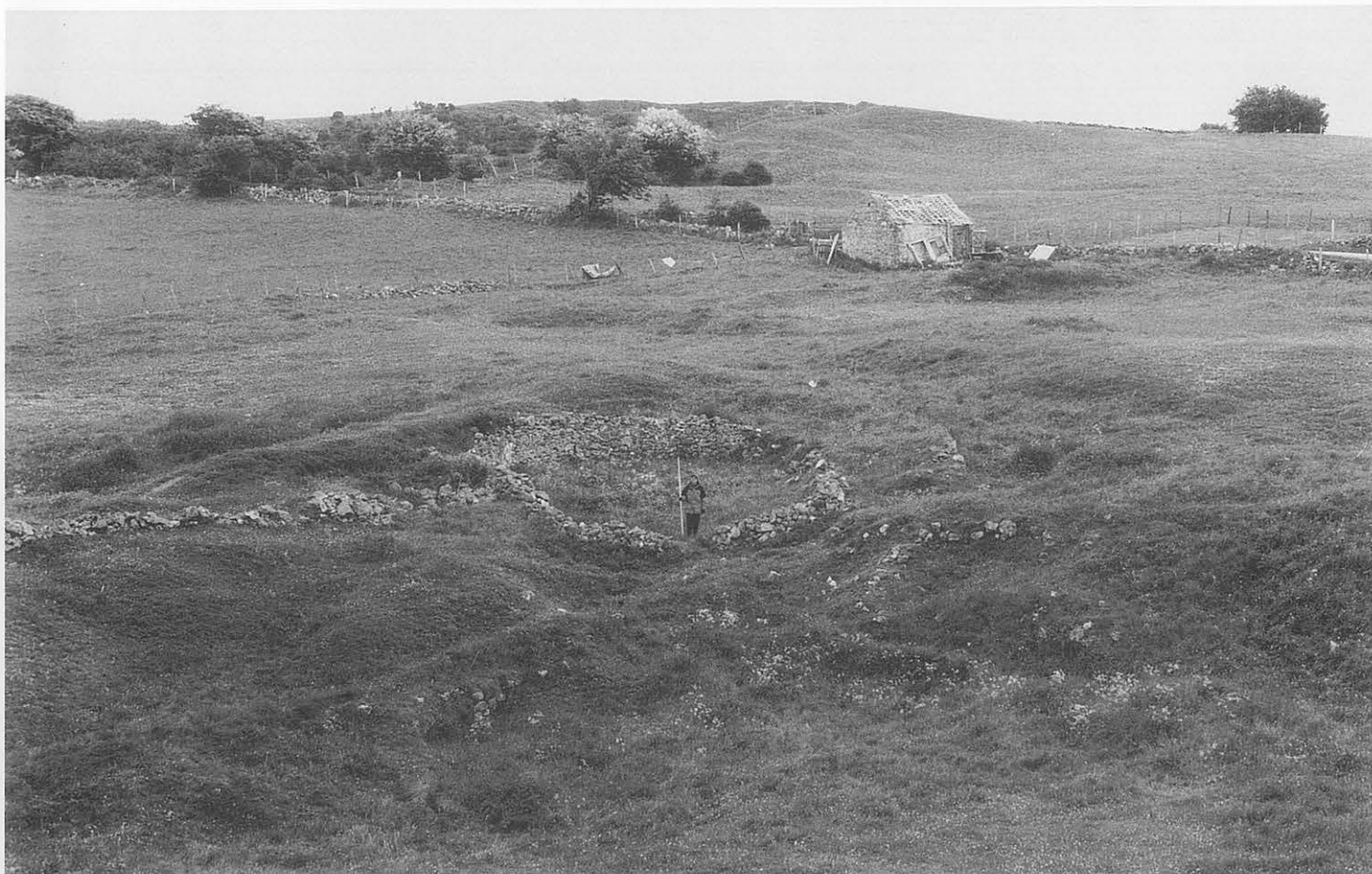
Figure 111 Stone-walled shaft enclosure (18737, see Fig 107) viewed from the west. The enclosure once surrounded one of the main shafts, now filled in, indicated by the surrounding heaps of development waste. The remains of an ore-bin and the main ore dressing floor lie in the foreground. (CPAT 348-25)
