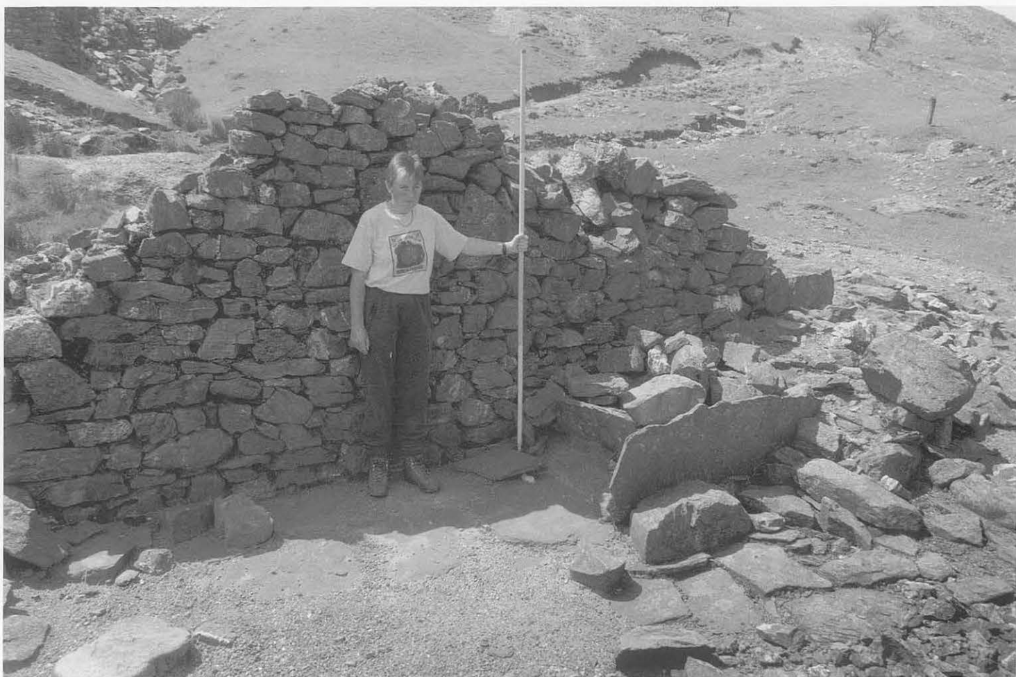
Figure 41 Dalrhiw mine: north side of the small wheelpit (18504) which probably to have powered jiggers on the platform just to the north. Against the east wall of the wheelpit are the remains of a trough built of stone slabs which probably acted as a settling tank. (CPAT 285-06)
