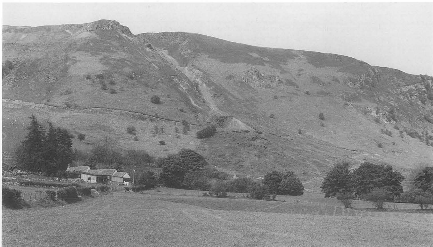
Figure 8 Hushing channel at Craig-y-Mwyn mine, Llanrhaeadr-ym-Mochnant, Powys. Hushing was used as a means of prospecting and extraction. Water collected in reservoirs and was released to remove overburden, exposing the ore-bearing rocks. This view from the valley bottom shows the broad fan of material washed out from the hushing channel on the hillside above. (CPAT 279-16A)
