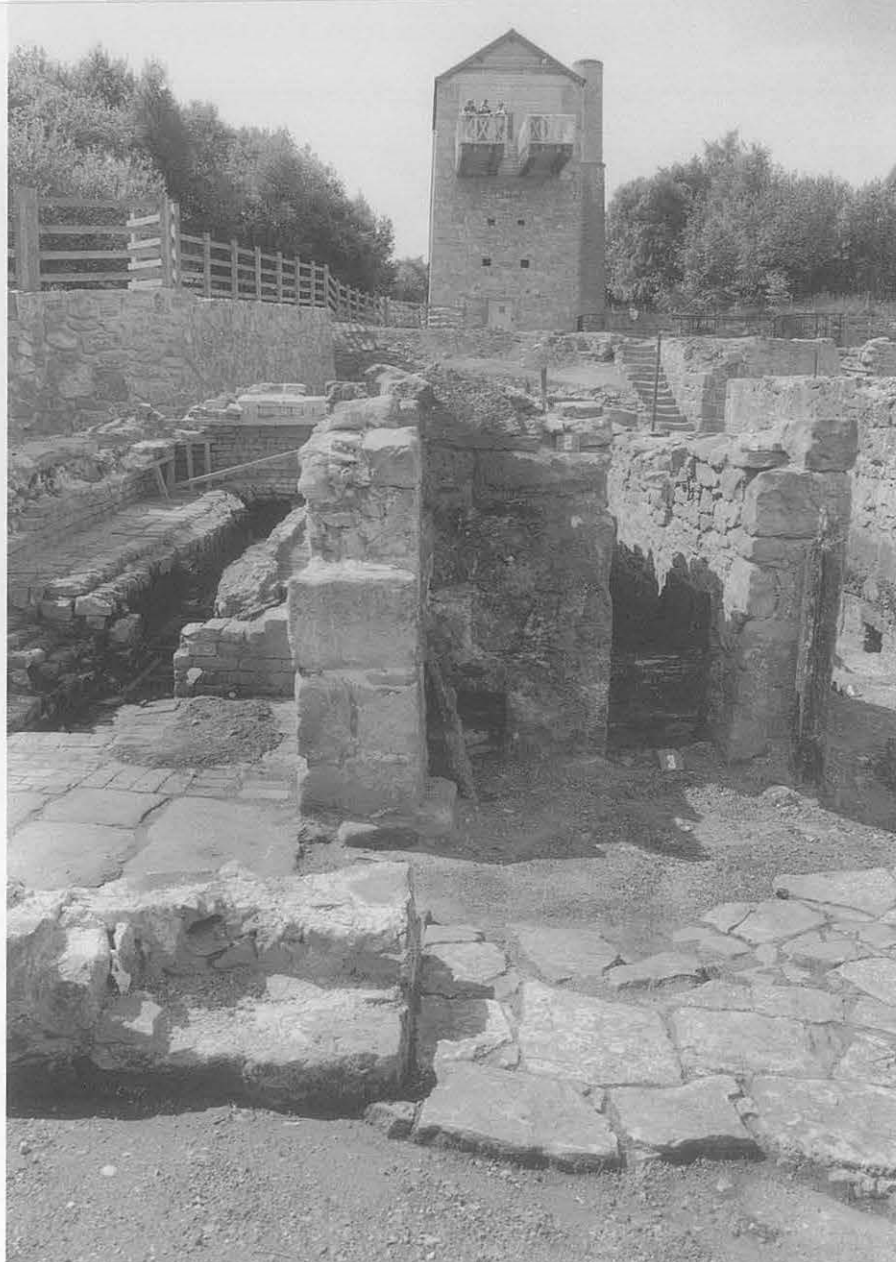
Figure 138 Minera Lead Mine Museum, Wrexham: the restored Meadow Shaft engine house dating to about 1857 with the base for a small winding and crushing engine in the foreground. (CPAT 241-4A)
