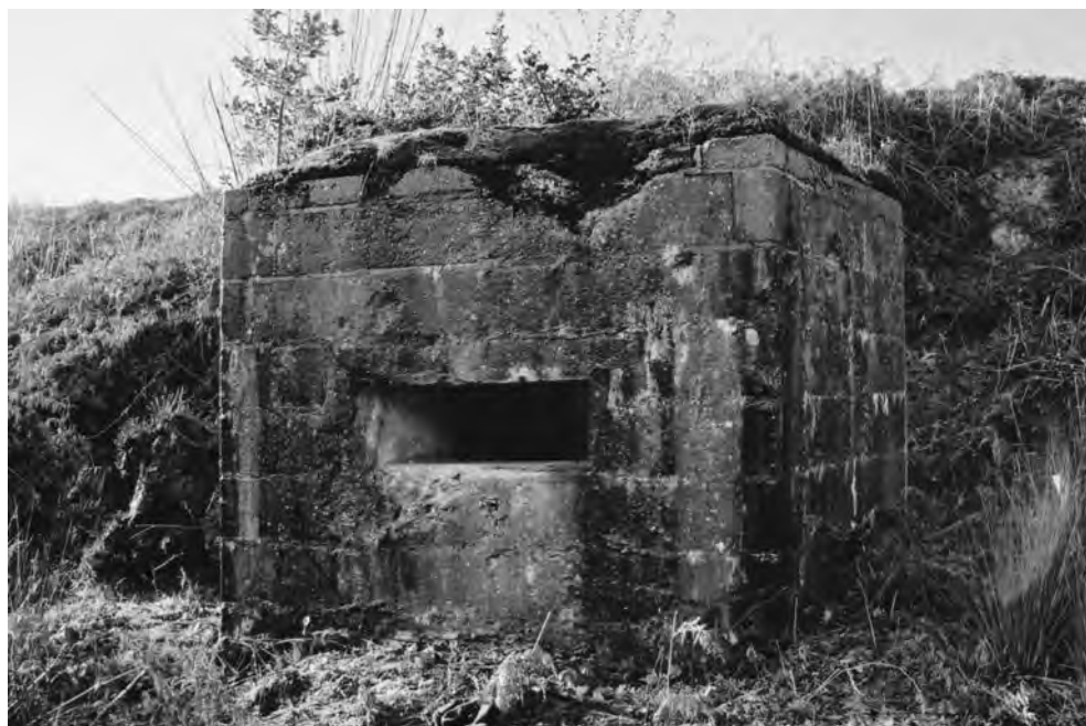
FIGURE 27 Medium machine gun pillbox [7716]. It shows damage probably caused during assault training in 1943/44. (PHOTO: THE AUTHOR, 19 JANUARY 2003)
