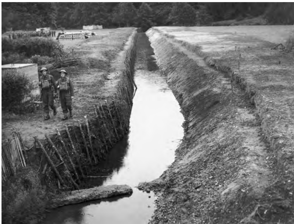
FIGURE 4 Length of anti-tank ditch on the GHQ Line near Farnham in Surrey, 24 July 1940. The vertical wall of the ditch on the defended side has been revetted with timber stakes, and the sloping face on the attack side broadens the width of the obstacle. The anti-tank cube may be the first of a line supporting the ditch or possibly protecting its junction with a road (out of view). Fieldwork should enable the exact location of this photograph to be determined. (PHOTOGRAPH COURTESY OF THE IMPERIAL WAR MUSEUM, LONDON IWM: H2473)
