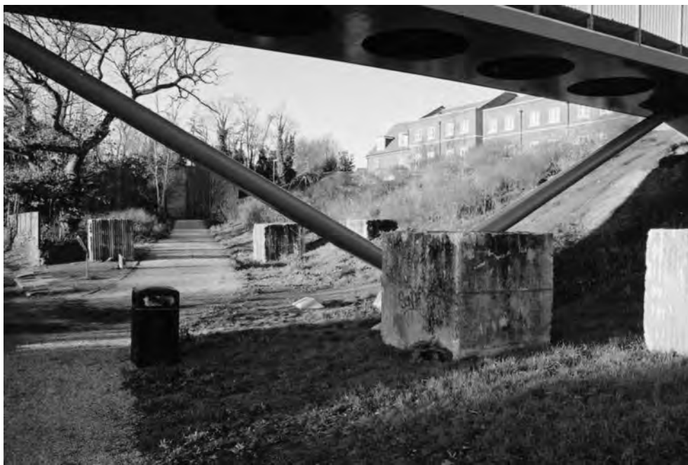
FIGURE 217 The two lines of anti-tank cubes [9509] crossing the towpath of the River Medway at Ringlestone, with the recently built footbridge to Whatman Park running above them. The cubes were part of the north-eastern perimeter defences of Maidstone fortress.
