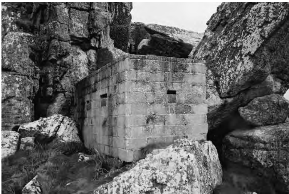
FIGURE 40 Trapezoidal-shaped pillbox [153], built to fit in a cleft in the rocks. It is made of concrete blocks and has very small embrasures. The entrance at the rear can be accessed with difficulty through a narrow gap in the rocks. (PHOTO: THE AUTHOR, 21 JANUARY 2003)
