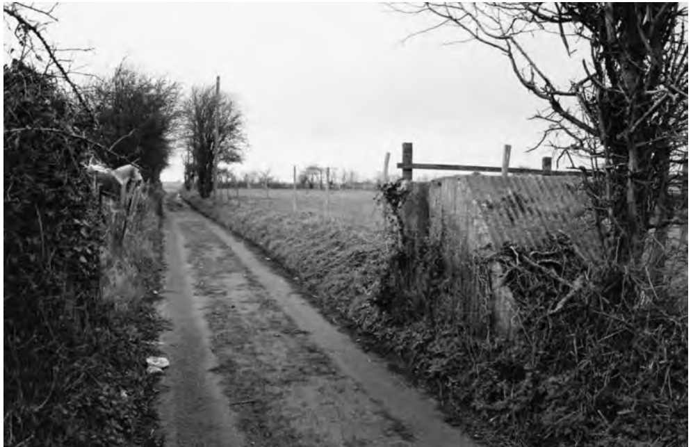
FIGURE 223 The slotted concrete supporting blocks of a horizontal rail roadblock [2707]. The anti-tank ditch crossed diagonally from left to right just beyond the blocks. (PHOTO: THE AUTHOR, 4 MARCH 2003)
