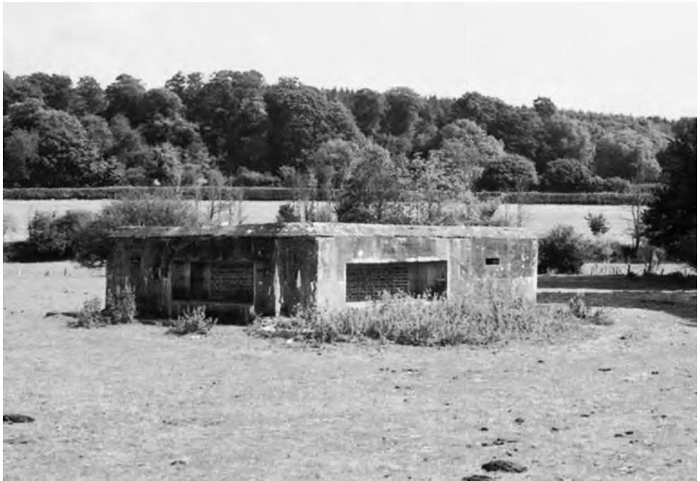
FIGURE 174 Type 28A 2pdr anti-tank gun emplacement [5719] with two main embrasures (now blocked in) facing different angled lengths of the anti- tank ditch in front of it. (PHOTO: THE AUTHOR, 3 SEPTEMBER 2003)
