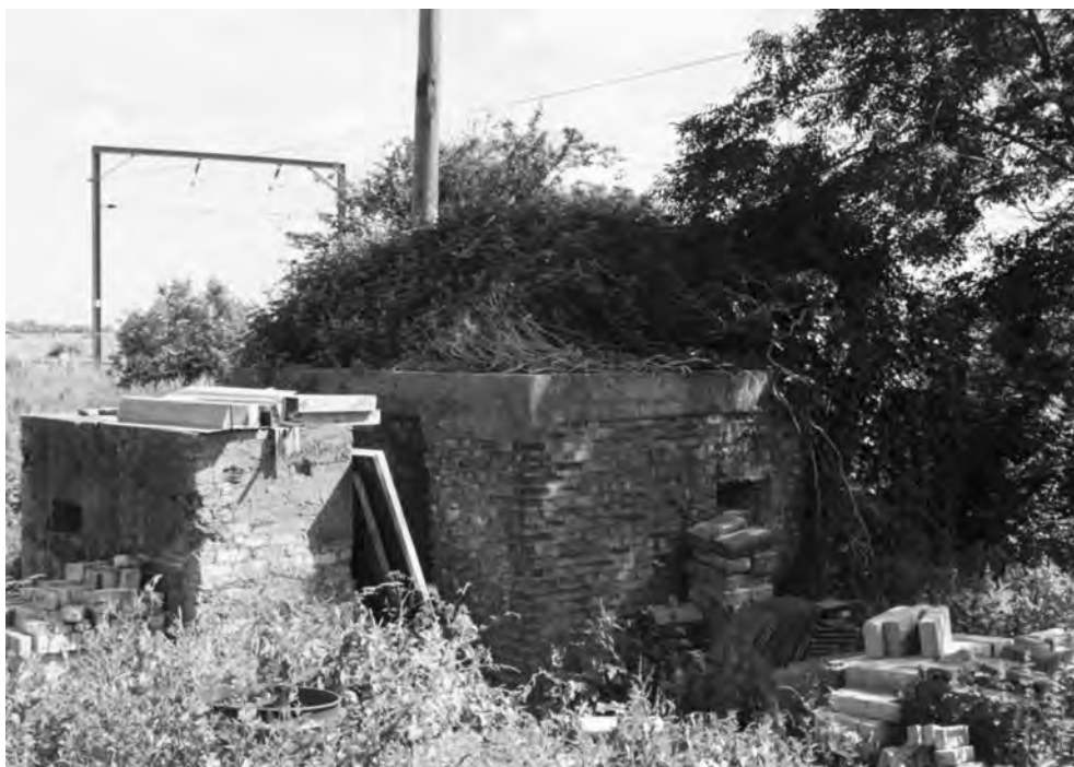
FIGURE 237 Brick-shuttered Eastern Command-type pillbox [4697] behind a house in Victoria Street, Littleport. The bricks facing the blast wall have been removed and may be those piled against it. (PHOTO: THE AUTHOR, 19 JUNE 2002)
