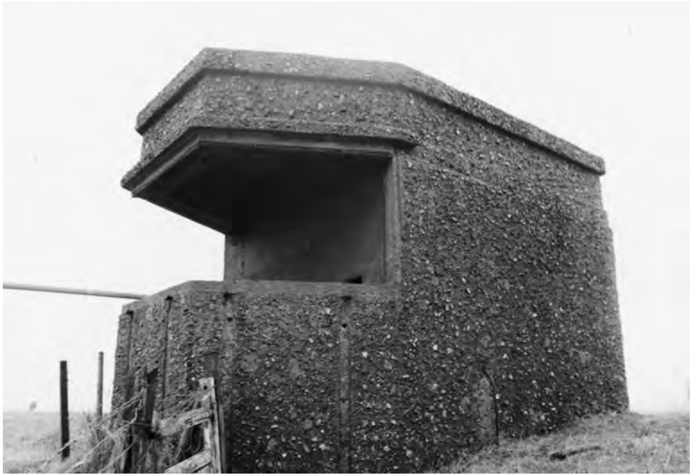
FIGURE 79 Structure to hold one of the two artillery searchlights (CASL) of the Freiston Shore Battery [16244]. (PHOTO: THE AUTHOR, 21 OCTOBER 2002)
