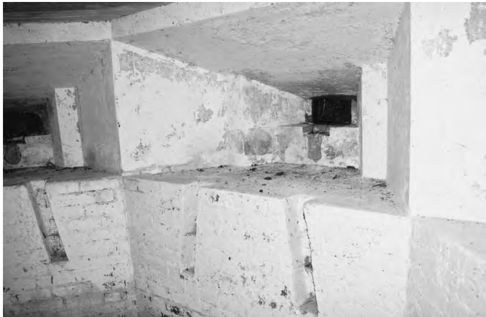
FIGURE 207 Interior of pillbox [663]. The slots in the whitewashed brickwork beneath the embrasures were to take the mountings for Bren light machine guns so that they could be fired on fixed lines. The thickness of the walls (42in/1.1m) can be appreciated from the depth of the splayed embrasures. (PHOTO: THE AUTHOR, 4 DECEMBER 2003)
