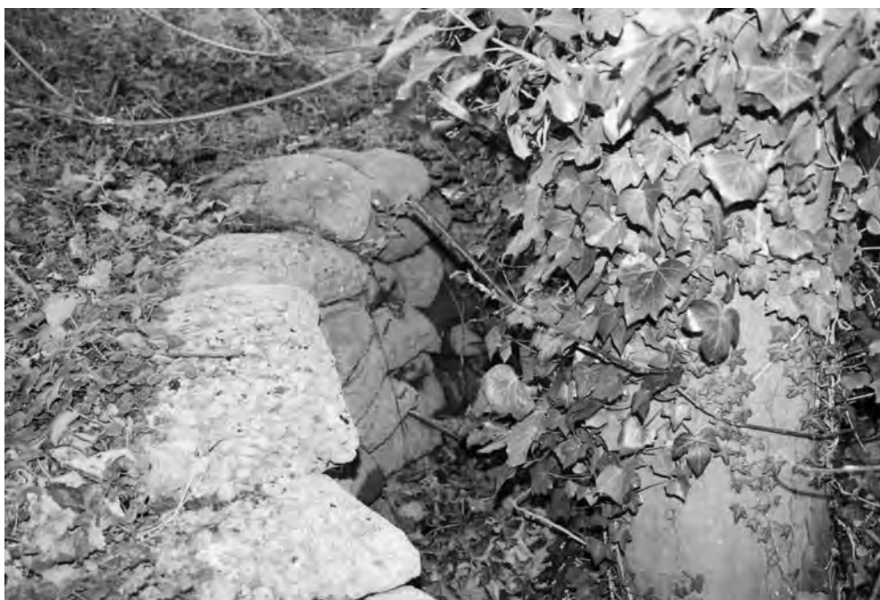
FIGURE 259 One of two weapon pits formed of concreted sandbags [16953] on the south side of Jude's Ferry Bridge. They have survived because trees were planted within them.
