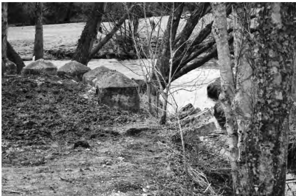
FIGURE 124 More anti-tank cubes by the mill race with, in the foreground, a number of concrete posts set at an angle in the river bank [16428]. The latter represents a defence work type that rarely survives: other examples to the south-west have been destroyed in recent years. (PHOTO: THE AUTHOR, 14 JANUARY 2003)
