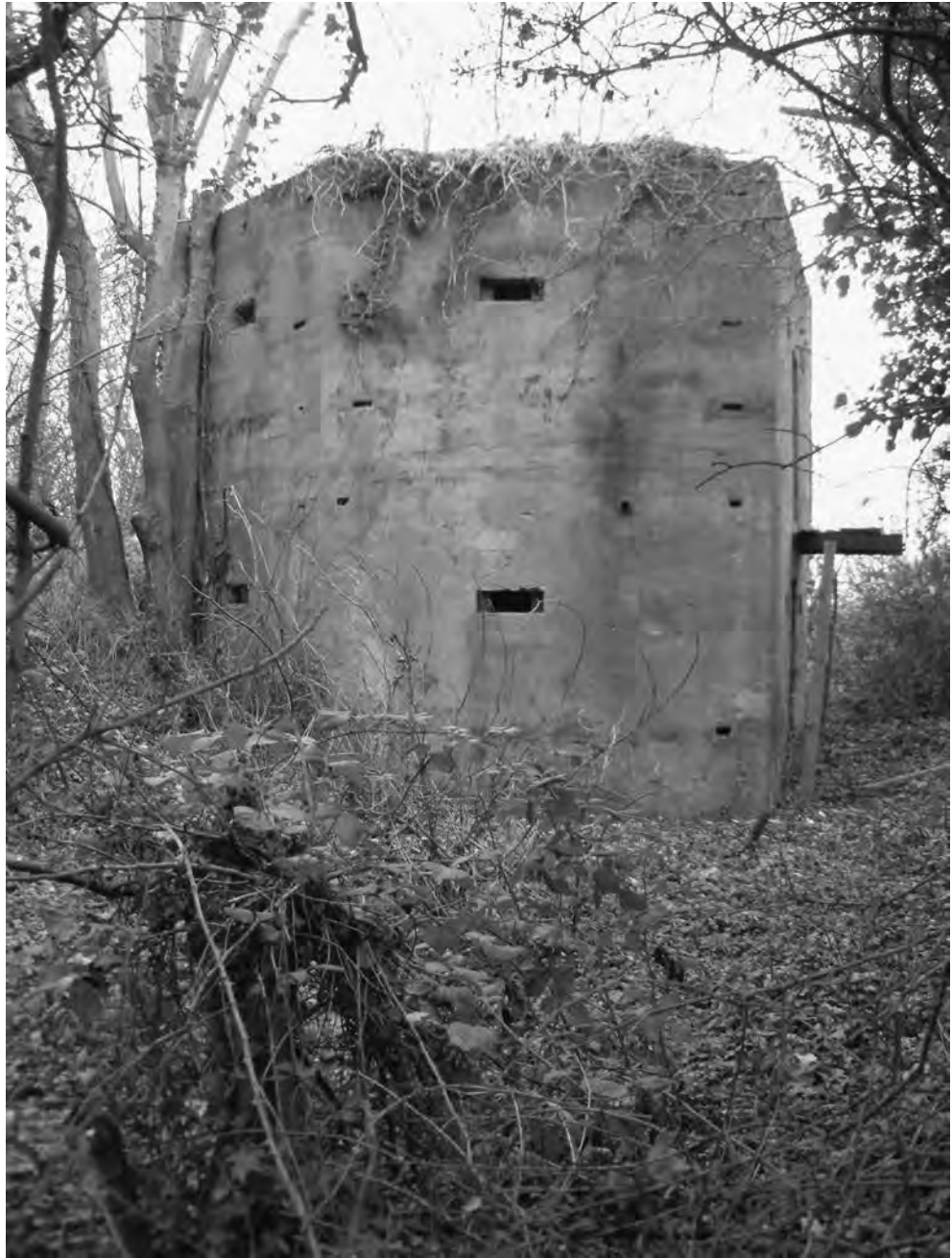
FIGURE 272 A rare two-storey pillbox [6780] constructed on the basic ground plan of a Type 24. It was built with an upper level of embrasures so that fire was possible across the railway embankment to the west as well as to the north and south. (PHOTO: R J C THOMAS, DECEMBER 2004)
