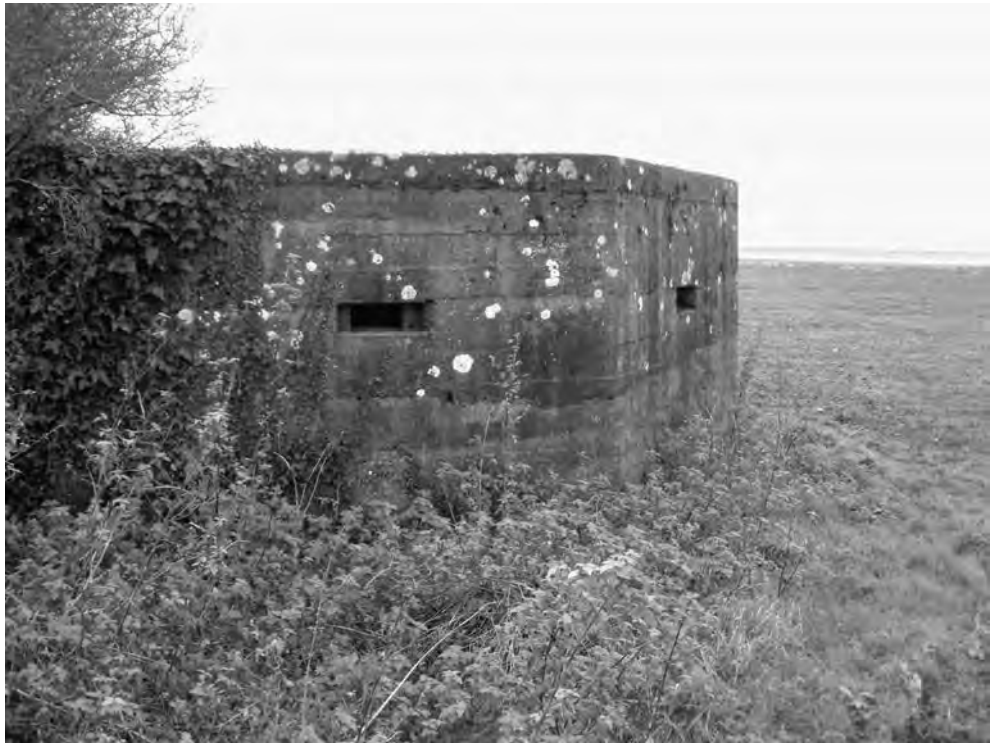
FIGURE 135 Thick-walled Type 24 pillbox [307] on the northern edge of Gaunts Road. (PHOTO: R J C THOMAS, DECEMBER 2004)
