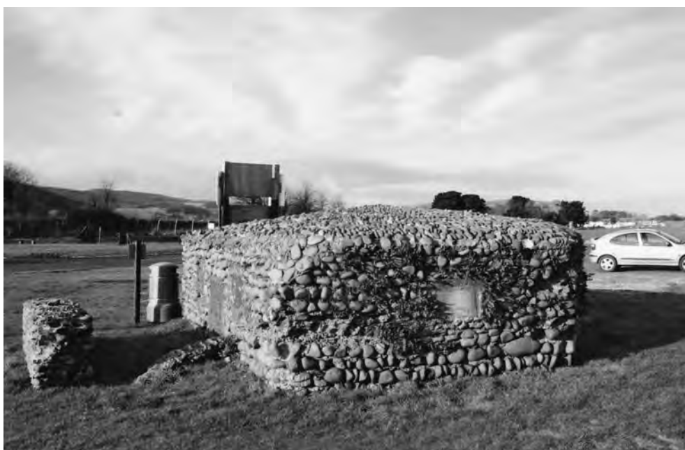
FIGURE 43 Type 24 pillbox [3024] with a detached blast wall, and with entrance and embrasures now blocked. The extensive use of beach pebbles as camouflage cladding is clear. The pillbox has become a feature in the Dunster Beach car park with signs placed against it. (PHOTO: THE AUTHOR, 16 JANUARY 2003)
