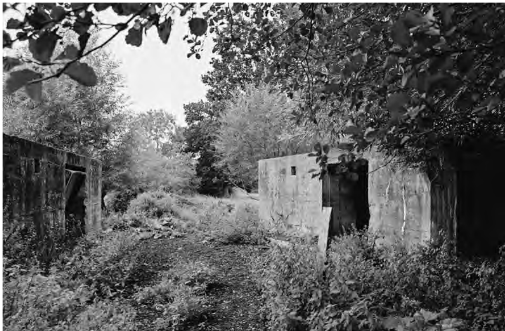
FIGURE 175 Single embrasure Type 28A anti-tank gun emplacements positioned back-to-back north of Oaklands Farm [16664 and 2682]. Each of these emplacements had a separate chamber for light machine gun fire. (PHOTO: THE AUTHOR, 3 SEPTEMBER 2003)
