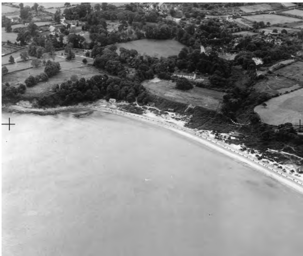
FIGURE 24 Oblique air photograph taken 16 August 1941 showing the defences around Redend Point. Tubular steel scaffolding and barbed wire line the beach, and a side valley is blocked by anti-tank cubes. Amongst various buildings on the beachfront are probably camouflaged gun positions. Fort Henry on wooded Redend Point has yet to be built, although the 4in gun emplacement behind its future site can just be made out. (ENGLISH HERITAGE (NMR) RAF PHOTOGRAPHY: MSO 31243/PO-046 SZ 0382/3)
