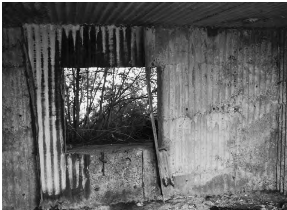
FIGURE 228 Corrugated-iron sheeting used as shuttering for the interior of Type 28A anti-tank gun emplacement [7186] at Hartford End. (PHOTO: THE AUTHOR, 16 MAY 2002)
