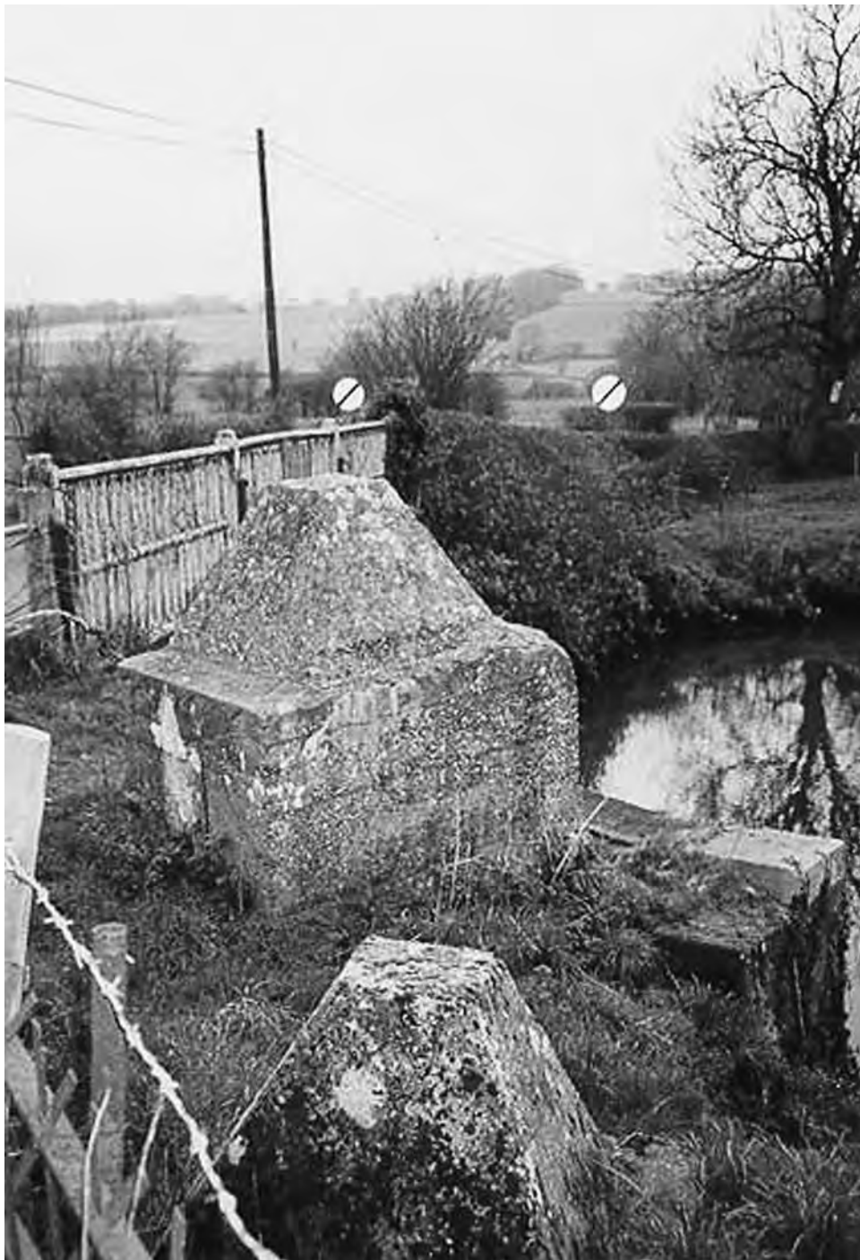
FIGURE 7 Anti-tank pimples at Chafford Bridge on the River Medway south of Penshurst, Kent. These concrete obstacles, known popularly as 'dragon's teeth', would have supported a roadblock at the bridge. Together with pillboxes, 'dragon's teeth' are the defence work most synonymous in the public mind with the events of 1940. (PHOTO: THE AUTHOR, 1998)
