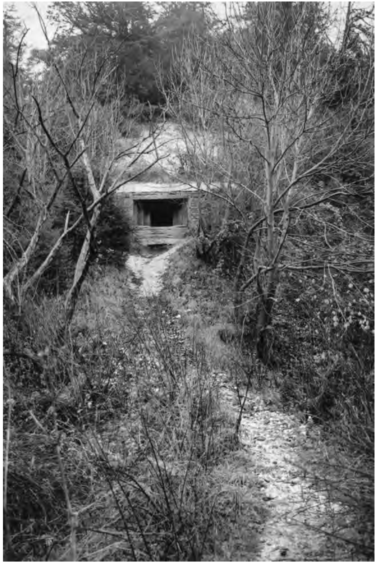
FIGURE 191 Emplacement for the 6pdr Hotchkiss anti-tank gun [9423] dug into the steep side of Box Hill. It commanded the line of the anti-tank ditch and the roadblock below. (PHOTO: THE AUTHOR, 3 DECEMBER 2003)
