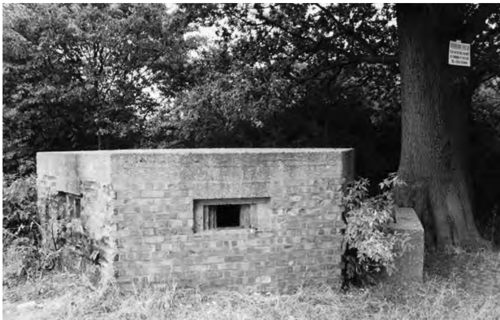
FIGURE 244 Type 22 pillbox [584] in Cheshunt Park with stepped embrasures and a low entry porch. It has been damaged recently by a fire lit against it, and the interior is full of rubbish. (PHOTO: THE AUTHOR, 22 AUGUST 2003)
