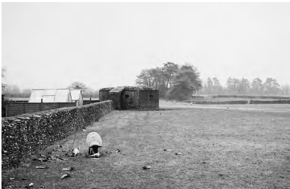
FIGURE 156 Type 24 pillbox [6850] at Star Farm Cottages on the attack side of the anti-tank ditch. It has a brick and concrete entry porch which served to protect the interior from blast. (PHOTO: THE AUTHOR, 6 FEBRUARY 2003)
