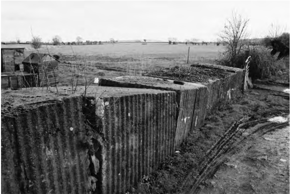
FIGURE 145 Anti-tank cubes [13973] from the line on the east side of Higher Bridge Farm. They have been moved from their original position and lined up by a farm track. The concrete shows evidence of the corrugated-iron shuttering used in their construction.
