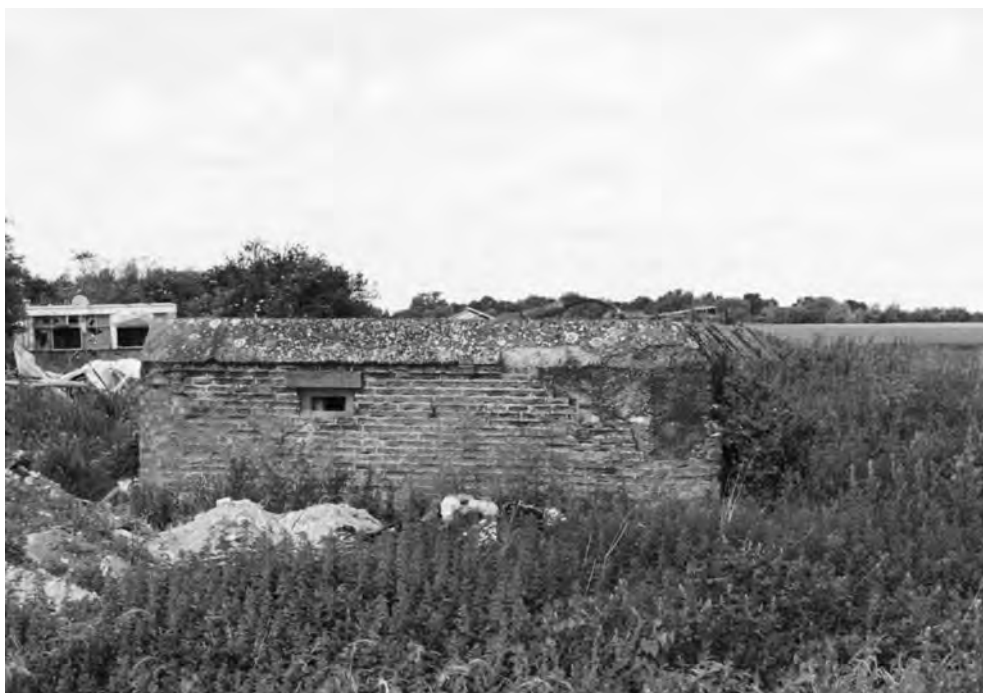
FIGURE 239 Type 28A anti-tank gun emplacement [1573] in a dilapidated condition in a yard off Cross Drove, east of Littleport. It controlled the north-eastern approaches to the town at the junction of two stop lines. (PHOTO: THE AUTHOR, 19 JUNE 2002)
