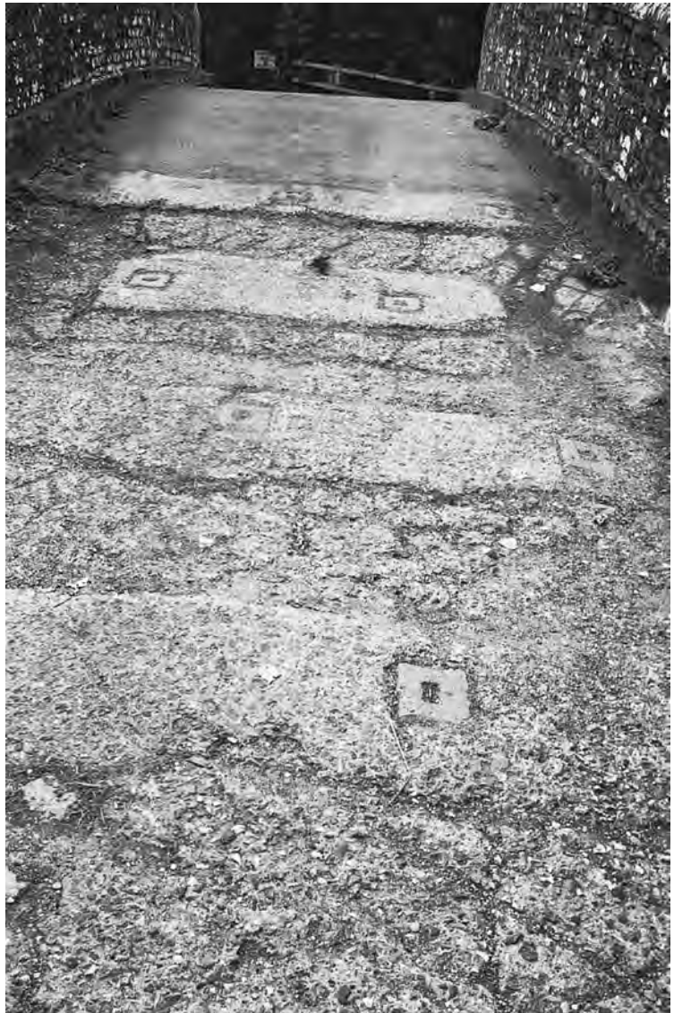
FIGURE 167 Plugged concrete sockets [8822] to take vertical rails to form a block on the bridge over the Kennet and Avon Canal at Wire Lock. (PHOTO: THE AUTHOR, 3 SEPTEMBER 2003)
