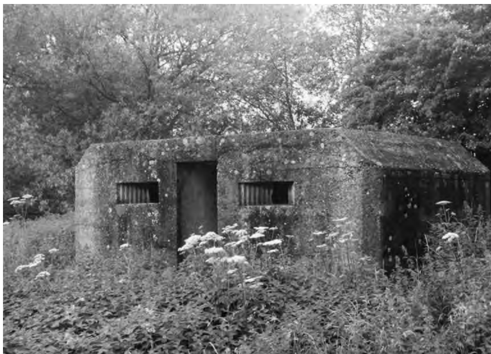
FIGURE 234 Shell-proof Type 24 pillbox [391], one of a pair of these pillboxes at a strongpoint by the River Cam north of Audley End. (PHOTO: THE AUTHOR, 7 JUNE 2002)
