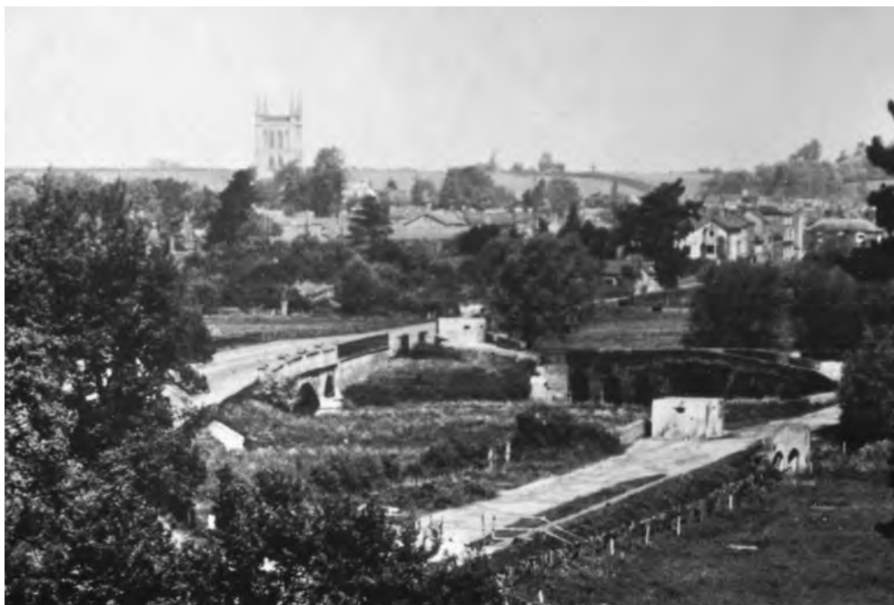
FIGURE 313 Photograph taken c 1946 showing the two pillboxes on Pershore old bridge shortly before their removal. (PHOTO: M FREEMAN)
