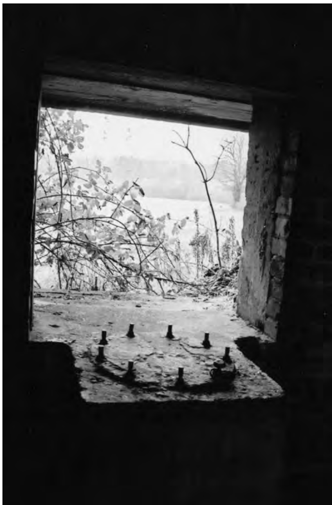
FIGURE 213 Holdfast for the 6pdr Hotchkiss gun in Type 28 emplacement [2434] north of Long Bridge on the River Eden.
