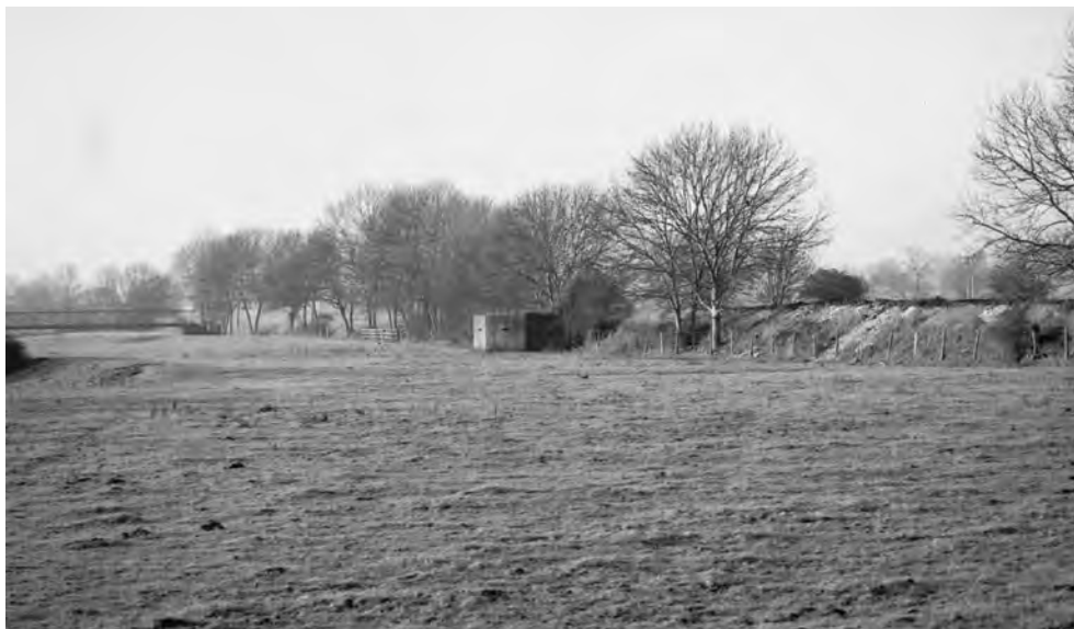
FIGURE 203 Type 24 pillbox [705] built against the embankment of the former railway line south-west of Barcombe Mills. (PHOTO: THE AUTHOR, 9 DECEMBER 2003)
