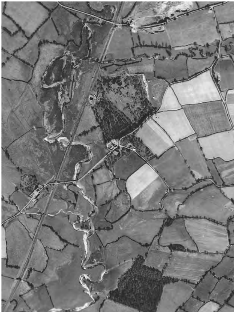
FIGURE 127 Air photograph taken 11 April 1947 of the Wadbroom defence area, showing the twisting course of the River Axe and the straight line of the railway. Towards the bottom left of the photograph, the river is crossed by a lane at Axe Bridge. The defence line was straightened and strengthened by digging short lengths of anti-tank ditch across the base of several of the river loops. These ditches still awaited backfilling when the photograph was taken. (RAF/CPE/UK/1974 fr4323. ENGLISH HERITAGE (NMR) RAF PHOTOGRAPHY)
