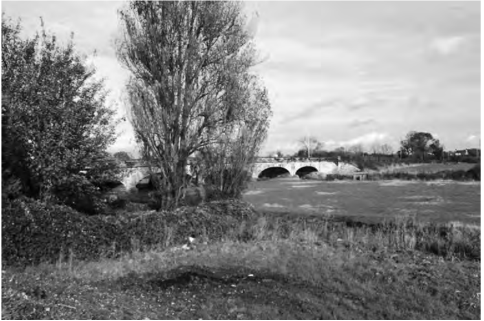
FIGURE 261 Hopwas Bridge seen from pillbox [5336]. (PHOTO: THE AUTHOR, 28 OCTOBER 2002)
