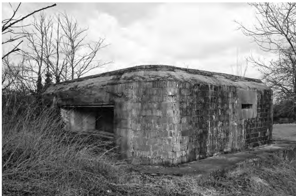
FIGURE 160 Type 28A 2pdr anti-tank gun emplacement [8113] with a side chamber for an infantry section. It commanded the road into Semington close to the anti-tank ditch on the southern perimeter. (PHOTO: THE AUTHOR, 4 FEBRUARY 2003)
