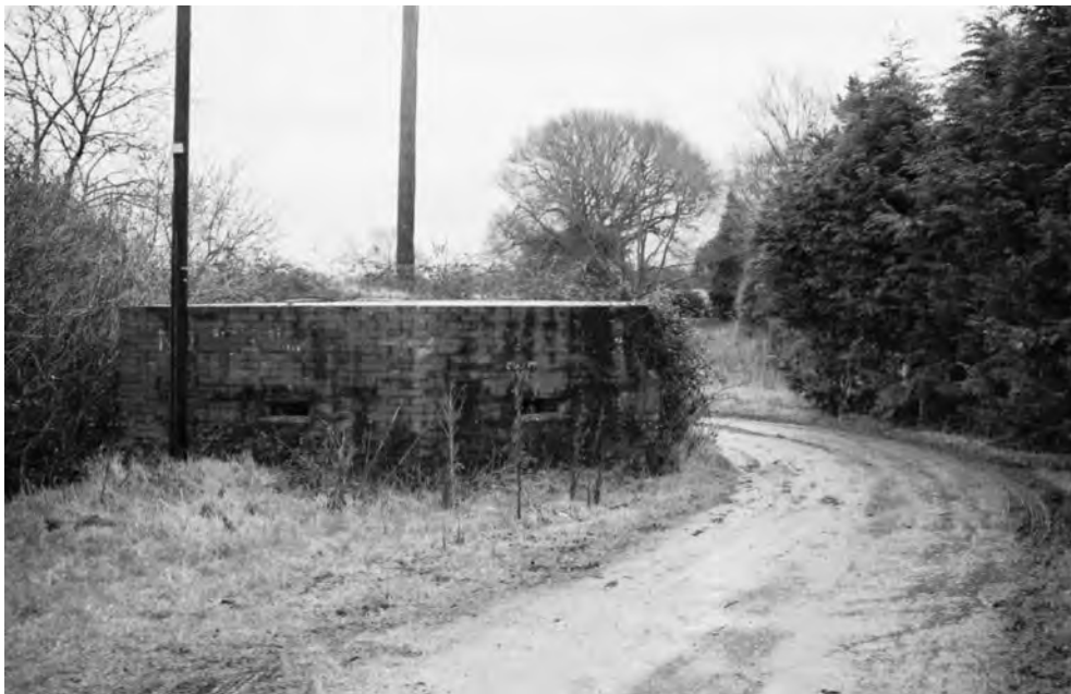
FIGURE 142 Type 24 pillbox [5667] close to River Bridge. (PHOTO: THE AUTHOR, 17 JANUARY 2003)
