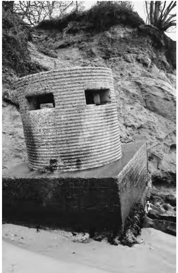
FIGURE 28 Type 25 pillbox [7718], shuttered with corrugated iron, in an exposed position beneath the cliffs of Redend Point. Its 54in (1.4m) thick base anchoring it in position has led to its remarkable survival. (PHOTO: THE AUTHOR, 19 JANUARY 2003)
