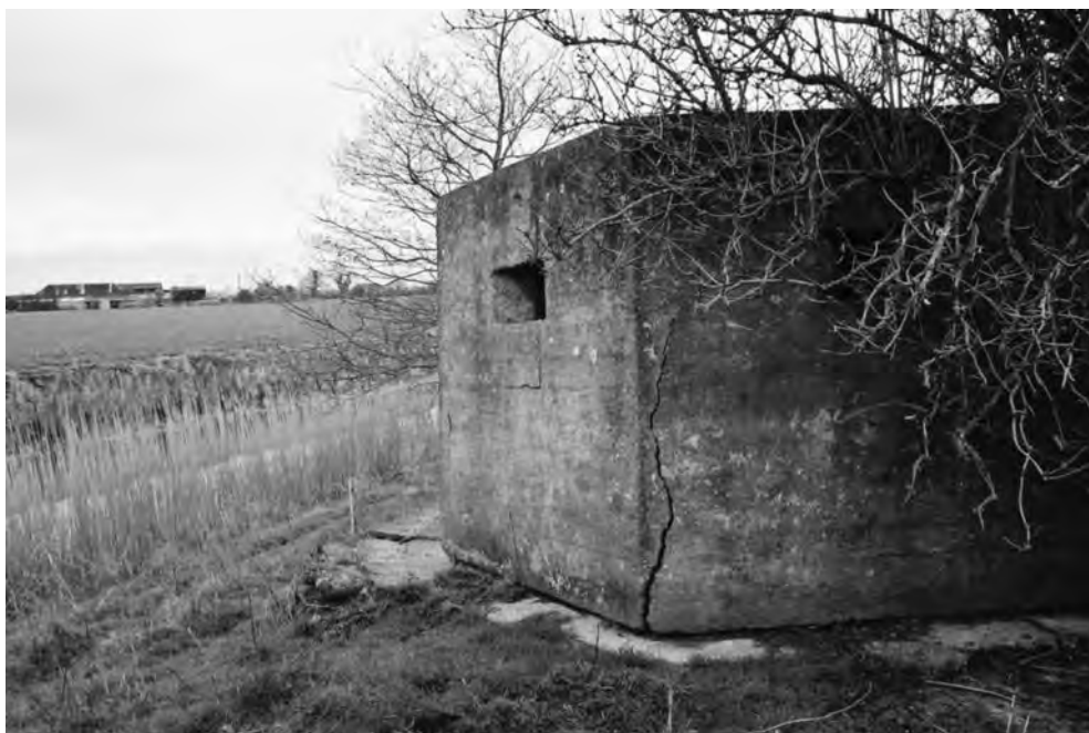
FIGURE 117 Type 22 infantry pillbox [8224] on the north bank of the Royal Military Canal east of Bilsington Bridge. Its walls are now badly cracked. This pillbox is recorded as 'unmanned' on an October 1940 defence map. (PHOTO: THE AUTHOR, 12 FEBRUARY 2004)
