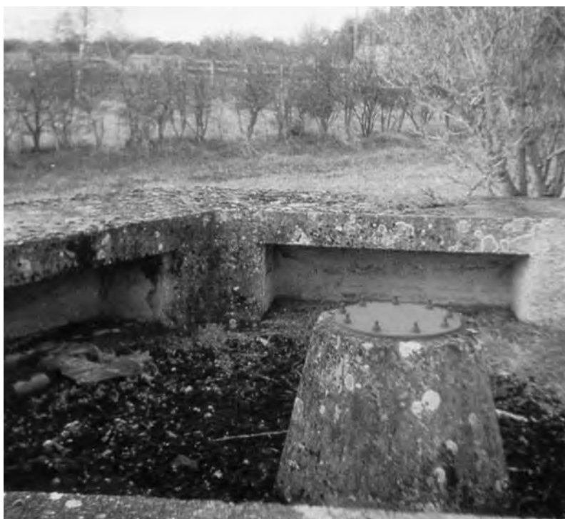
FIGURE 172 A 6pdr gun pit at Frilford [7200], with central pedestal and hold-fast to mount the swivelling Hotchkiss 'QF' gun. Lockers for ammunition surround the emplacement. (PHOTO: L C SMITH)
