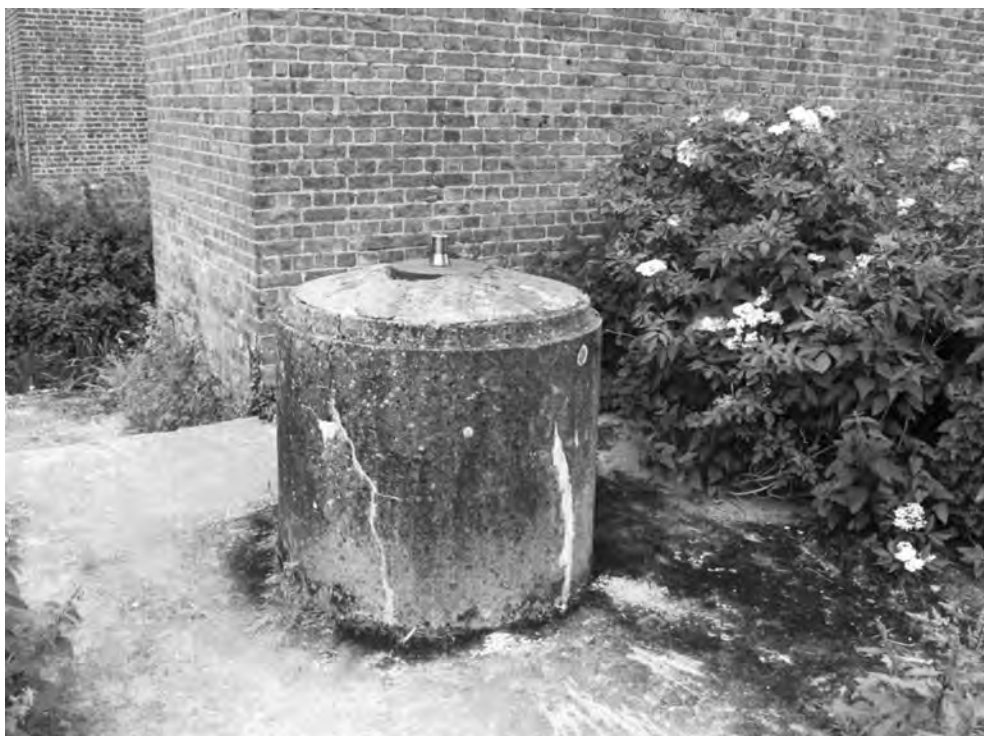
FIGURE 250 Spigot mortar pedestal [15691], one of two spigot mortar firing positions by the viaduct close to the south bank of the River Colne. (PHOTO: THE AUTHOR, 14 JUNE 2002)
