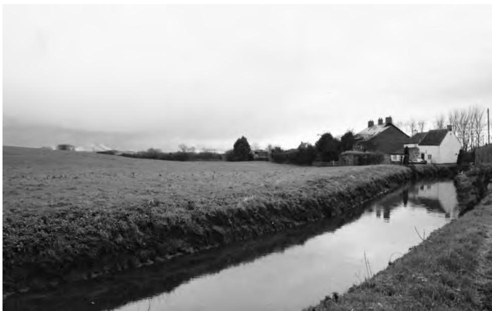
FIGURE 144 At Upper Godney, the anti-tank ditch [16340] ran diagonally across this meadow supplementing the obstacle provided by the River Sheppey in the foreground. Pillbox [8390] can be seen by the houses. (PHOTO: THE AUTHOR, 17 JANUARY 2003)
