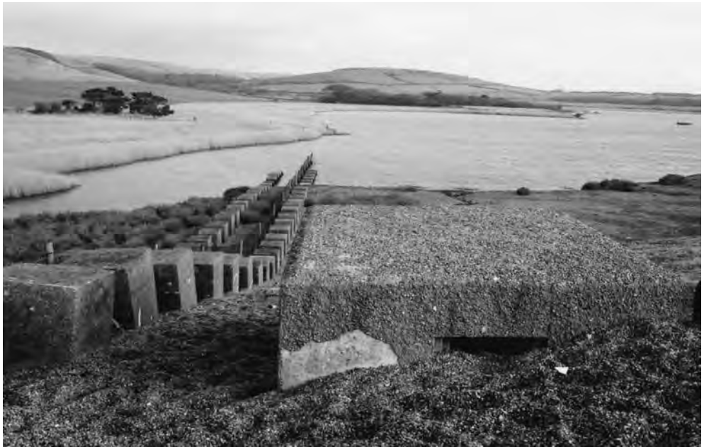
FIGURE 21 The double line of cubes forming the anti-tank barrier [12099] crosses the northern slope of the Chesil Bank and extends into the waters of the West Fleet. Pillbox [3114] is now half-buried by shingle. (PHOTO: THE AUTHOR, 18 JANUARY 2003)
