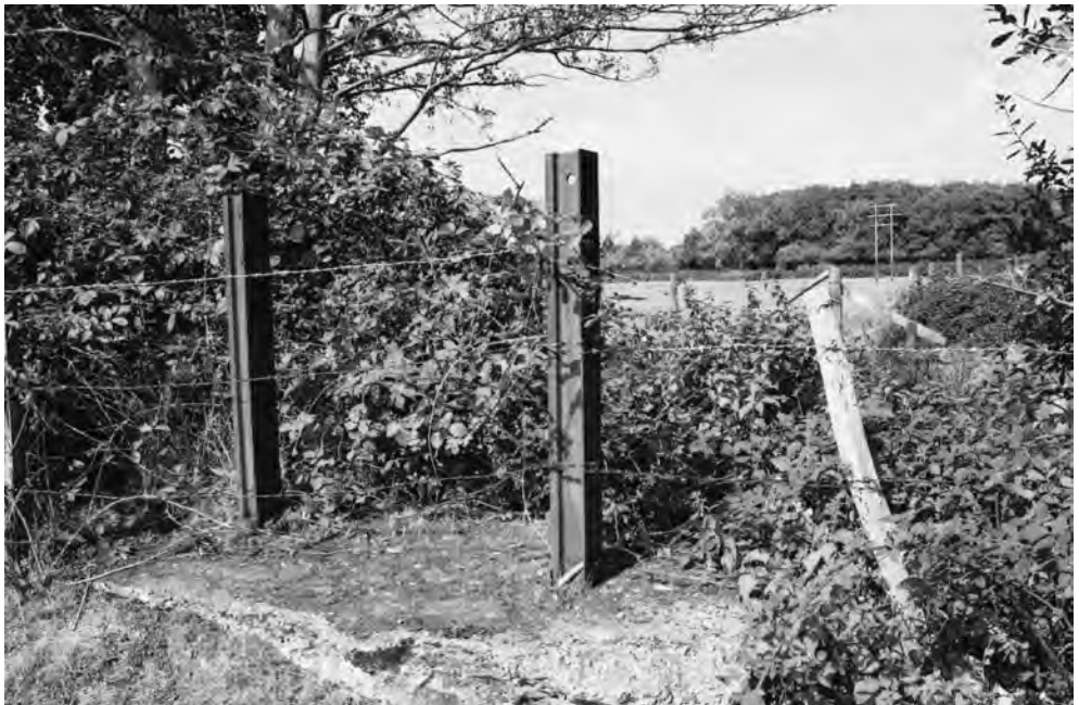
FIGURE 177 These two vertical steel rails set in a concrete base [5717], used today as posts for a barbed wire fence, once blocked a gap in the anti-tank ditch south of Sulham. Other rails may be hidden by bushes. (PHOTO: THE AUTHOR, 3 SEPTEMBER 2003)
