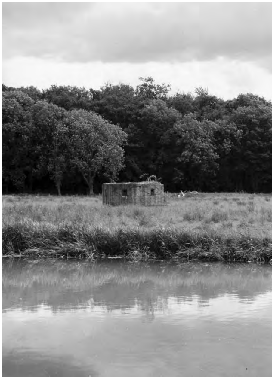
FIGURE 255 Type 27 pillbox [6411], with brick shuttering removed, on the far bank of the Stour south of Sudbury. Steel plates are in place at the embrasures.
