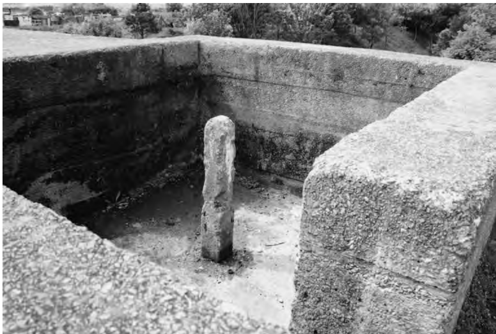
FIGURE 50 The concrete post for mounting an anti-aircraft gun in the open rear bay of Type 23 pillbox [16618]. (PHOTO: THE AUTHOR, 21 MAY 2003)
