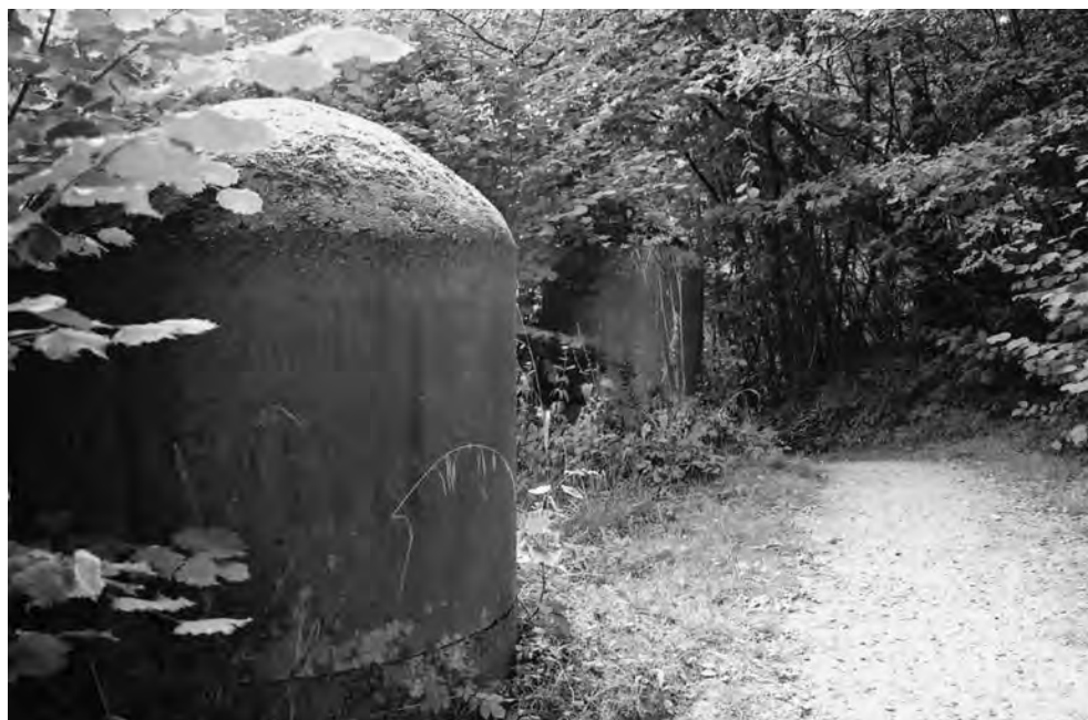
FIGURE 182 Massive domed anti-tank cylinders [16752] on the towpath of the Basingstoke Canal opposite Coxmoor Wood. This was the point where GHQ Line 'A' joined the Canal having crossed Coxmoor Wood by a double line of some 300 similar cylinders. (PHOTO: THE AUTHOR, 28 AUGUST 2003)
