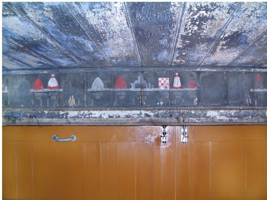
Landguard Fort, Suffolk Battery Observation Post: gunnery range and bearing marks – range is shown above and bearing beneath. The building in the middle is Roughs Tower, a Maunsell fort, an offshore anti-aircraft battery (© R J C Thomas)
