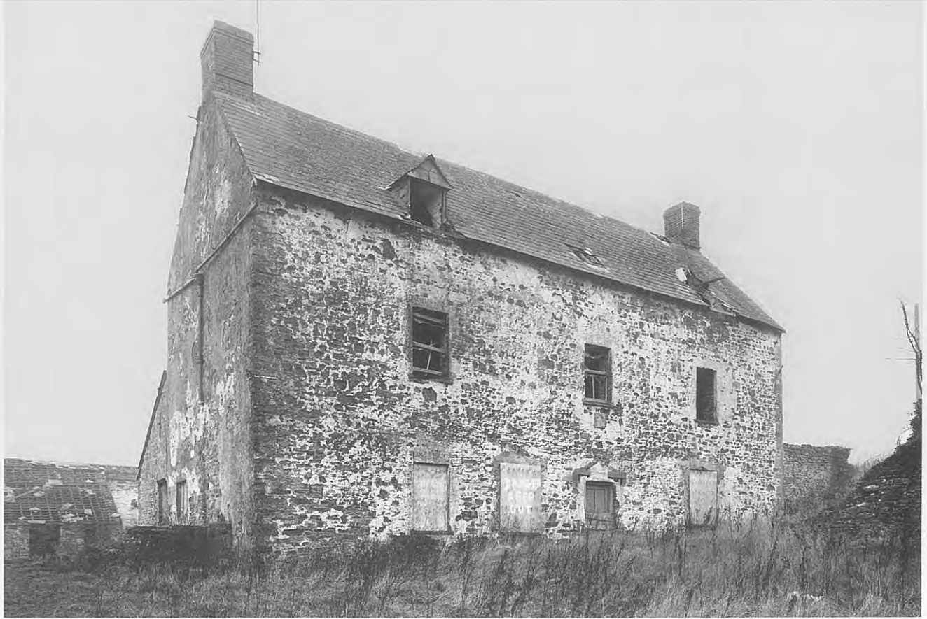
8.1 Penrhos, Caerleon, Monmouthshire. An abandoned multi-period gentry house, a reconstruction dated 1718 of an earlier 17th-century house, itself perhaps with medieval origins. (Crown copyright: RCAHMW)
