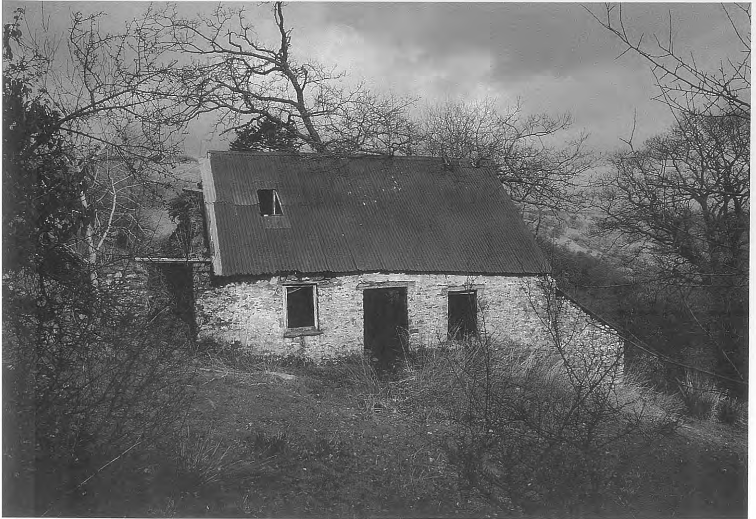
5.11 Abandoned cottage, Mynydd Llansadwrn, Carmarthenshire (photo: Paul Sambrook)
