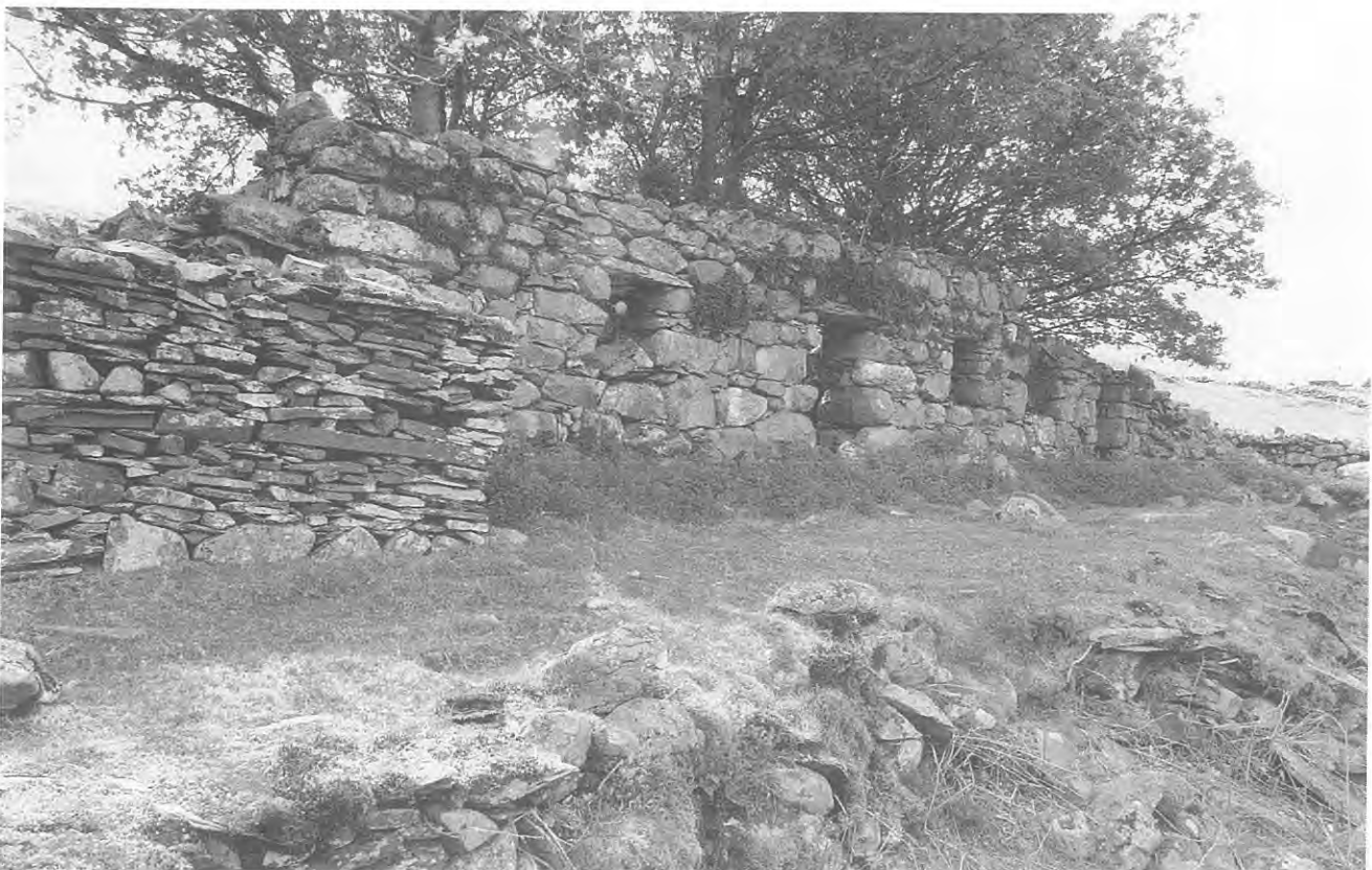
8.2 Ruined quarry cottages above Waunfawr, Gwynedd, clearly illustrating local traditions of stone working (Crown copyright: RCAHMW)
