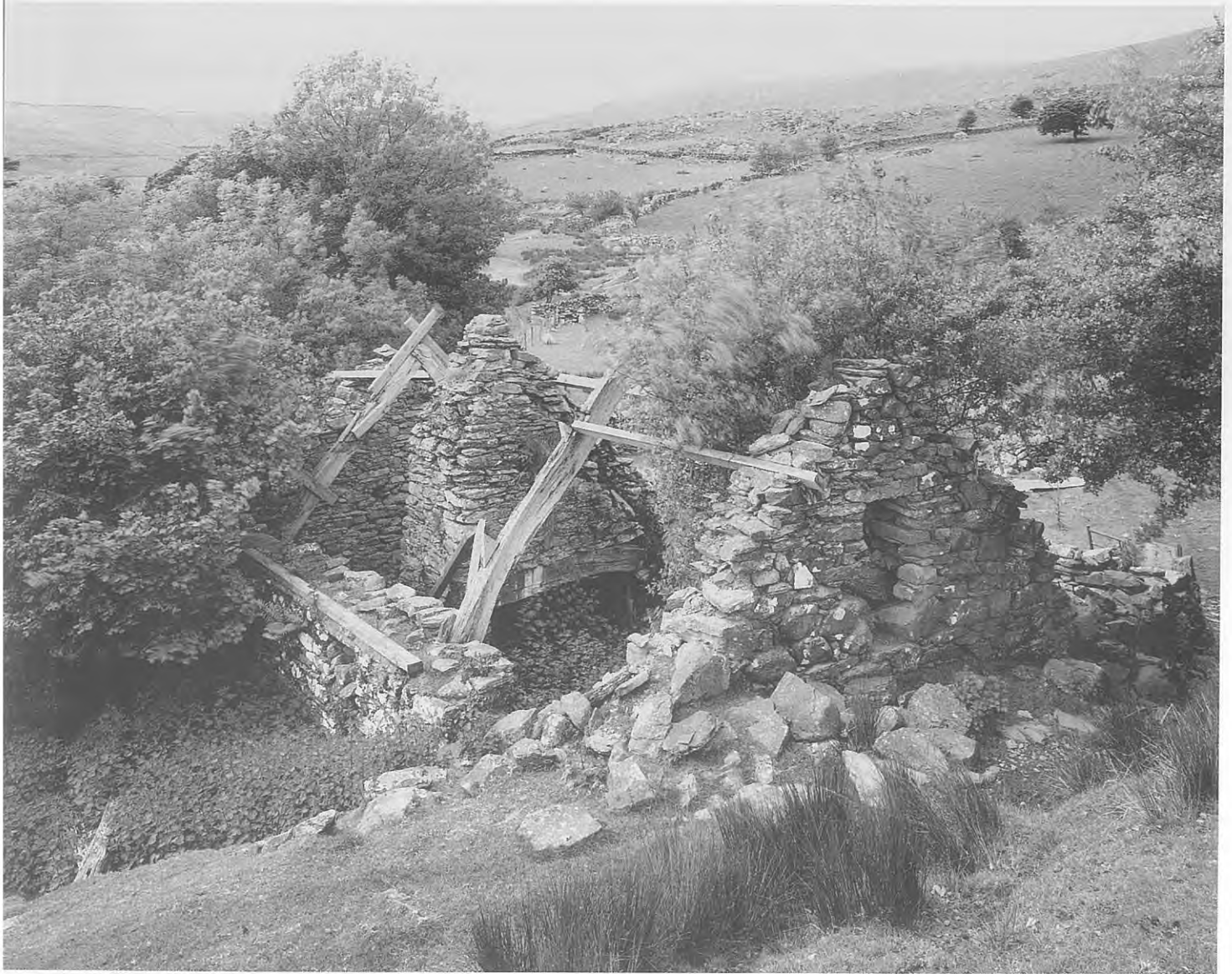
8.6 Relics of a cruck tradition, encapsulated in an upland farm, Llanaber, Gwynedd (Crown copyright: RCAHMW)
