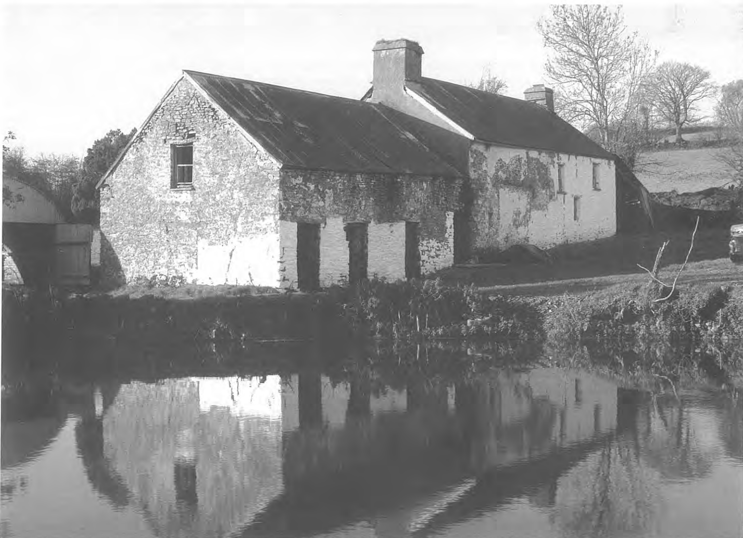
8.11 Rhiwson Uchaf, Ceredigion: exterior. A longhouse-derived plan, in which the house is entered from a through-passage in the adjoining farm range (Crown copyright: RCAHMW)
