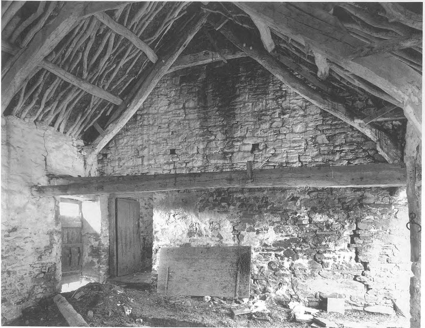
8.12 Rhiwson Uchaf, Ceredigion: interior. This retained a traditional roof construction, in which branches form rough rafters under the thatch (Crown copyright: RCAHMMW)
