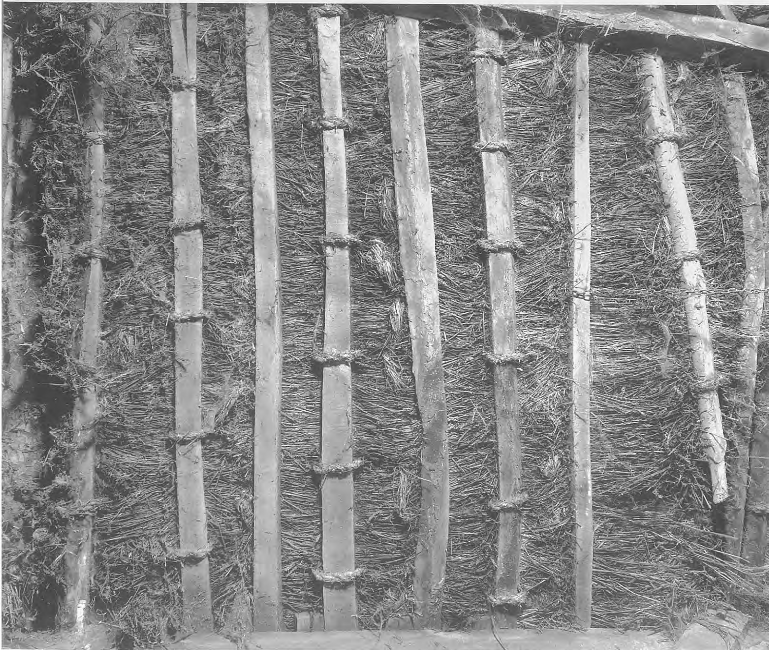
8.10 Abercych, Ceredigion: interior. A simple Ceredigion dwelling recorded in 1997. The underhatch, fixed by rope to rough rafters, provides an example of the type of fragile detail often lost in buildings which remain in use (Crown copyright: RCAHMW)
