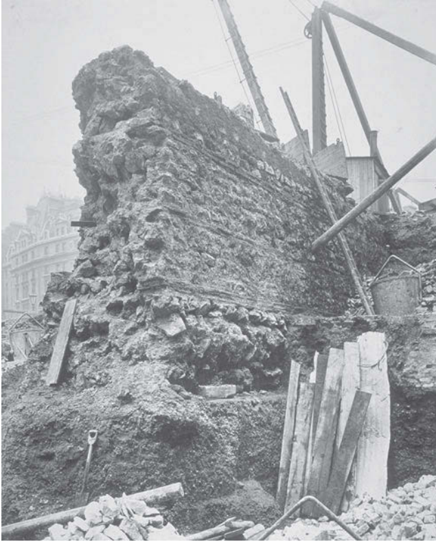
Fig 1.2.12 Anon 1903. View of the excavations at Newgate, showing a portion of the Roman defensive wall. Photograph to paper (maximum dimension 0.29m) (Guildhall Library Print Room La.Pr.446/OLD(1) © Corporation of London)
