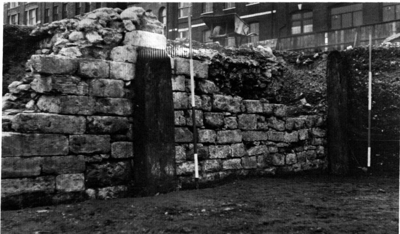
Fig 13 London: timber rubbing posts protected vessels moored in Baynards Castle dock from damage by the stone wall
