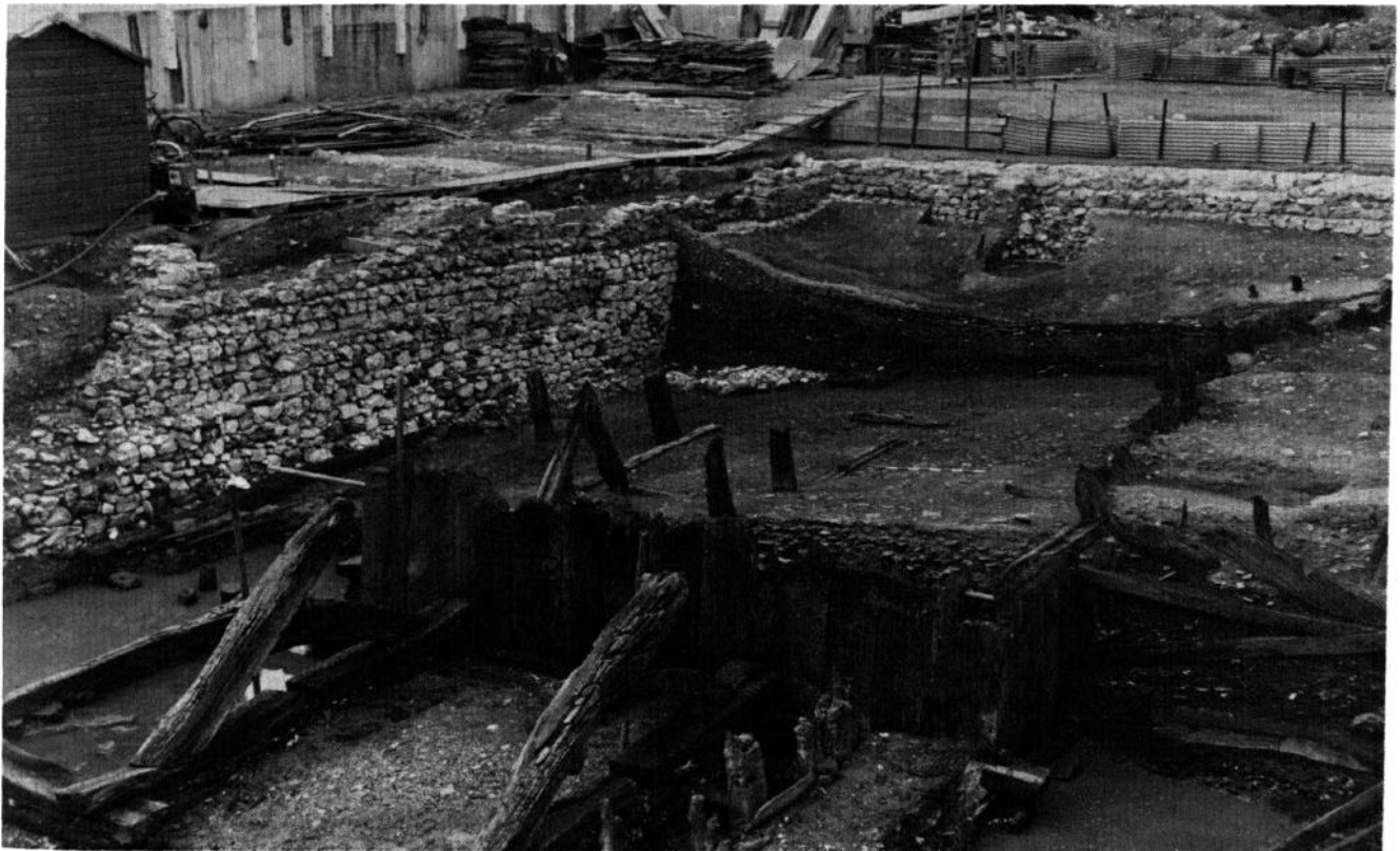
Fig 36 London: Trig Lane excavations looking south-west, river to south, showing back-braced riverfront revetments behind 15th century river wall
