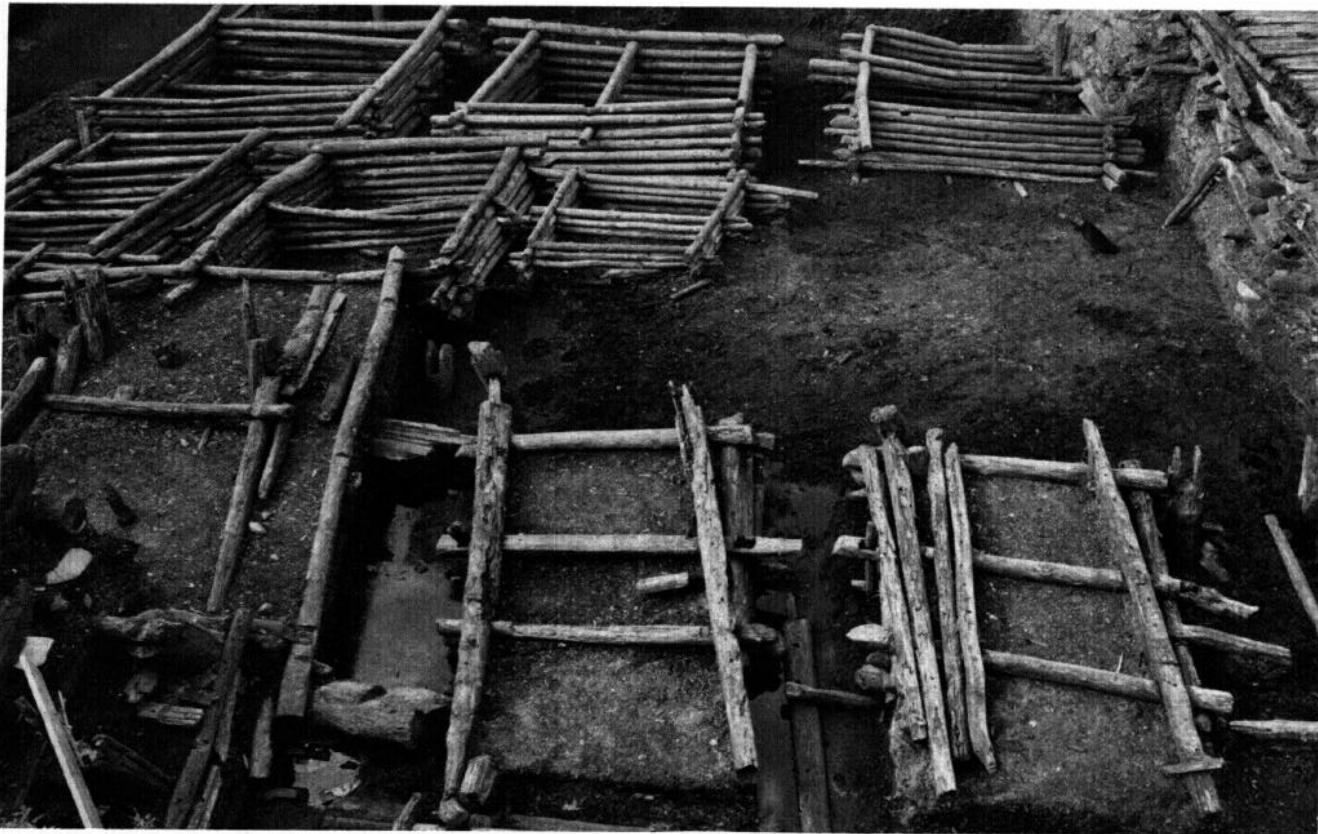
Fig 85 Bergen: square-built timber boxes without stone ballast used as house foundations in deeper water
