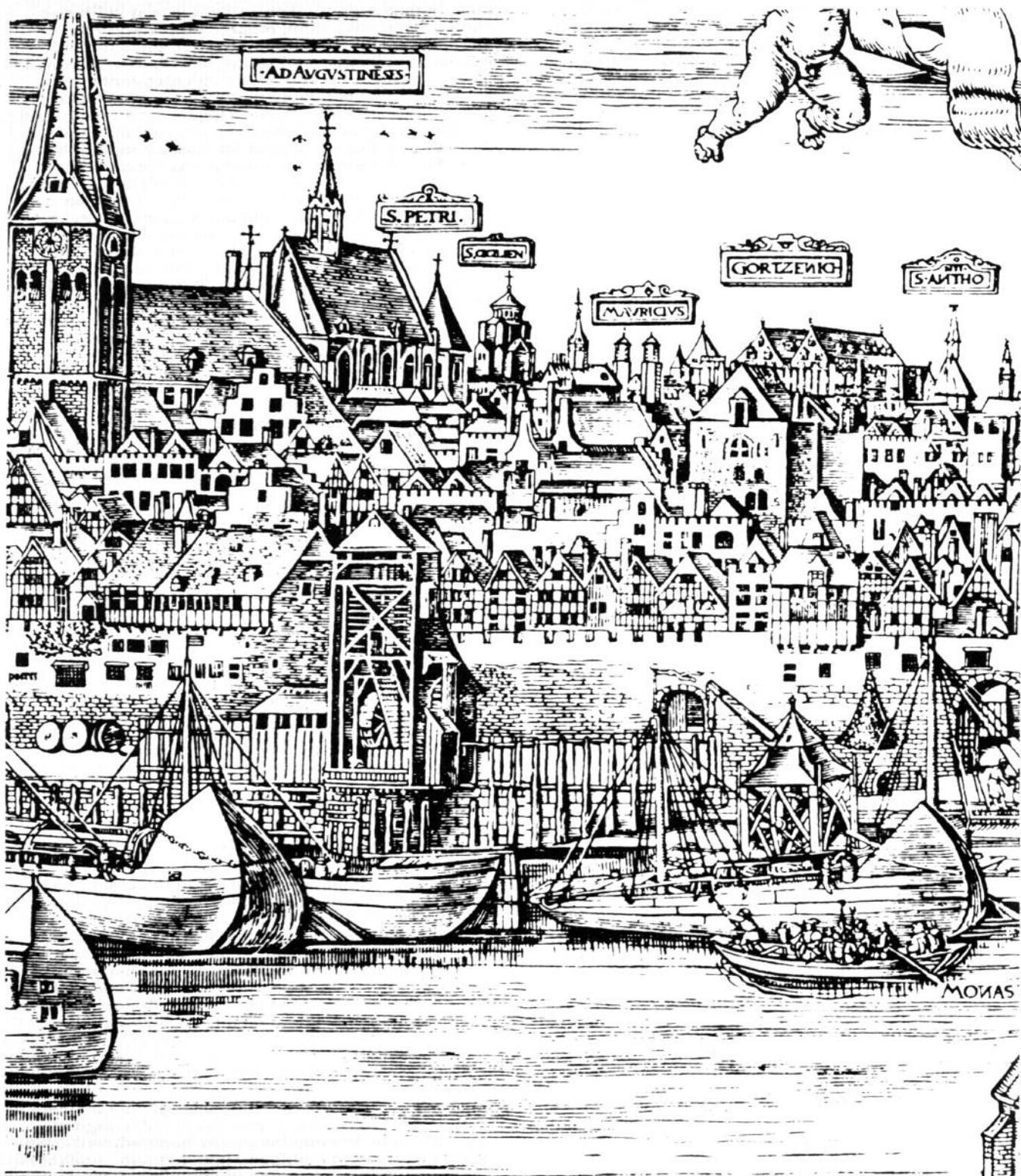
Fig 93 Mast crane and floating crane at Köln (detail from woodcut by A Woensam, 1531)
