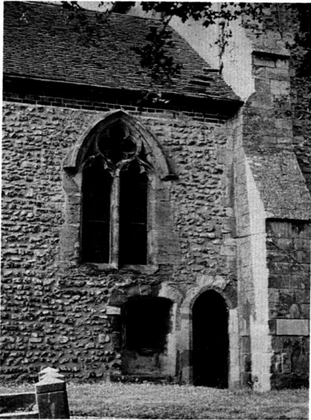
Fig 81 Kingston Buci, West Sussex, St Julian: chancel from north, showing squint
