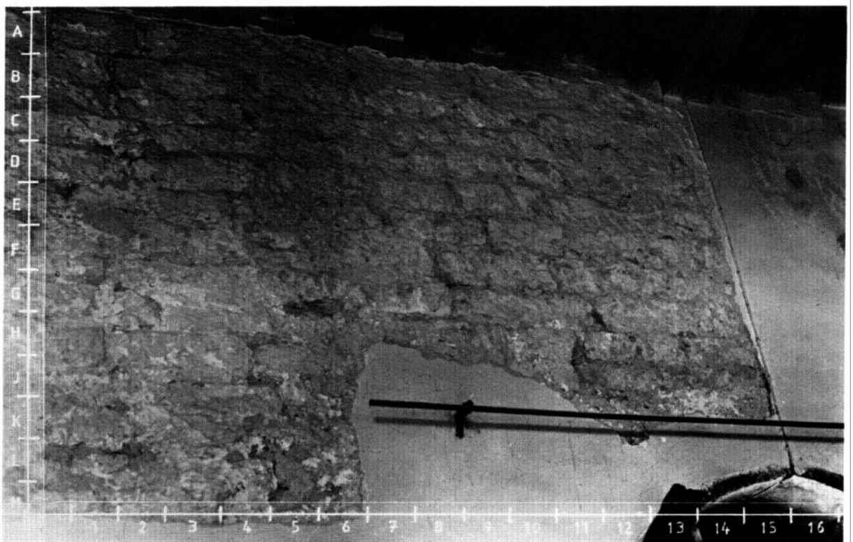
Fig 142 North Muskham church, Notts: south wall of south aisle during plaster stripping using TYPE 4.1 imagery (photo: Christopher J Brooke)
