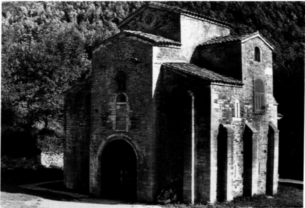
Fig 49 San Miguel de Lillo (Oviedo): church of 9th century, aisles demolished in 17th century; note several trabea type (claustra) window-frames
