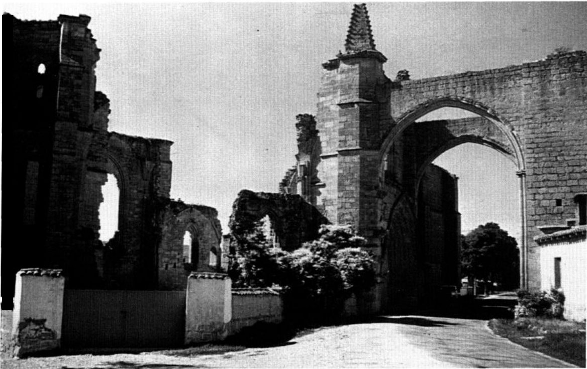
Fig 38 San Anton (Burgos): monastic church; the pilgrim route goes through its 'north transept', entry to the church being through a large doorway in what elsewhere would be the north side of the crossing
