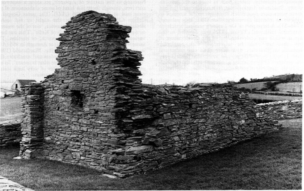
Fig 92 The south church at Deny (Co Down) from the north-east; the church had antae projecting from the east wall, of which the southern survives intact, but the northern has collapsed (Crown copyright, Historic Monuments and Buildings Branch, DOENI)
