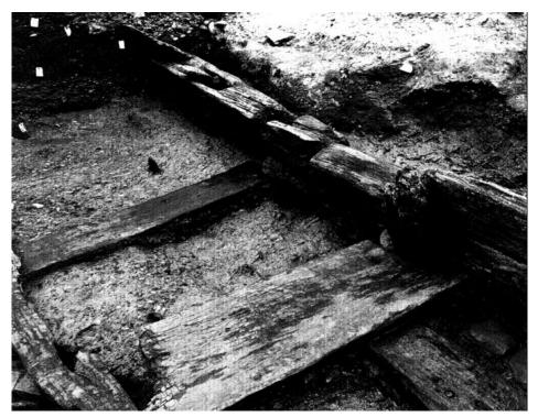
Plate VI Revetment timbers of outfall from SE; W corner of second mill wheelhouse in foreground, with plank 177 and upright 95 on right; timbers 178 and 277 of first mill on left
