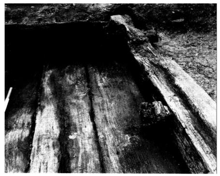
Plate VII N corner of mill 2 wheelhouse from S; by-pass emplacement 296 on upper right; upright 271 and wedge 295 in foreground, set in floor 160 (scale on right in cm and 10cm)
