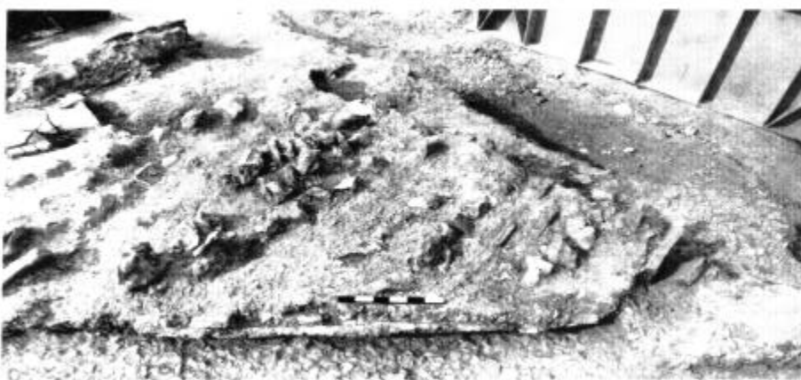
Fig 6.7 Meonstoke: the gable line of the roof of the nave, viewed from the south
