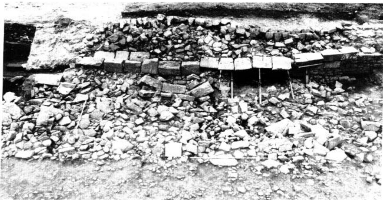
Fig 9.3 Intact panel of the collapsed east wall of the fort
