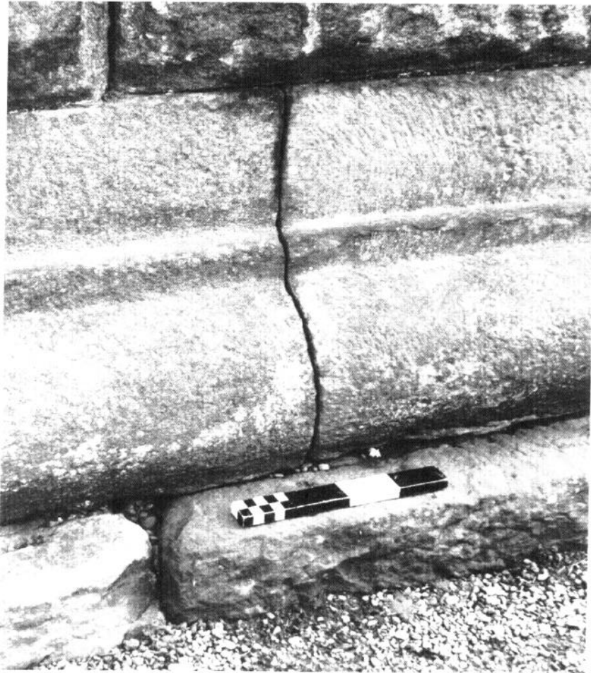
Fig 2.6 Rusticated masonry and base moulding, Building II, Corbridge
