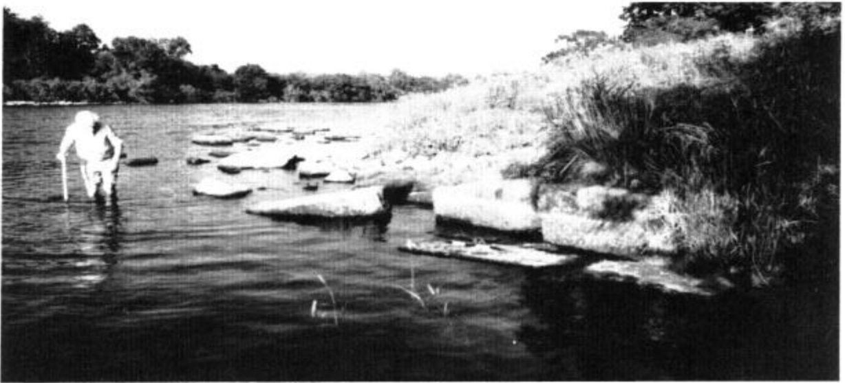
Fig 11.4 Stones of the southern abutment at Corbridge (N Hodgson)
