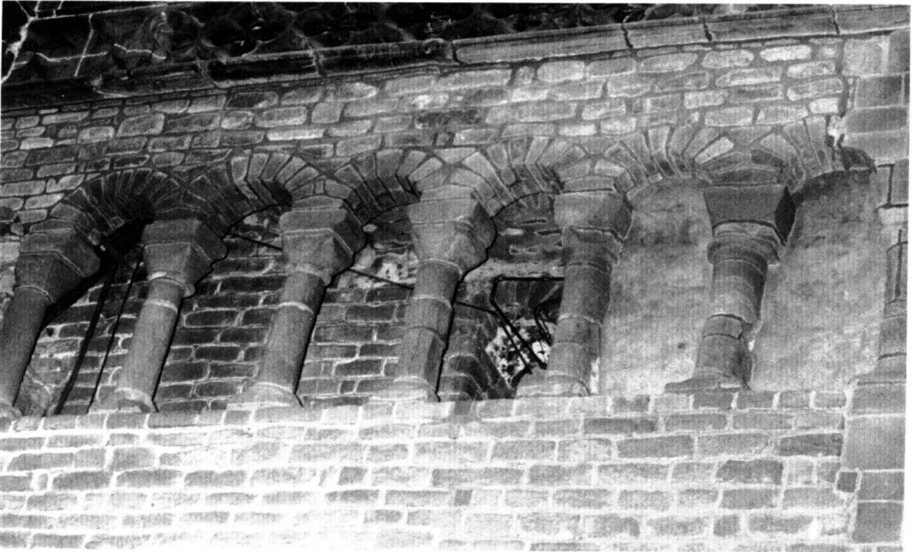
Fig 10.19 Part of the Norman fabric of Chester cathedral showing re-used legionary barrack veranda colonnade capitals (first and second from the right) and probably also re-used column drums and petit appareil
