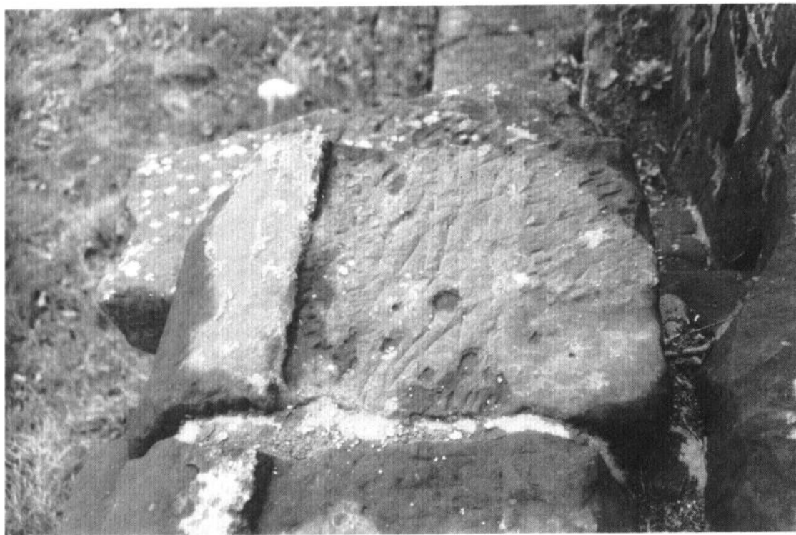
Fig 10.12 Detail of the cornice and parapet rebate-structure restored west of the North Gate, Chester. Note the rebate-block with tooling to suggest the former existence of a traverse at that point
