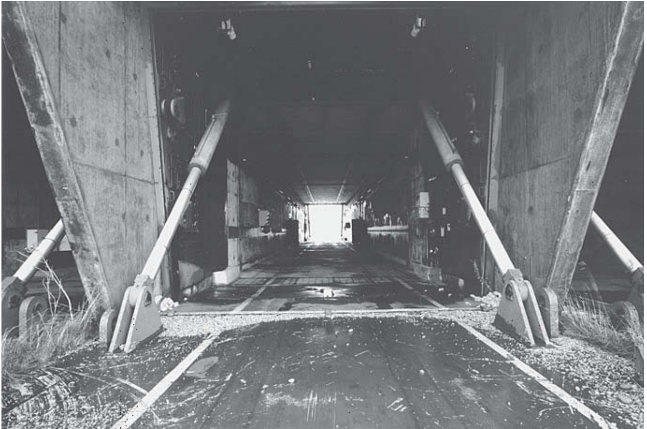
Figure 31 Former RAF Greenham Common, West Berkshire. The draw-bridge like door of one of the shelters used to house the cruise missile launchers during the 1980s (© English Heritage, AA000532)
