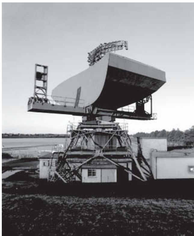
Figure 1 RAF Neatishead, Norfolk. Early 1960s Type 84 radar – this is the last surviving large fixed Cold War radar in England (© English Heritage, AA98/05747)
