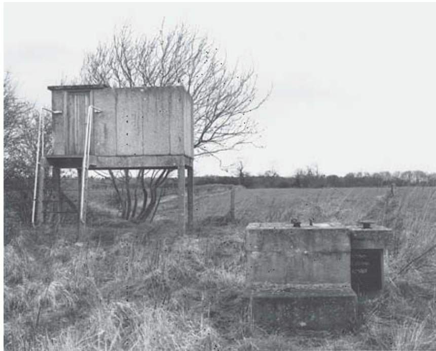
Figure 4 A Royal Observer Corps post at Watton, Norfolk. To the rear is the early 1950s raised Orlit post for the visual plotting of aircraft movements. In the foreground is the entrance to the late 1950s underground monitoring post, which was designed to detect and monitor the results of any nuclear attack on the country (© Crown copyright. NMR BB98/30036)
