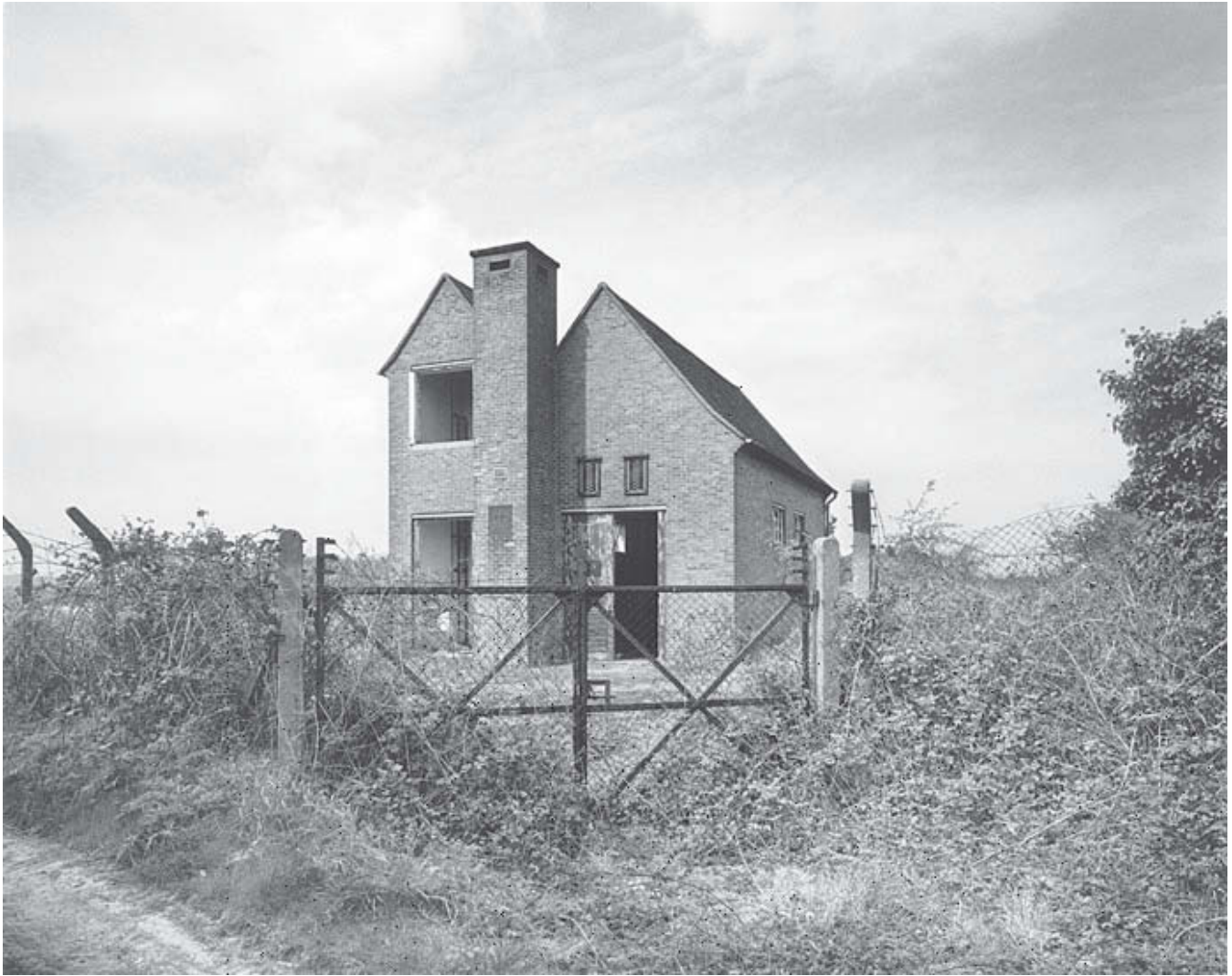
Figure 34 Kelvedon Hatch, Essex. Many of the surface structures associated with the early 1950s Rotor radar programme were constructed in a local vernacular style, such as this generator building with its chapel-like appearance. Such designs offered a degree of camouflage, but may also reflect the continuation of pre-war concerns about the intrusion of RAF facilities in the rural landscape (© Crown Copyright. NMR, AA00/01060)
