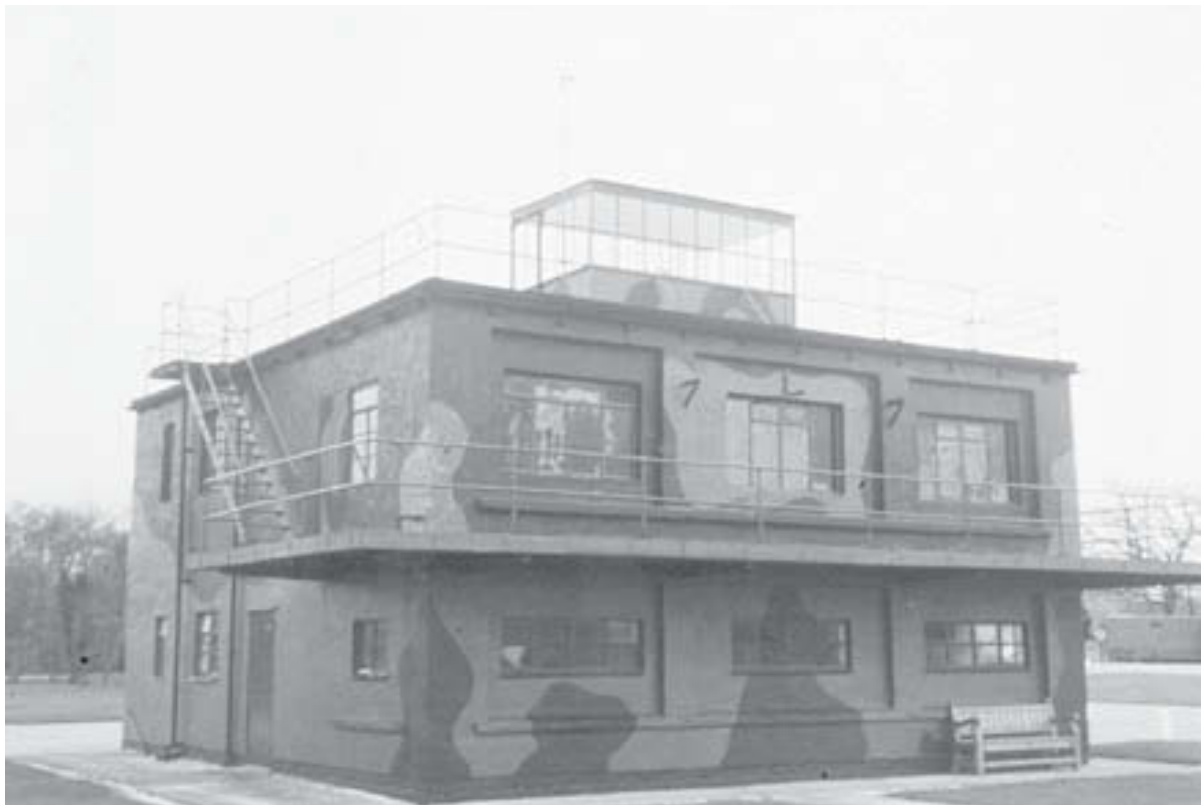
Figure 29 The control tower at East Kirkby, Lincolnshire. This control tower has been restored as the centrepiece of a museum that commemorates the history of this airfield, opened in 1943 in support of Bomber Command's offensive. It was one of 160 Watch Office for All Commands control tower buildings constructed, of which 82 survive (Photograph: Jeremy Lake)
