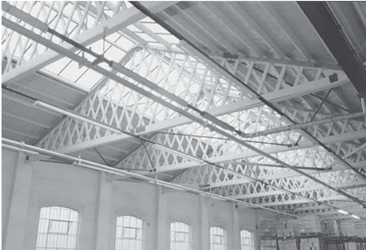
Figure 10 The Belfast truss roof of a surviving building at the former Handley Page factory at Chadderton, Manchester (Photograph: Roger J C Thomas)
