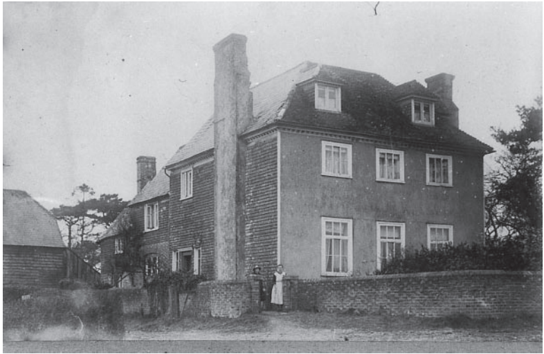
Fig. 3. The Upper or New Lodge. This hunting lodge provided accommodation for the Dorset family when they visited the Broyle and also, to the rear, a residence for one of the two keepers. After enclosure this was used as a pesthouse and then as a farmhouse. Today it belongs to the Raystede animal sanctuary.
