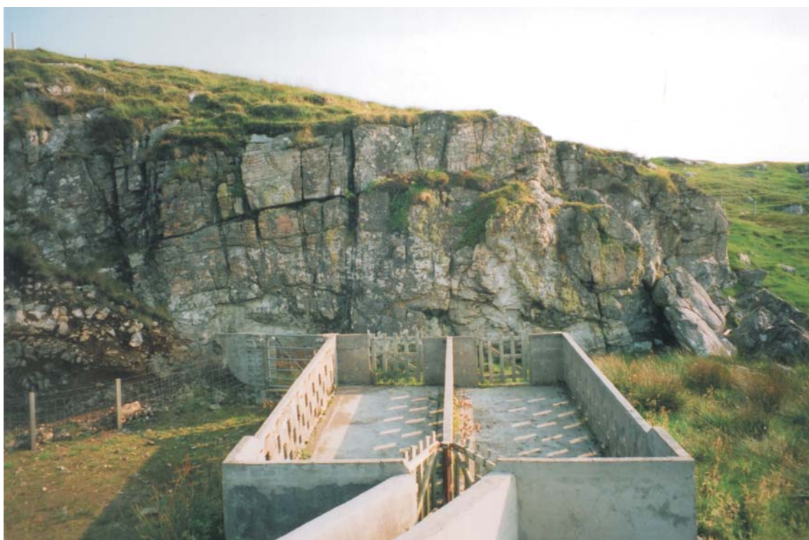
Illus 2 View of the Cnoc Dubh rock face and vein, from the north-west.
