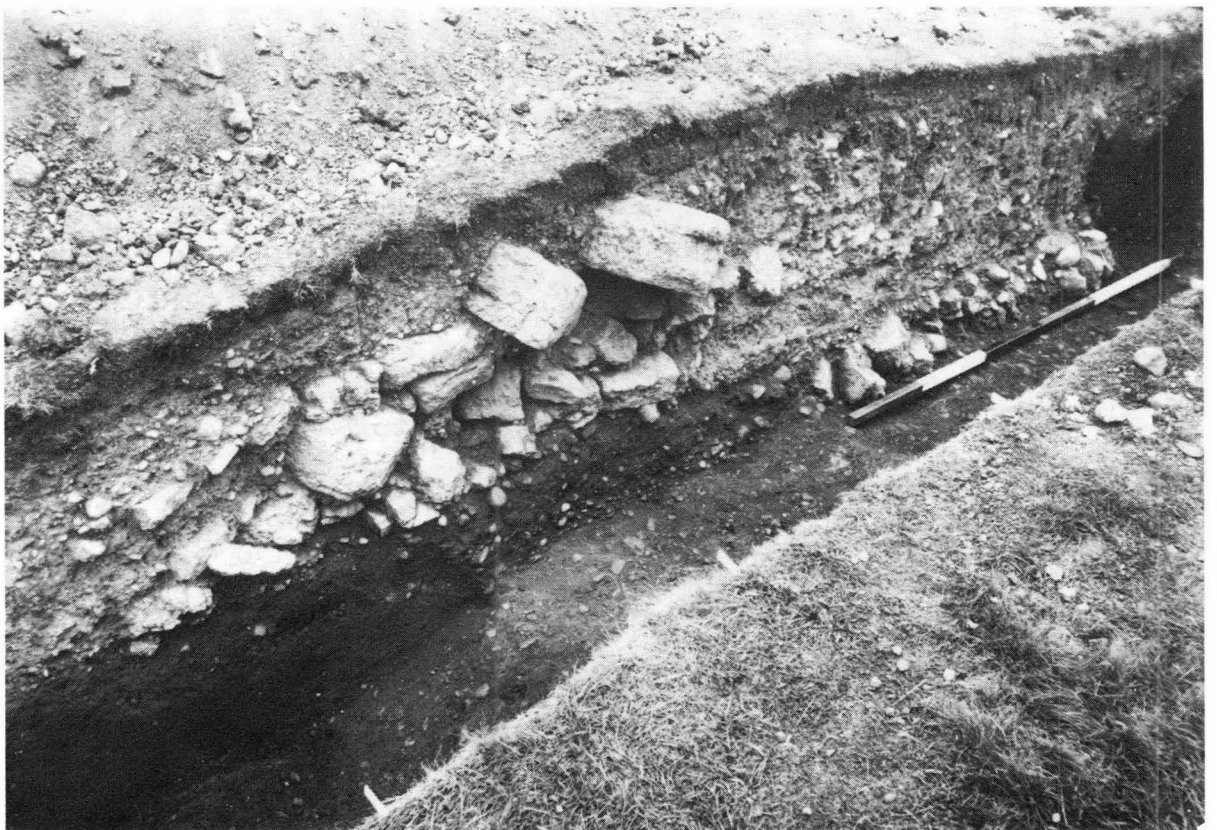
Pl. VI B Wall footing on south-east side of the fortress (right), with tumbled stonework (left) overlying the berm (p. 67).
