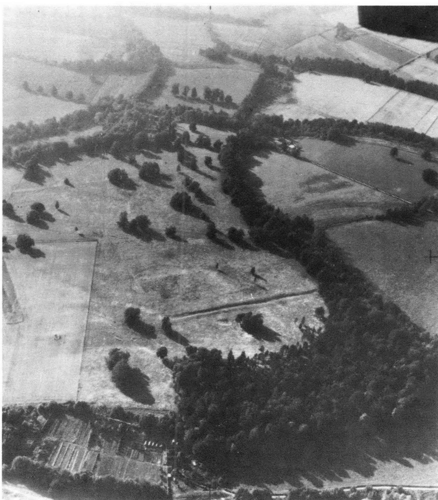
(Photo: Cambridge University Collection (XB 58), July 1958. Ministry of Defence, Crown copyright reserved) Pl. IV Inchtuthil, oblique view looking north across the fortress. The low sunlight picks out the earthworks.
