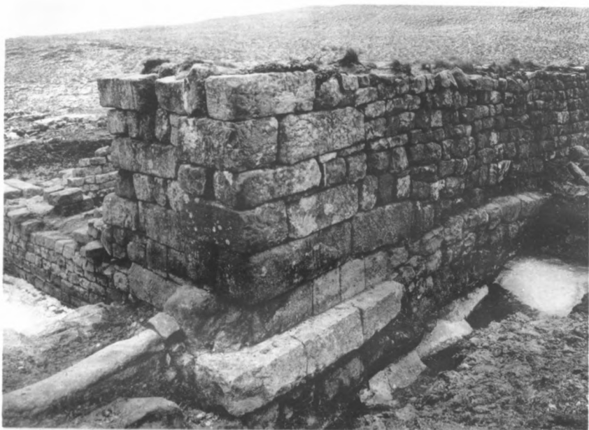
Fig. 2. KNAG BURN GATEWAY, DETAIL OF WEST SIDE FROM NORTH.
