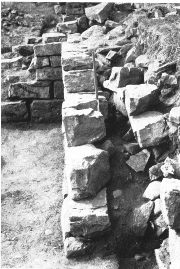
1. Turret 29a, east wing wall with narrow wall built on
