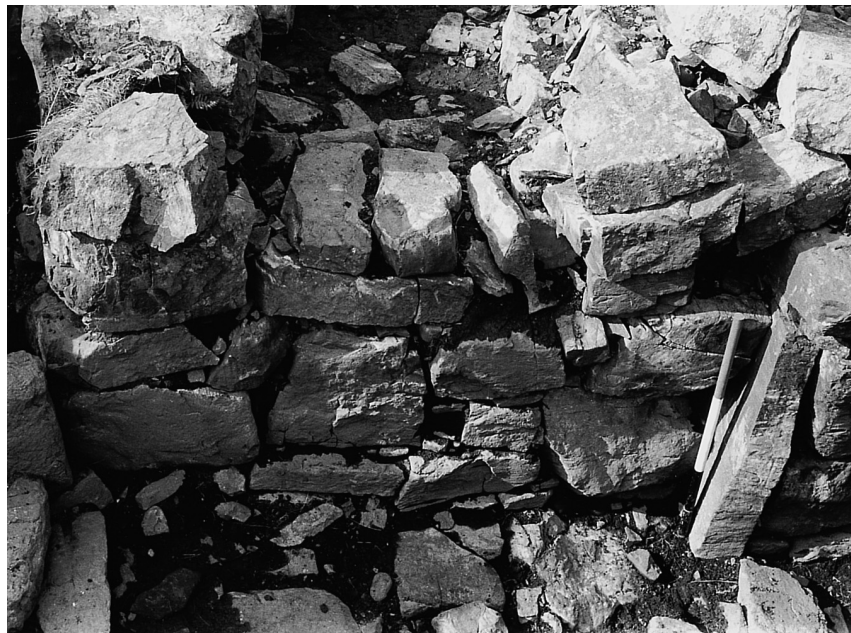
Illus 12 The raised sill of the entrance to the guard cell, seen from across the main passage; the secondary steps are still in position on the left
