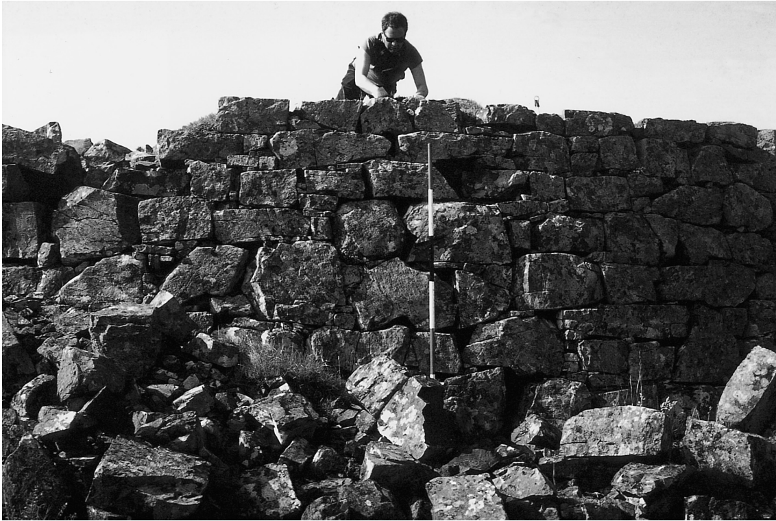
ILLUS 4 Close-up of dun wall before excavation
